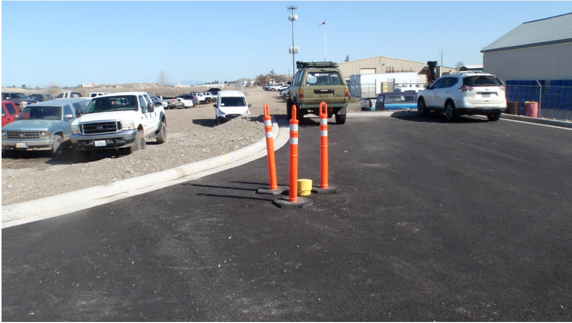
Photo #4: Monitoring well MW-4; to be converted to a traffic-rated flush mount.
