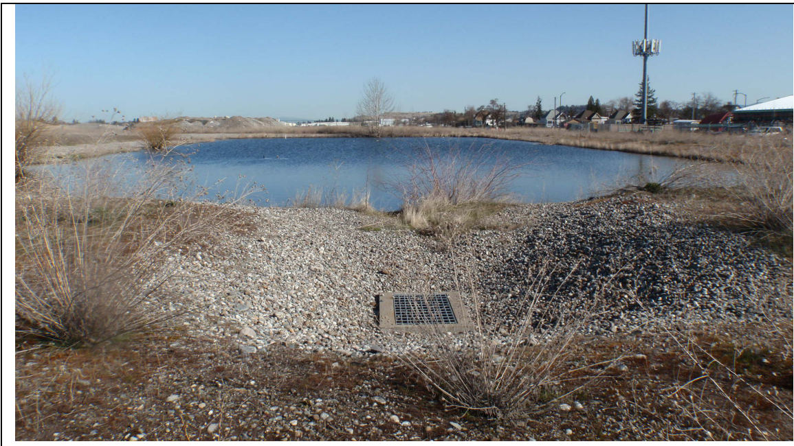
Photo #2: Stormwater retention pond and overflow sump.
