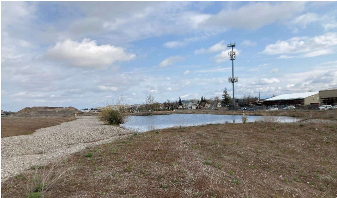
Photo #6: Stormwater retention pond and inlet channel.
