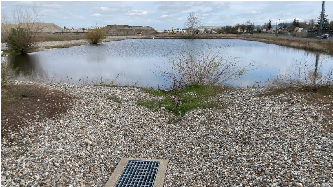
Photo #4: Stormwater retention pond and overflow sump.
