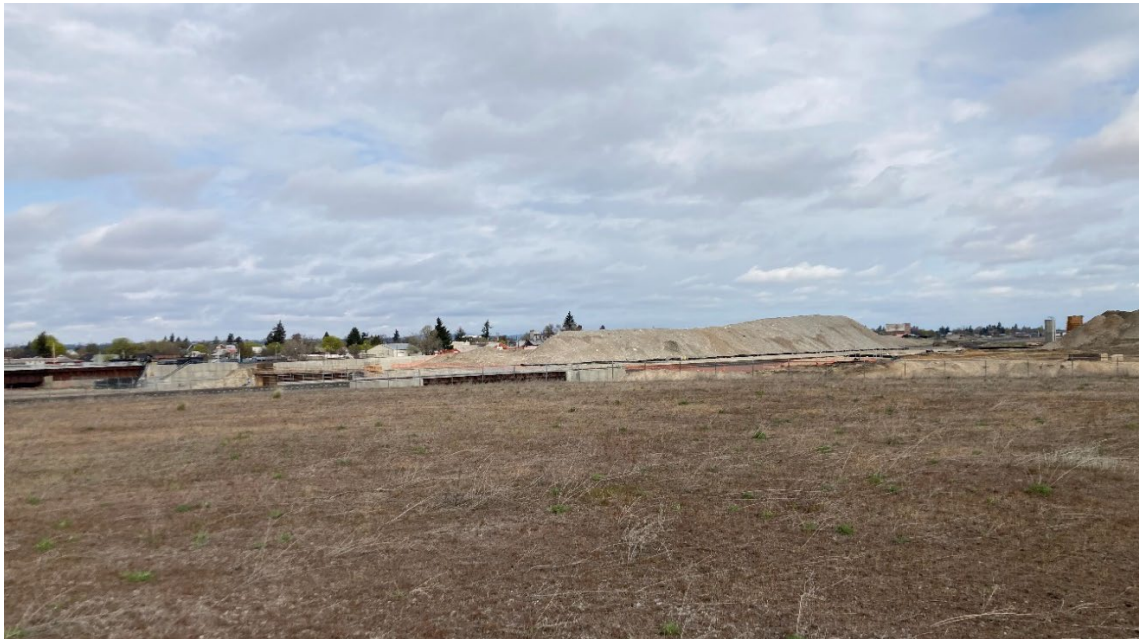
Photo #8: Ongoing WSDOT work adjacent to the Site.
