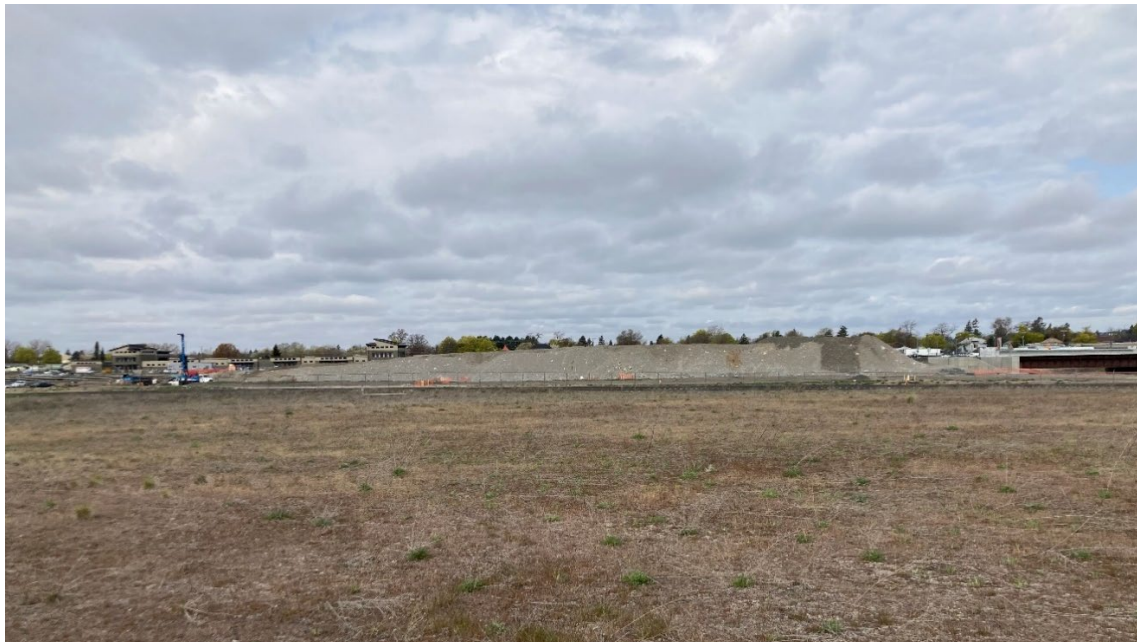
Photo #9: Ongoing WSDOT work adjacent to the Site.
