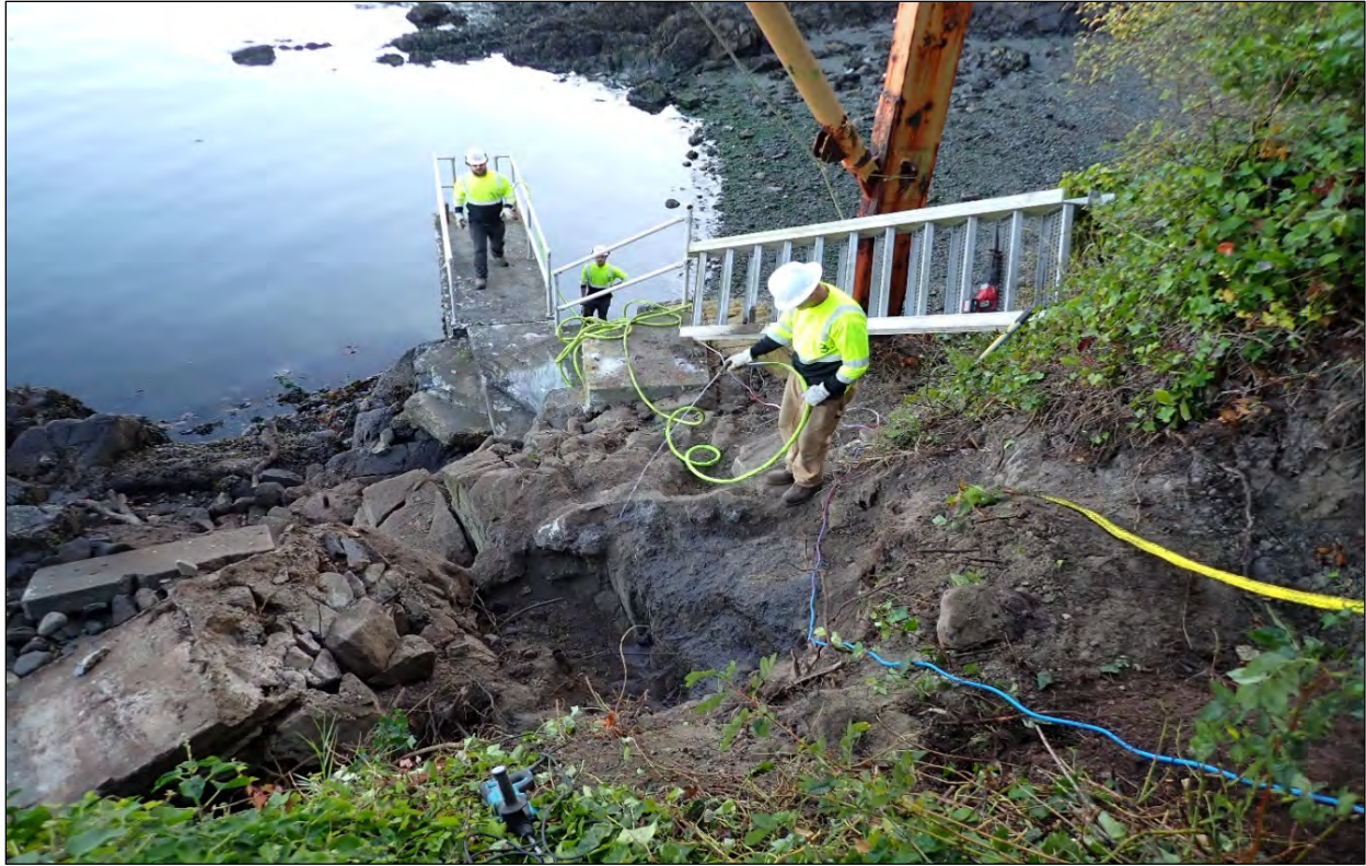
Figure 7. Hosing off the bedrock and exposing for drilling at the staircase. View to the north.
