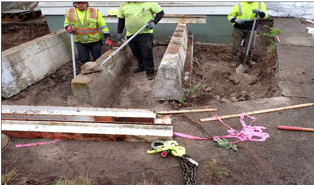
Figure 17. Hand-excavation in between water tank concrete support on the northeast corner of Duplex. View to the west.
