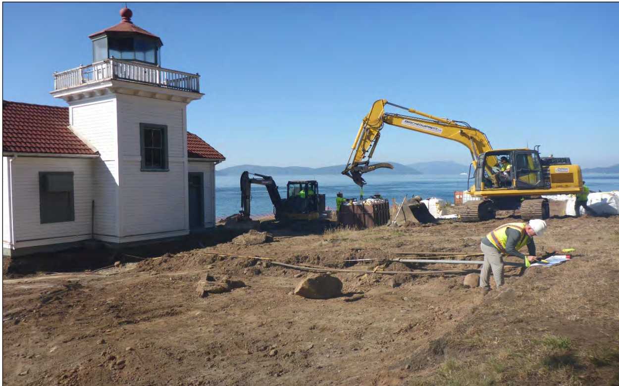
Figure 5. Arcadis personnel collecting soil samples for testing. View northwest.
