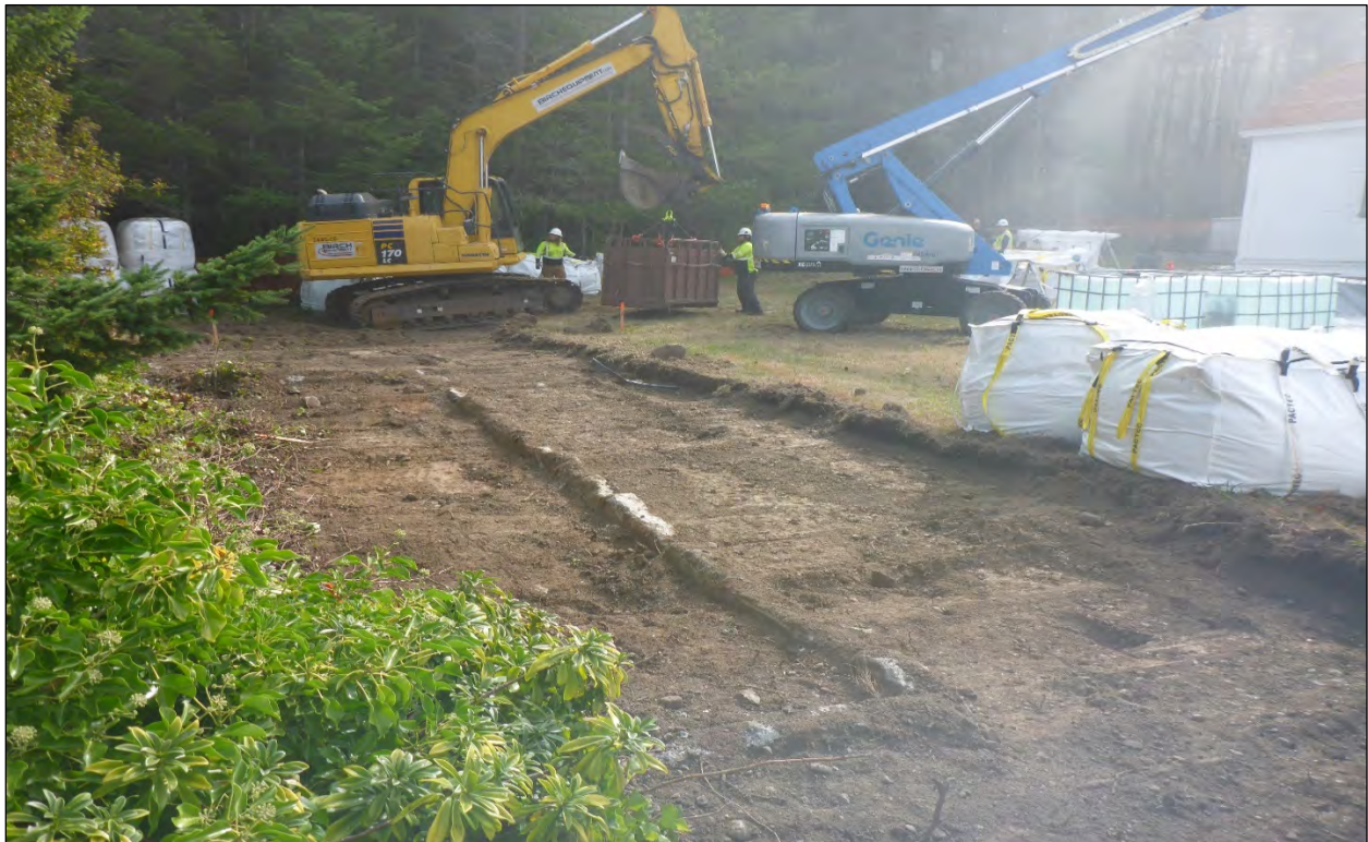
Figure 10. Area G excavation exposing concrete wall foundation from the former Officer-in-Charge Quarters. View to the southeast.
