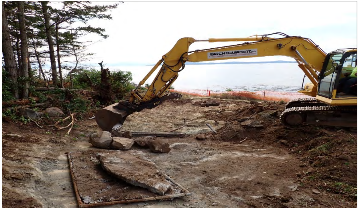
Figure 20. Overview of Area K east-half. Operator removing concrete/fence slab. View to the southwest.
