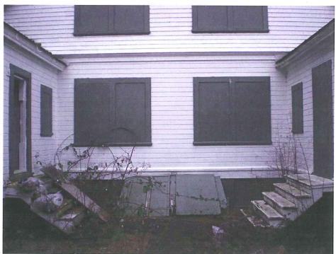
**USCG – Burrows Island Light Station:** *Photo* 10 – View of backside side of Duplex showing deteriorating stairs, opened doors and scattered debris.
