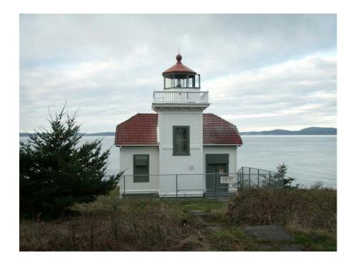
The light house has virtually no shade, and the top coast curing process was relatively quick with full sun and wind exposure. It was not necessary to wait 24 hours before applying the second coat to this building.
