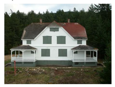
The Duplex had higher moisture content in the wood than the other buildings. The building location has become relatively "forested." Prior to this project the Duplex was almost completely covered with vines and foliage, preventing sun from reaching the building surfaces. Removal of growth within 10 feet of the building was still inadequate to allow sufficient sun and wind for natural paint curing. As remedy, propane "blast" heaters were used to expedite drying.
