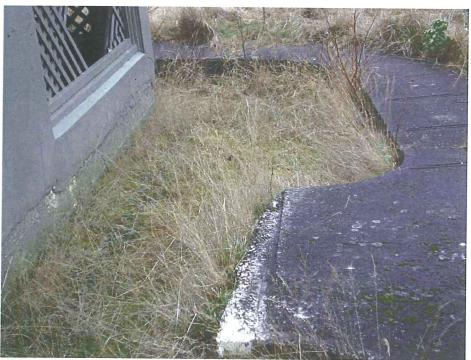
**USCG – Burrows Island Light Station:** *Photo 12* – View of depression inside the concrete foot path of Duplex where previous removal action has taken place. The excavated area has since been overgrown with grass and shrubs.
