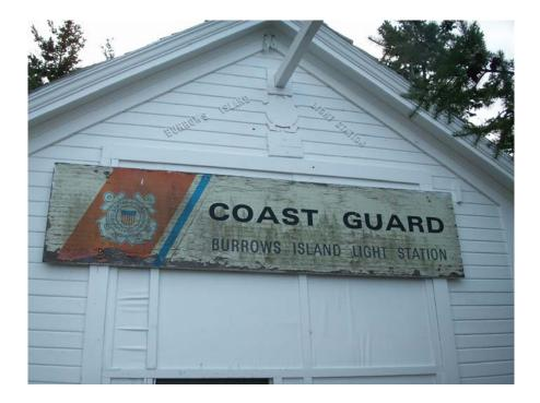
The Coast Guard sign over the Boat House was completely removed and stored during the painting process and was reinstalled following completion of that structure's painting. Due to shade and high humidity (>70%) the curing process took longer than expected in some areas, but no intervention was needed
