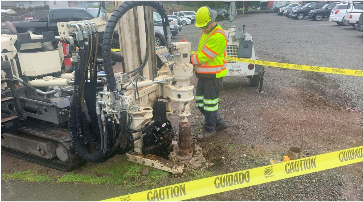
Photo 2: Each boring was over drilled using 8-inch outside diameter augers to total depth and then backfilled with hydrated bentonite chips. The above photo shows drilling out GP-3.
