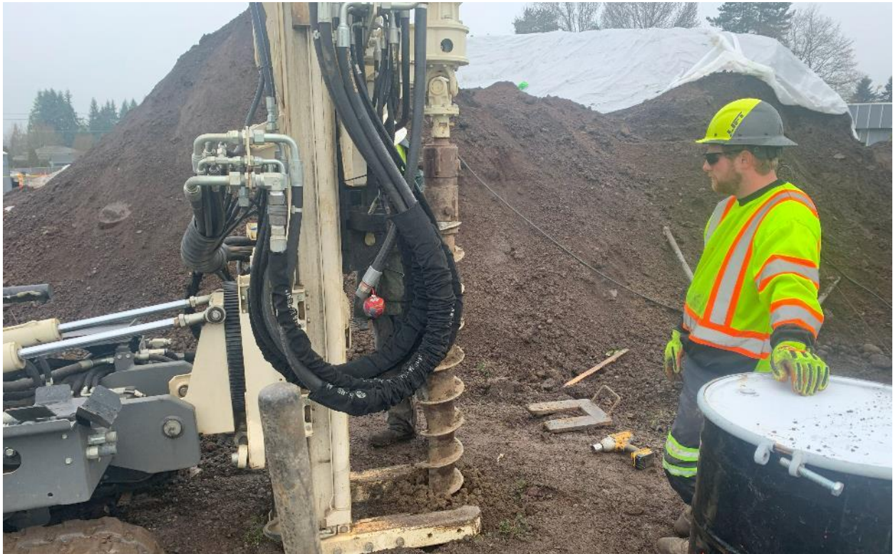
Photo 6: View of over drilling GP-05.
