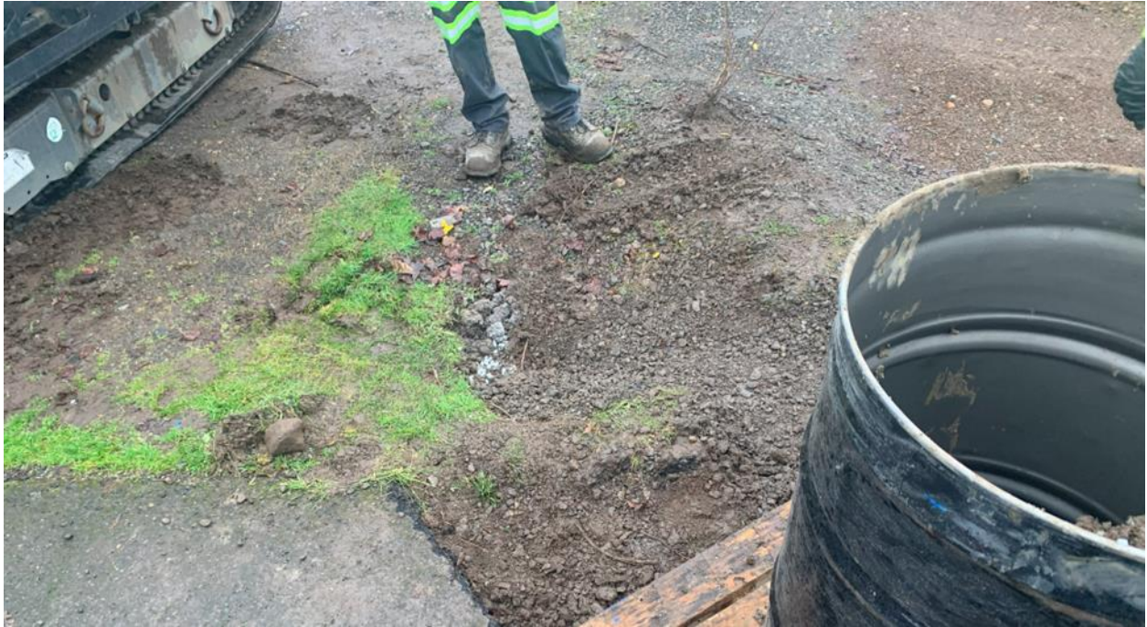
Photo 3: View of GP-3 when finished. Backfilled with bentonite chips and then gravel over the surface. Note all drill cuttings were placed into 55-gallon, labeled drums.
