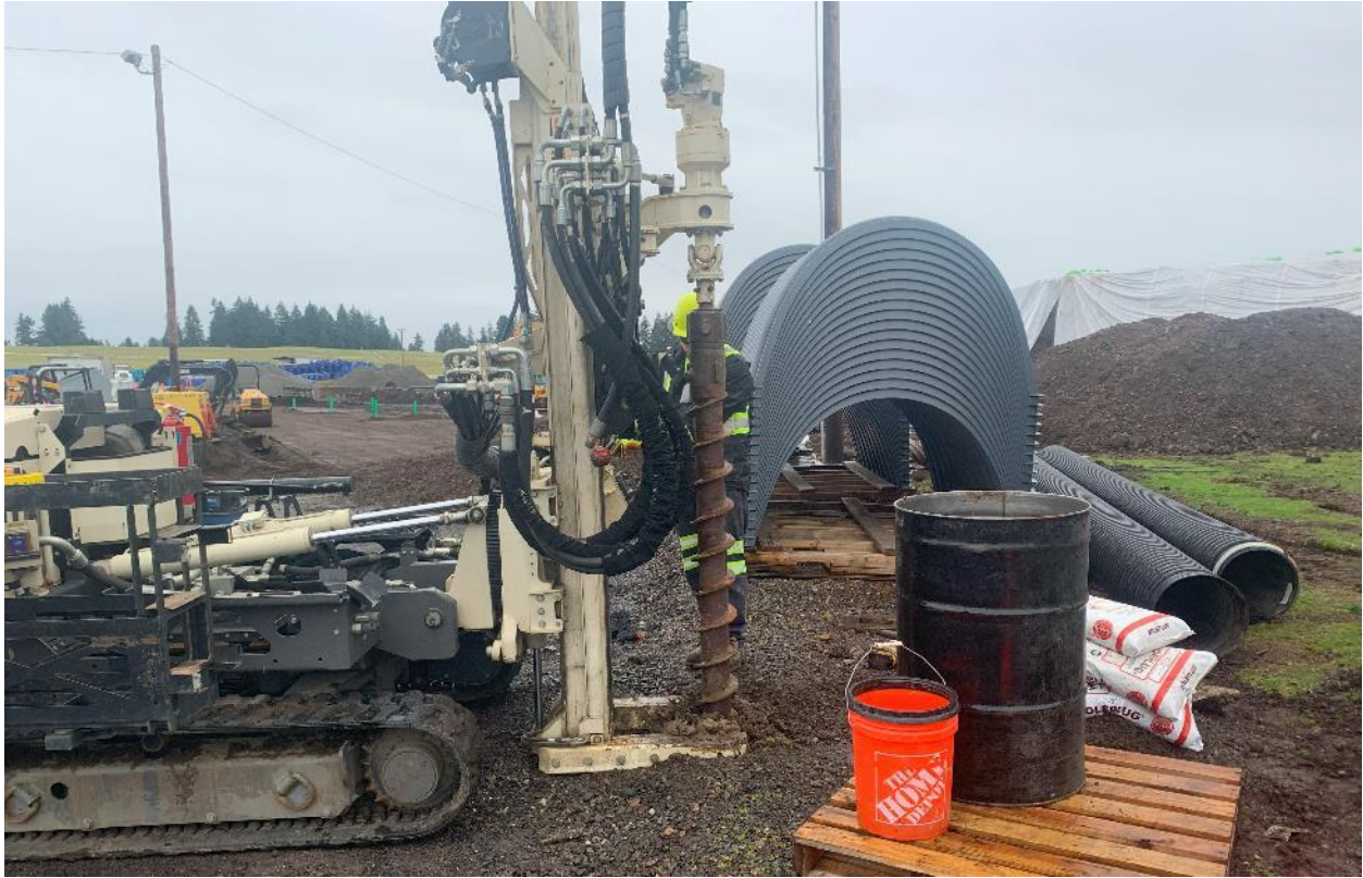
Photo 5: View of drill rig setup on GP-4, getting ready to over drill the boring to total depth (16.5 ft).
