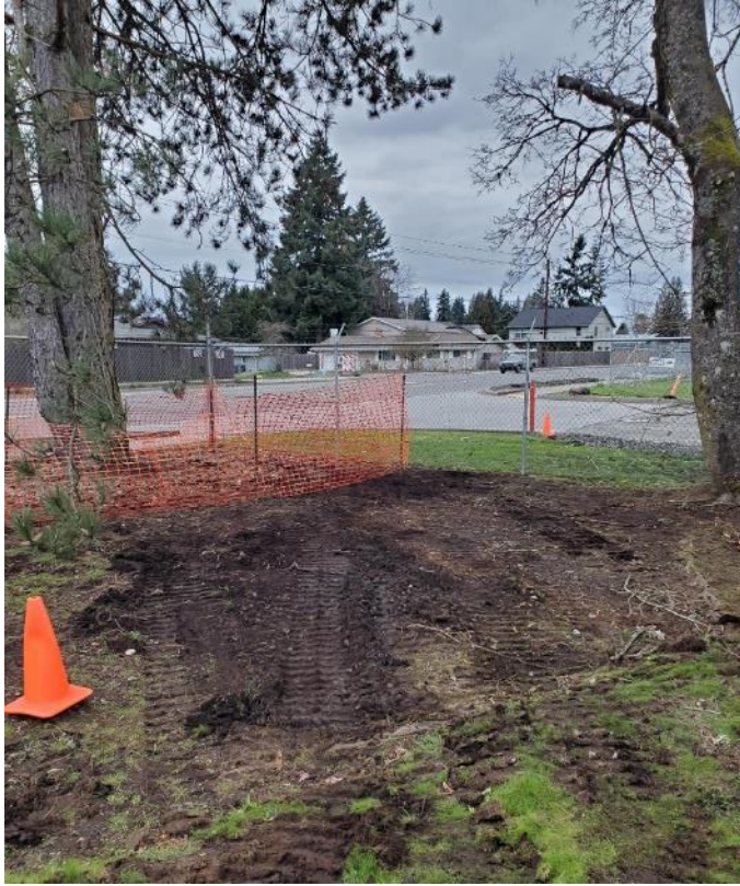
Photo 11: View of the area following well decommissioning.
