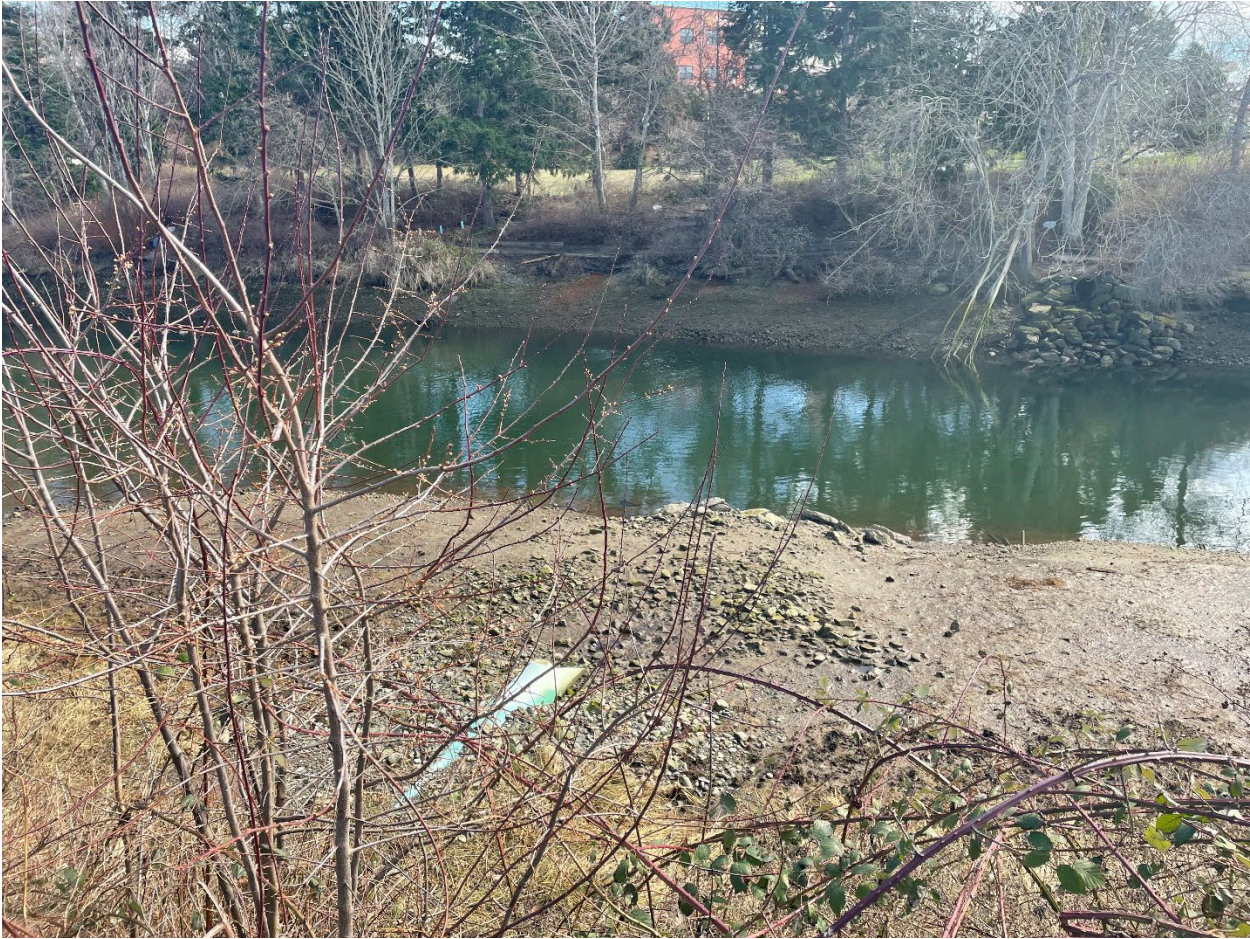
Photo 7: Looking southeast at Whatcom Creek channel with decommissioned Astor Street outfall.
