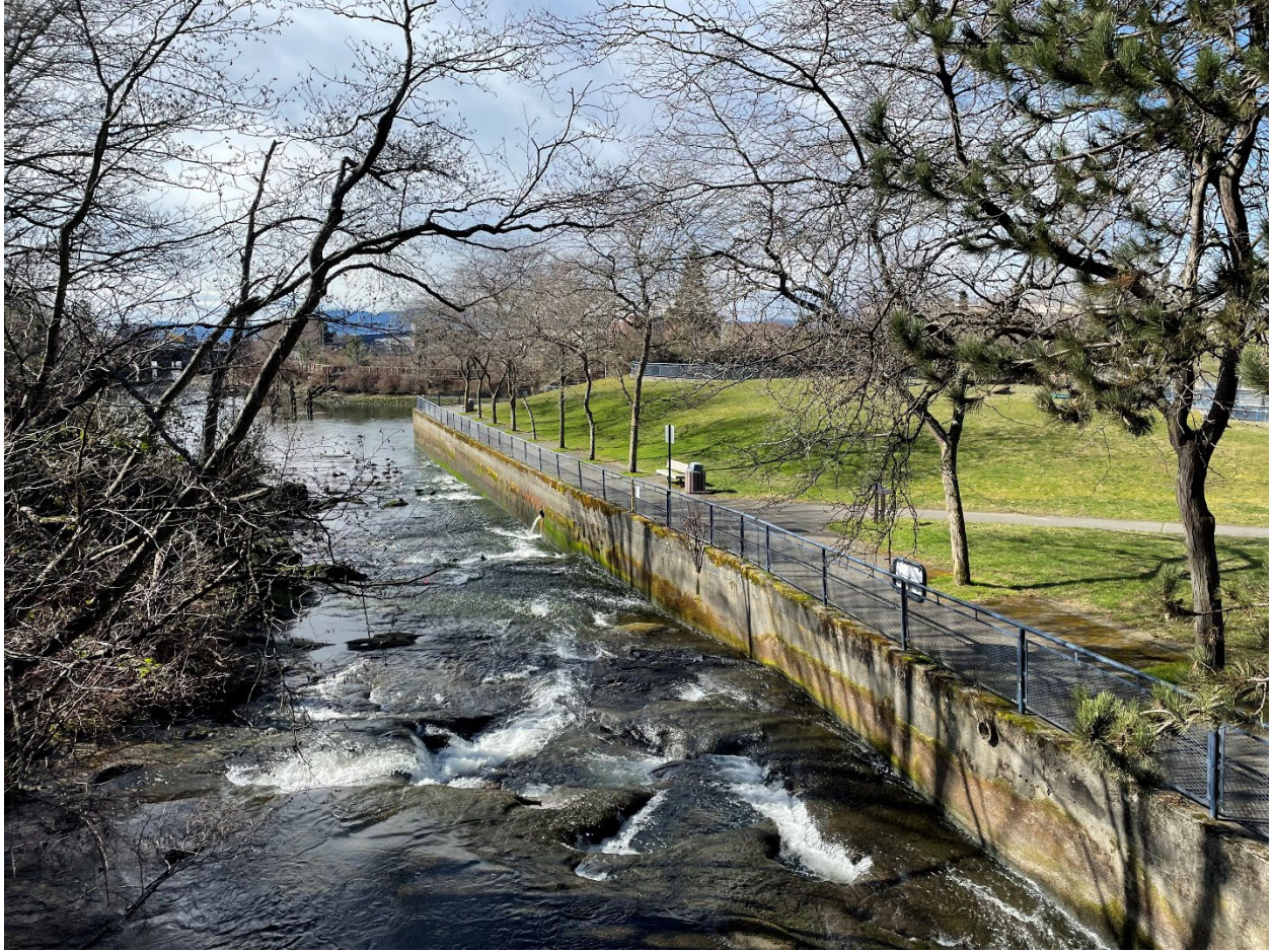
Photo 5: Looking southwest at upper Maritime Heritage Park and Whatcom Creek channel northeast bank and former Holly Street Landfill northern lobe.
