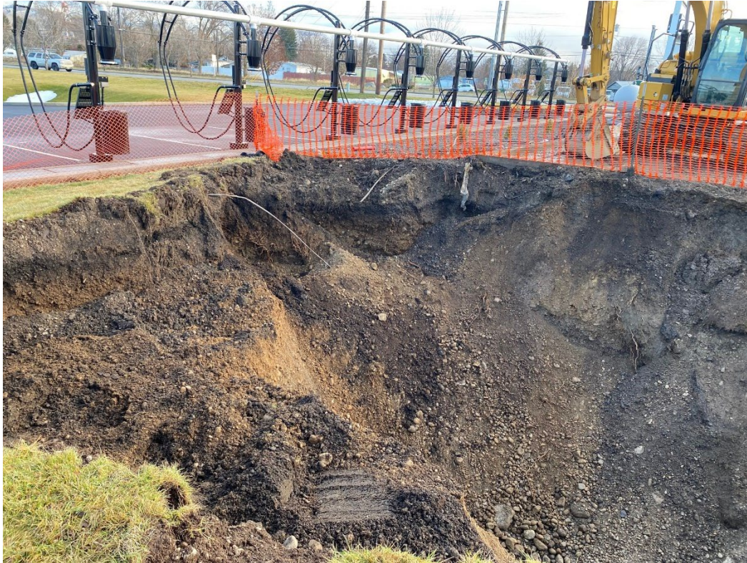
Photo shows final excavation, taken facing a southeasterly direction.
