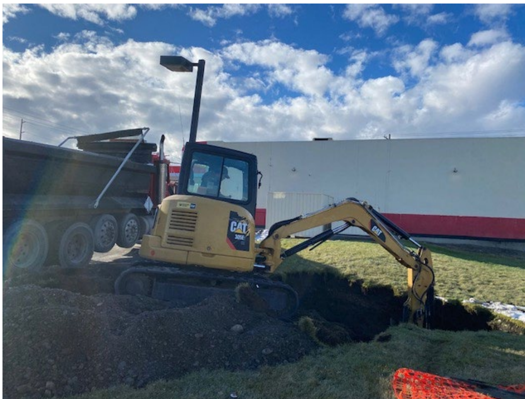
Photo shows excavation process, taken facing a westerly direction.
