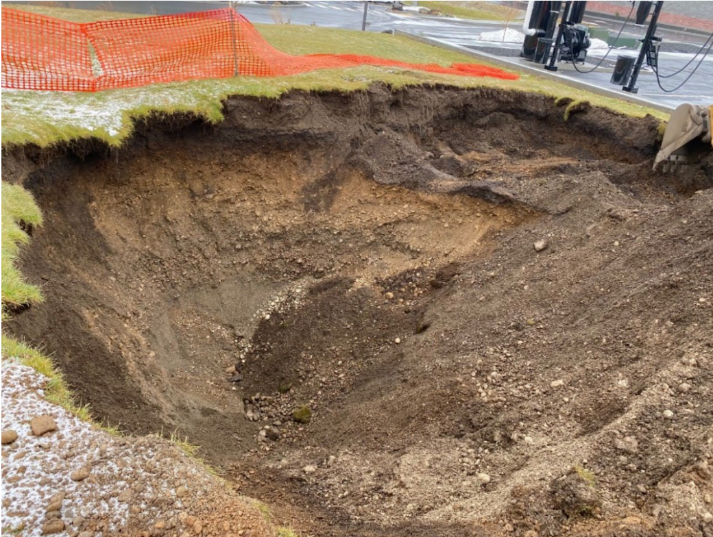
Photo shows excavation, taken facing a northeasterly direction.
