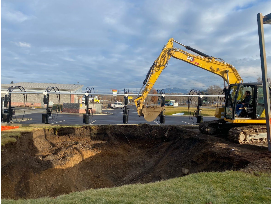
Photo shows final excavation process, taken facing an easterly direction.
