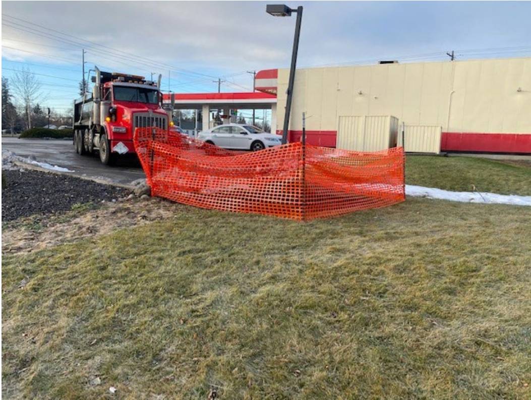
Photo shows excavation upon second trip, facing a southwesterly direction.
