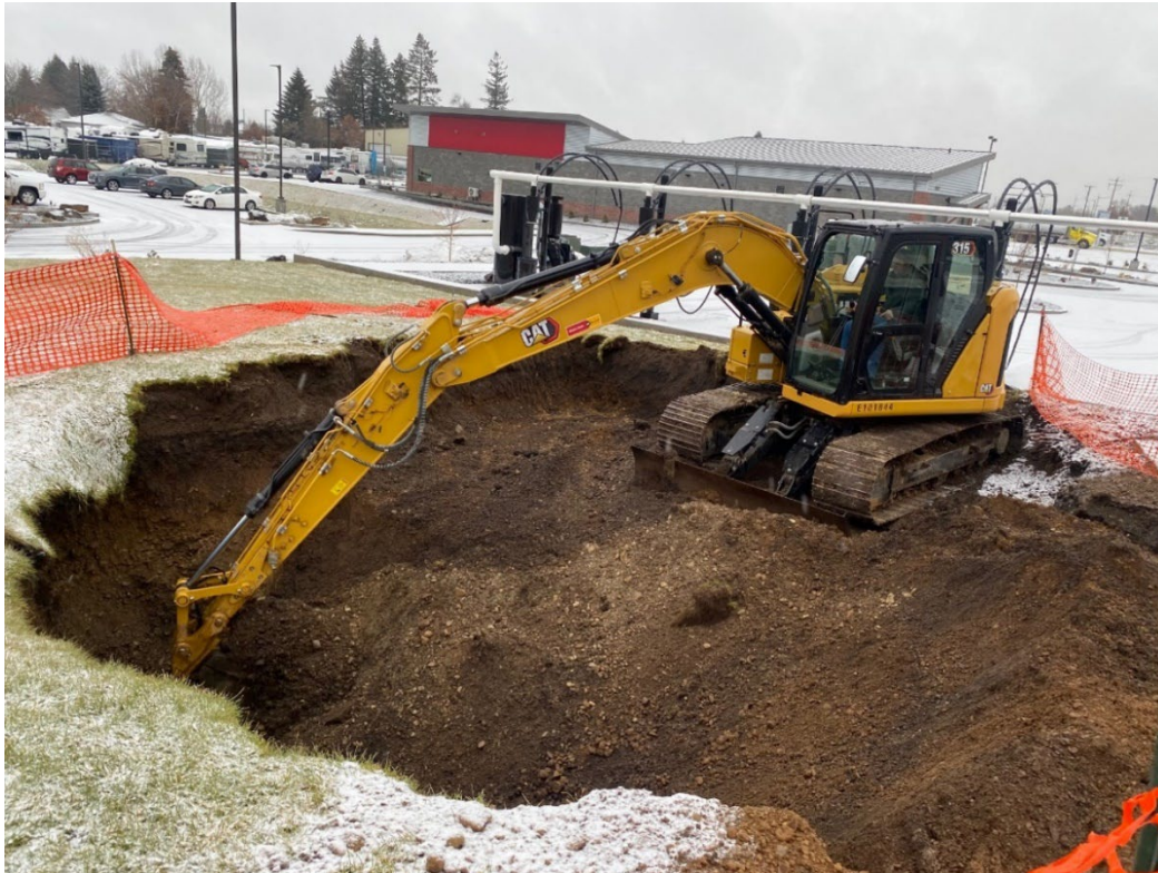
Photo shows excavation process, taken facing a northeasterly direction.
