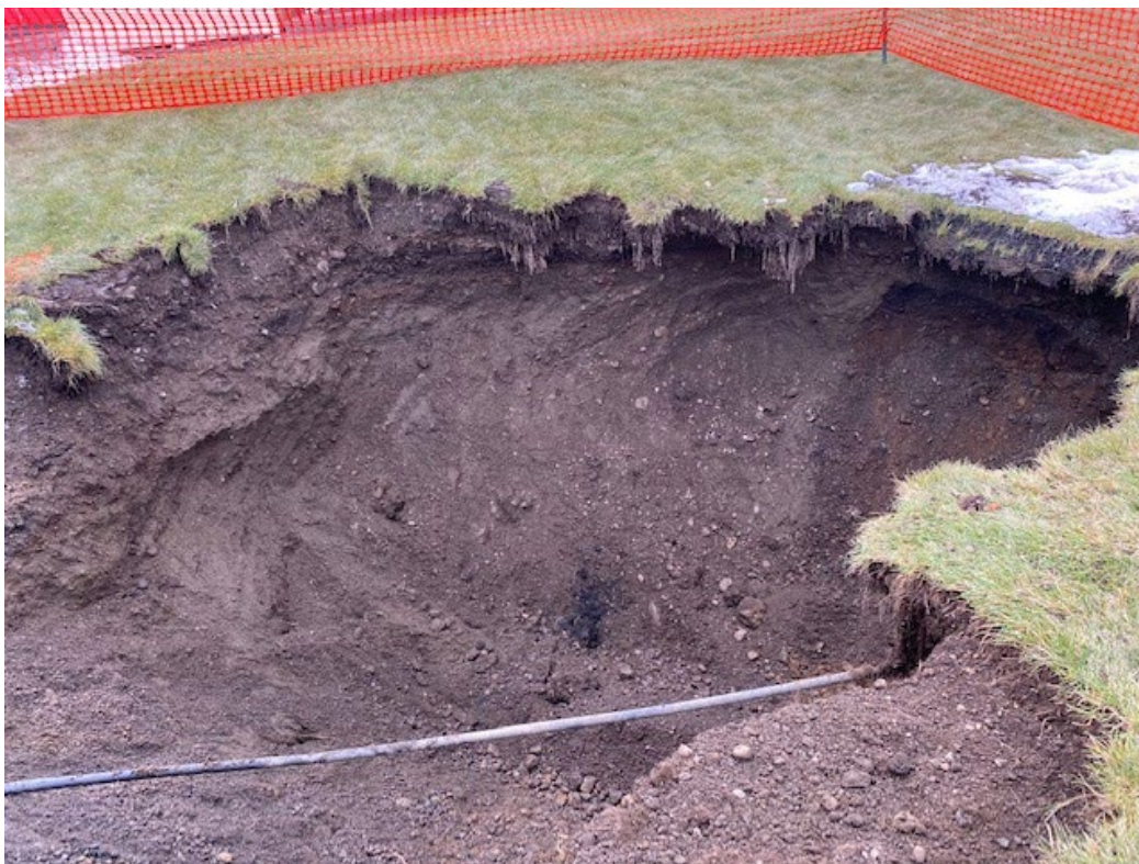
Photo shows excavation, taken facing a westerly direction.
