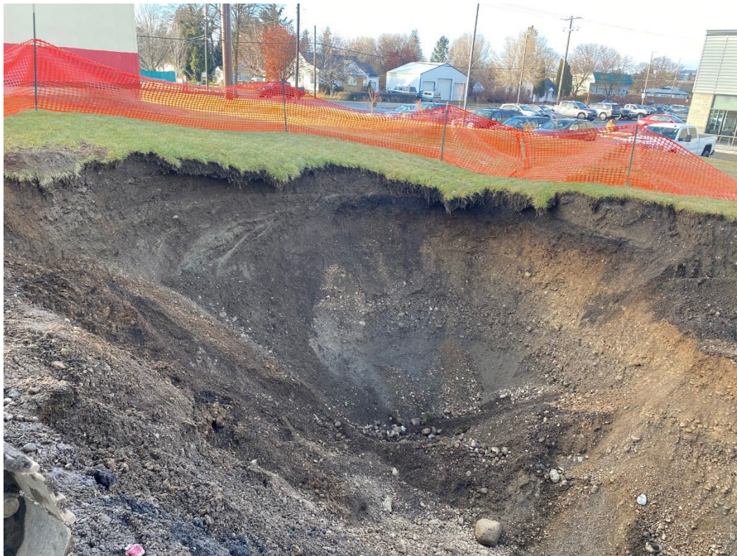
Photo shows final excavation, taken facing a westerly direction.
