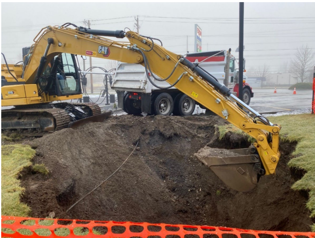
Photo shows excavation process, taken facing a southerly direction.
