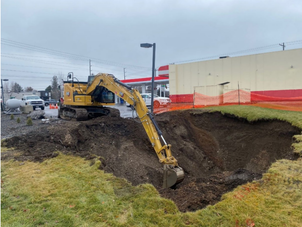
Photo shows final excavation process, taken facing a southwesterly direction.
