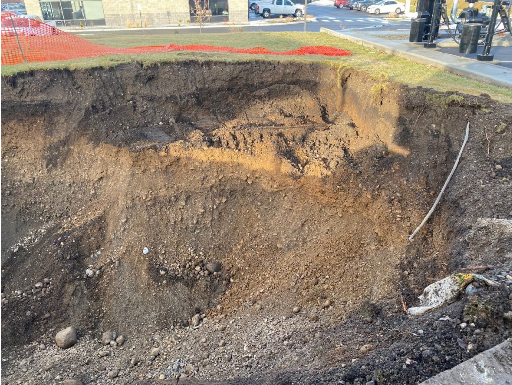
Photo shows final excavation, taken facing a northely direction.
