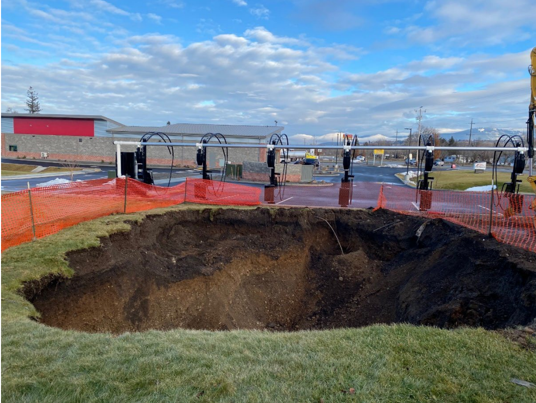
Photo shows final excavation, taken facing an easterly direction.
