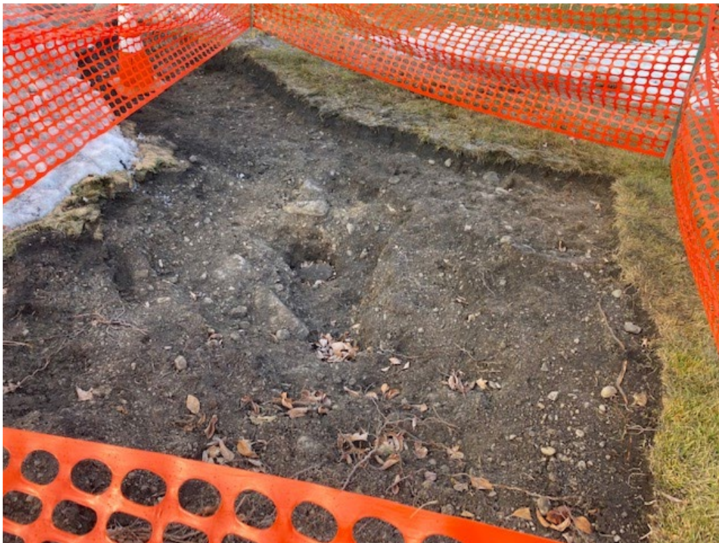
Photo shows excavation site, taken facing a westerly direction.
