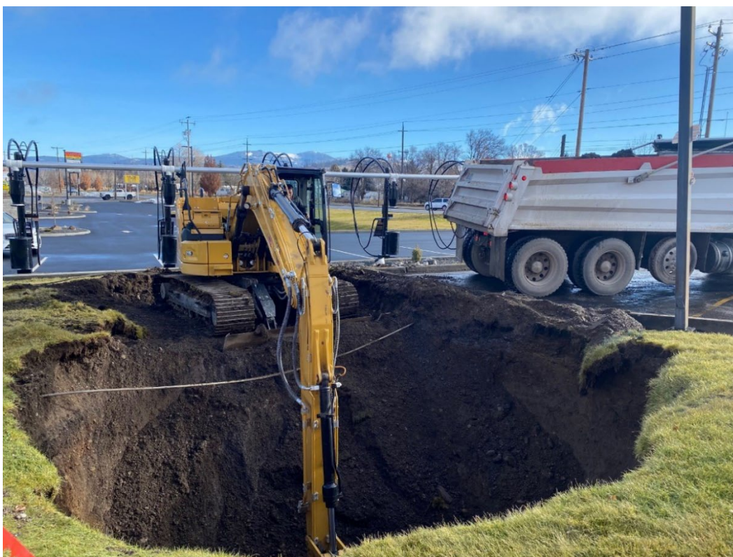
Photo shows excavation process, taken facing an easterly direction.
