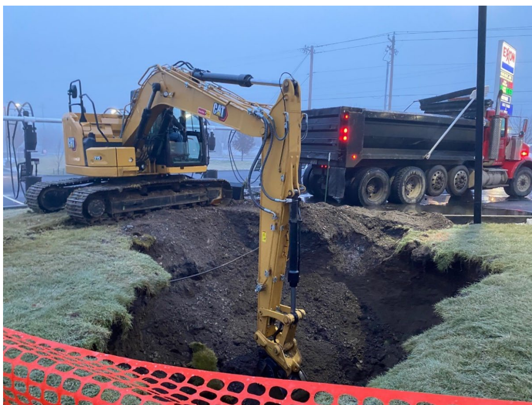
Photo shows excavation process, photo taken facing a southeasterly direction.
