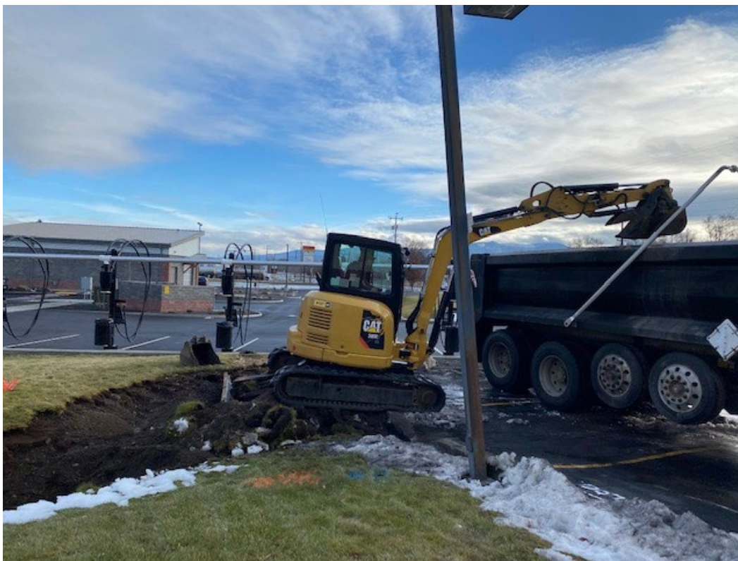
Photo shows excavation process, taken facing an easterly direction.
