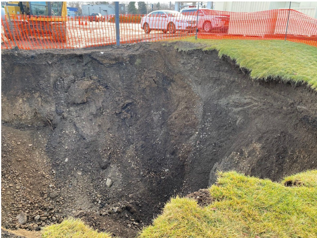
Photo shows final excavation, taken facing a southerly direction.
