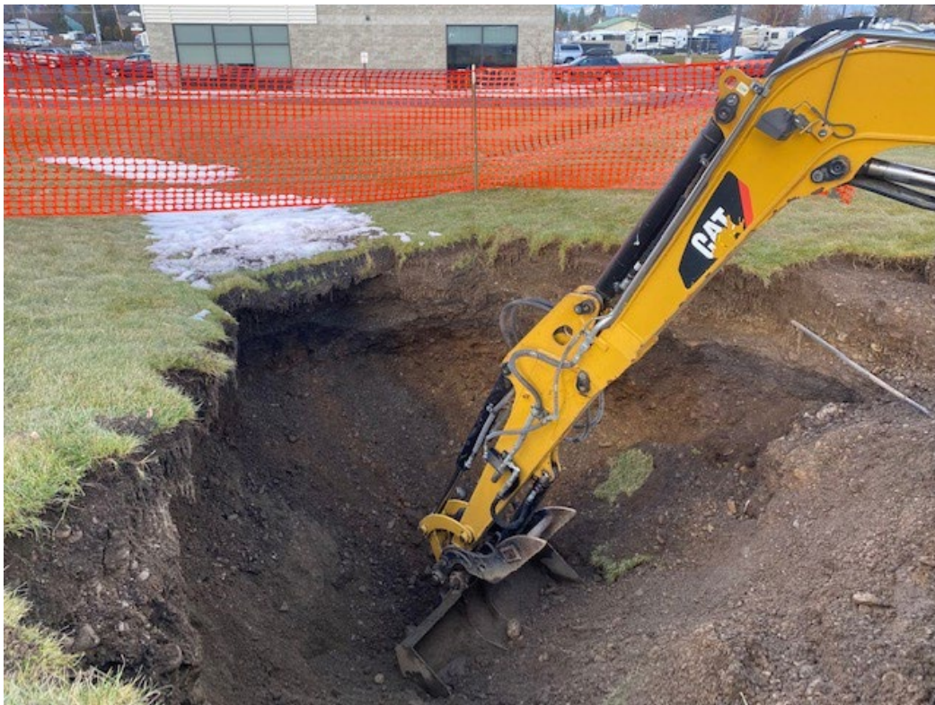
Photo shows excavation process, taken facing a northerly direction.
