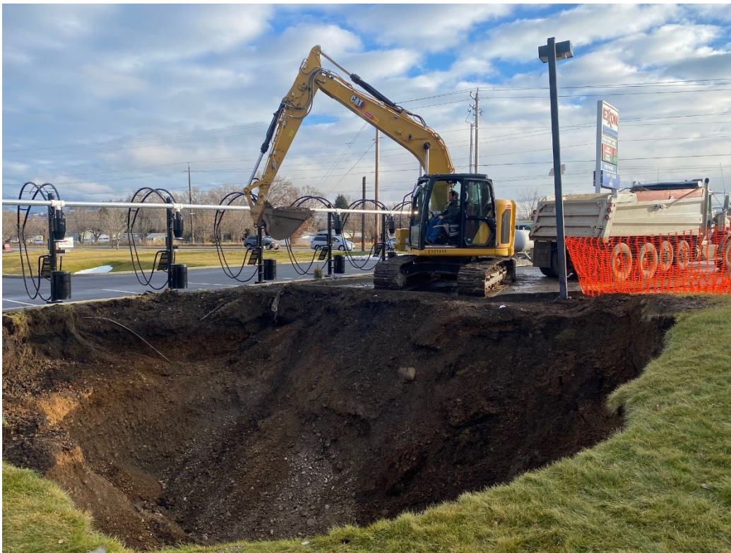
Photo shows final excavation process, taken facing a southerly direction.
