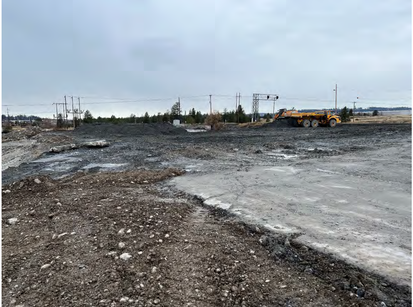
Photograph 1: UPRR property with dross stockpiled in loadout area.
