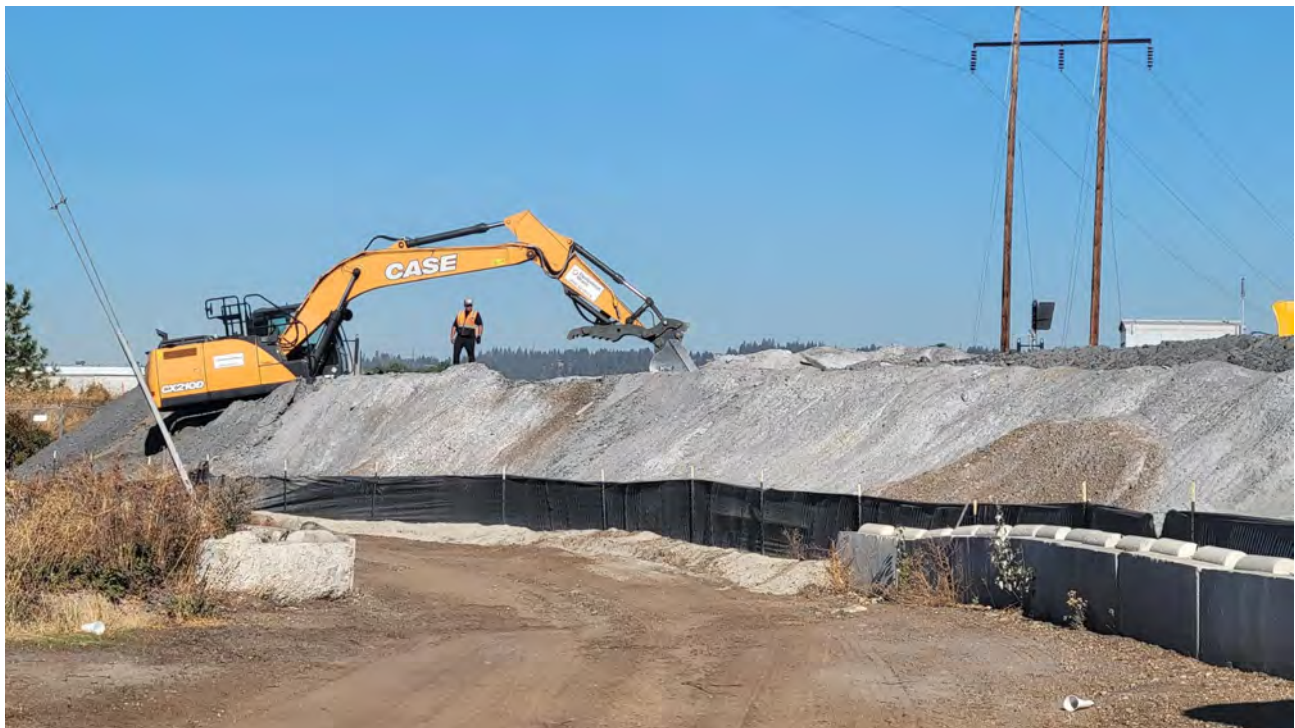
Photo 5. Excavator enters the dross pile under BPA wires.
