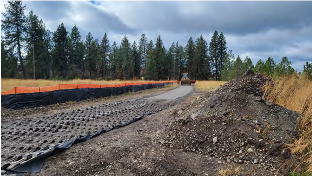
Photo 3. Gravel being added to haul road west of rumble strips.
