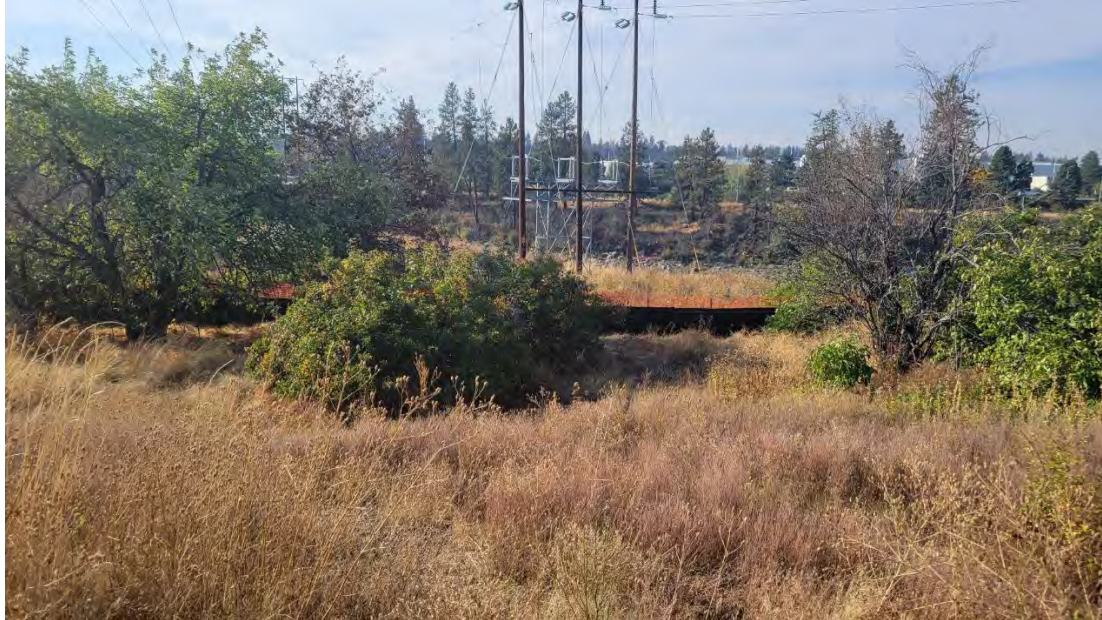
Photo 1. Silt/Construction fence installed thru grass on south boundary
