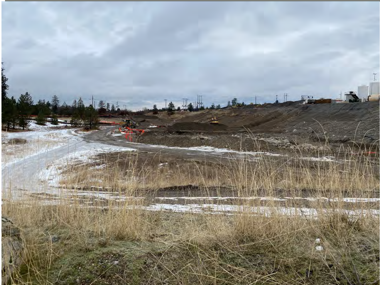
Photograph 2. Placing stockpile between Excavations 6 and 8 on UPRR slope.
