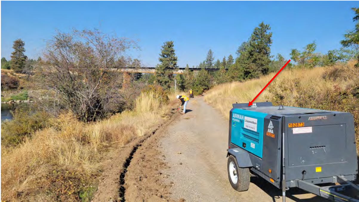
Photo 5. Trenching reaches road east of the river.
