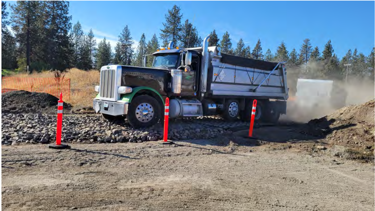
Photo 4. Truck and trailer crossing rumble strips and quarry spalls.
