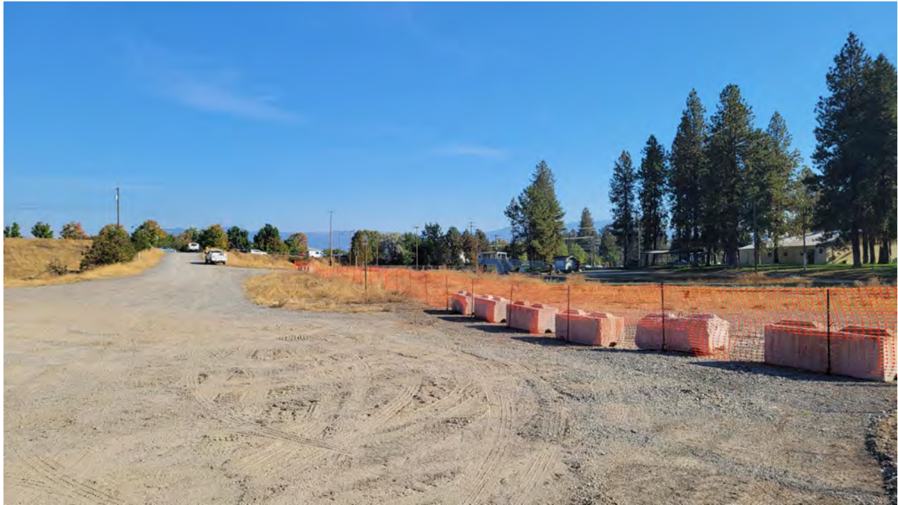
Photo 11. Construction fence from eastern access road to berm by trailer.
