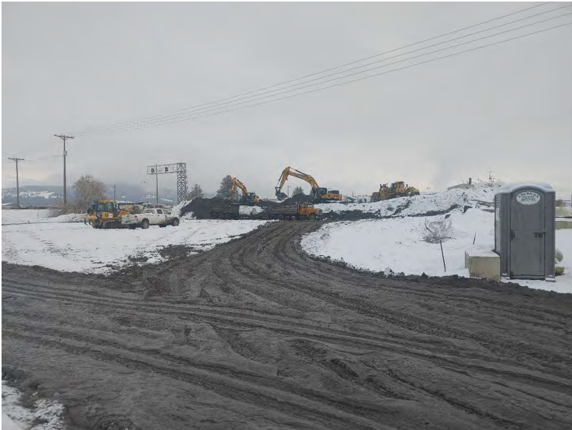
Photograph 1: Dross stockpile excavation and loading activities
