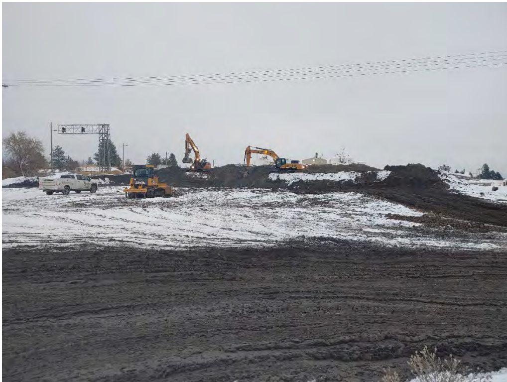
Photograph 4: Dross stockpile excavation activities.
