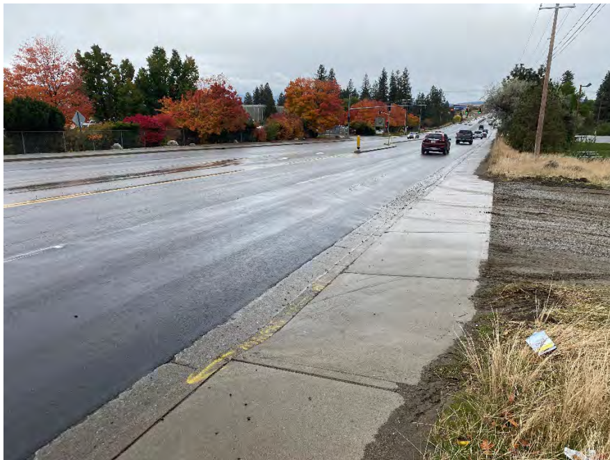
Photo 2. Track out on Sullivan minimal fines but gravel is being tracked out.
