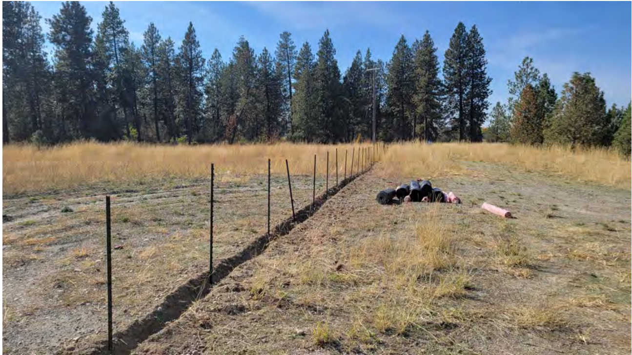
Photo 4. Posts for silt fence extending west from office trailer.
