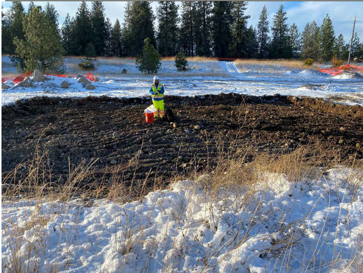
Photo 1. XRF sample location in 1-foot deep excavation.
