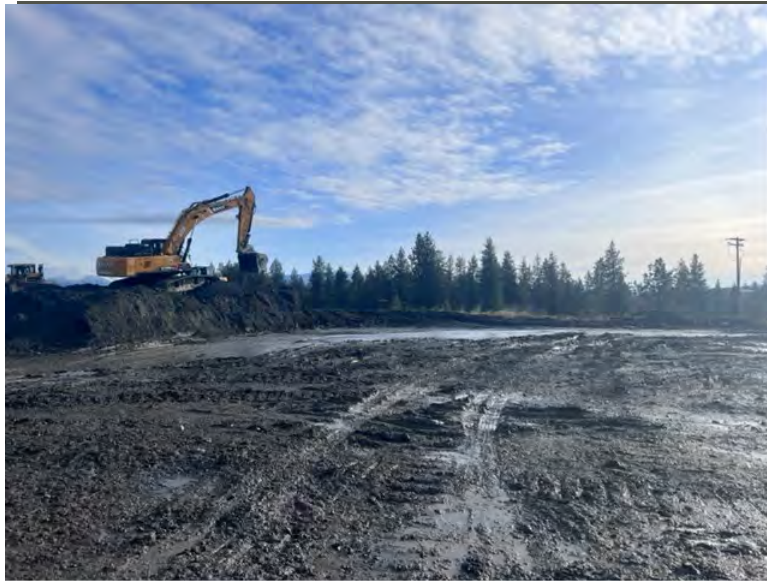
Photograph 2: Roadway @ Dross Pile
