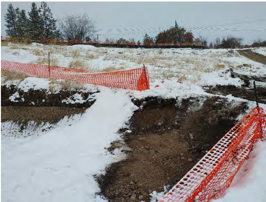
Photograph 2b: Finished expansion of northern west wall of Excavation 5.
