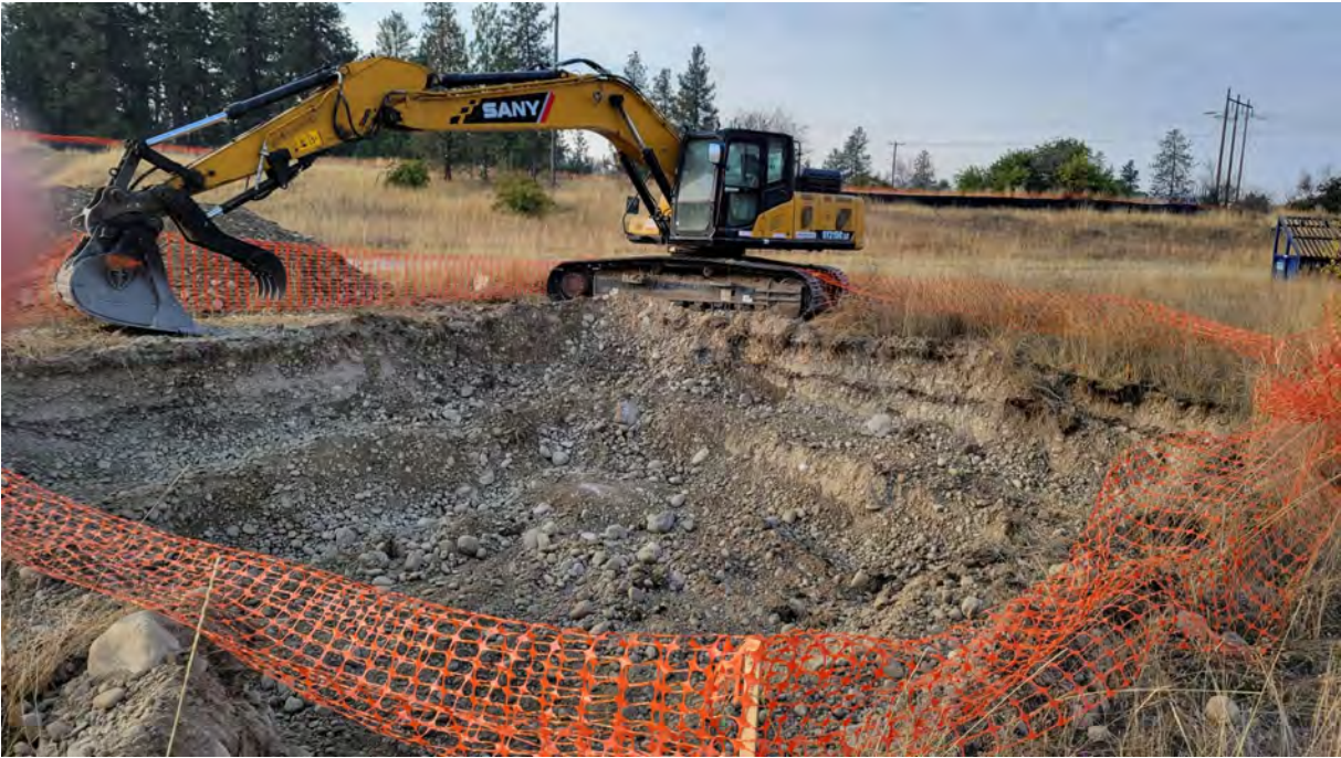
Photo 3. Finished excavation #6 on WSDOT.
