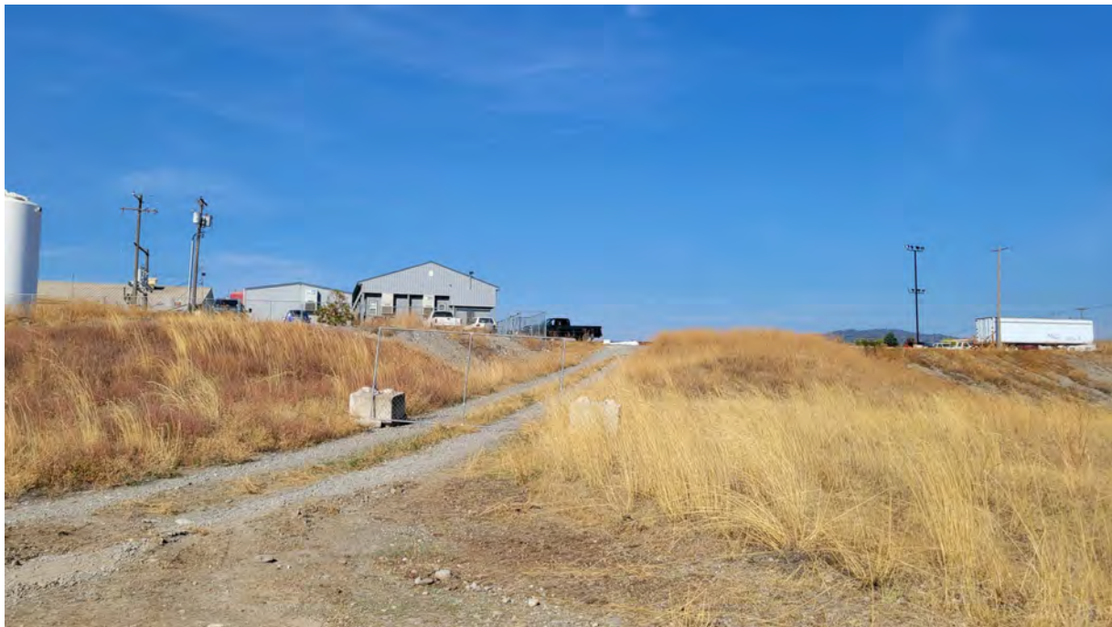
Photo 8. Road north to Kemira blocked by temp fence.
