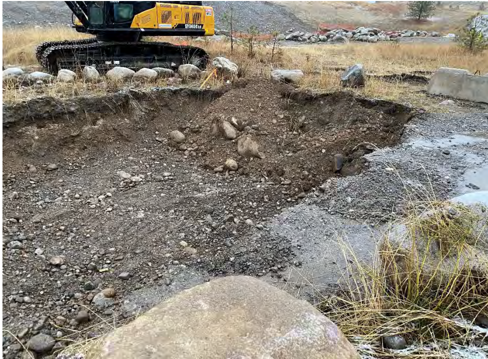
Photo 1. Extending east end of Excavation 7 to collect confirmation samples.
