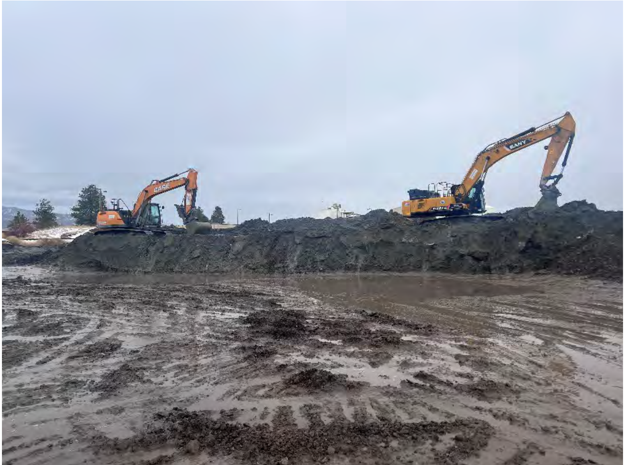
Photograph 1: Staging area for dross loading.
