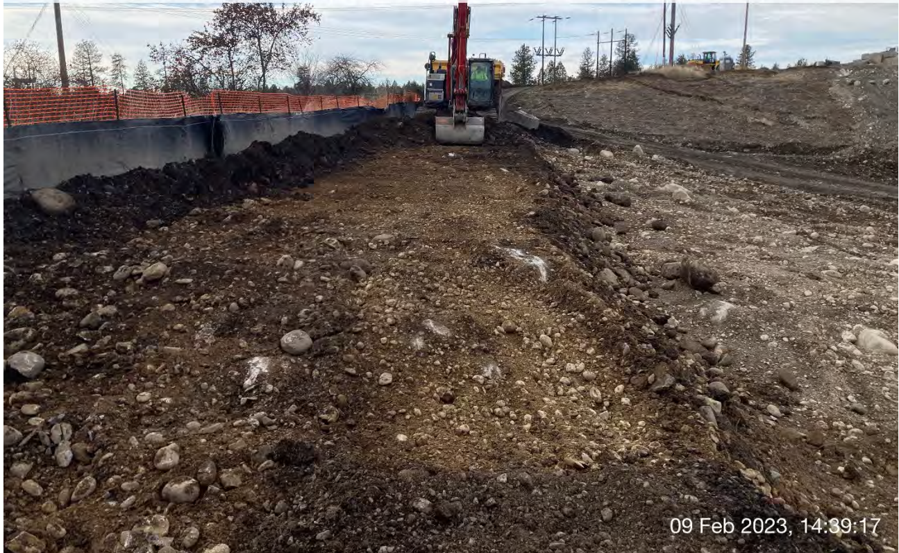
Photograph 2: 2-foot excavation area on WSDOT property along southern exit haul route.
