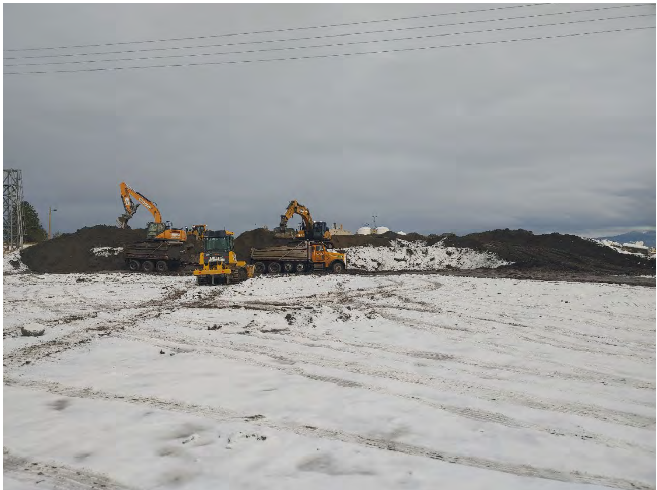
Photograph 1: Dross stockpile excavation activities.
