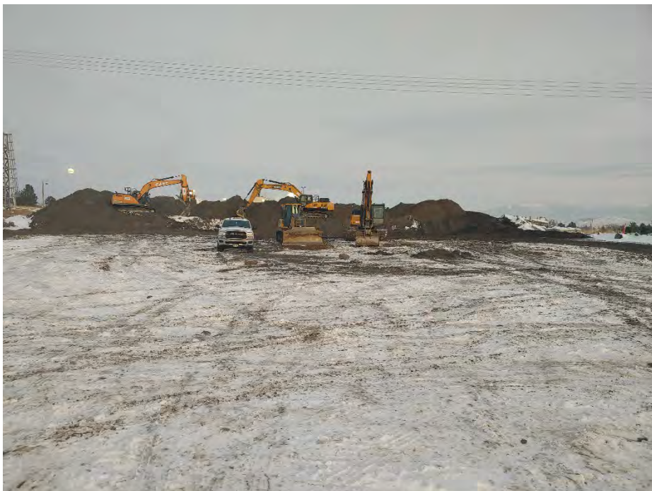
Photograph 5: End of day at the cross stockpile
