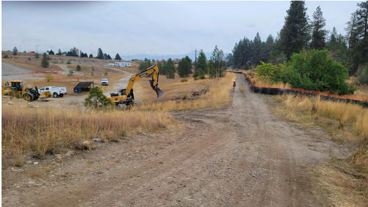
Photo 3. GrayMar is adjusting the in-bound haul road to miss WSDOT excavation #7.
