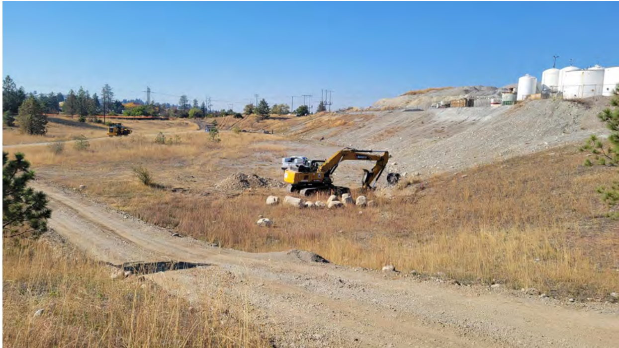
Photo 4. Eastern most WSDOT dig excavation.
