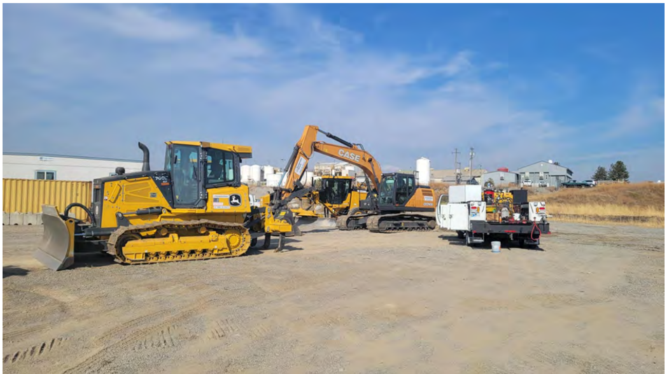
Photo 4. Bulldozer arrived 10/6 and Trackhoe arrived 10/7.
