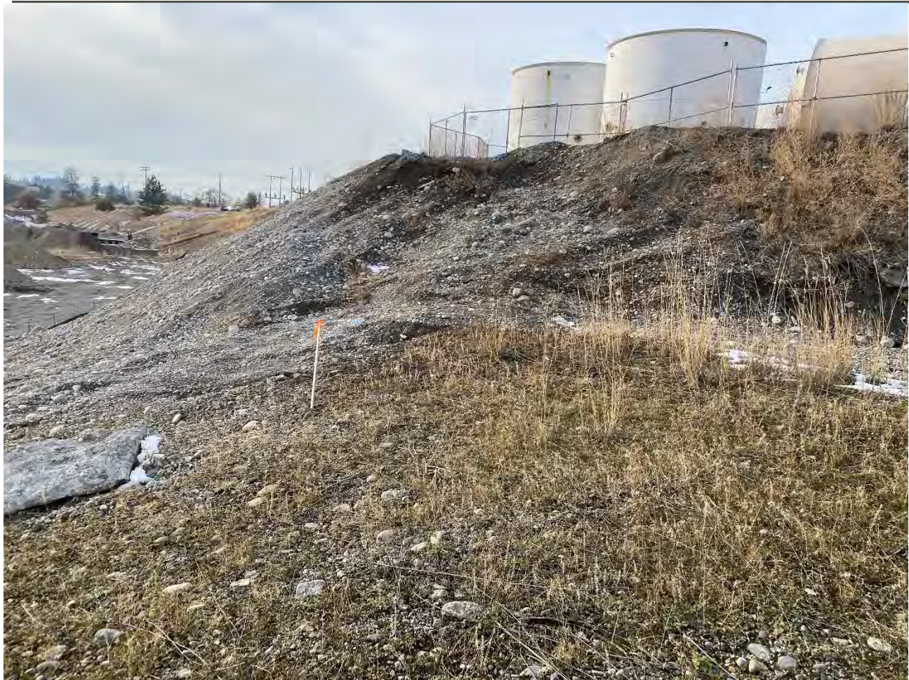
Photo 1. Surveyed WSDOT/UPRR property boundary.
