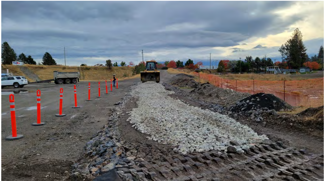
Photo 5. SW corner of dross stockpile being lowered.
