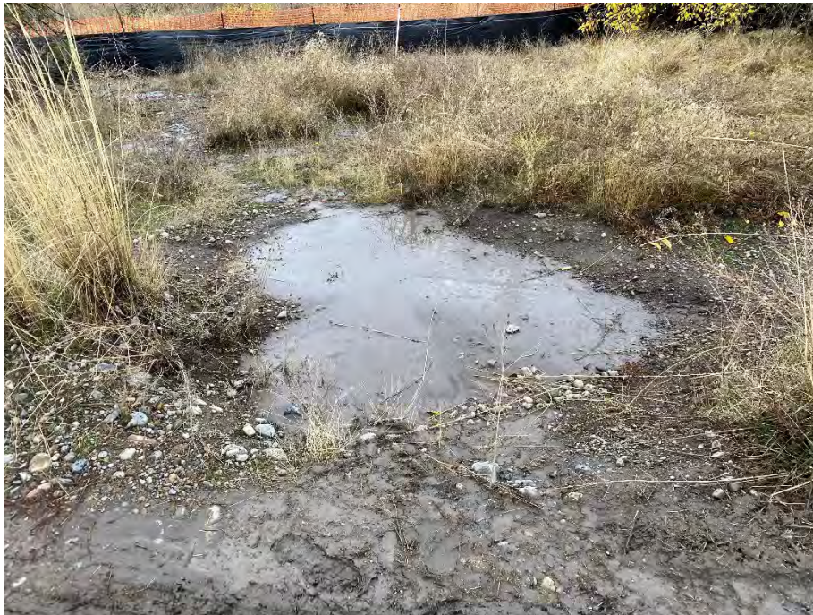
Photo 2. South haul out road breach from yesterday. GrayMar addressed condition with road grading ditch.
