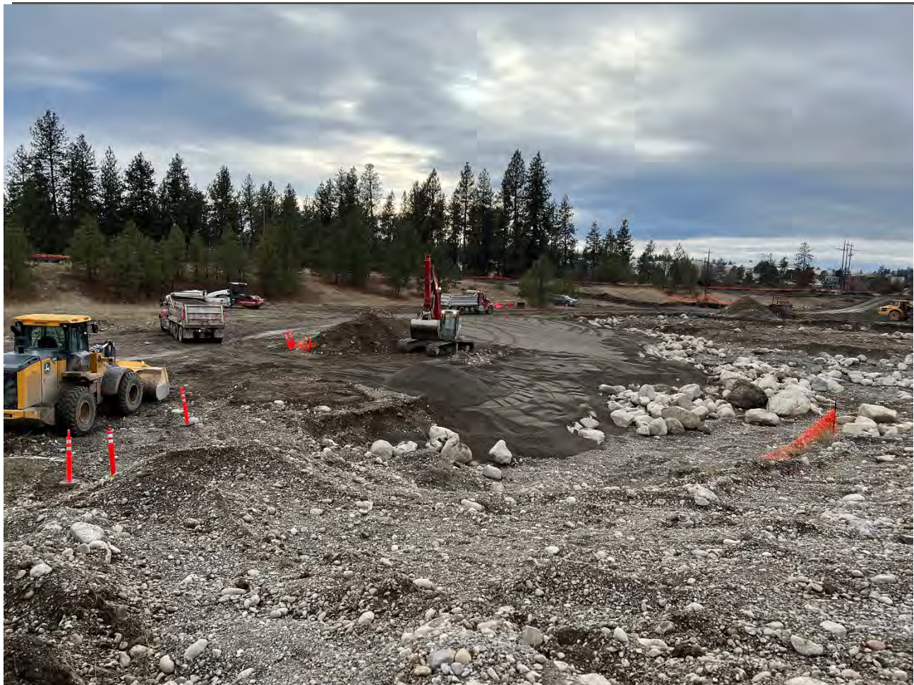
Photograph 3: Placement of backfill on WSDOT property.
