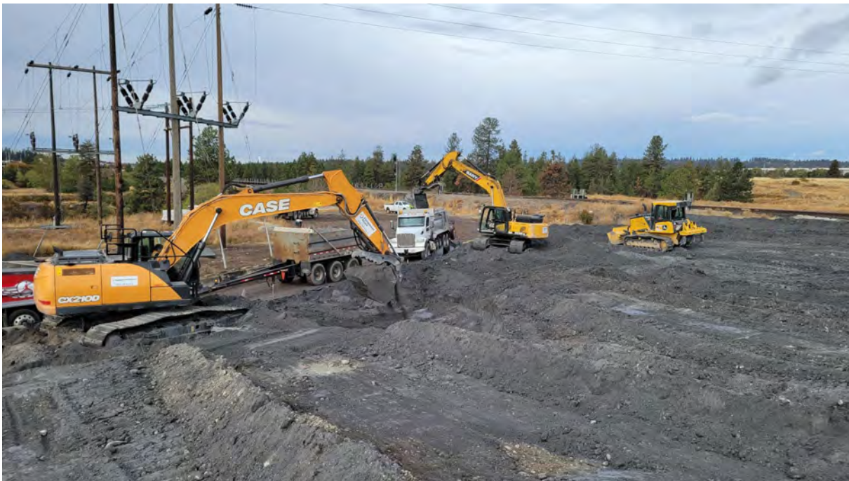
Photo 3. Excavators reaching subgrade at west end of dross pile.
