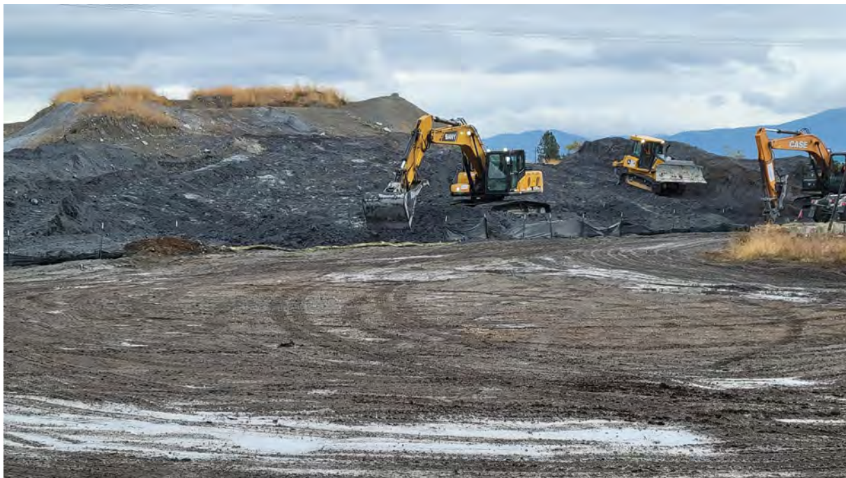
Photo 4. Bulldozer pushing dross to two excavators.
