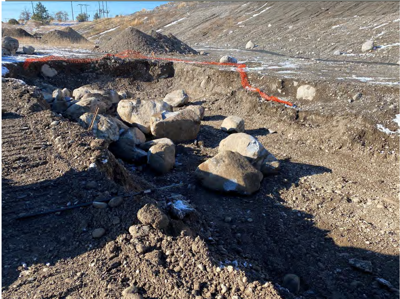
Photo 3. Excavation #8/9 facing northwest 6-feet deep, boulders left in the excavation.
