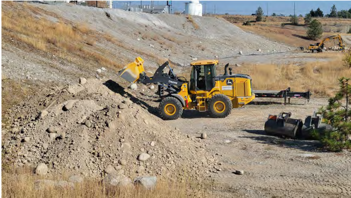
Photo 5. Stockpile of WSDOT excavation material.
