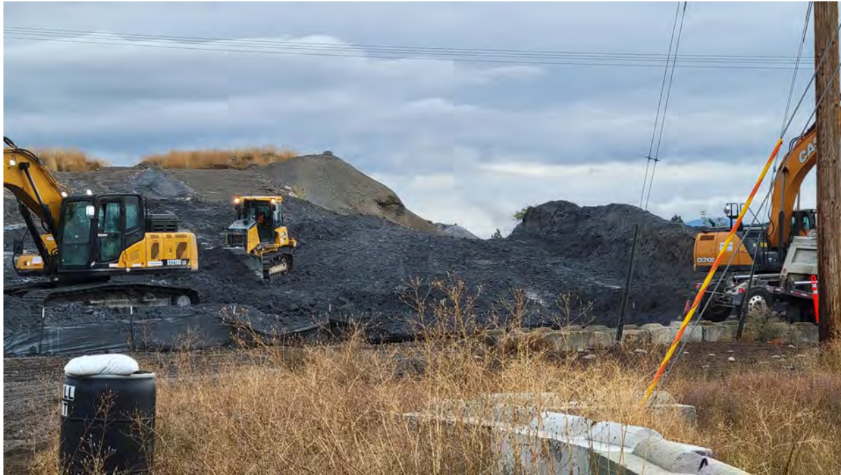
Photo 5. SW corner of dross stockpile being lowered.
