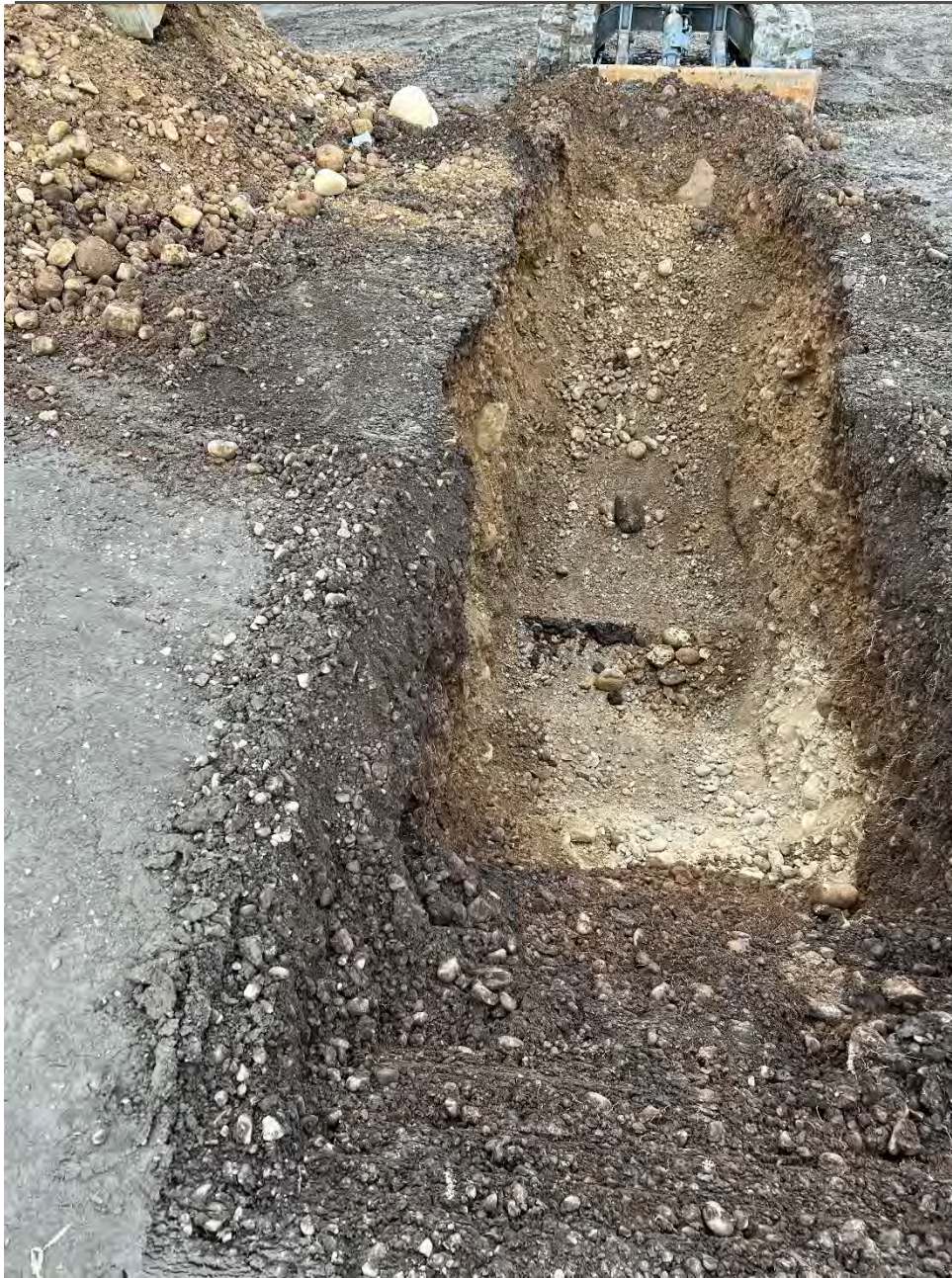
Photograph 6. Excavation down to 6ft bgs at Avista's underground utility location.
