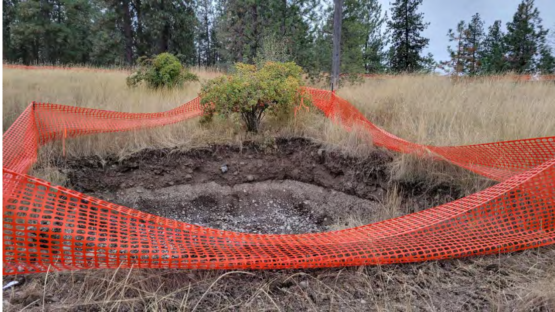
Photo 1. Security fence installed around WSDOT excavation #5, which was excavated 10/21/22.
