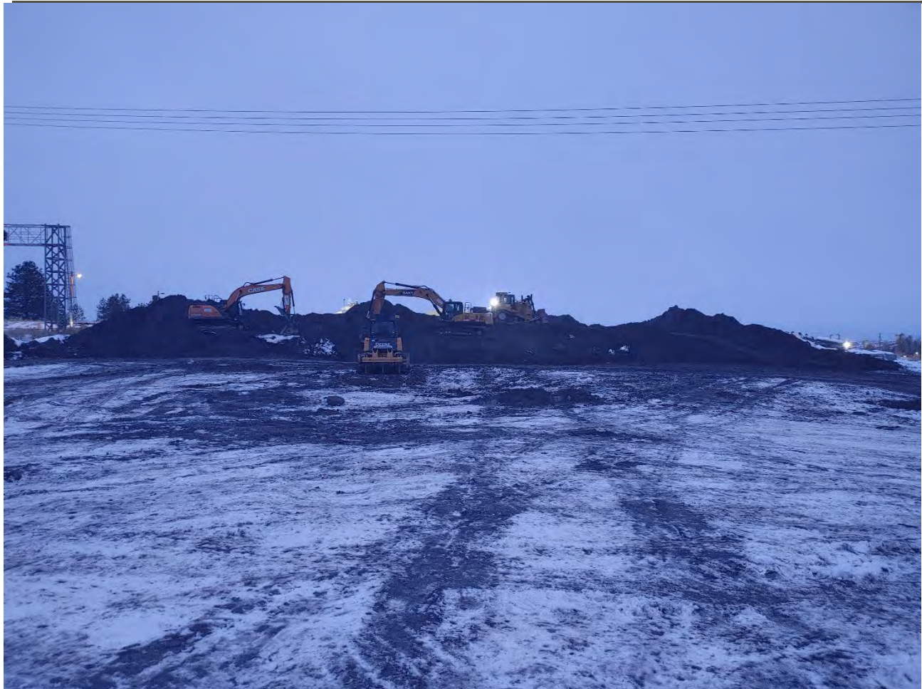
Photograph 4: End of day at the dross stockpile area.
