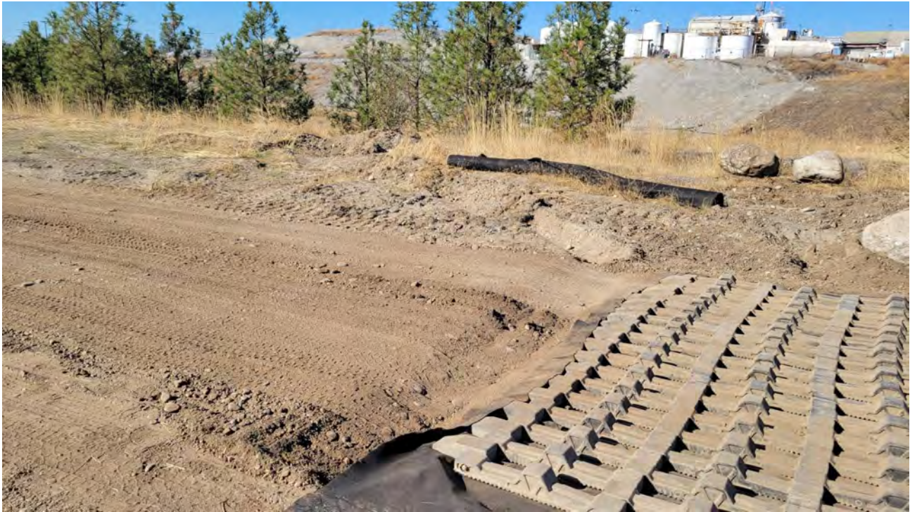
Photo 6. Drain system for rumble strips.
