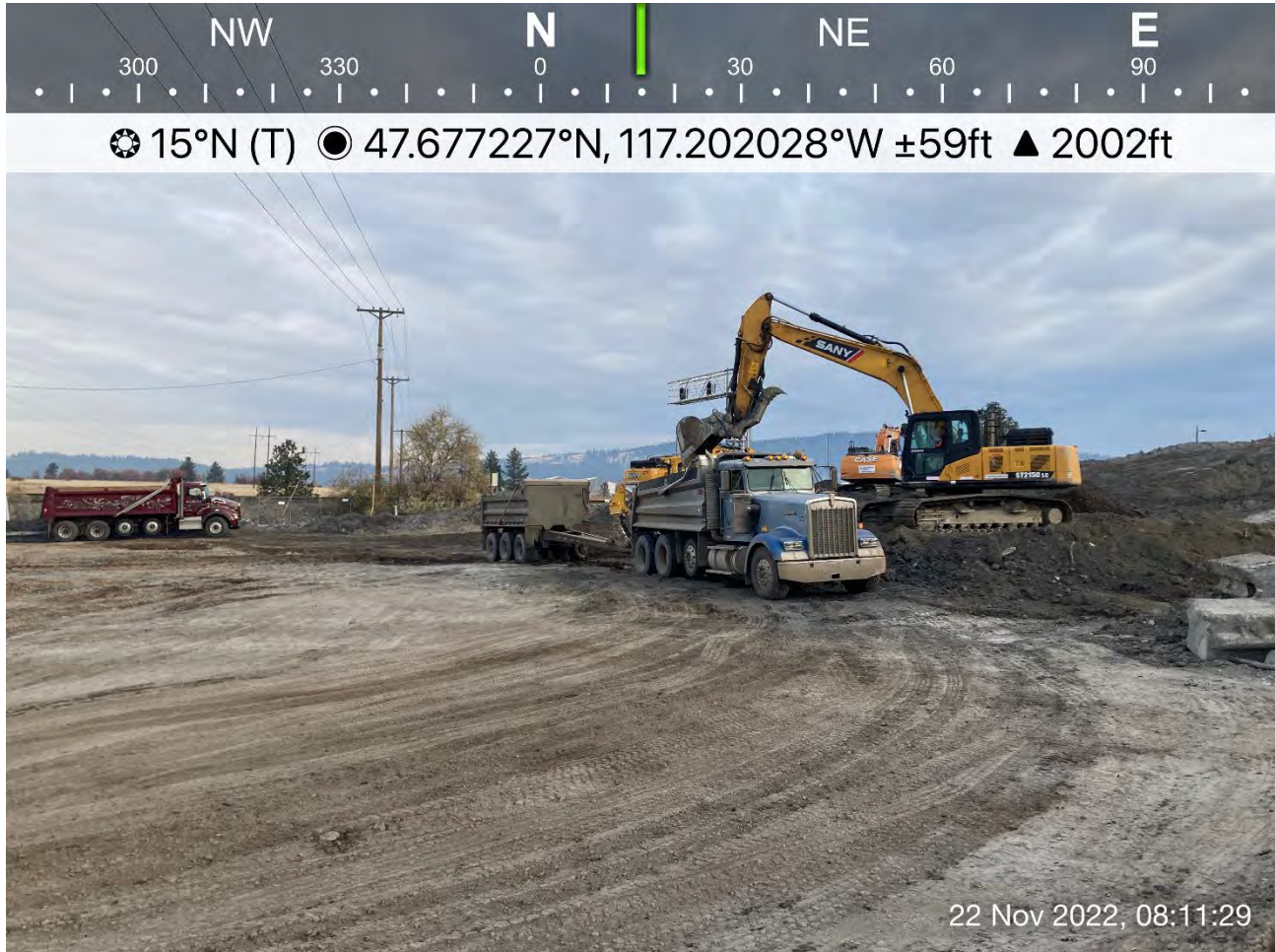
Photo 1: Sany SY215C LC trackhoe loading a haul truck with dross material.
