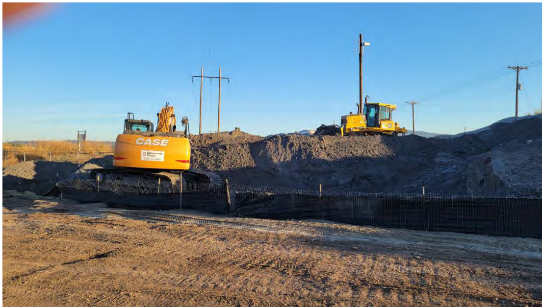
Photo 1. Bulldozer and excavator reducing west end of dross pile.
