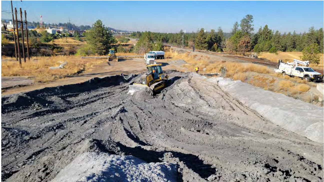
Photo 4. Bulldozer lowering area under the BPA wires.
