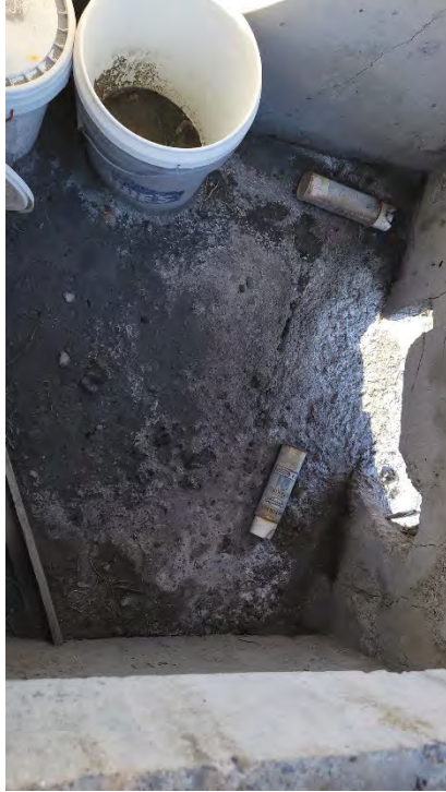
Photo 1. Looking into south vault
