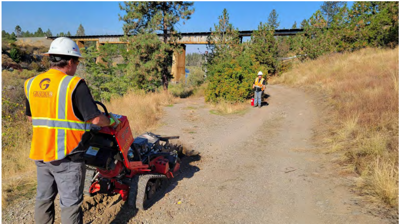
Photo 6. Trenching east of the river toward trestle.
