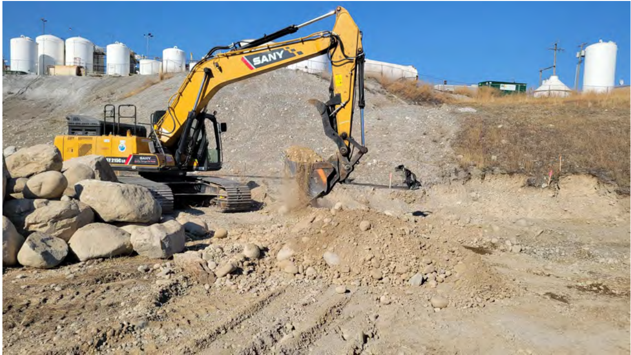
Photo 7. Continued excavation on WSDOT #9.
