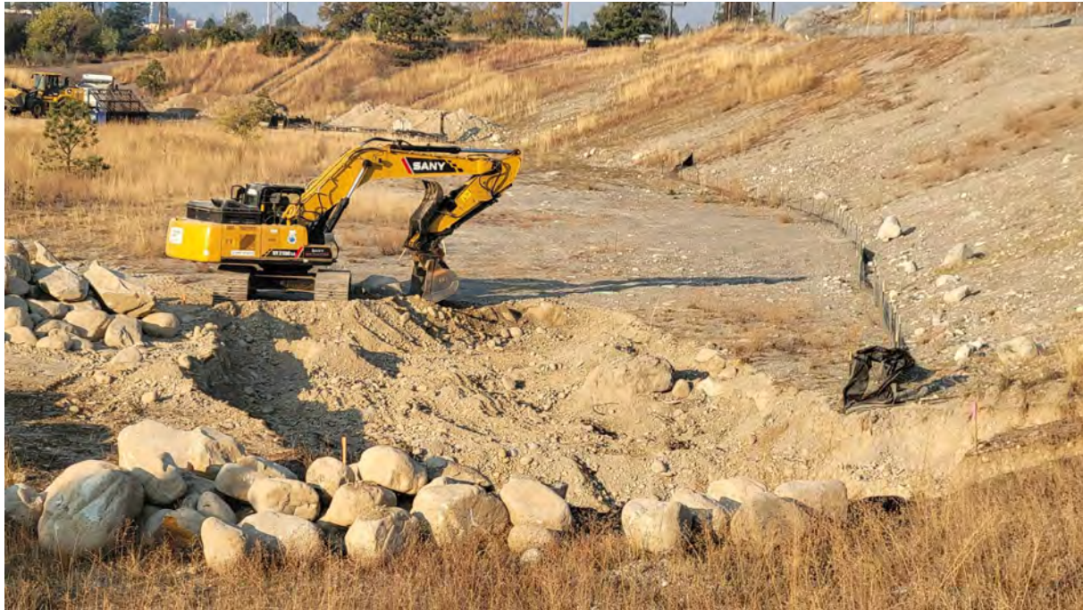
Photo 3. Start of excavation on WSDOT #8.
