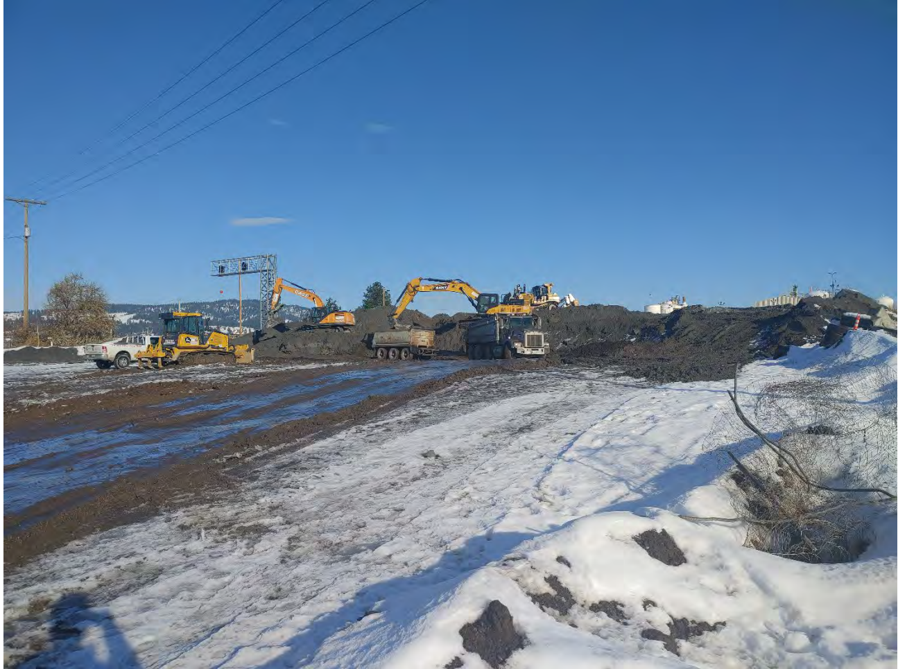
Photograph 1: Dross stockpile excavation activities.
