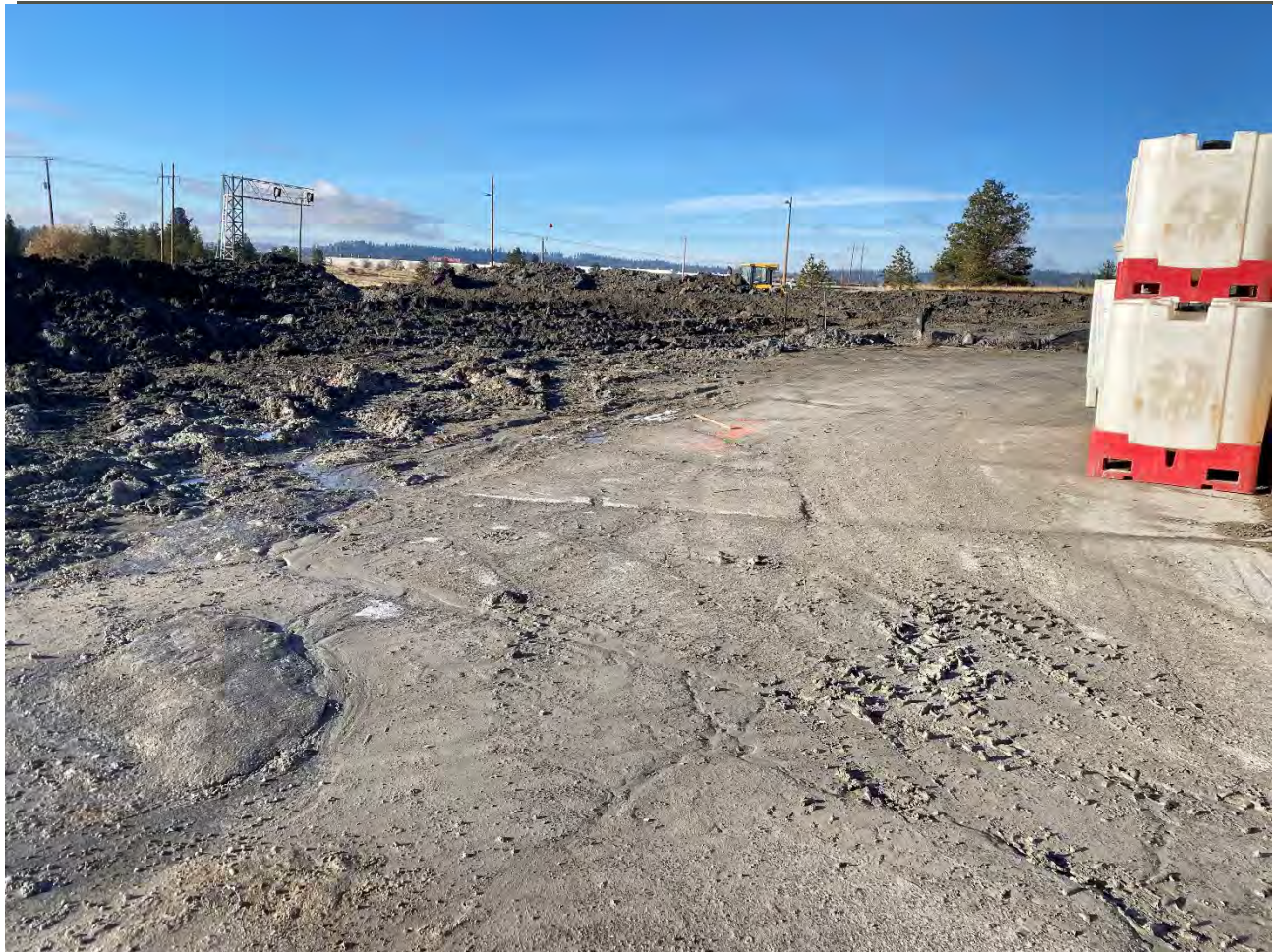
Photograph 2. Dross stockpile area looking northwest from southeast corner on Kemira.
