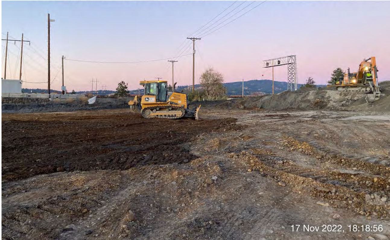
Photo 3: John Deere 700L bulldozer grading staging area near cross pile.
