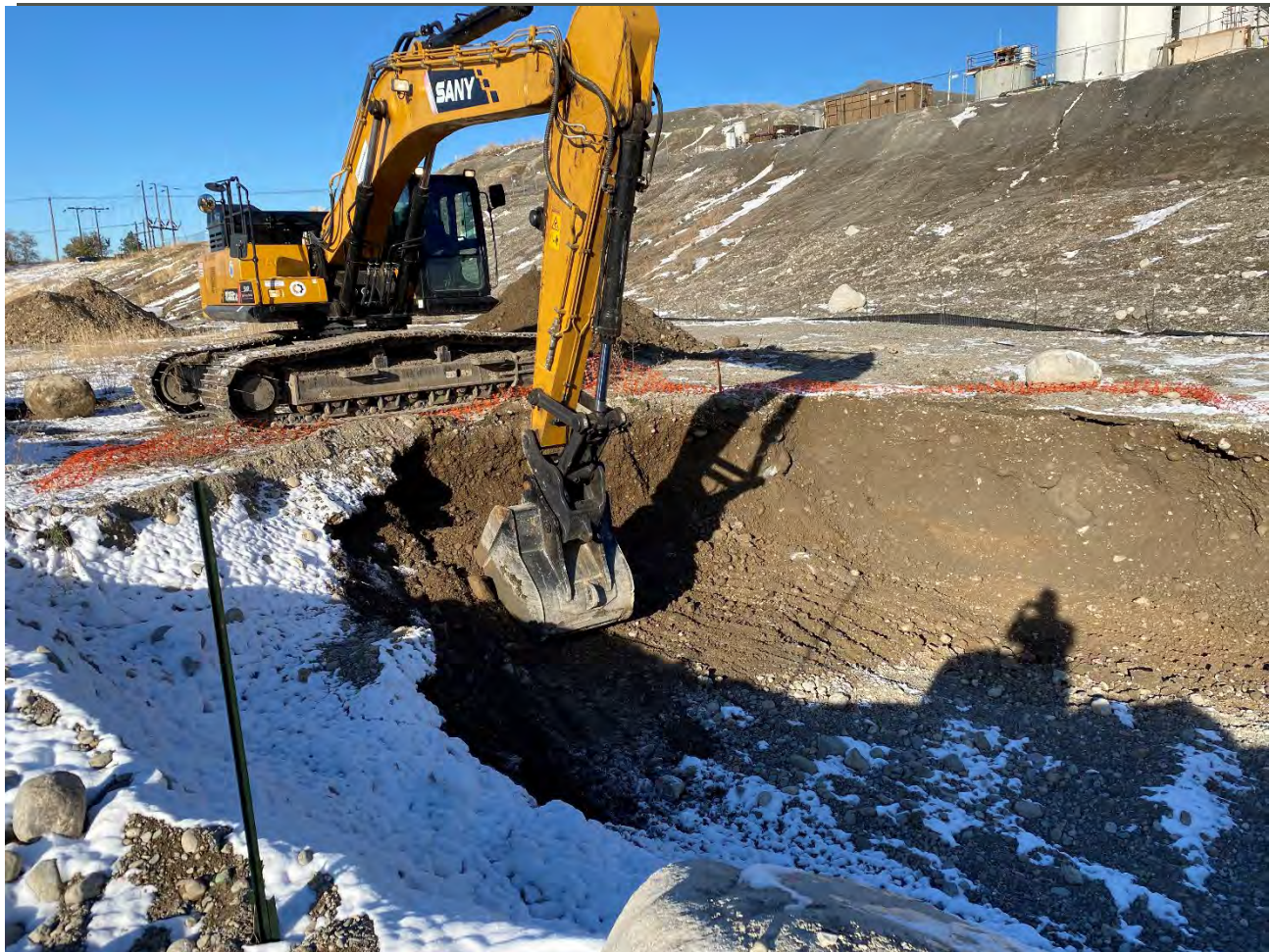
Photo 1. Extending west wall of Excavation #8.
