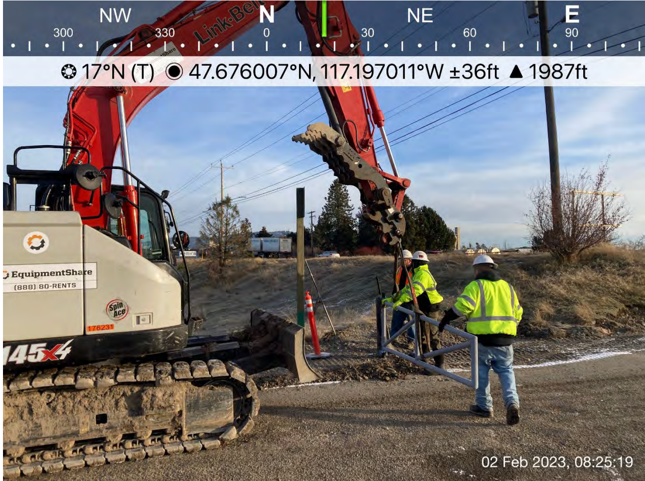
Photograph 2: Checking the alignment of the entrance gate.
