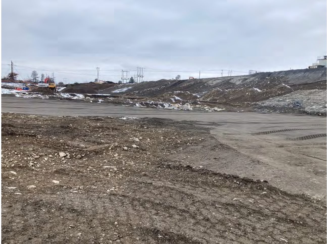
Photograph 1: Backfilled target excavation area on WSDOT property.
