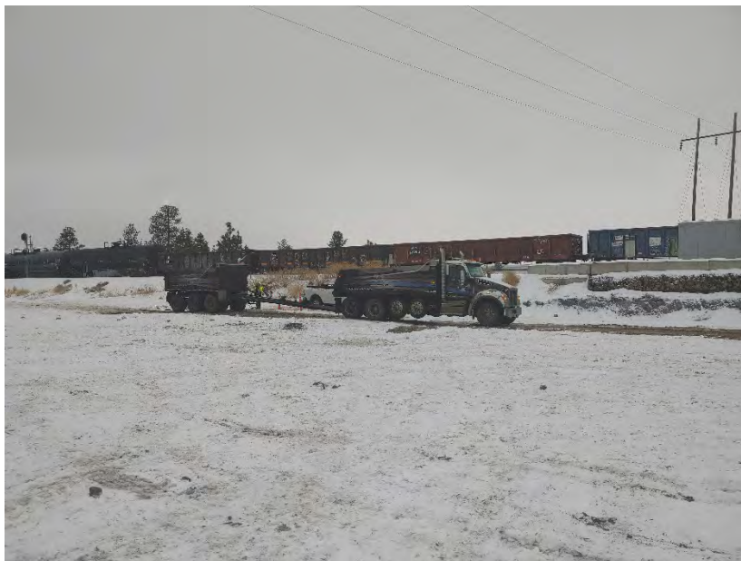
Photograph 3: Haul Truck Bed Lining
