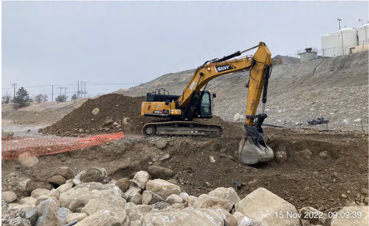
Photo 2: Excavation #8 & #9 facing northwest 4-feet deep.
