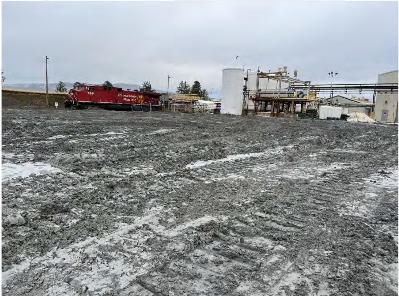
Photograph 2: Grading on east end of former stockpile area near Kemira facility.
