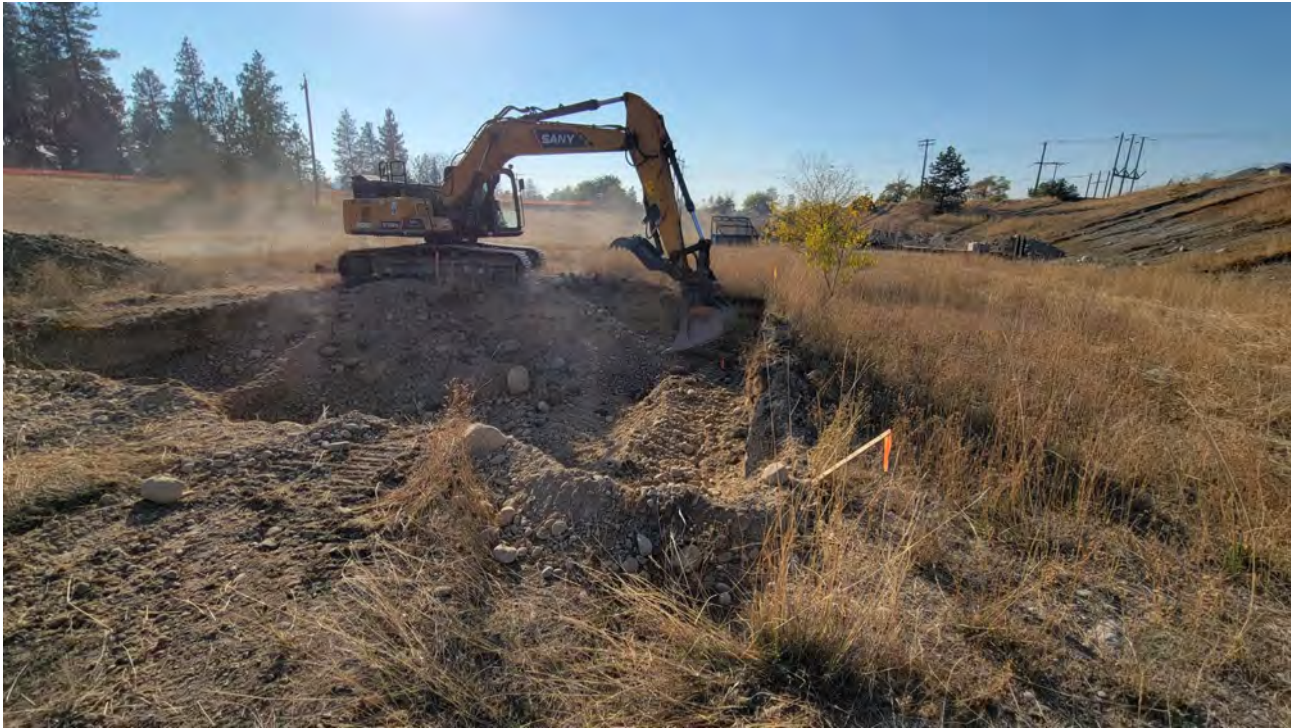
Photo 7. Excavation on WSDOT #6.
