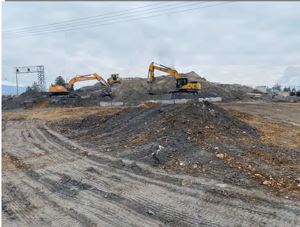
Photo 2. Continued cross removal typical.
