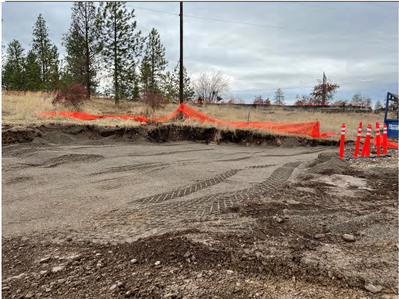
Photograph 2: Excavation 5 backfilled and rolled with DYNAPAC CA2500D up to 2ft depth.
