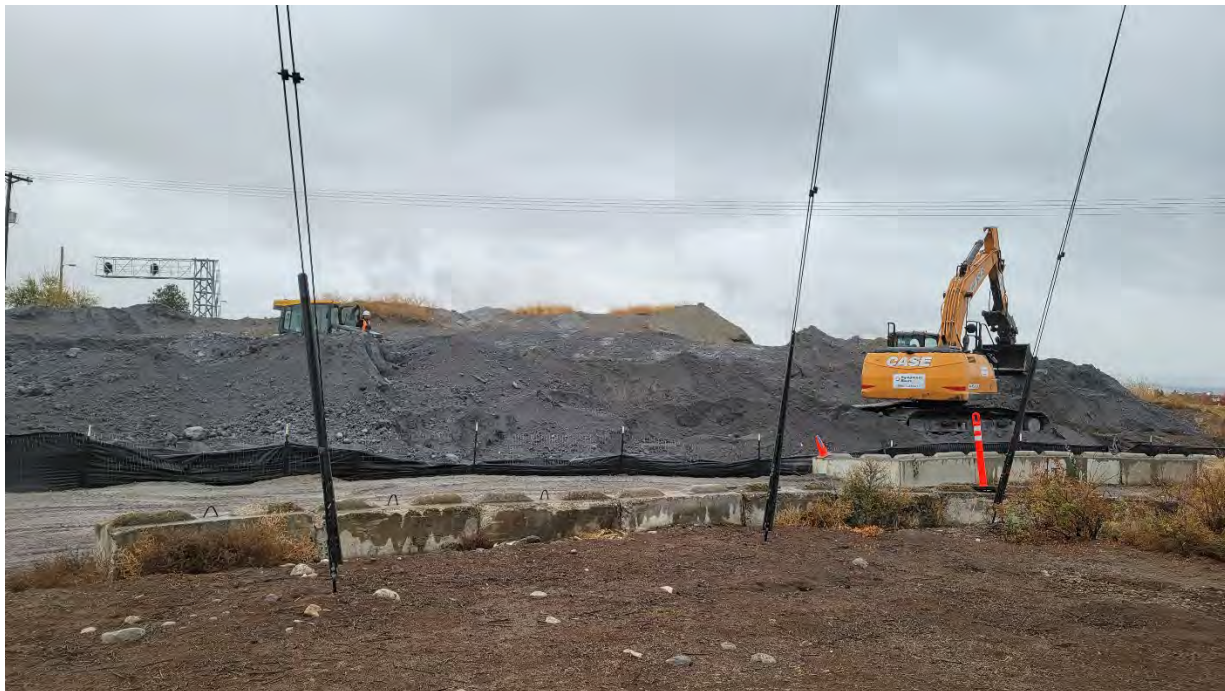
Photo 6. Progress on cross pile.
