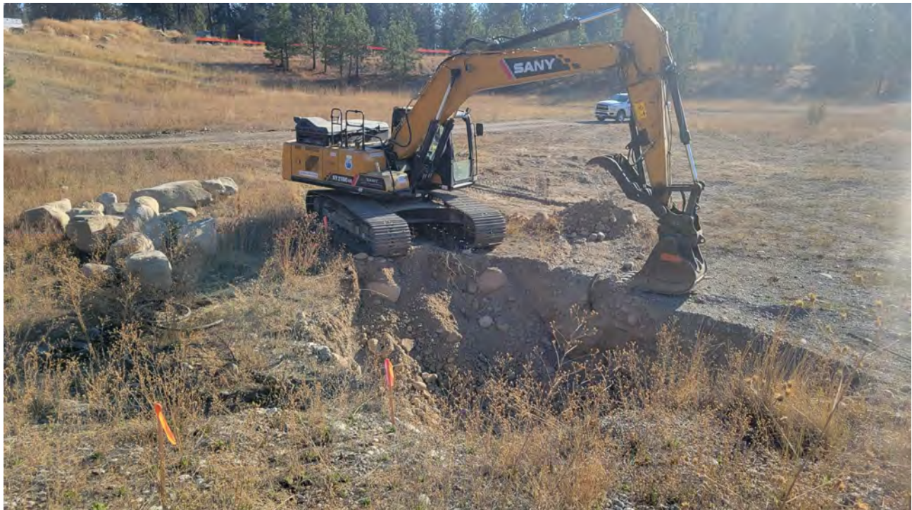
Photo 5. Boulders on left of photo came out of one 20'x20'x6' hole.
