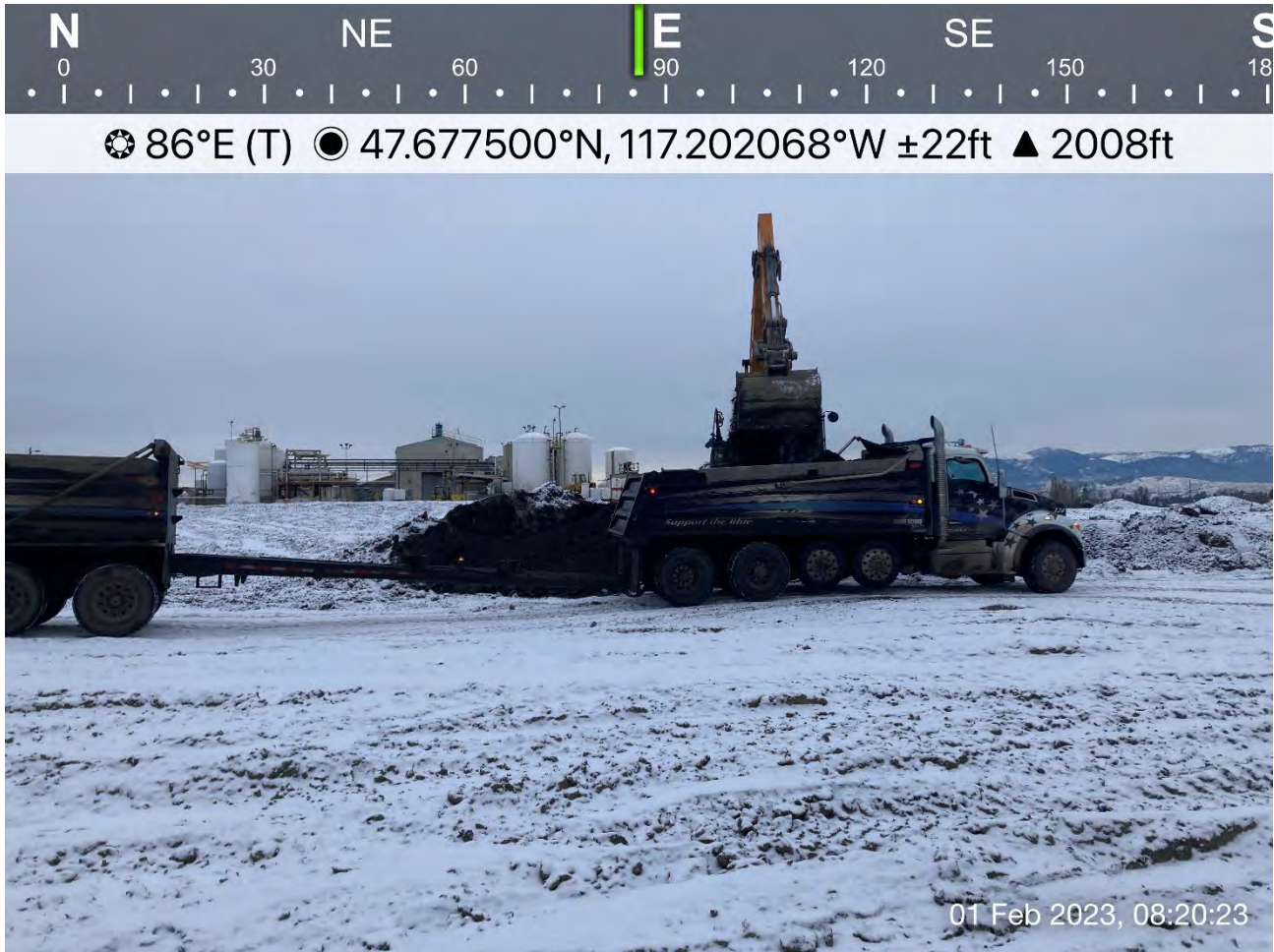
Photograph 1: Loadout activities at the dross pile located on UPRR property.
