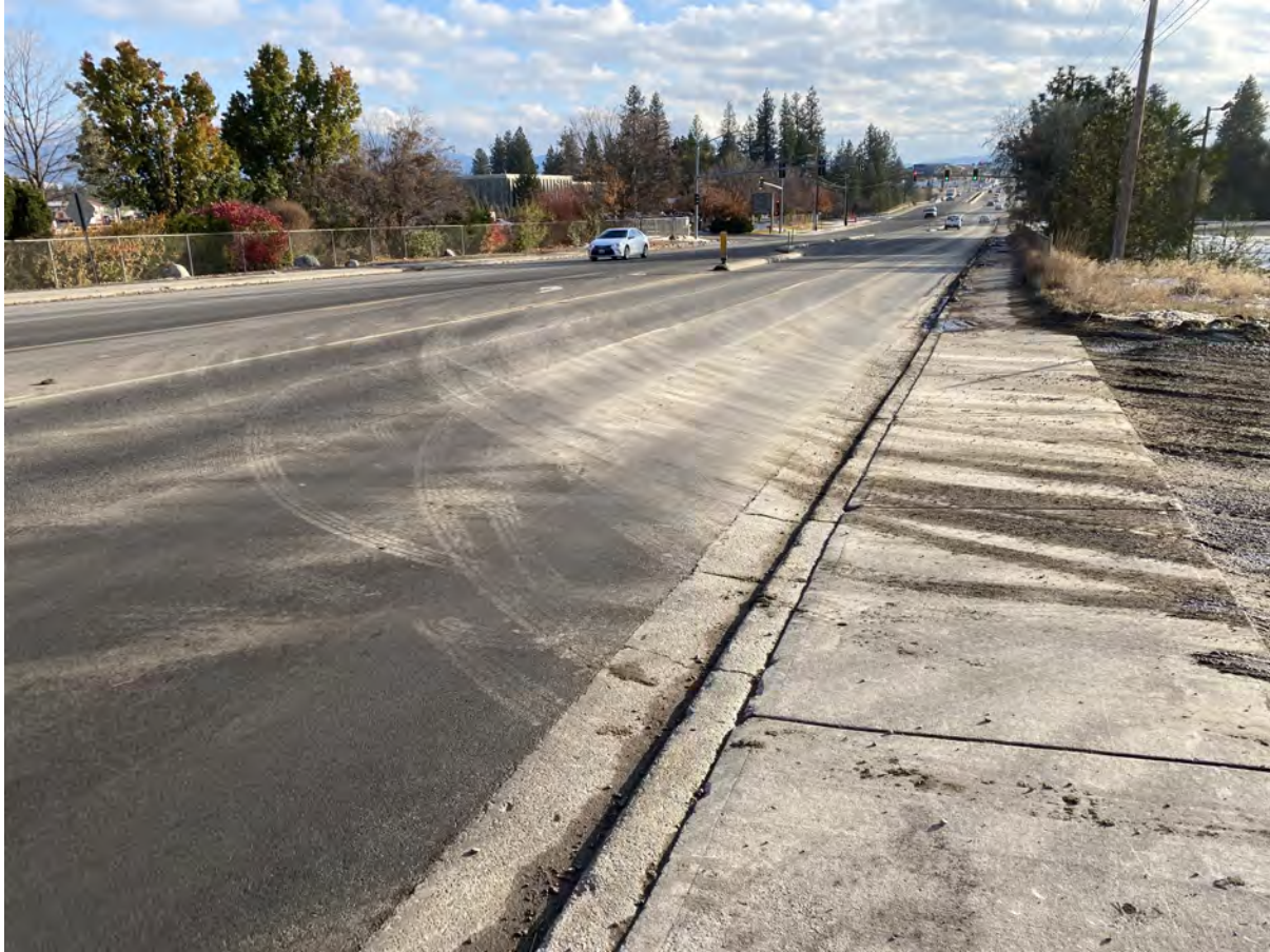
Photo 2. Track out on Sullivan prior to sweeping.
