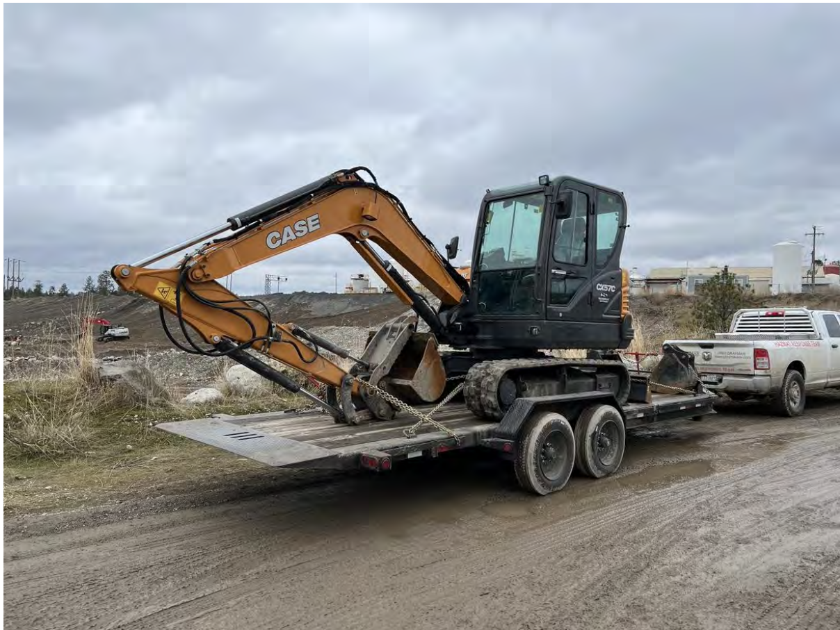
Photograph 1: Mini trackhoe (CASE CX57C) brought to site.
