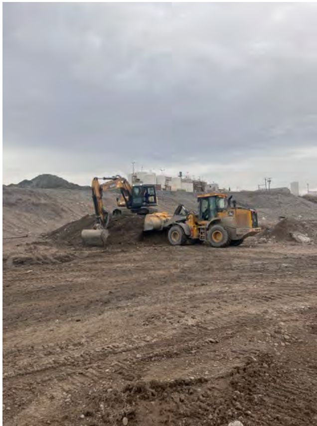
Photograph 1: Progress on Stockpiles.
