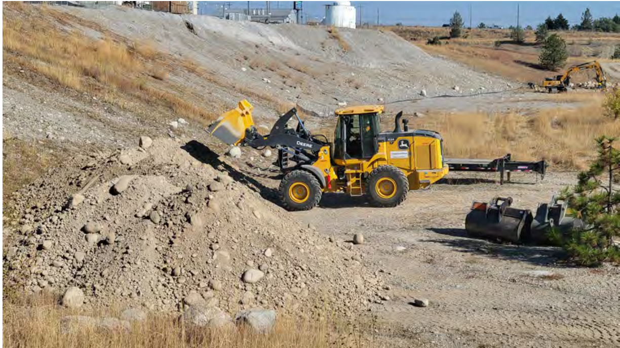
Photo 5. Stockpile of WSDOT excavation material.
