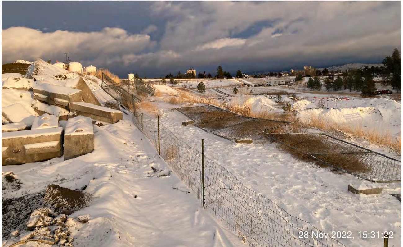
Photo 2: Temporary fencing around UPRR disassembled and staged for removal.
