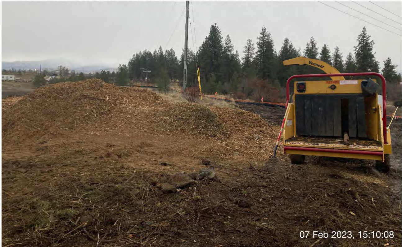
Photograph 3: Woodchip pile and trailer-mounted woodchipper near the junction of the Pentzer, WSDOT and UPRR properties.
