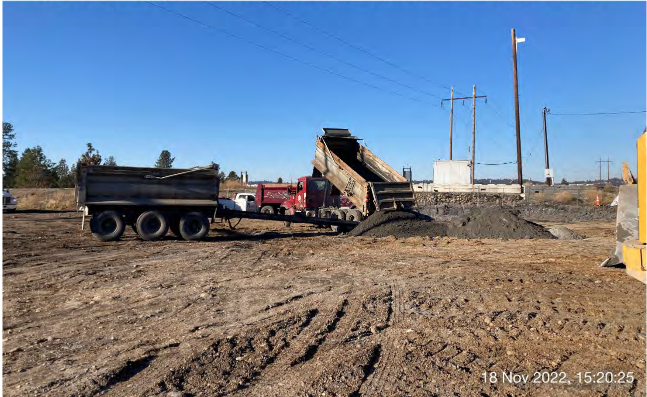
Photo 3: Haul truck dumping stuck dross into an existing pile near the staging area.
