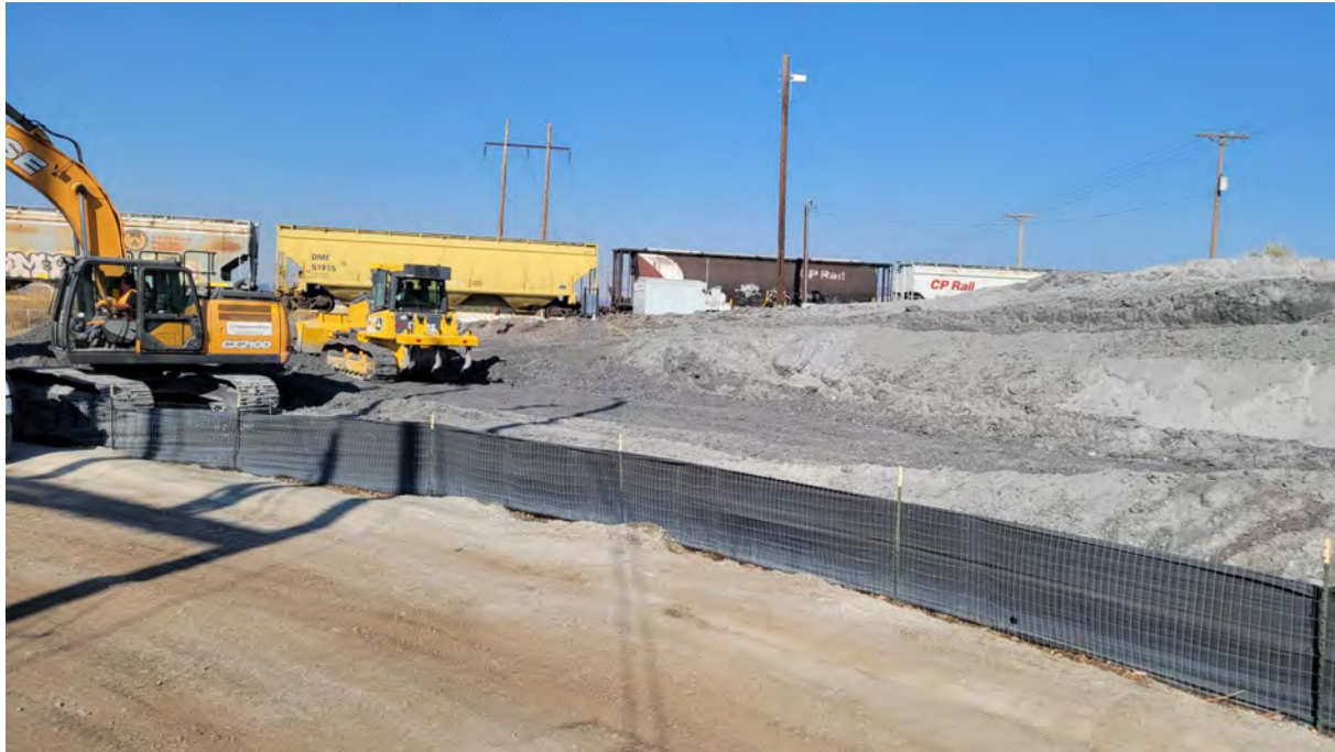
Photo 3. West end of pile almost to grade level.
