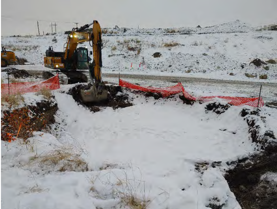
Photograph 2a: Beginning of expansion of northern west wall of Excavation 5.
