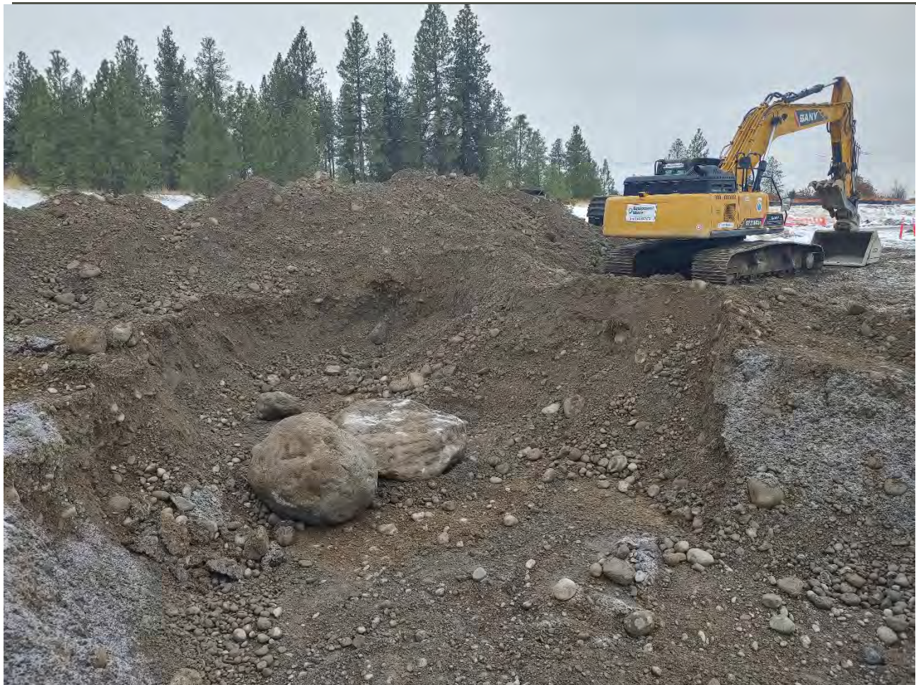
Photograph 2: Continuing southward expansion of southeast corner of Excavation 8, following visible dross.
