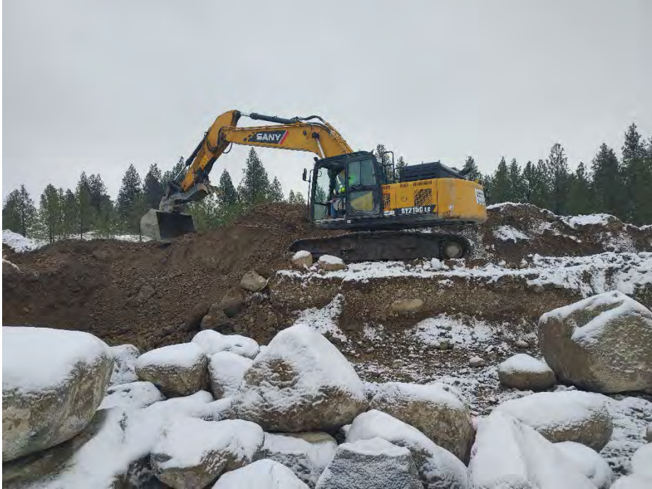
Photograph 2: Beginning of Excavation 8 southern expansion with visible cross layer below trackhoe.
