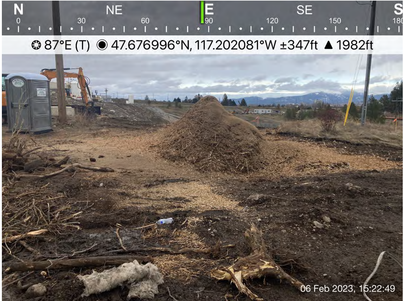
Photograph 2: Woodchip pile generated from chipping the brush generated through the clearing and grubbing of the Pentzer and WSDOT properties.
