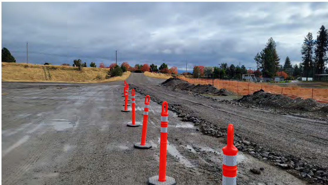
Photo 2. Gravel placed on driveway to control mud getting to Sullivan Rd.
