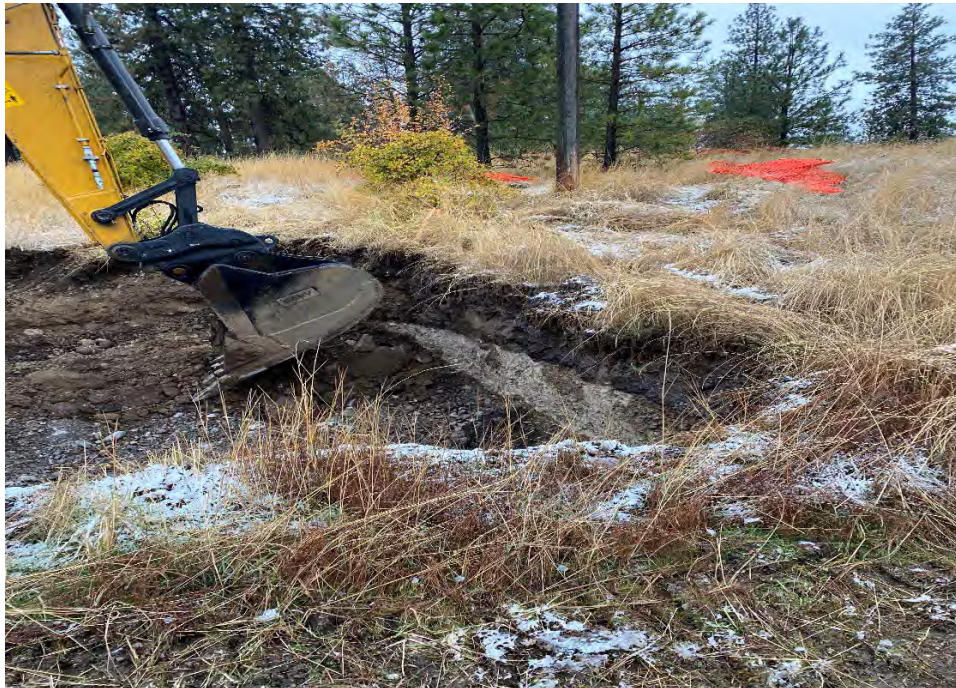
Photo 2. Extending south wall of Excavation 5 for additional confirmation sampling.
