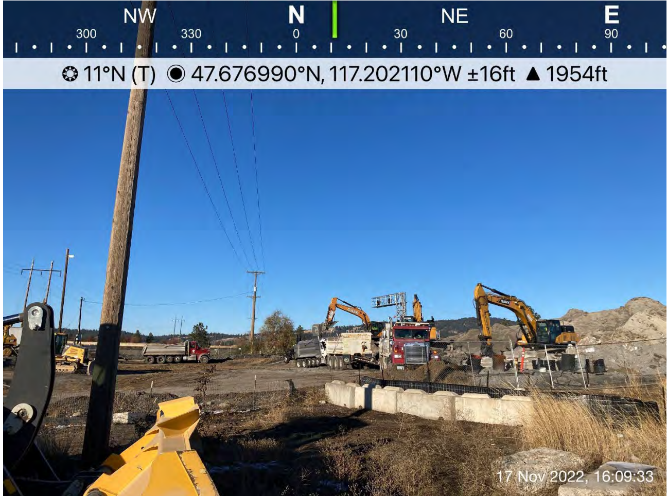
Photo 2: Trackhoes loading haul trucks with dross at the staging area.
