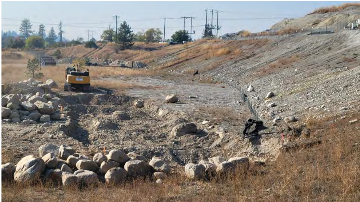
Photo 6. Large boulders left in WSDOT #8 & #9.
