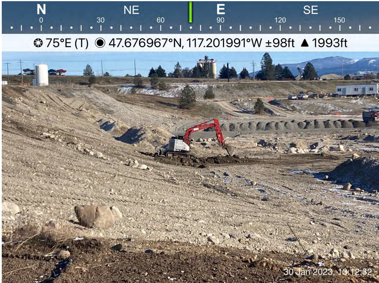
Photograph 2: Excavation of 2-foot cut area on WSDOT property north of Excavation 6.
