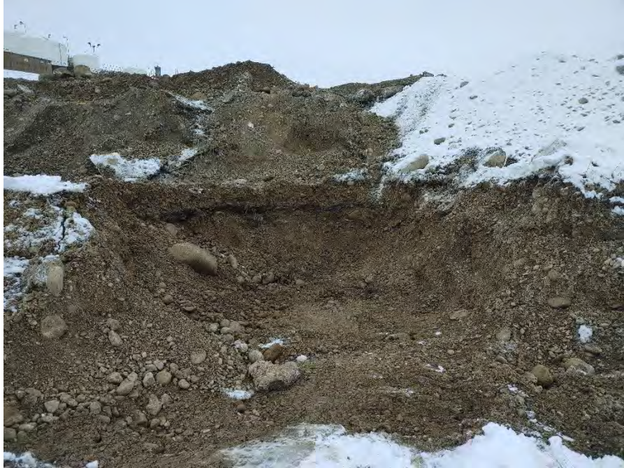
Photograph 3: Expansion of northern east wall of Excavation 6.
