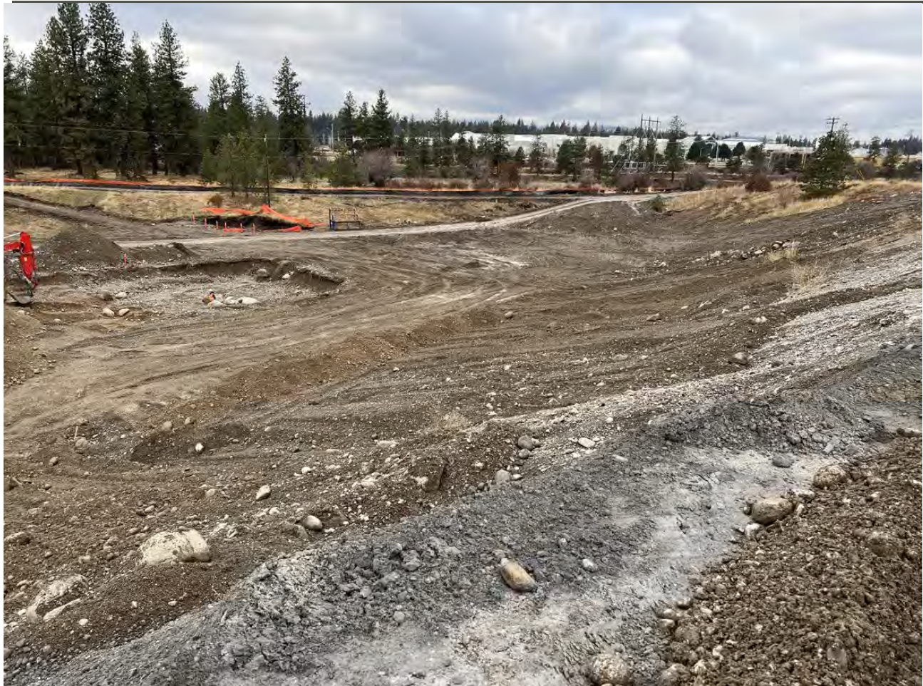
Photograph 4: Excavated WSDOT material stockpiled at base of slope on UPRR.
