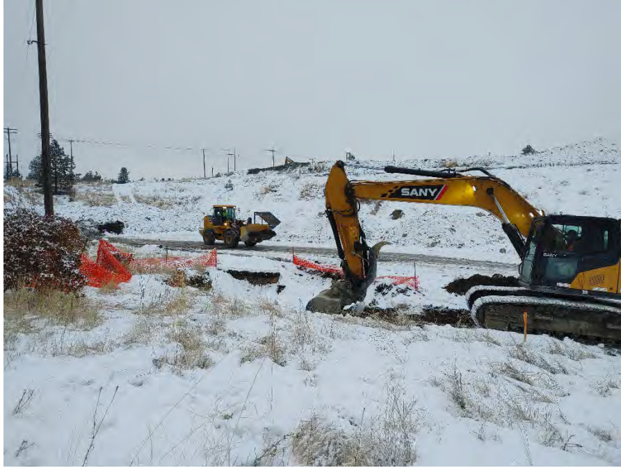
Photograph 1a: Partial expansion of eastern south wall of Excavation 5.
