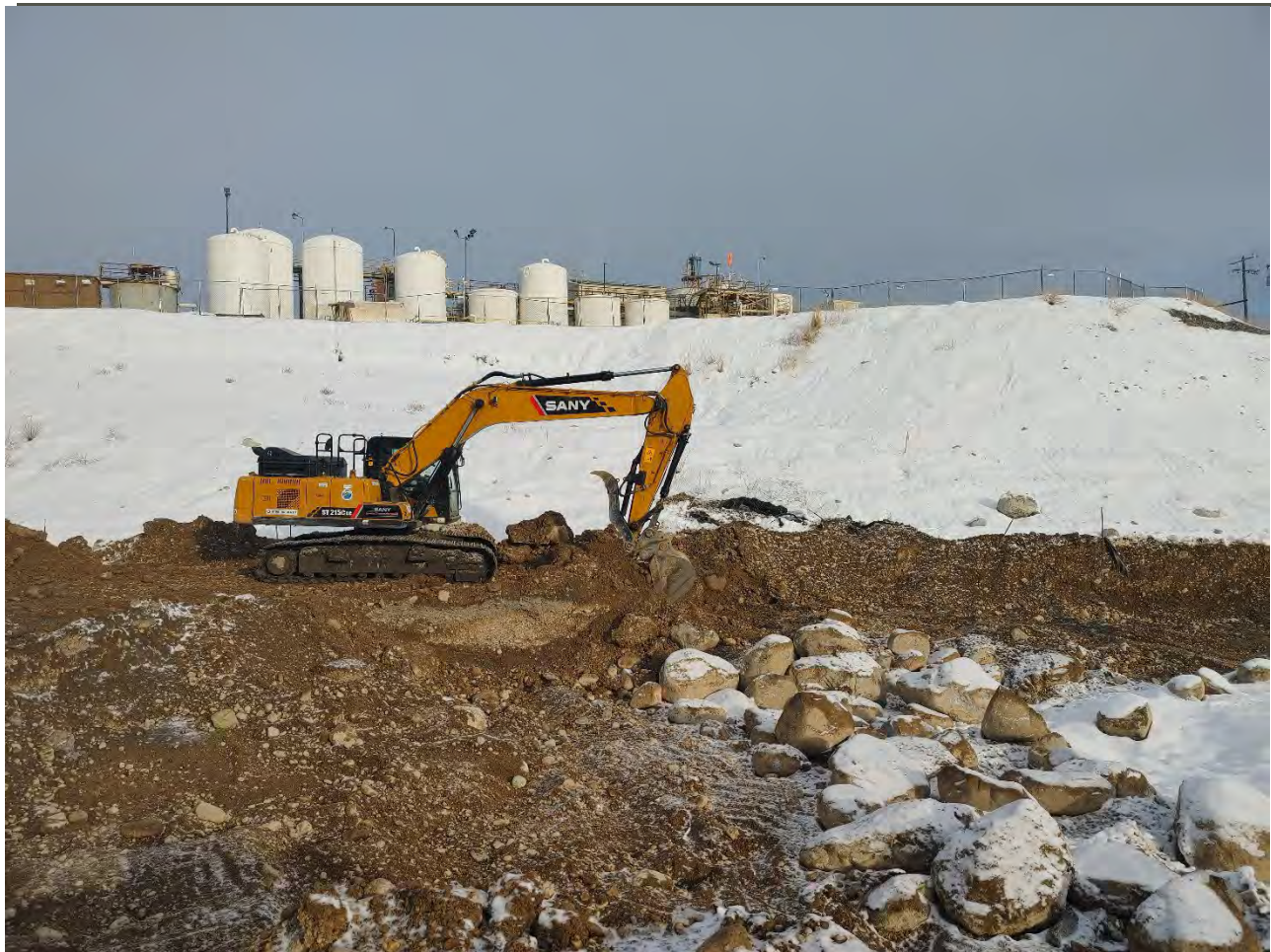
Photograph 3: Next iteration of west wall expansion of Excavation 8. Visual dross material observed approximately two feet below ground surface towards the northern end of the west wall (shown) and in a separate section towards the southern end of the west wall (not shown).
