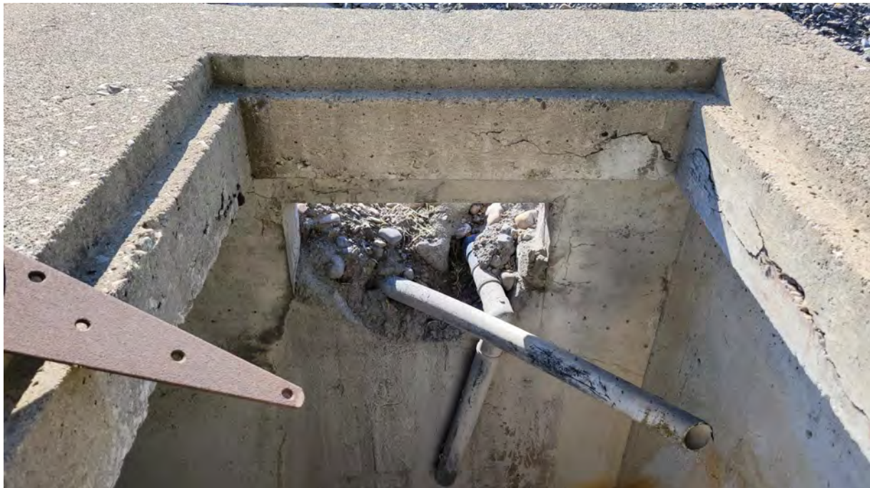
Photo 2. Two views inside of north vault.
