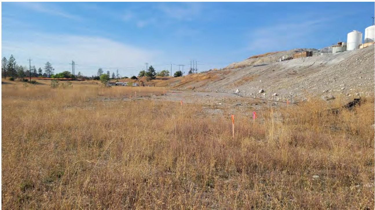
Photo 4. Eastern most WSDOT dig out laid out
