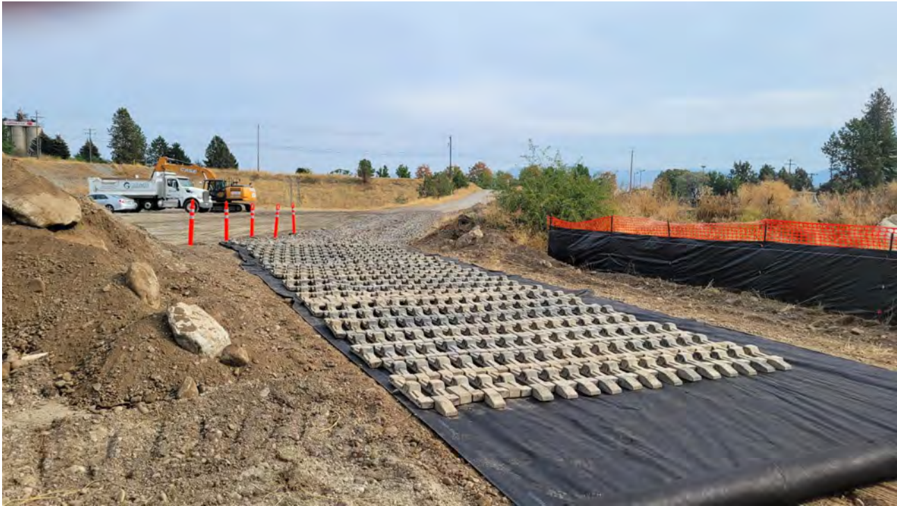
Photo 6. Truck rumble mats placed and ready.
