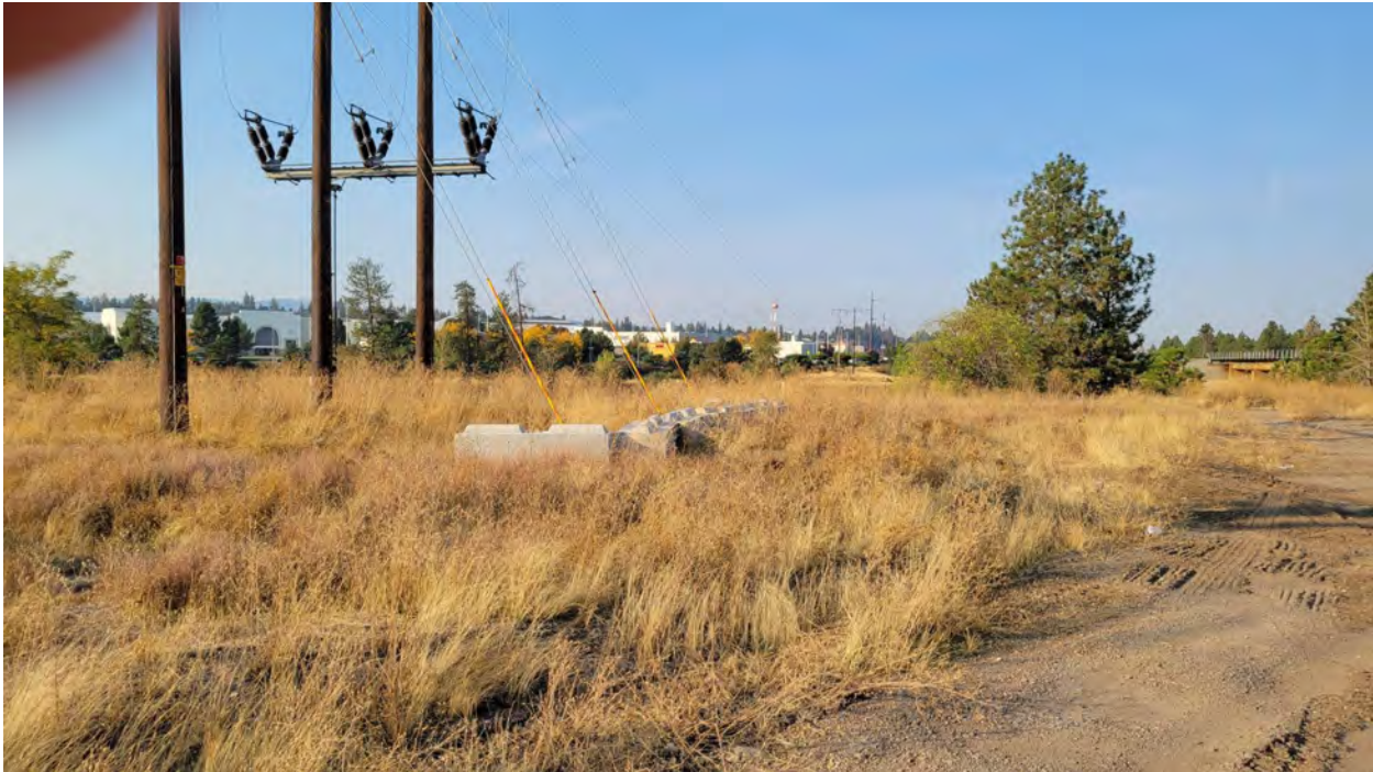
Photo 7. More ecology blocks placed around BPA guy wires for protection.
