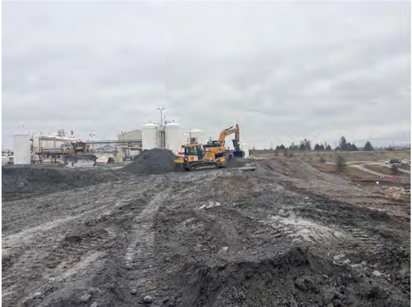
Photograph 1: Dross removal progress looking east approaching grade .
