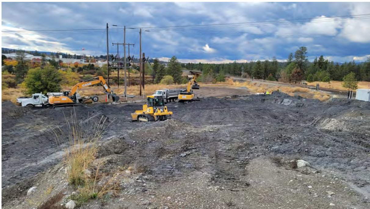
Photo 4. Bulldozer pushing dross to two excavators.
