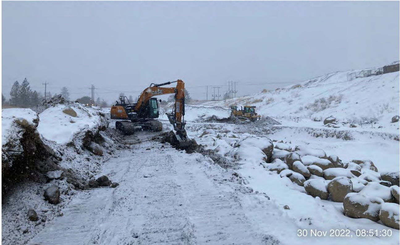
Photo 1: SANY 215C LC trackhoe expanding the south sidewall of Excavation 8.
