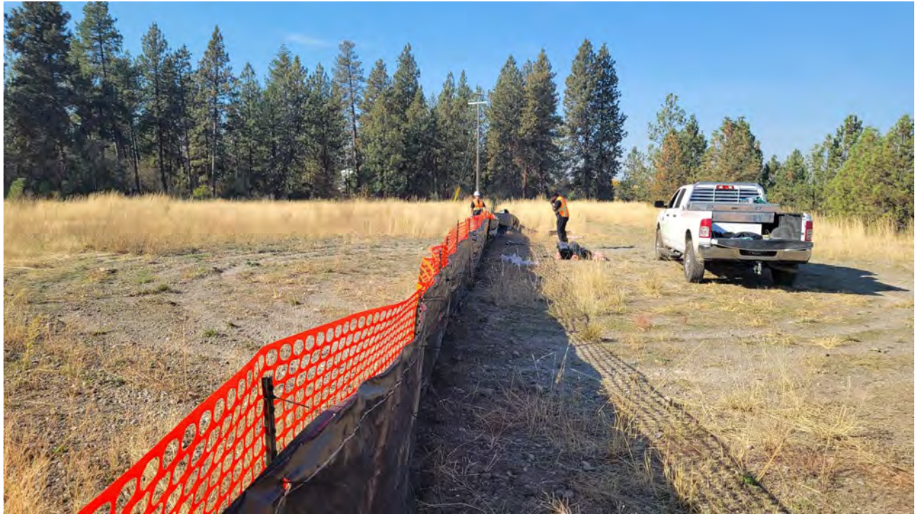
Photo 3. Silt and construction fence installed extending west from office trailer.
