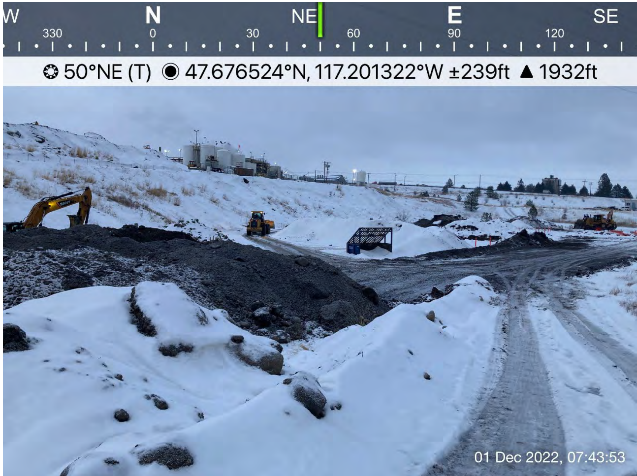
Photo 1: View of temporary storage pile located near the planned Excavation 4.
