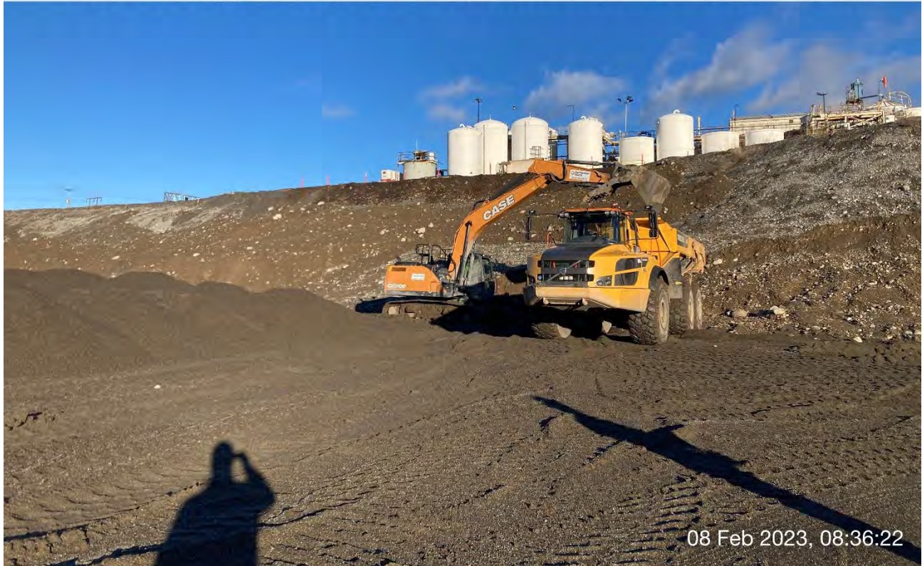
Photograph 2: Excavation of 2-foot excavation area on WSDOT property slope north of Excavation 8.
