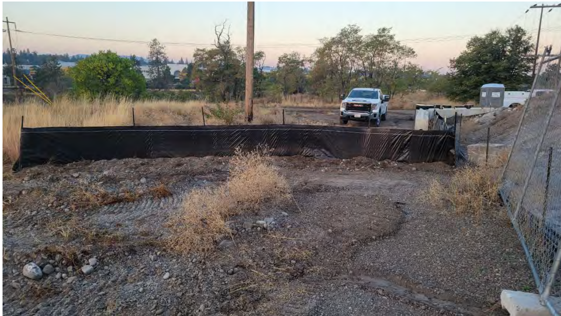
Photo 1. SW corner of dross pile, with silt fence against ecology blocks to deflect drainage off of pile.
