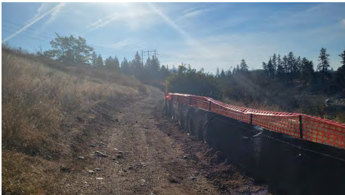
Photo 2. Silt/Construction fence east of river.
