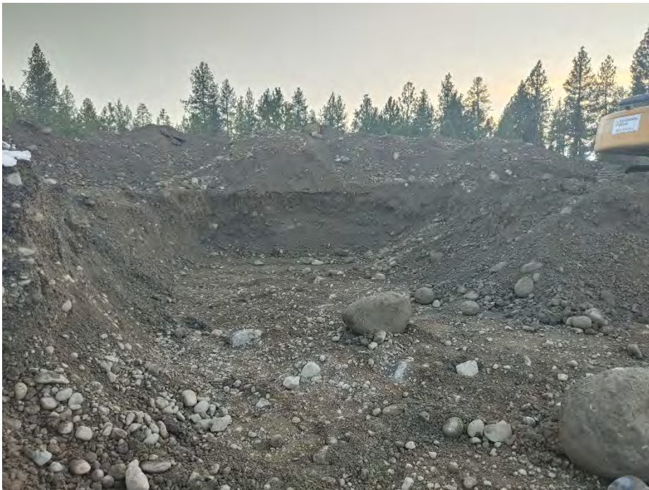
Photograph 3: Southern expansion of Excavation 8 at its southeastern extent at the end of 12/9/2022. Expanded approximately 20'x15'x6' with visible cross still approximately 3 ft bgs at southern wall.
