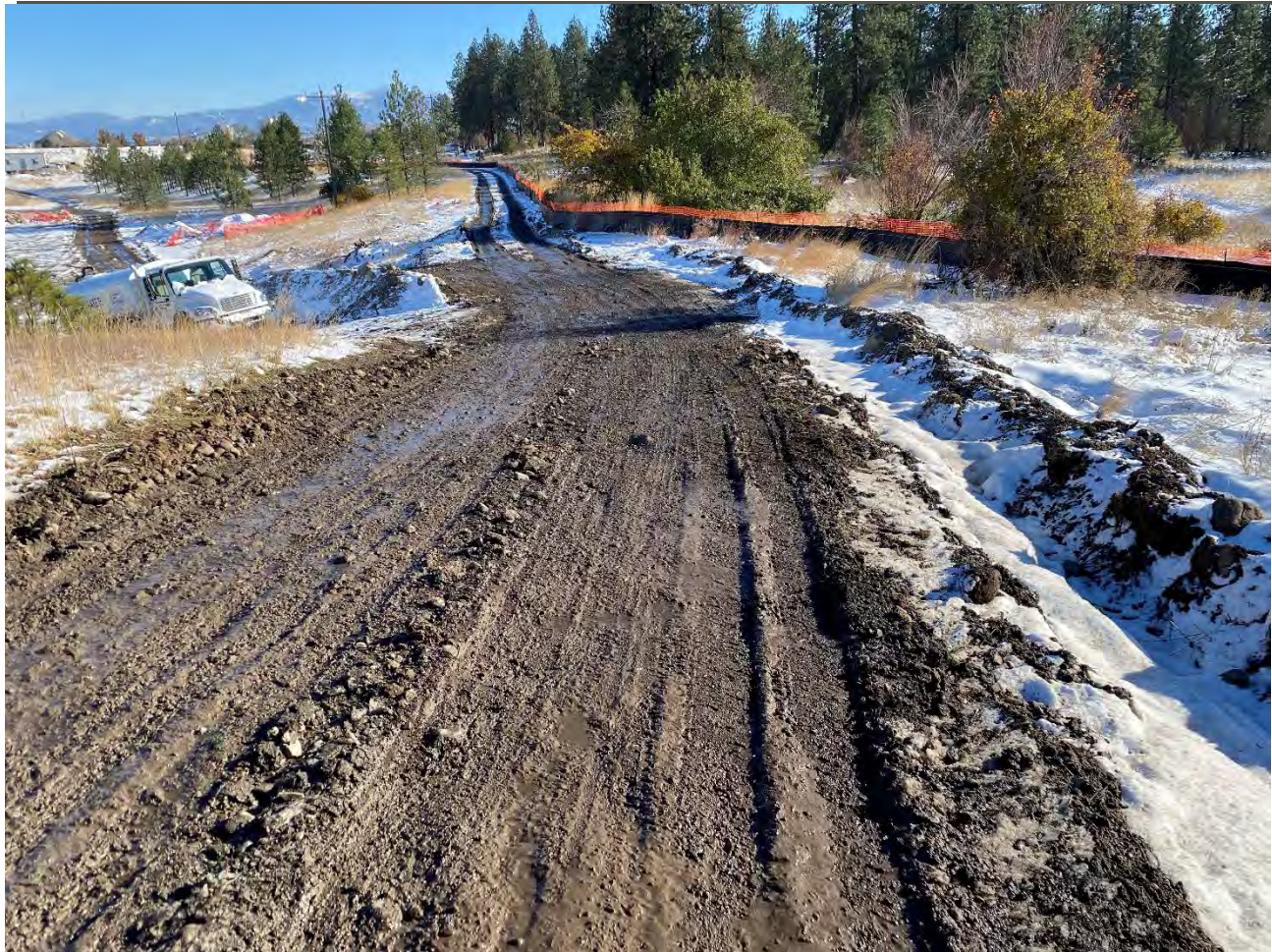
Photo. 3 South haul road thawing out in sun still firm hard pack frozen gravel.
