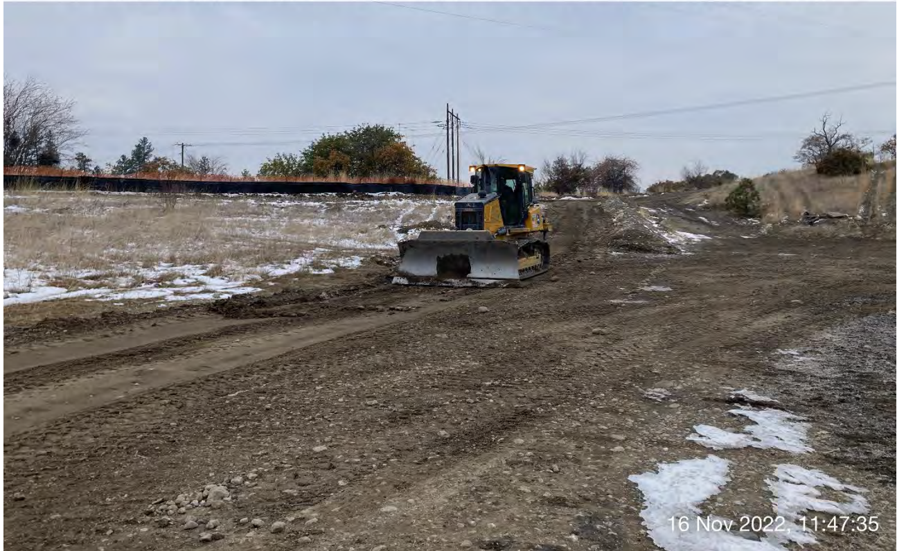
Photo 3: John Deere 700L bulldozer grading haul road.
