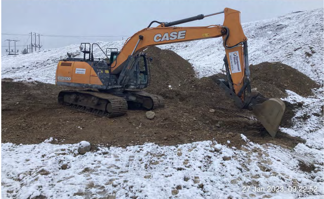
Photograph 2: Excavation of 2-foot cut area on WSDOT property north of Excavation 6.
