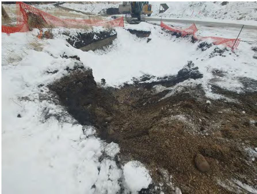
Photograph 1b: Finished expansion of eastern south wall of Excavation 5.
