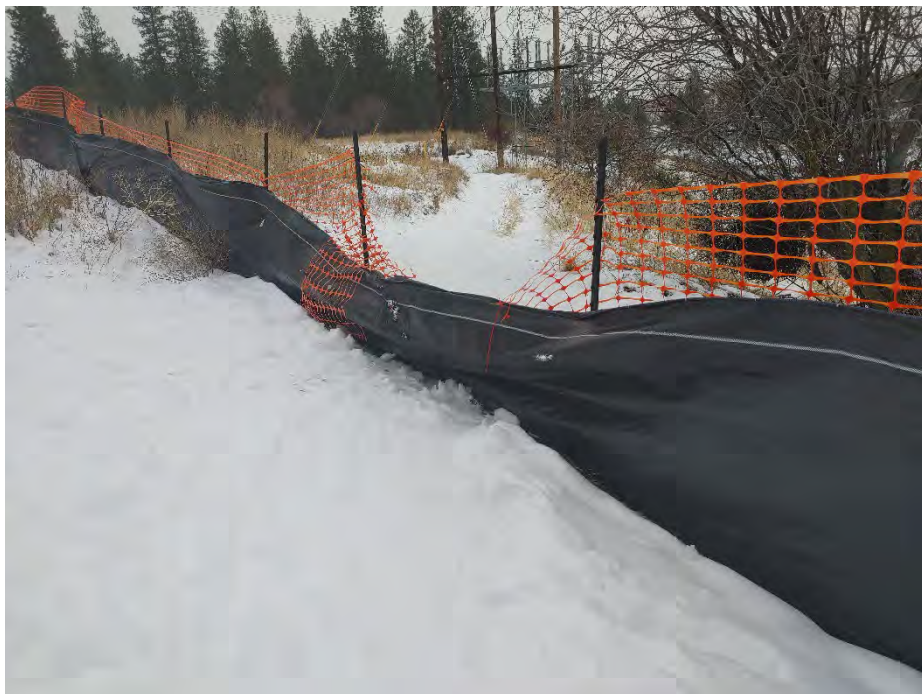
Photograph 2b: Attempted silt fence repair near trail at western edge of the site.
