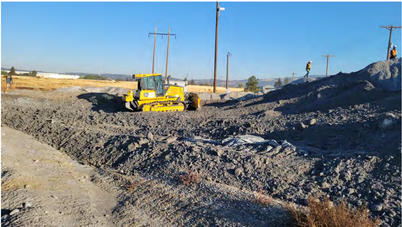
Photo 3. Bulldozer grading out future loading area.
