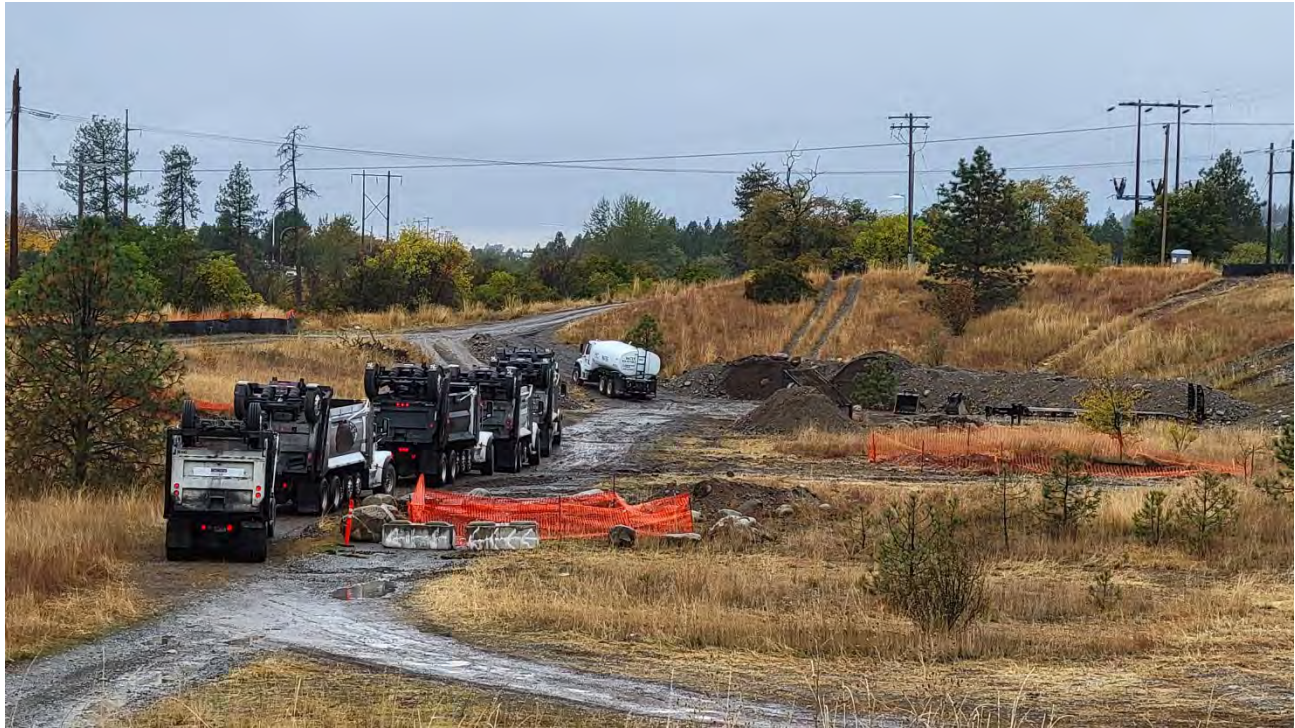
Photo 7. Line of trucks waiting to access loading area.
