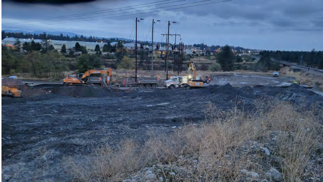
Photo 1. Excavators working on Pentzer property.
