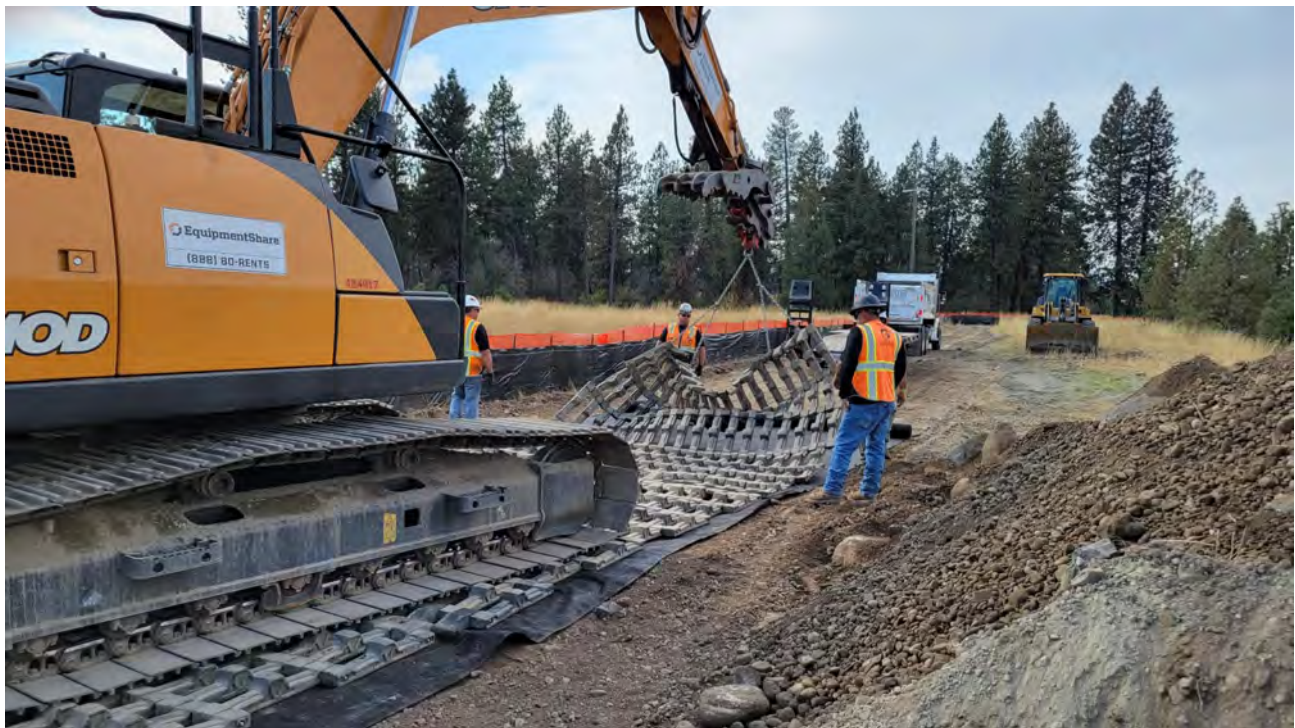
Photo 4. Placing three sets of truck rumble mats.
