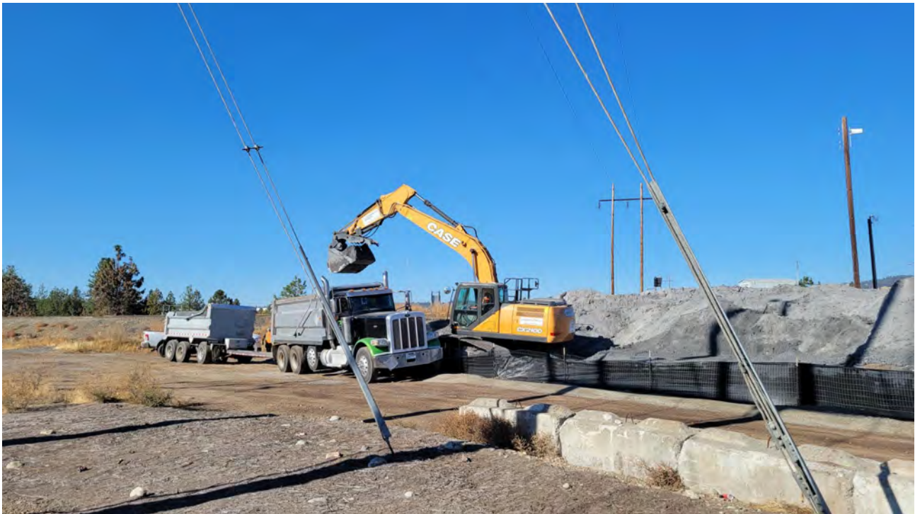
Photo 7. Tenth truck overall for the day being loaded at approximately 2:30 pm.
