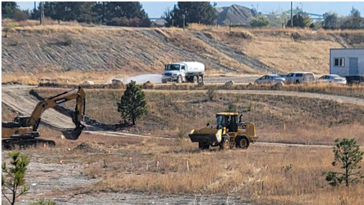
Photo 3. Excavation on WSDOT deep digs begins
