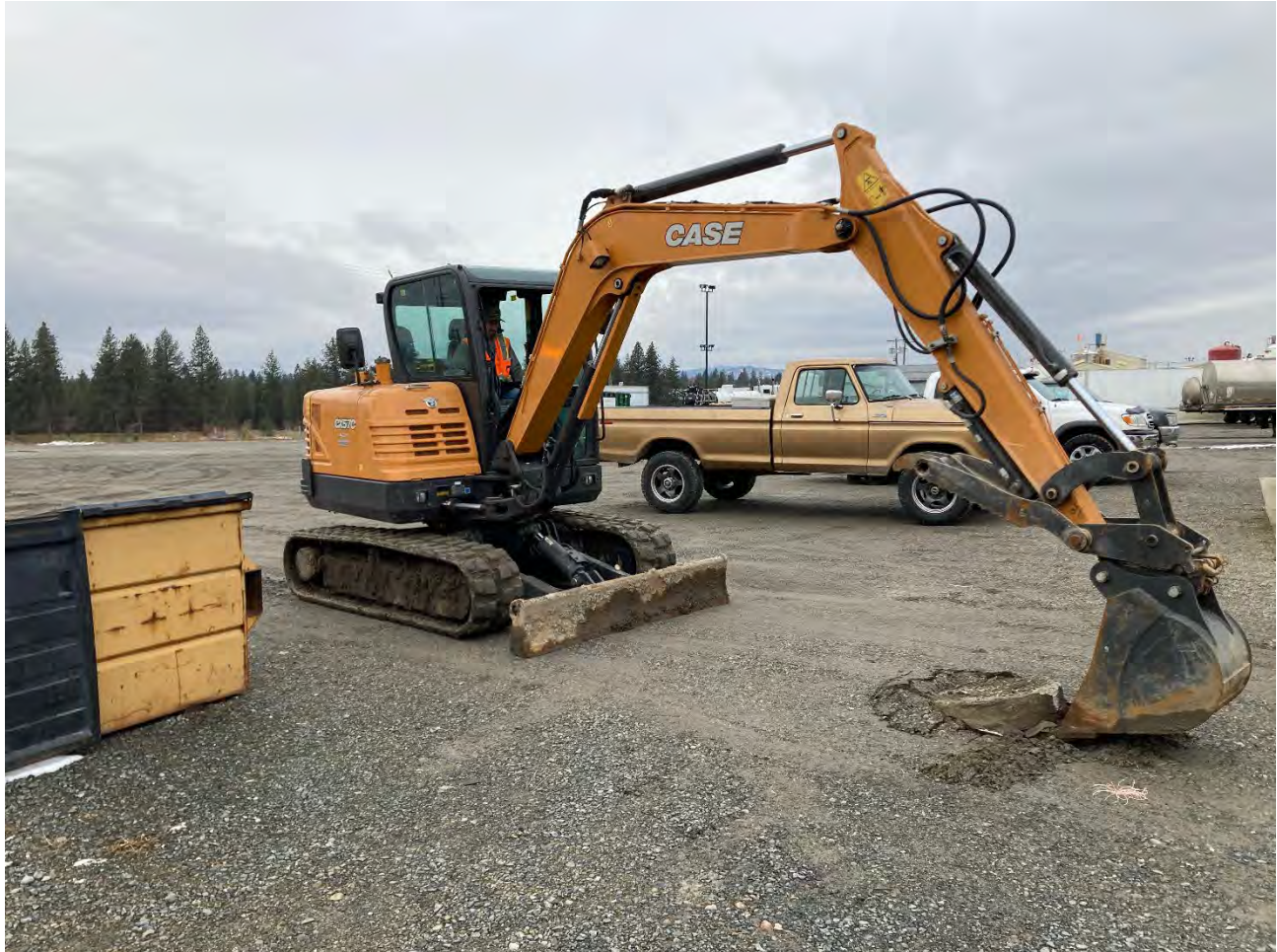
Photograph 1: Removal of MW-1 monument to complete well removal task.
