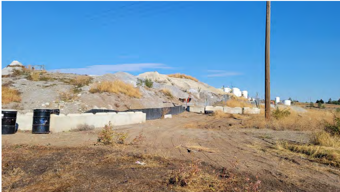
Photo 1. SW corner of dross pile, with drainage blocks in the background.
