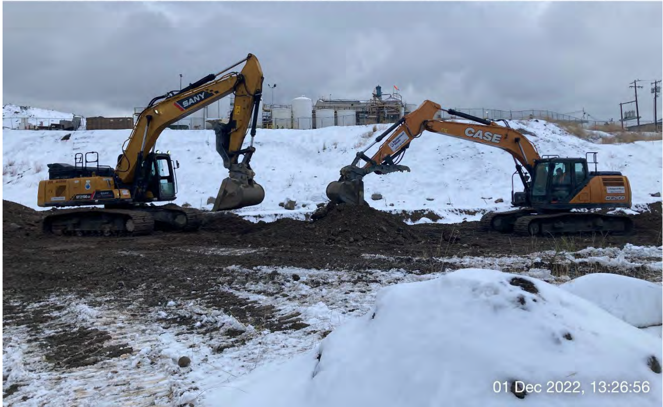
Photo 2: Sany 215C LC and CASE 210D trackhoes moving material excavated from Excavations 8 and 9 to the temporary storage pile near planned Excavation 4.
