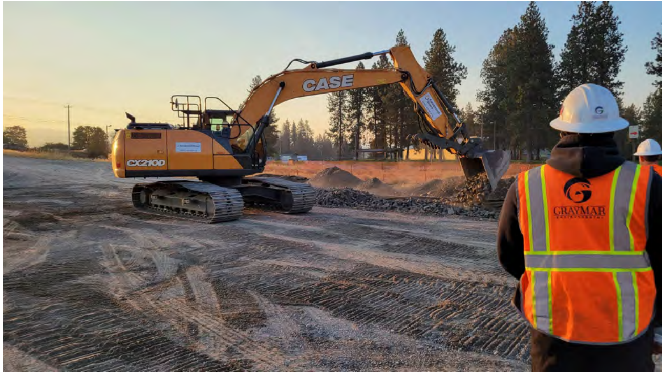
Photo 3. Quarry spalls being placed for truck ramp.
