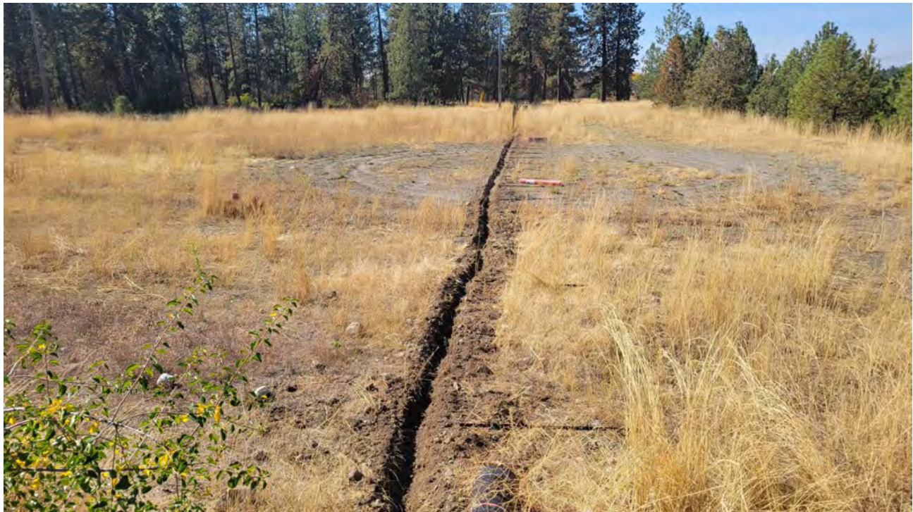
Photo 1. Trench for silt fence extending west from office trailer.
