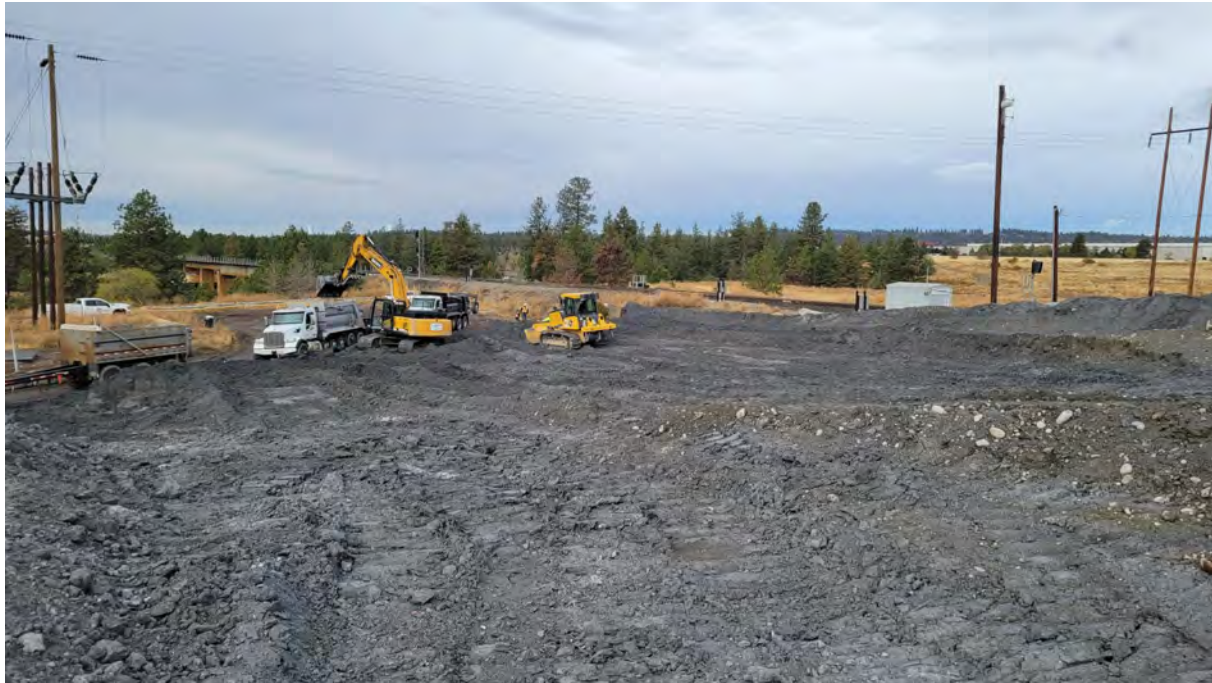
Photo 4. Bulldozer pushing dross to two excavators.
