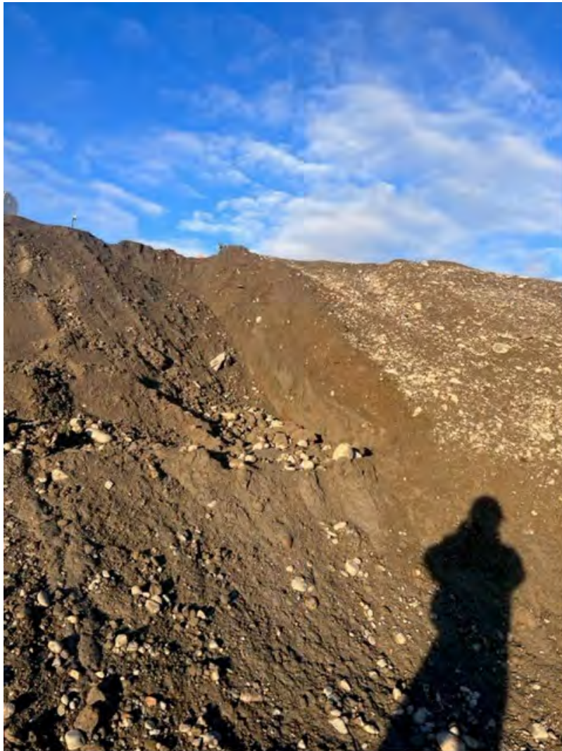
Photograph 1. Dross removal from slope below Kemira
