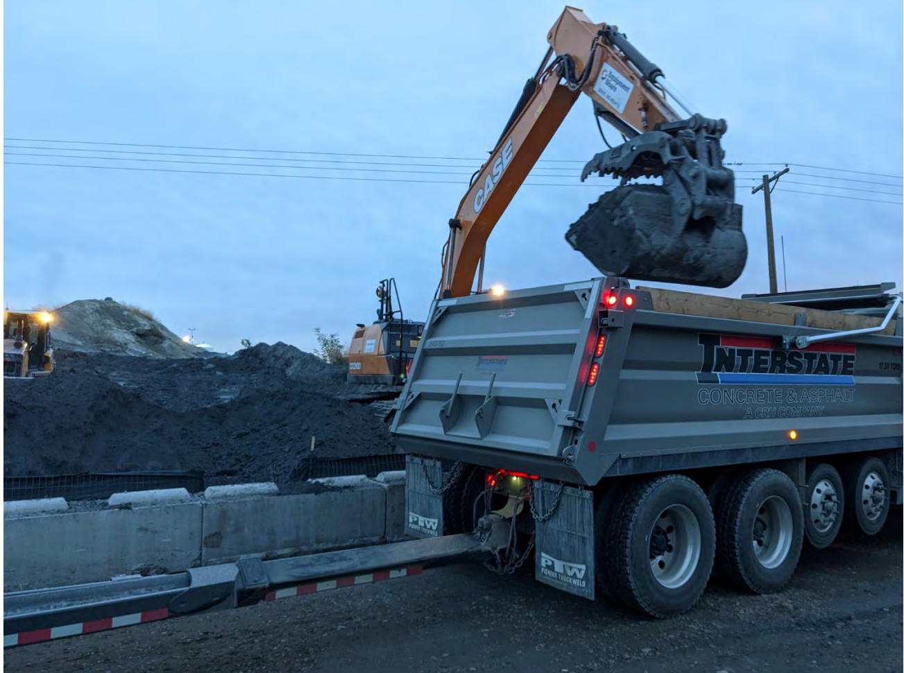
Photo 1. Excavator loading first trucks of the day.
