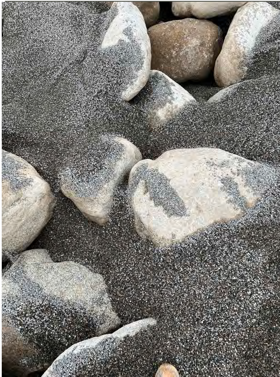
Photograph 2: Placement of backfill between boulders in WSDOT excavations.
