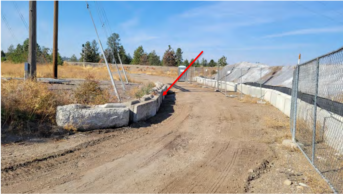
Photo 6. Ecology blocks placed around guy wires to protect from truck traffic.
