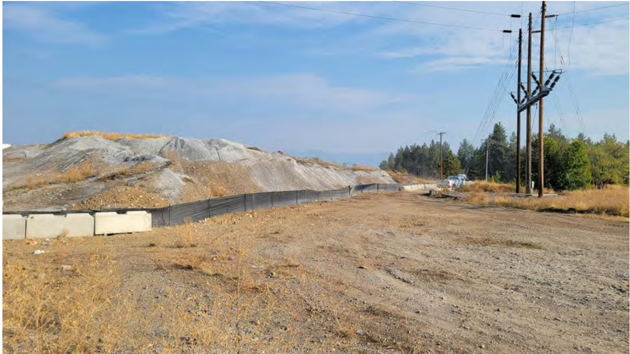
Photo 10. Temp fence and ecology blocks removed from west end of dross pile for use elsewhere. Silt fence is maintained.
