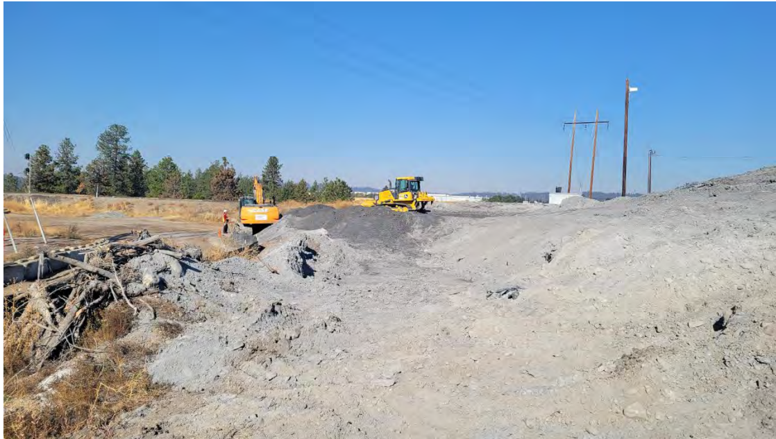
Photo 2. Progress on lowering western edge of pile.
