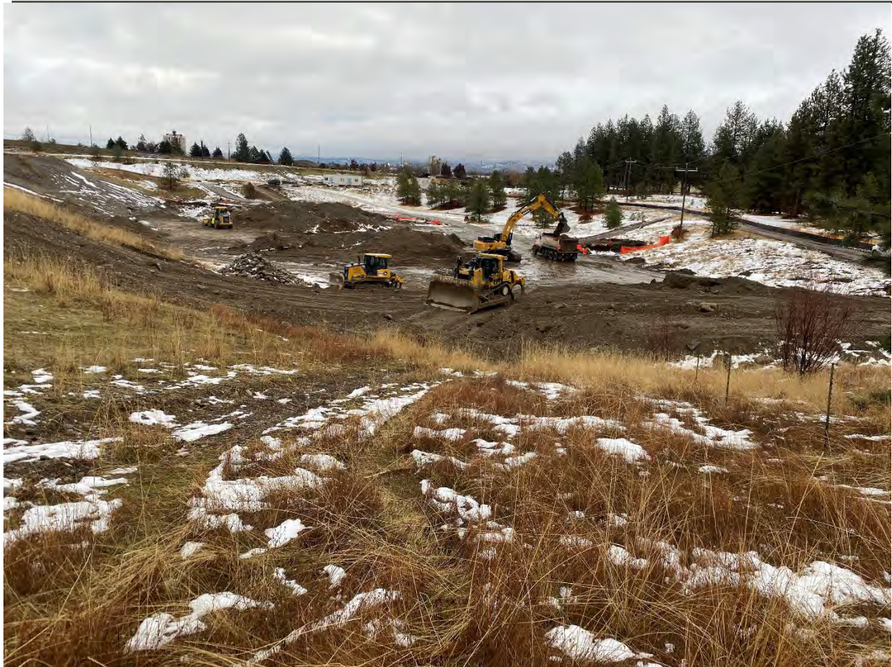
Photograph 2. Placing off-property excavated soil from WSDOT onto UPRR sloped industrial area.
