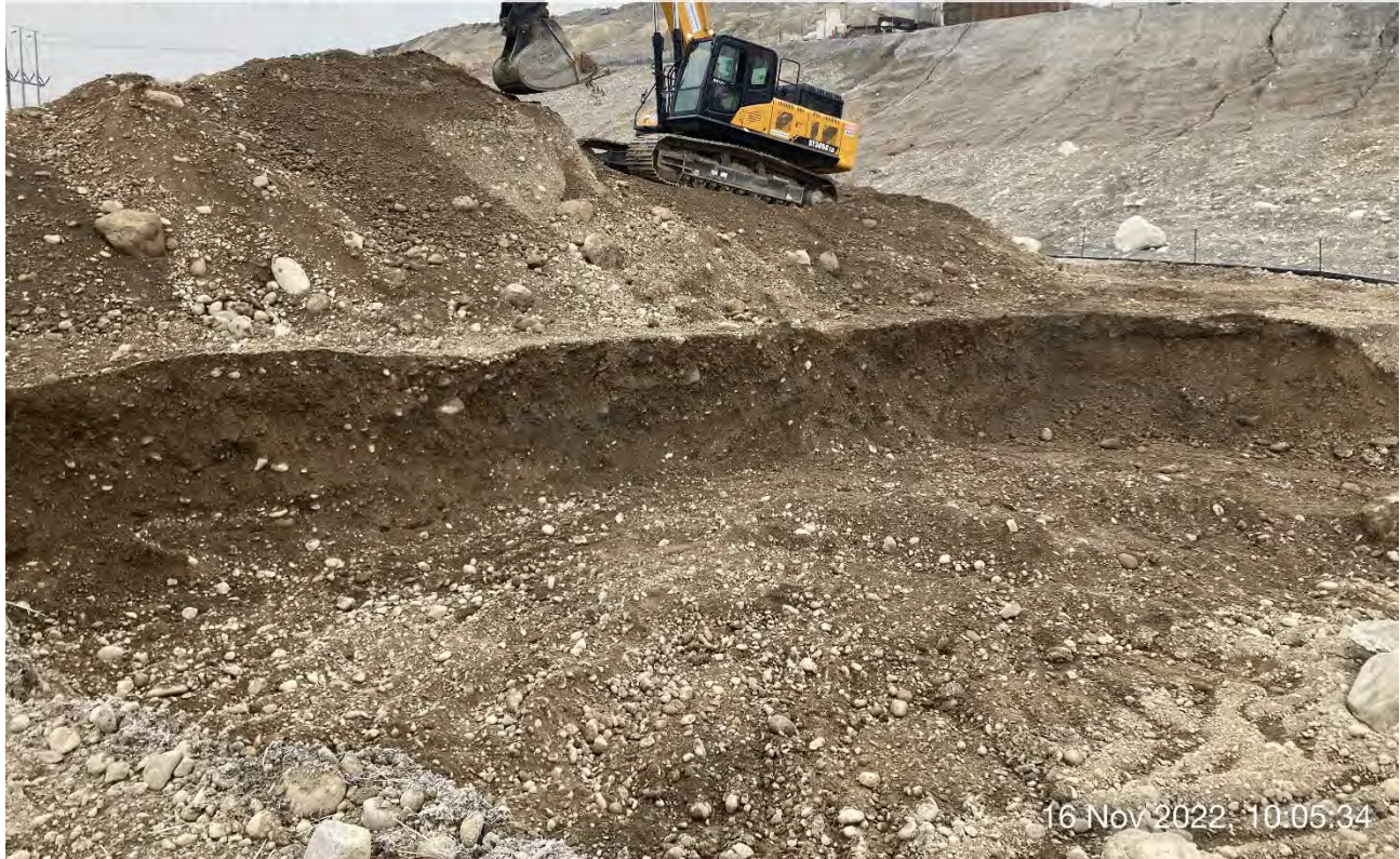
Photo 2: West side wall of excvation #8 facing northwest, 6-feet deep.
