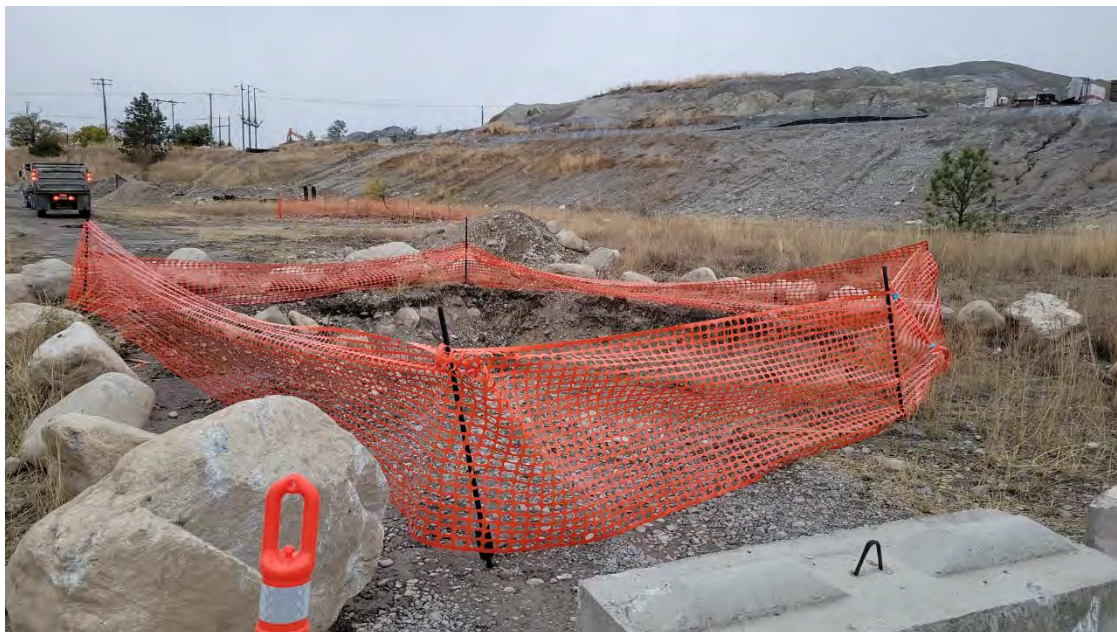
Photo 2. WSDOT #7, also excavated 10/21/22.
