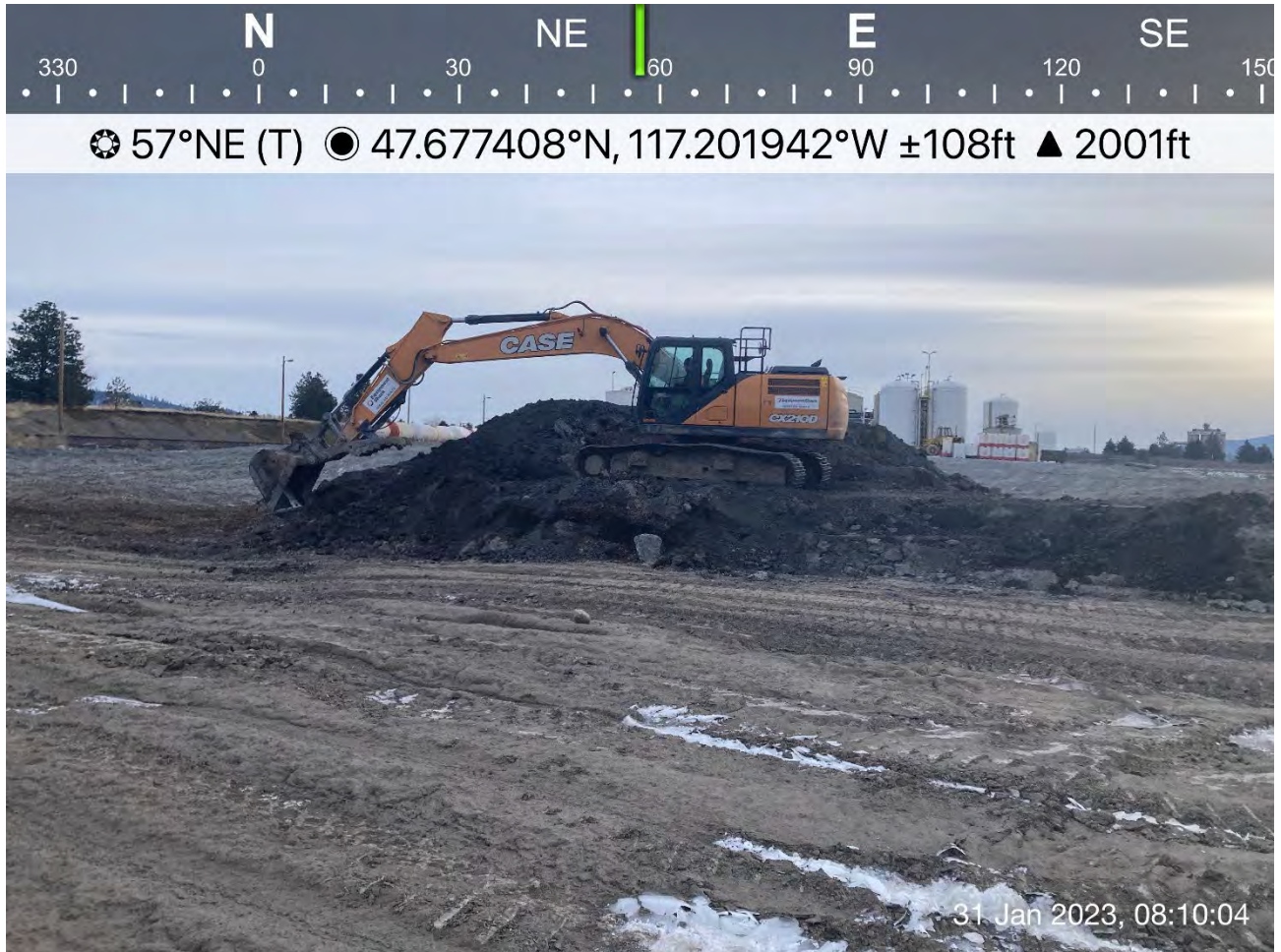
Photograph 2: Loadout activities at the cross pile located on UPRR property.
