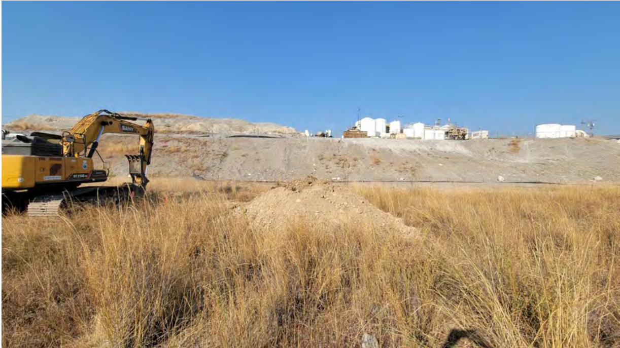
Photo #8. Spoils pile at WSDOT #6. Almost no rocks over 1 foot diameter.
