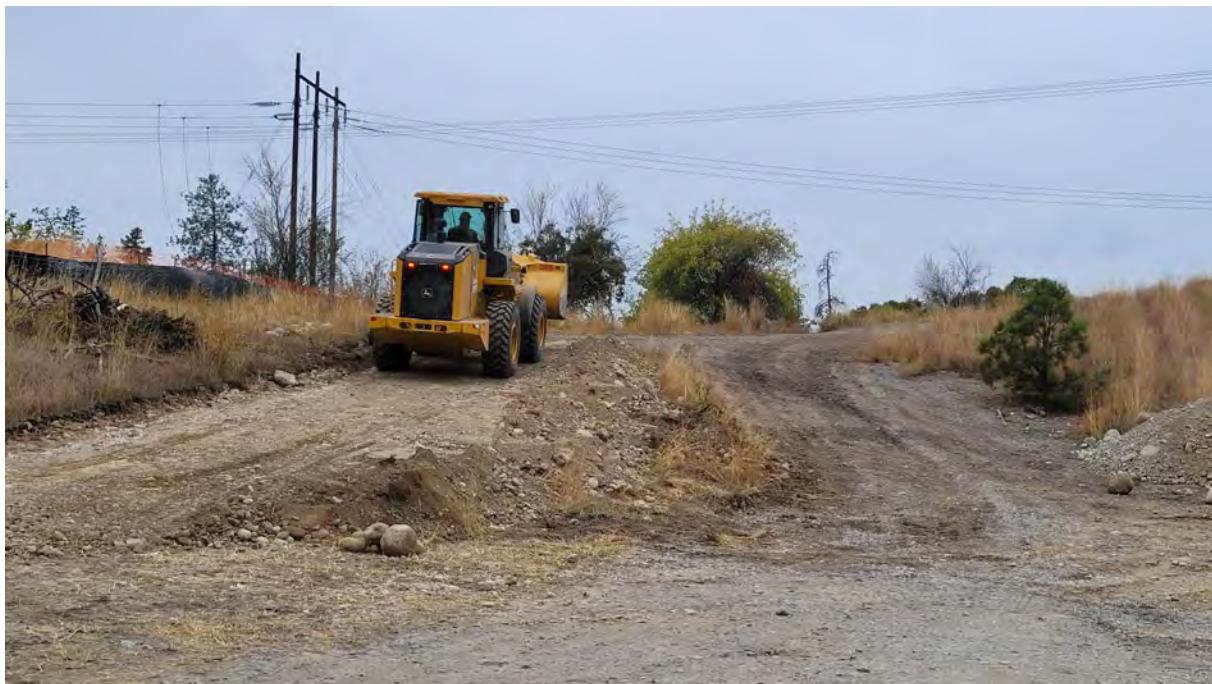
Photo 4. New in-bound haul road ramp.
