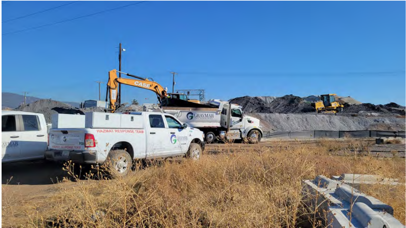
Photo 6. Loading of first truck.
