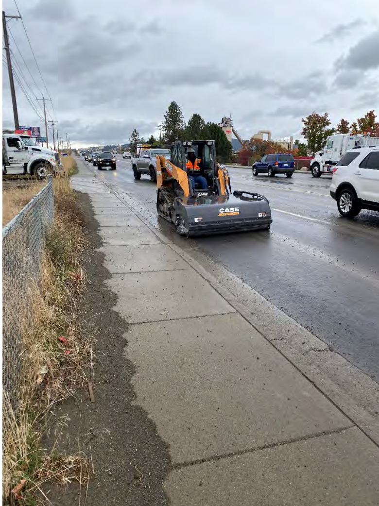
Photo 3. Sweeper entering traffic removing rock from Sullivan, Next pass used a truck with flashing lights behind sweeper for rear escort.
