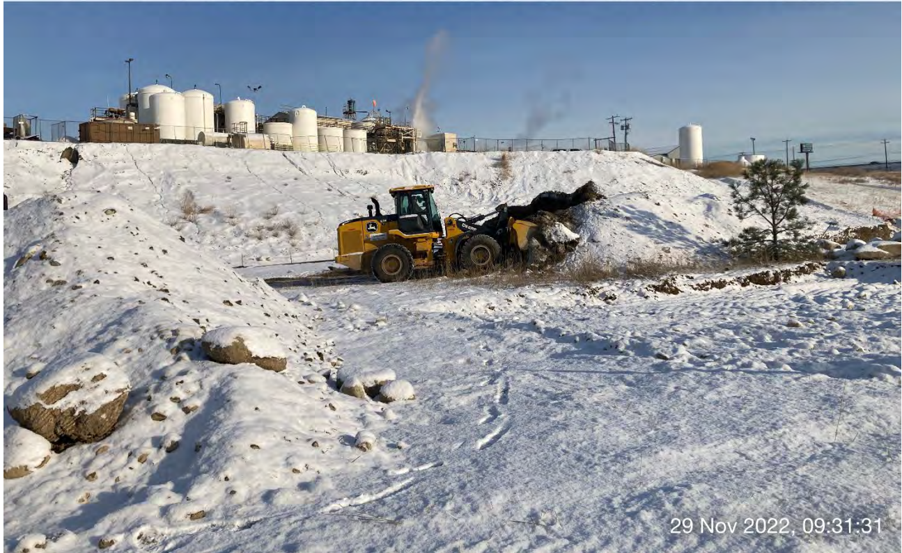
Photo 2: John Deere 624 front-end loader moving excavated material from the pile located west of Excavations 8 & 9 to a location near planned Excavation 4.
