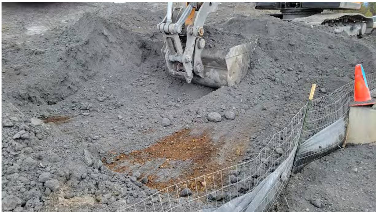
Photo 5. Excavator reaching bottom of dross stockpile.
