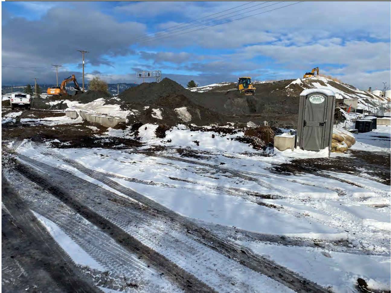
Photo 2. Bulldozer pushing dross to prepare for Tuesday load out.
