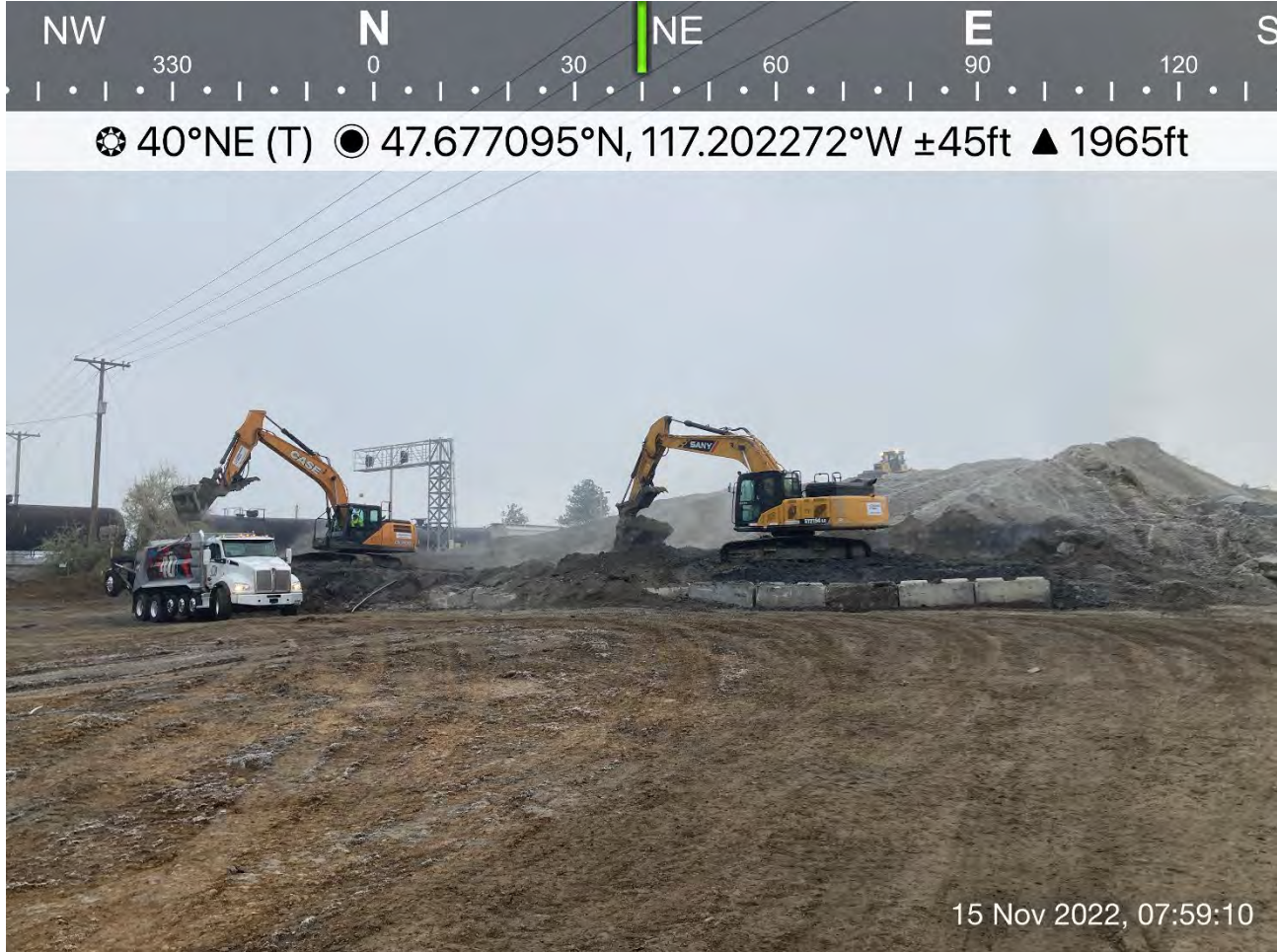
Photo 1: Loading of dross into a haul truck at the dross pile. Steam is observed in this photograph due to the temperature difference between the air and the dross.
