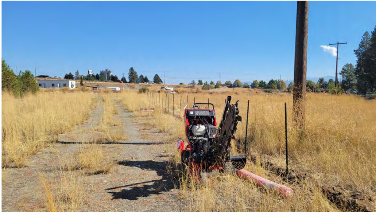
Photo 2. Trencher looking back at trailer.
