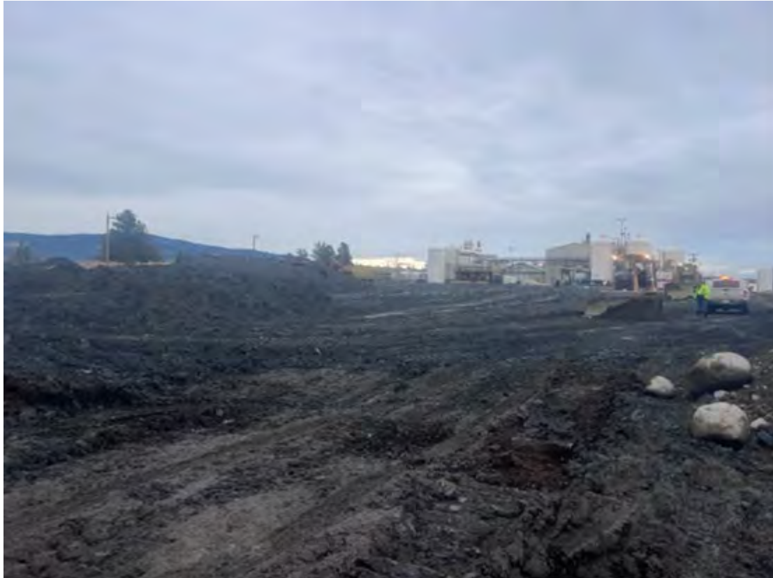
Photograph 1: Dross removal progress.
