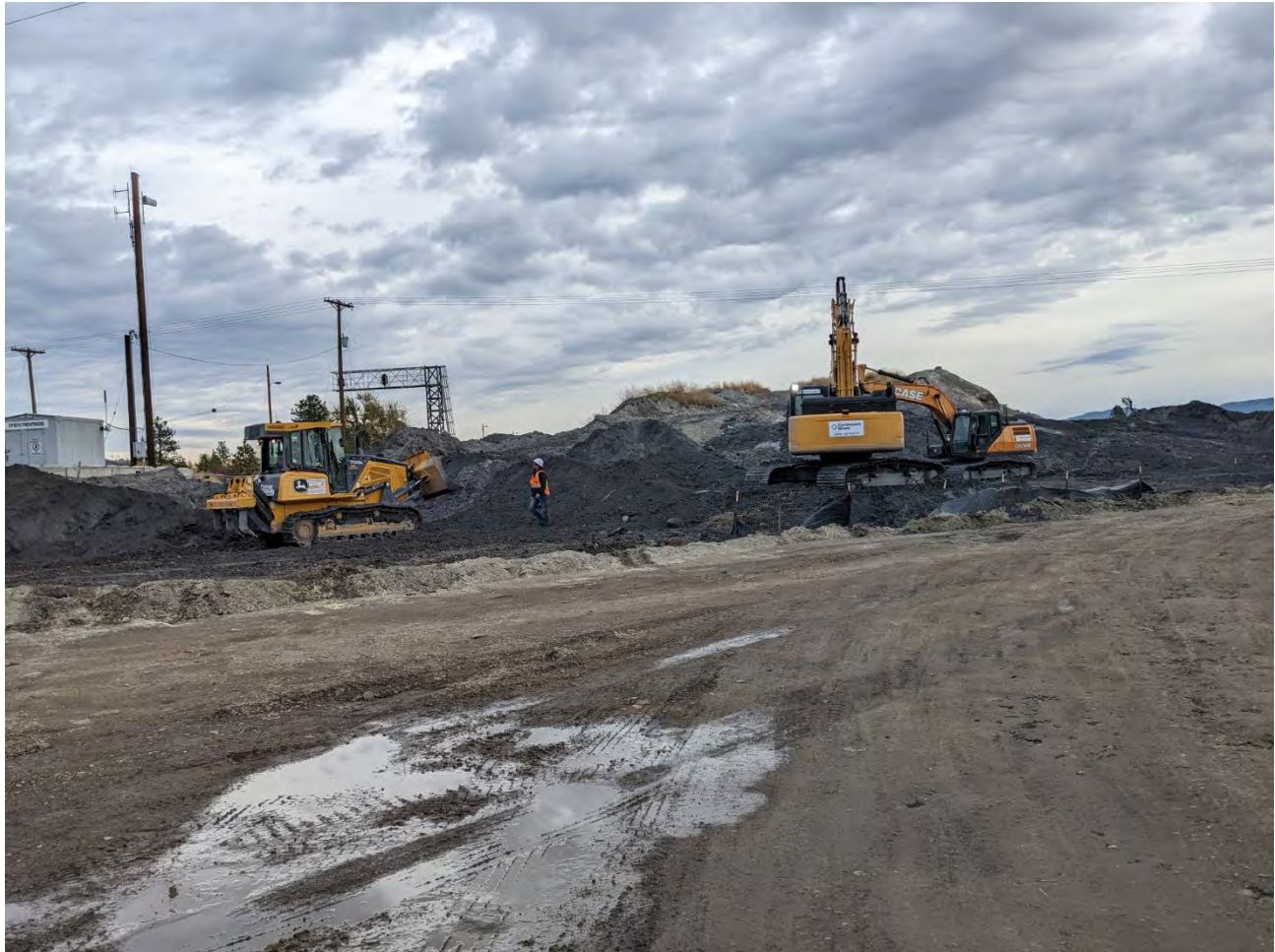
Photo 2. Bulldozer pushing dross to two excavators.
