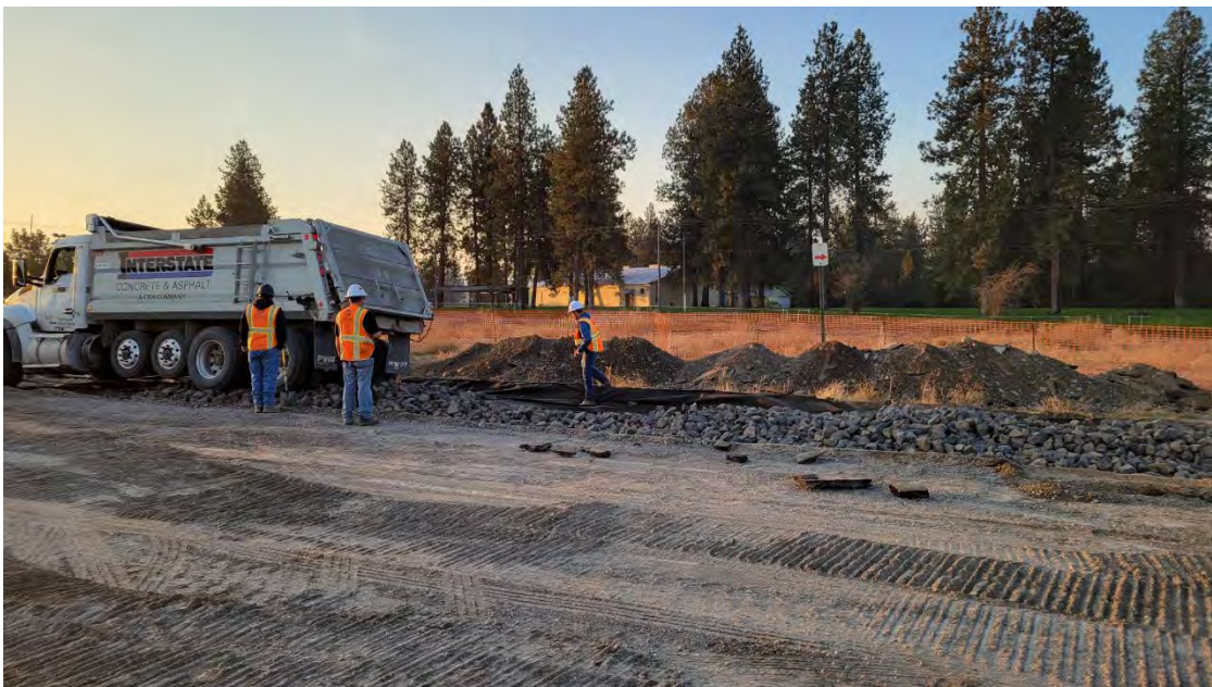
Photo 2. Quarry spalls being dumped for truck ramp.
