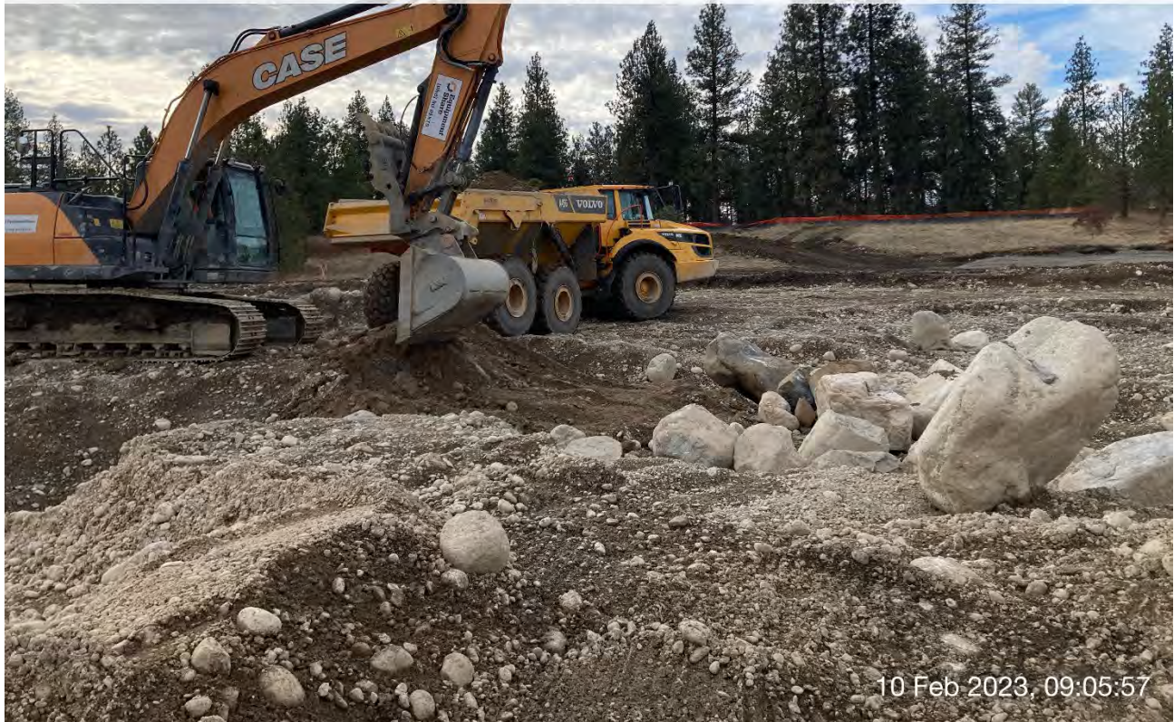
Photograph 2: Excavation of area between Excavation 6 and Excavation 8 that exceeded CULs.
