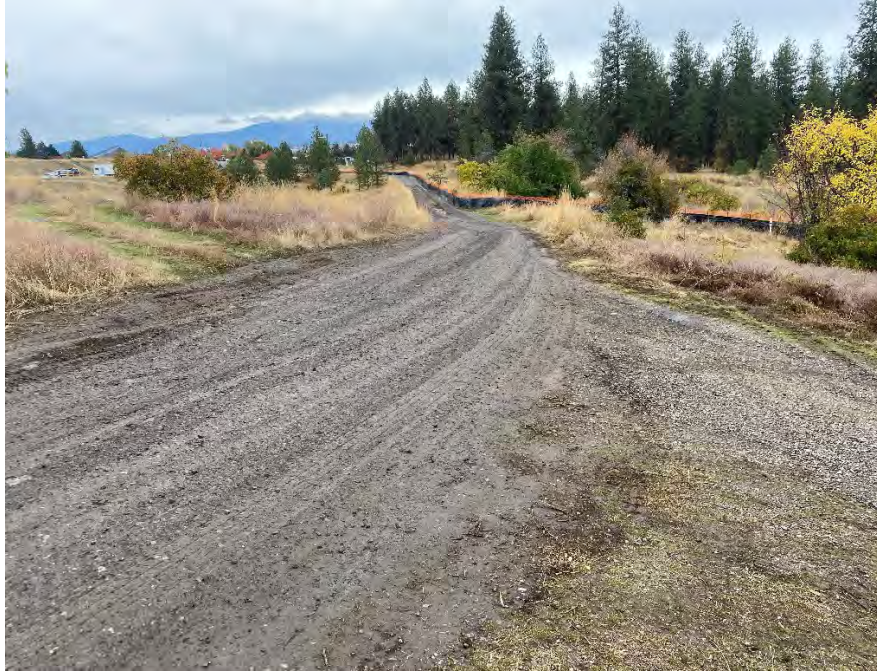
Photo 1. South haul out road damp from rain minimizes dust.
