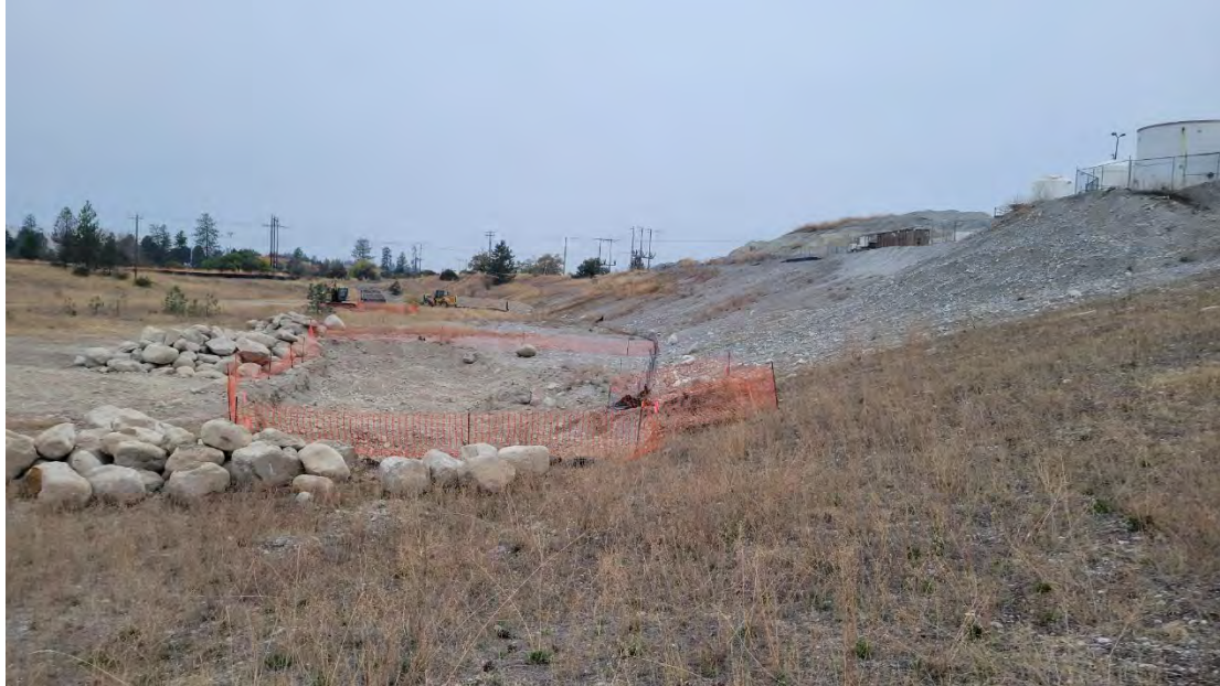
Photo 1. Security fence installed around WSDOT excavations.
