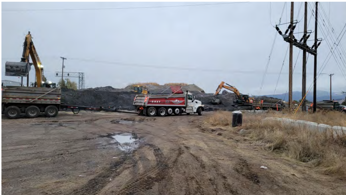
Photo 4. GrayMar modified operations to load two with two excavators.
