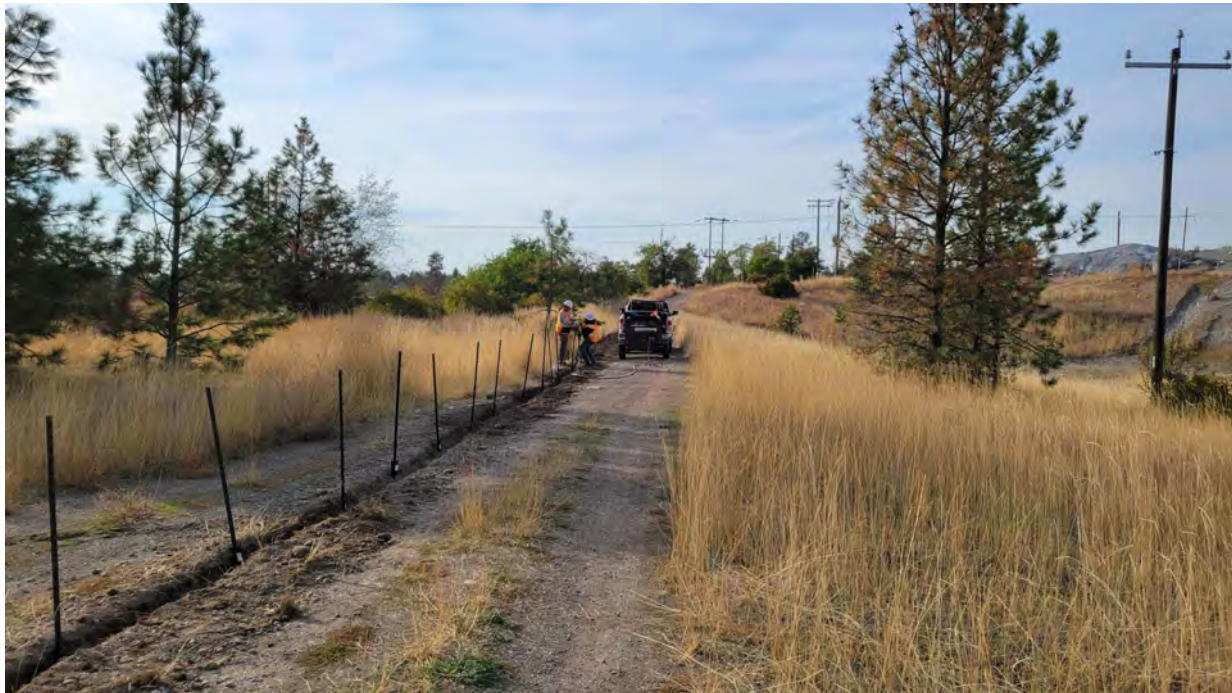
Photo 7. Looking west, crew installing silt fence posts.
