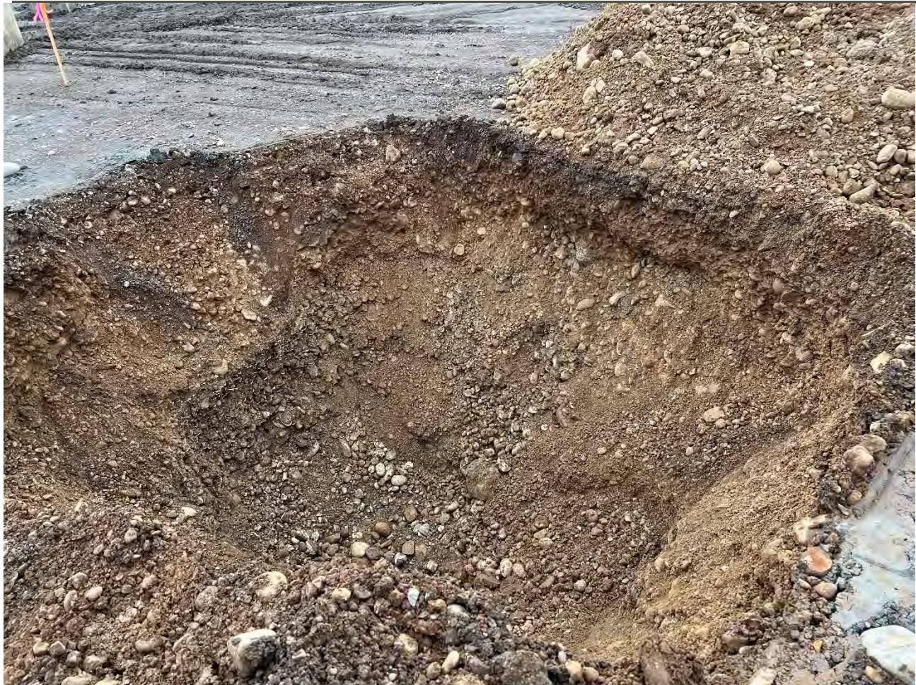
Photograph 5: Excavation down to 6ft bgs at unknown underground utility location.
