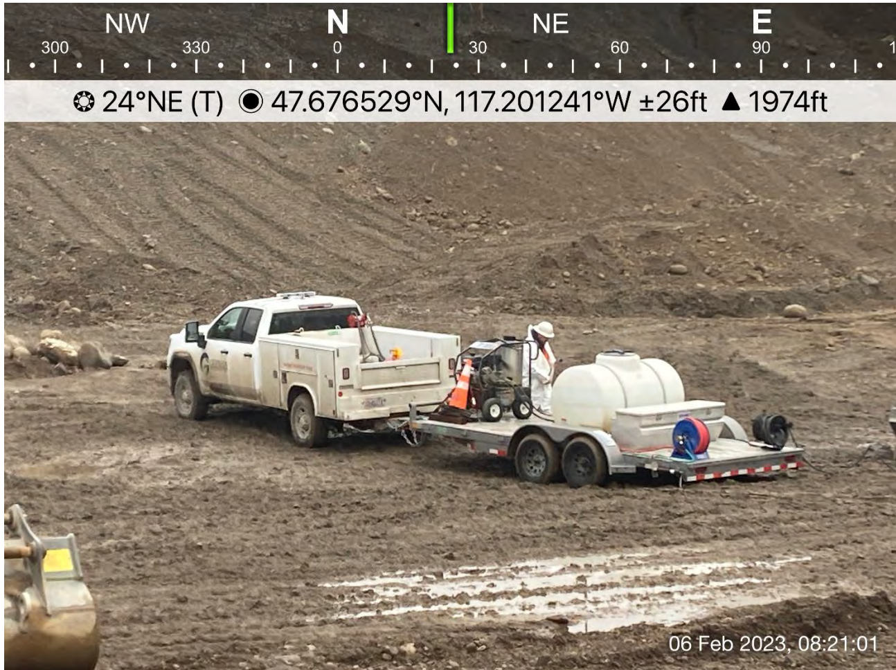
Photograph 1: Trailer-mounted pressure washer used to clean the LinkBelt 145x4 prior to its removal from site.
