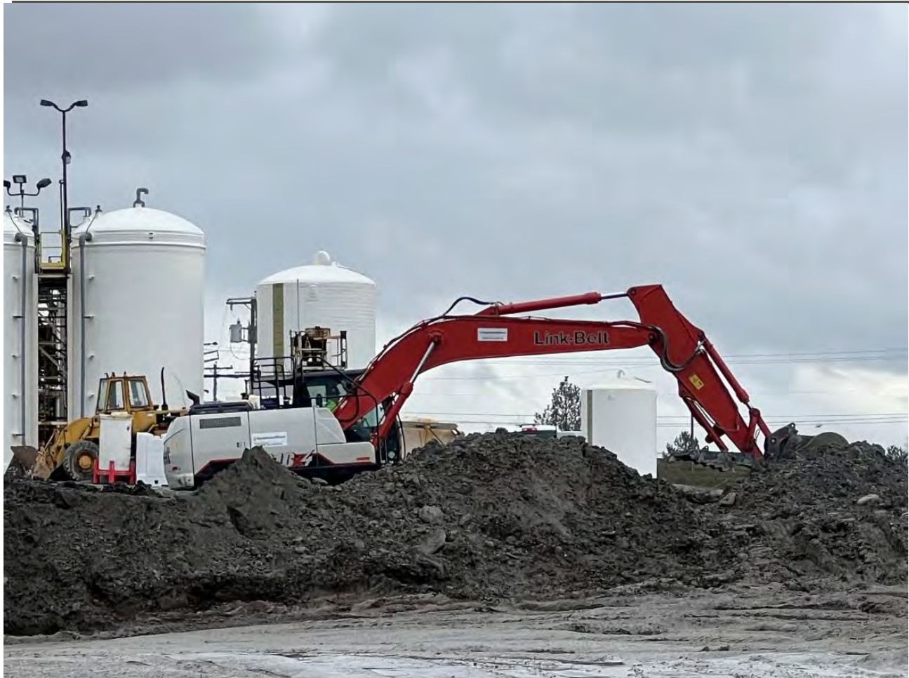
Photograph 3: Replacement trackhoe (LinkBelt 210x4) brought to site on 1/16/2023.
