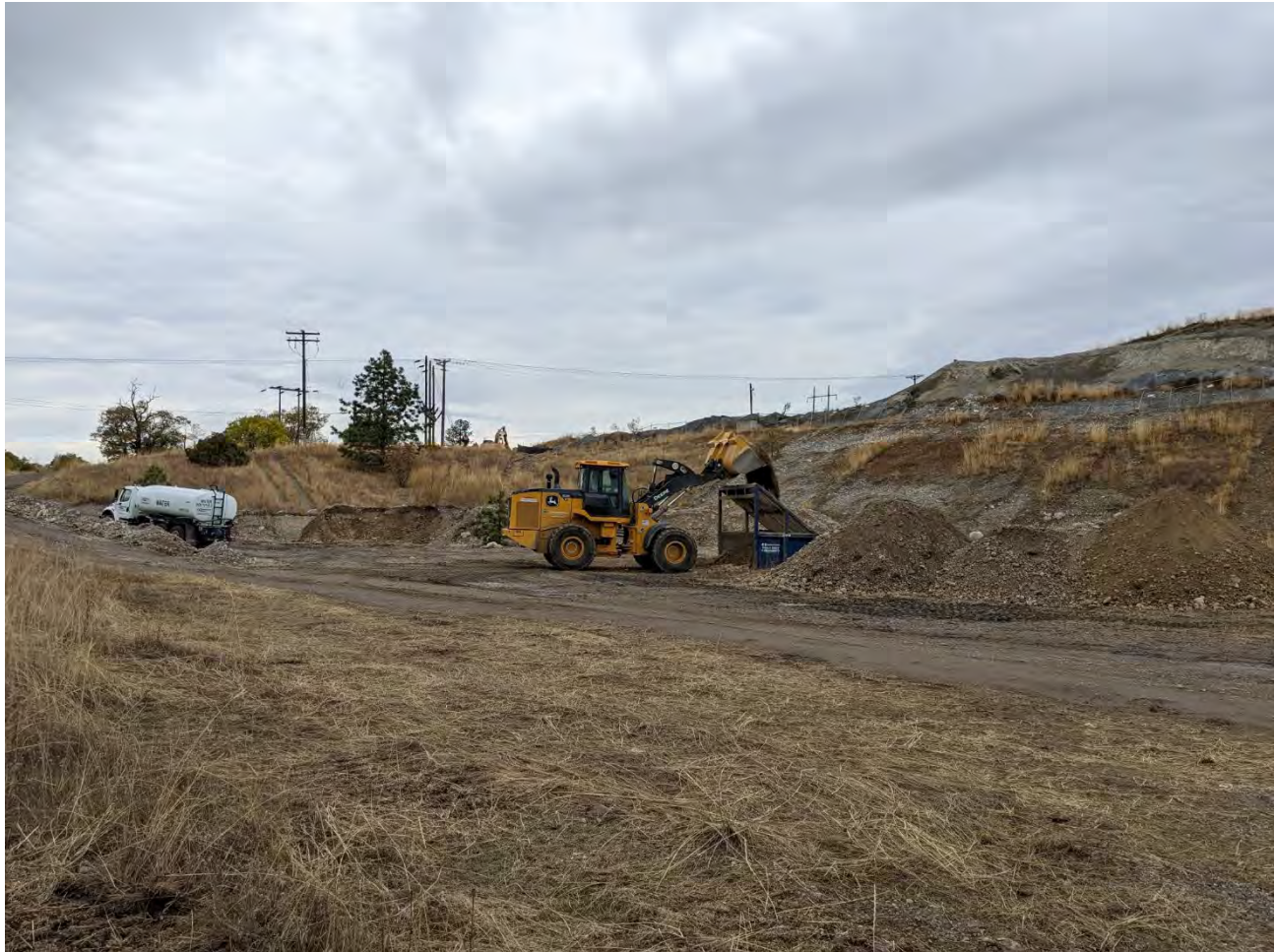
Photo 3. Loader screening excavation stockpiles to remove large rock debris.
