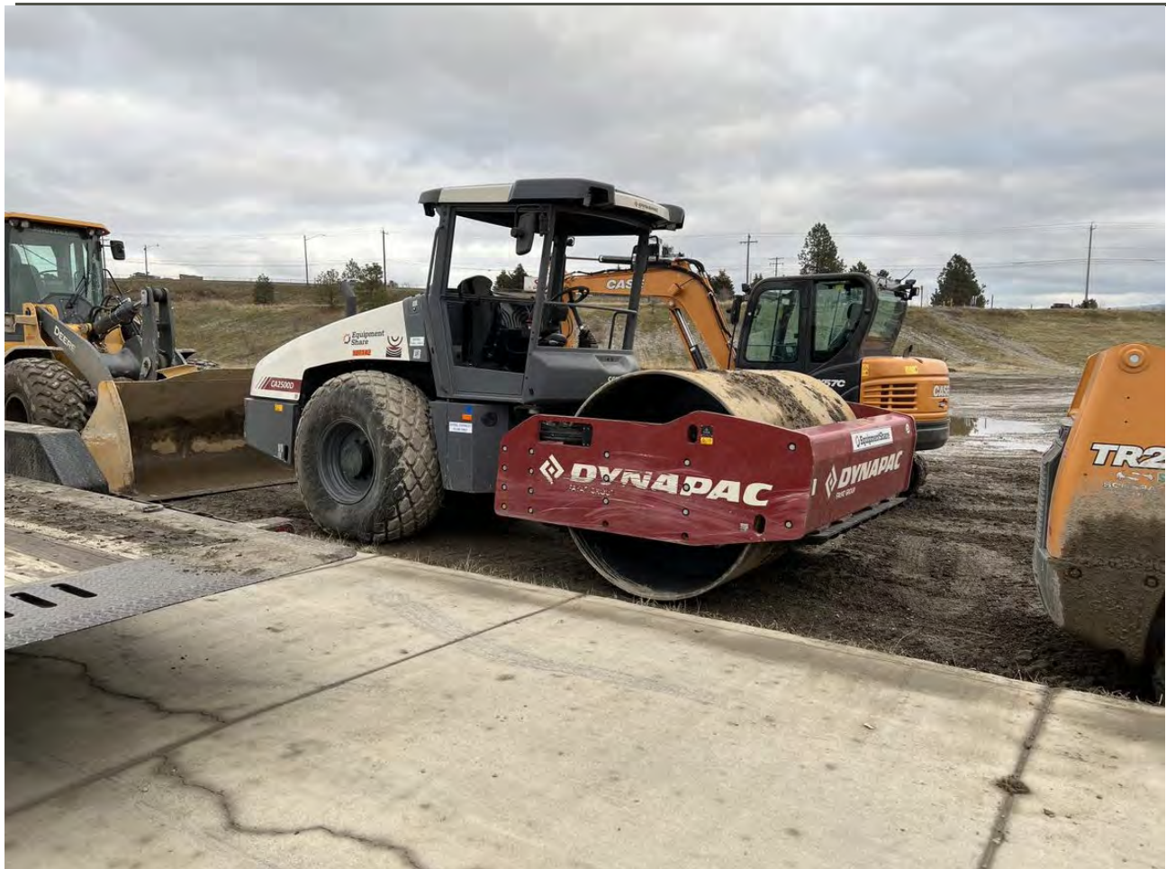
Photograph 2: Roller (DYNAPAC CA2500D) brought to site.
