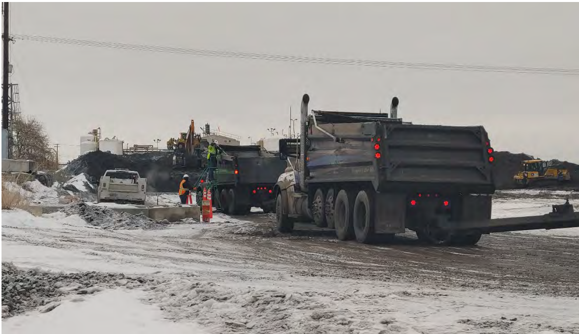
Photograph 1b: Placing plastic sheeting with a telescoping pole.
