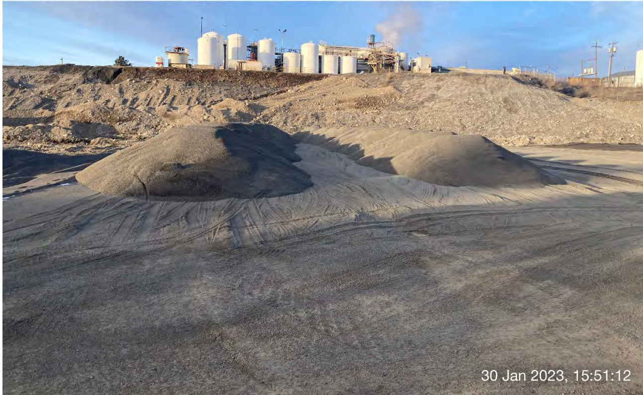
Photograph 3: Backfill stockpile located on filled portions of Excavations 8 & 9 on WSDOT property.
