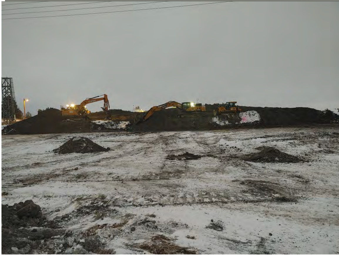
Photograph 4: End of Day at the Dross Stockpile
