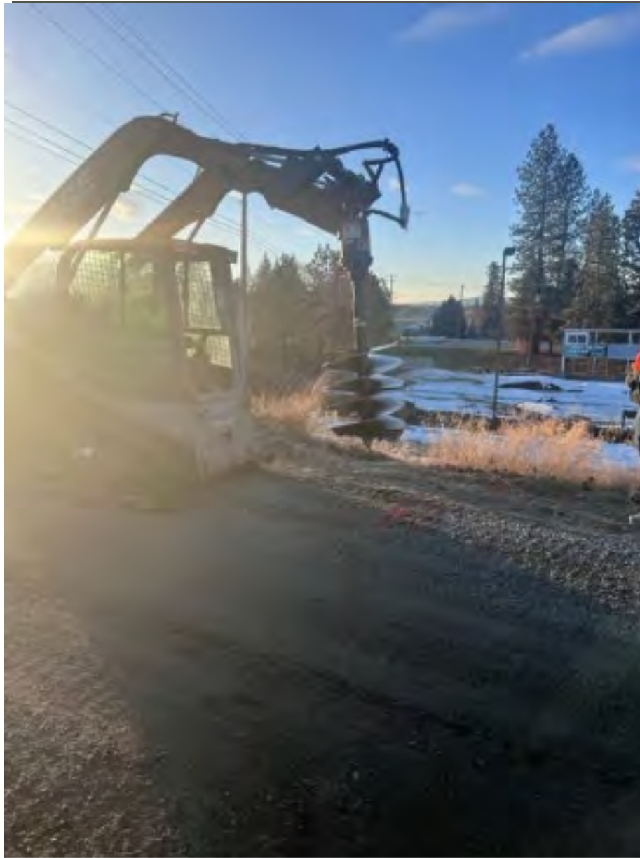
Photograph 2. Auger to install entrance gate on N. Sullivan.
