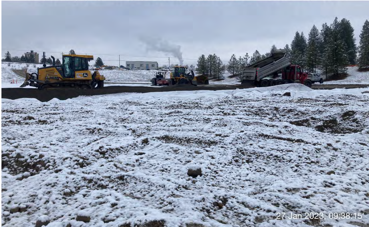
Photograph 3: Backfill activities in Excavations 8 & 9 with clean backfill from approved offsite source.
