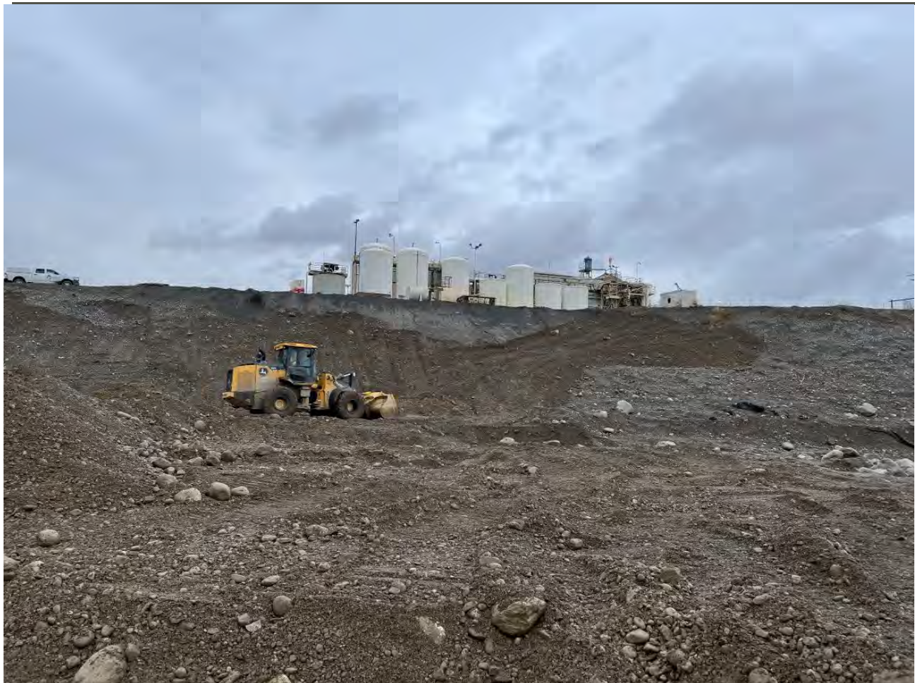
Photograph 4. Stockpiled material at base of slope on WSDOT from excavations 5 through 9.
