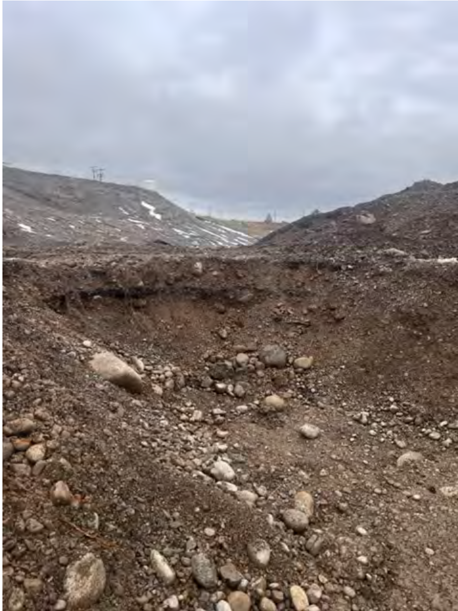
Photograph 1: Over excavation/Sample Location at Excavation 6
