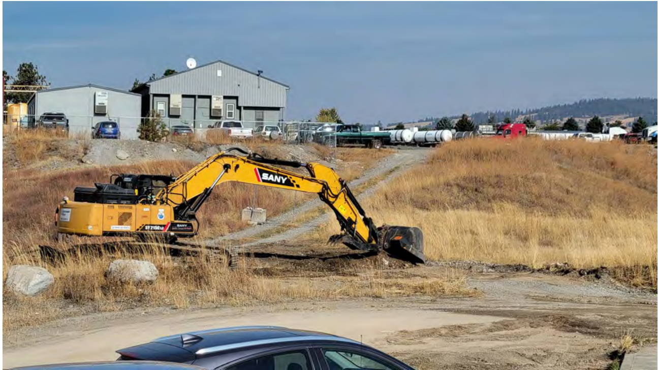
Photo 5. Grading of in-bound haul route on north side of site.
