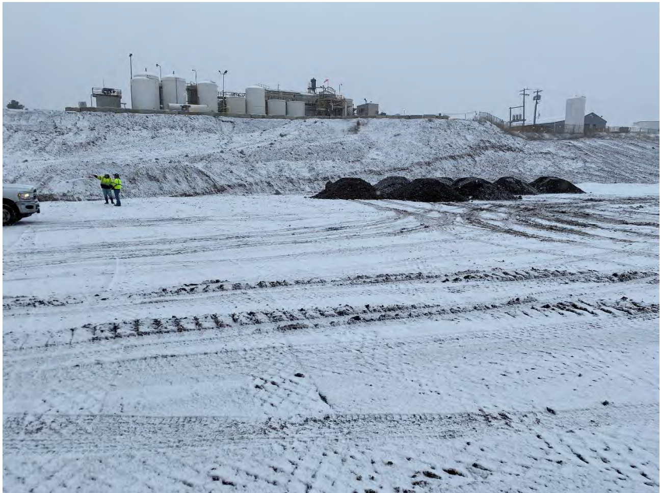
Photograph 1: Placement of backfill #5 on WSDOT.
