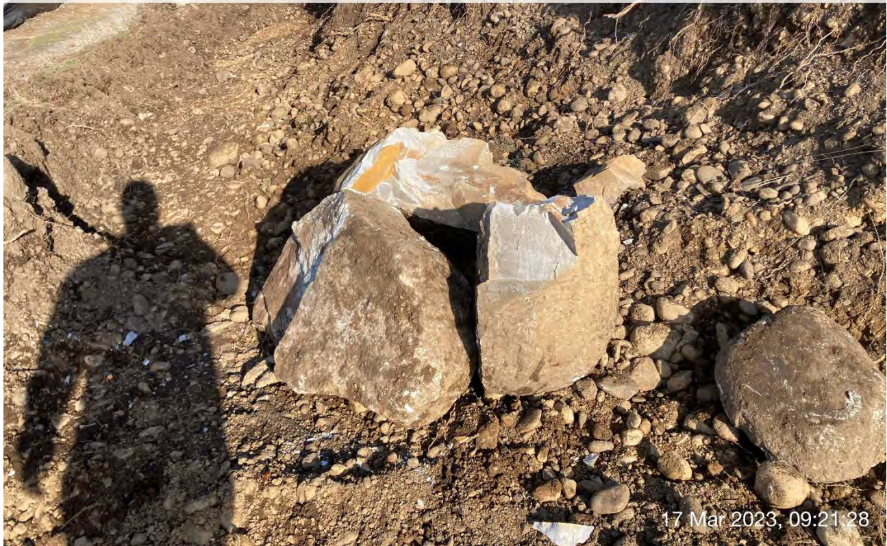
Photograph 2: Broken boulder that caused rock fragments to be sent airborne. A wider berth around the LinkBelt trackhoe was provided after this potential safety hazard occurred.
