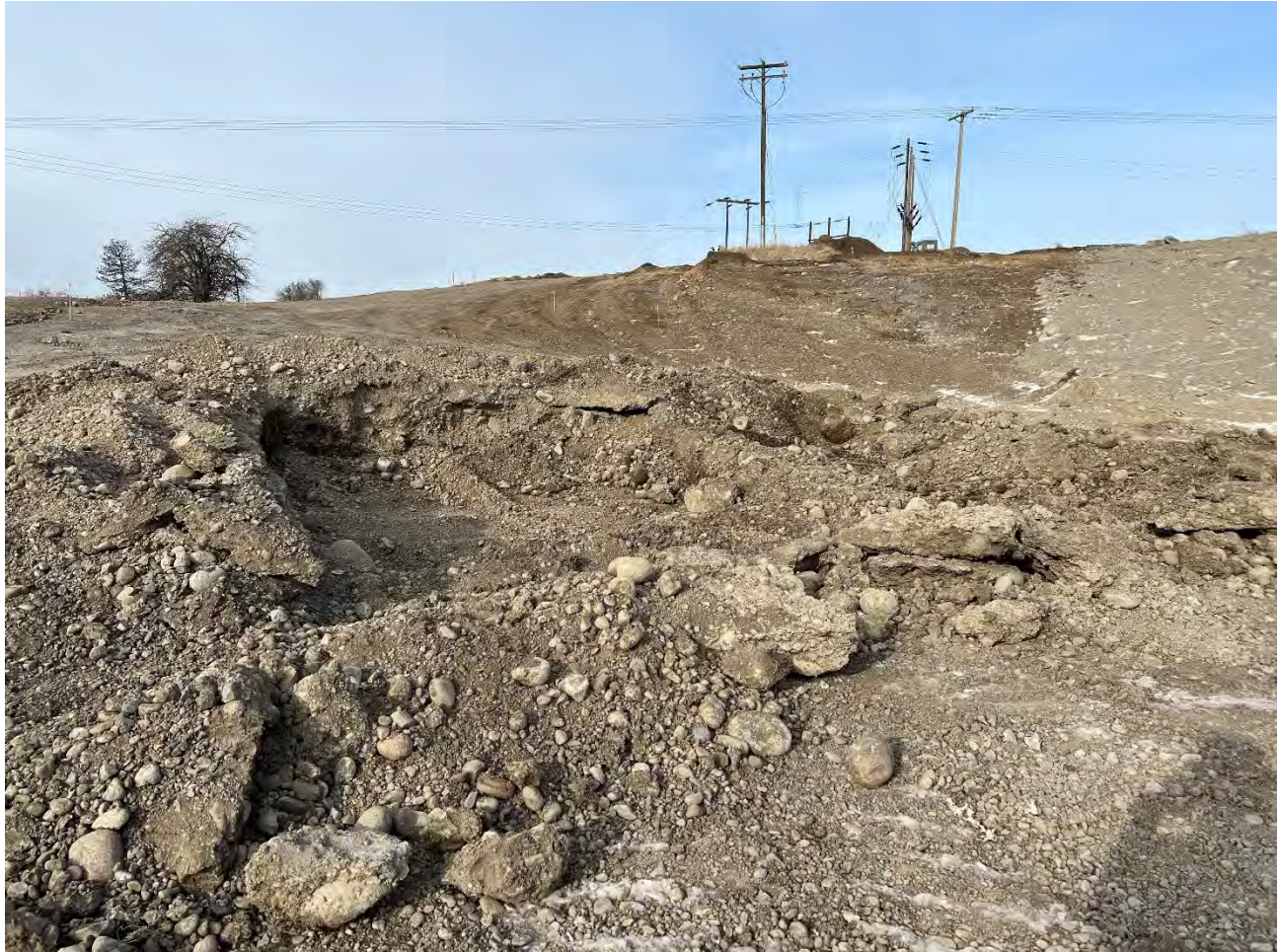
Photograph 1: Excavation 4 with safety berms around edge of excavation.
