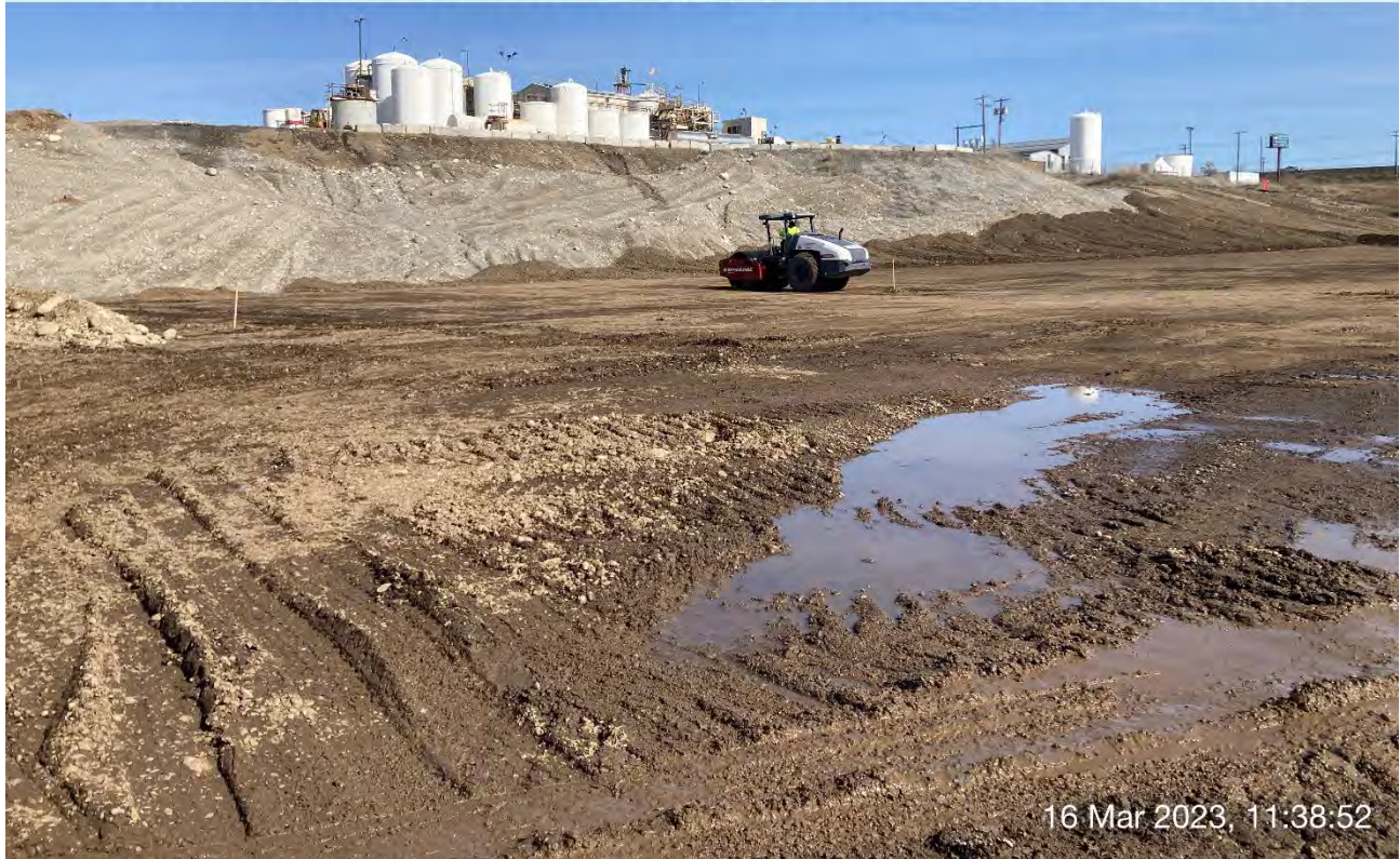
Photograph 6: DYNAPAC CA2500D Roller utilized to compact backfill on WSDOT property.
