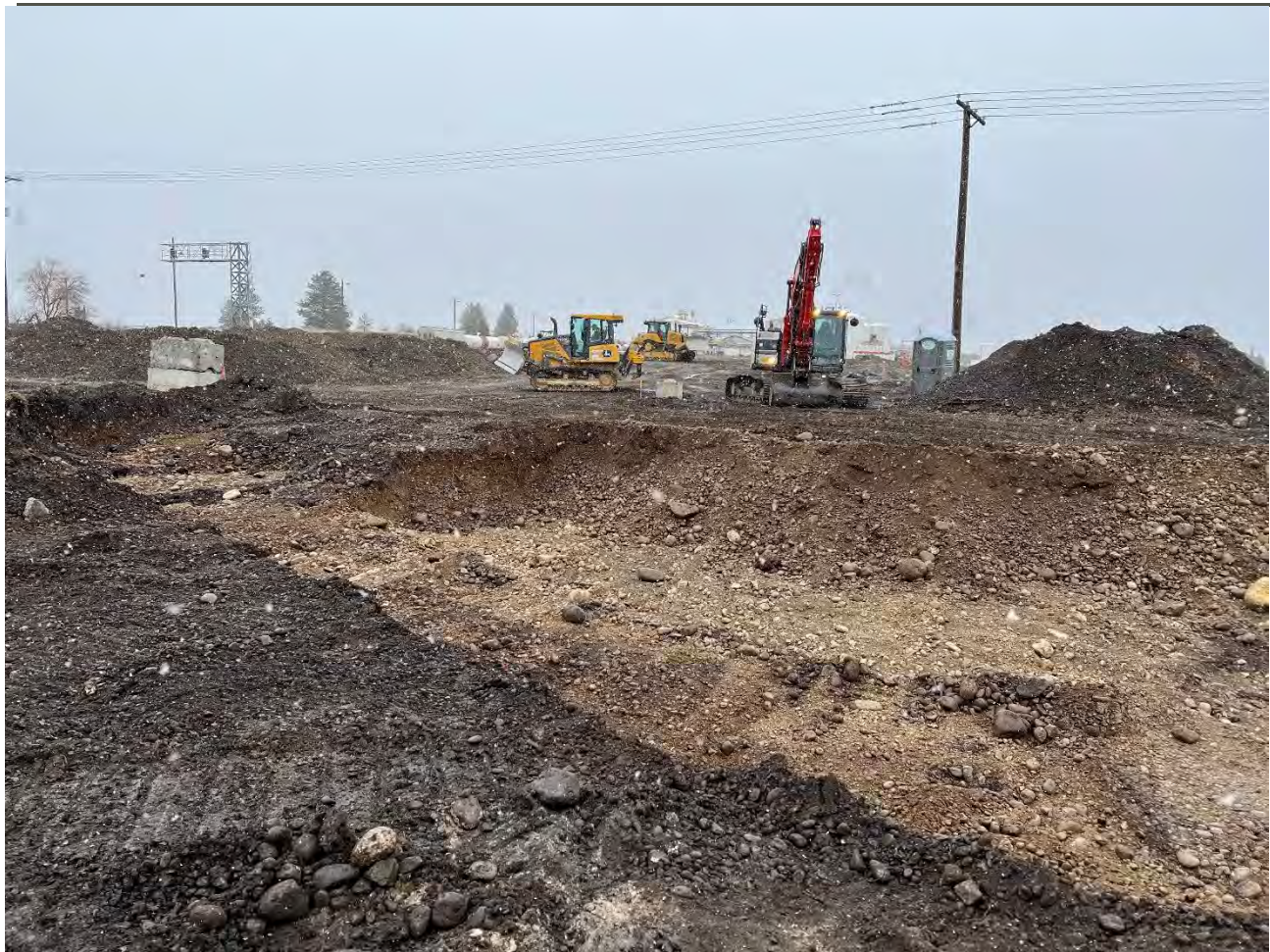
Photograph 2: Excavation 2 excavated down to 2ft, 4ft, and 6ft depths.
