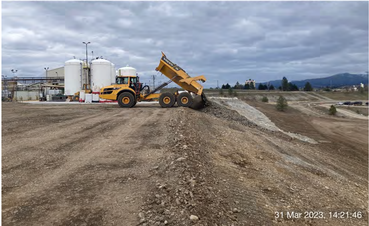
Photograph 5: Off-road haul truck dumping rip-rap material removed from the trackout pad onto the UPRR slope.
