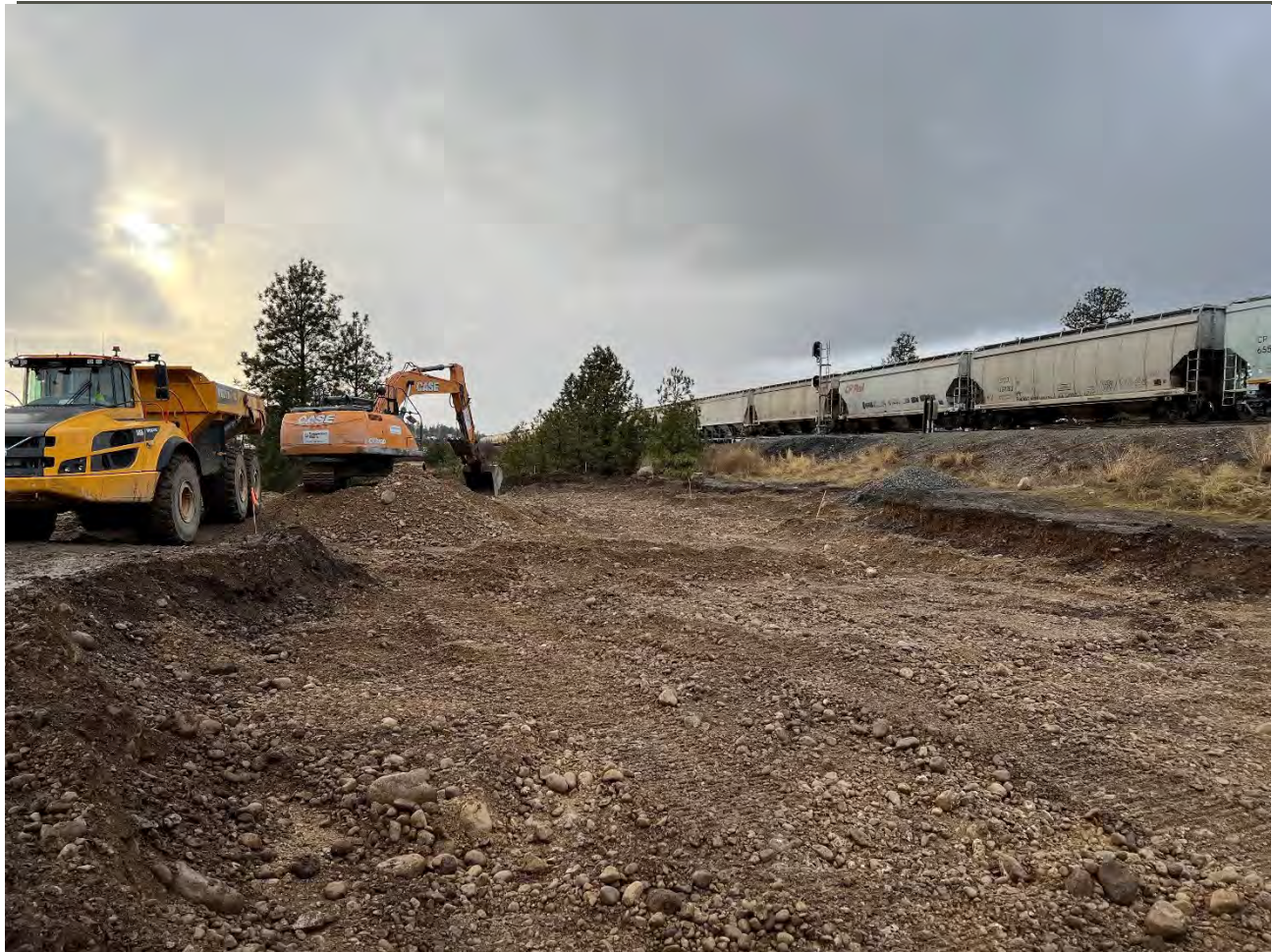
Photograph 8: Excavation 1 on Pentzer property being excavated to 4ft depth.
