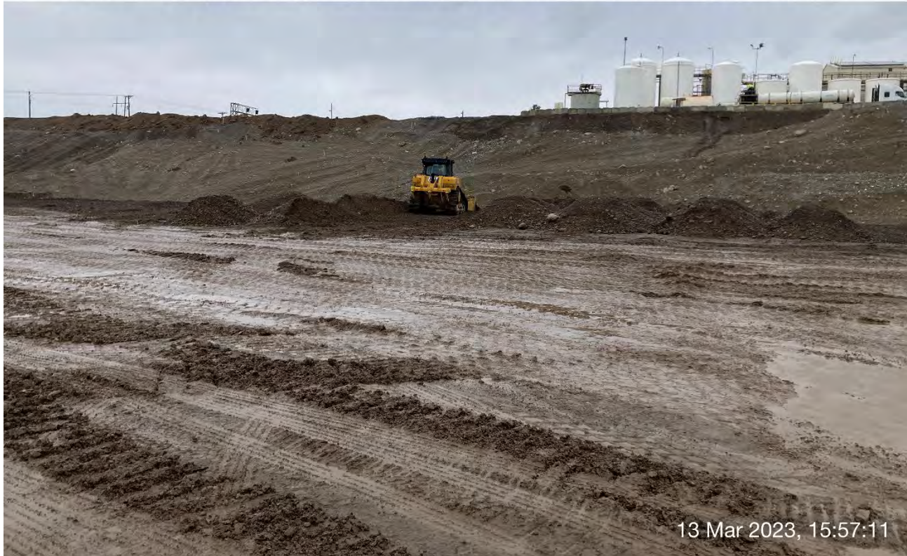
Photograph 4: CAT Dozer used to spread backfill materials on the WSDOT property.
