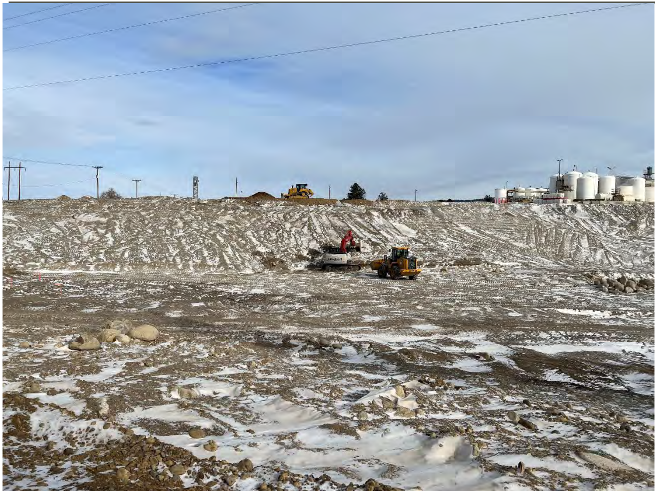
Photograph 3: GrayMar placing and spreading boulders in excavation 6.
