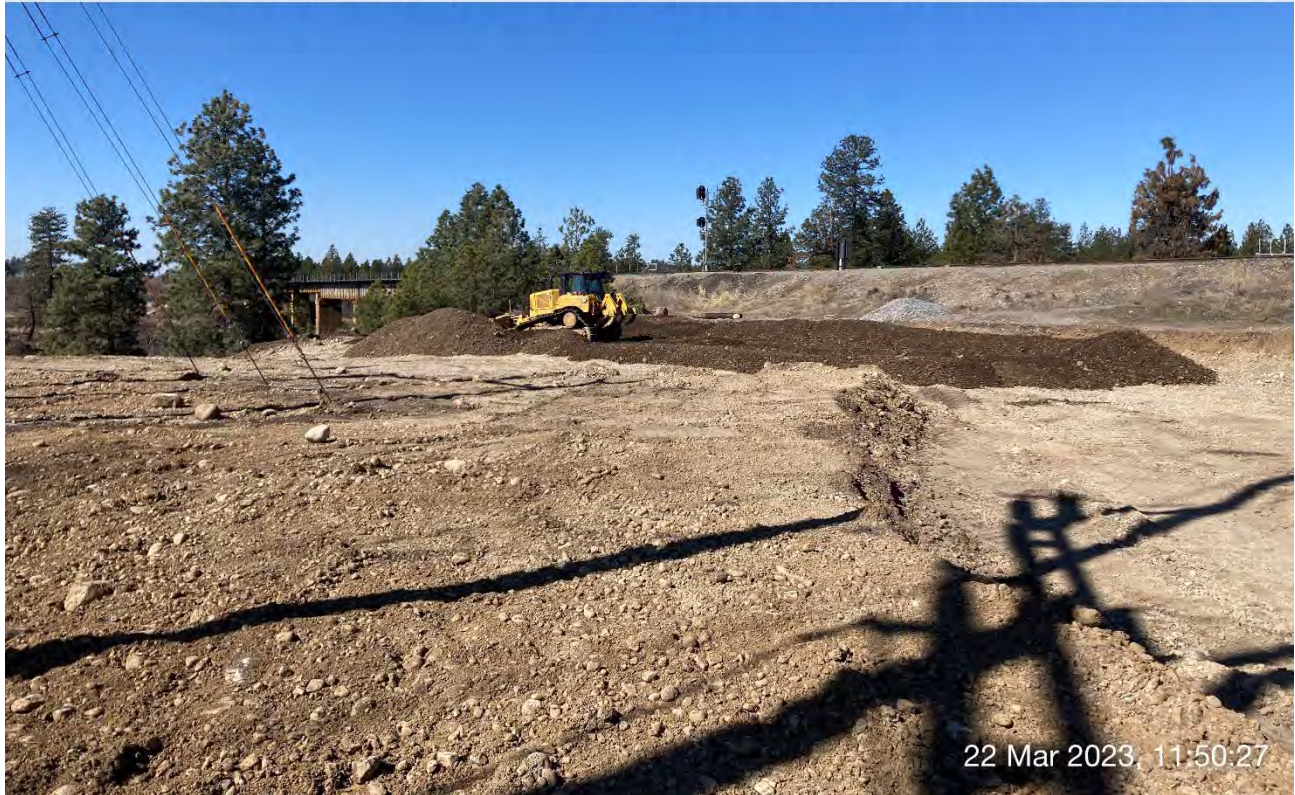
Photograph 4: CAT D6 dozer spreading and grading backfill dumped in Excavation 1 on the Pentzer property.
