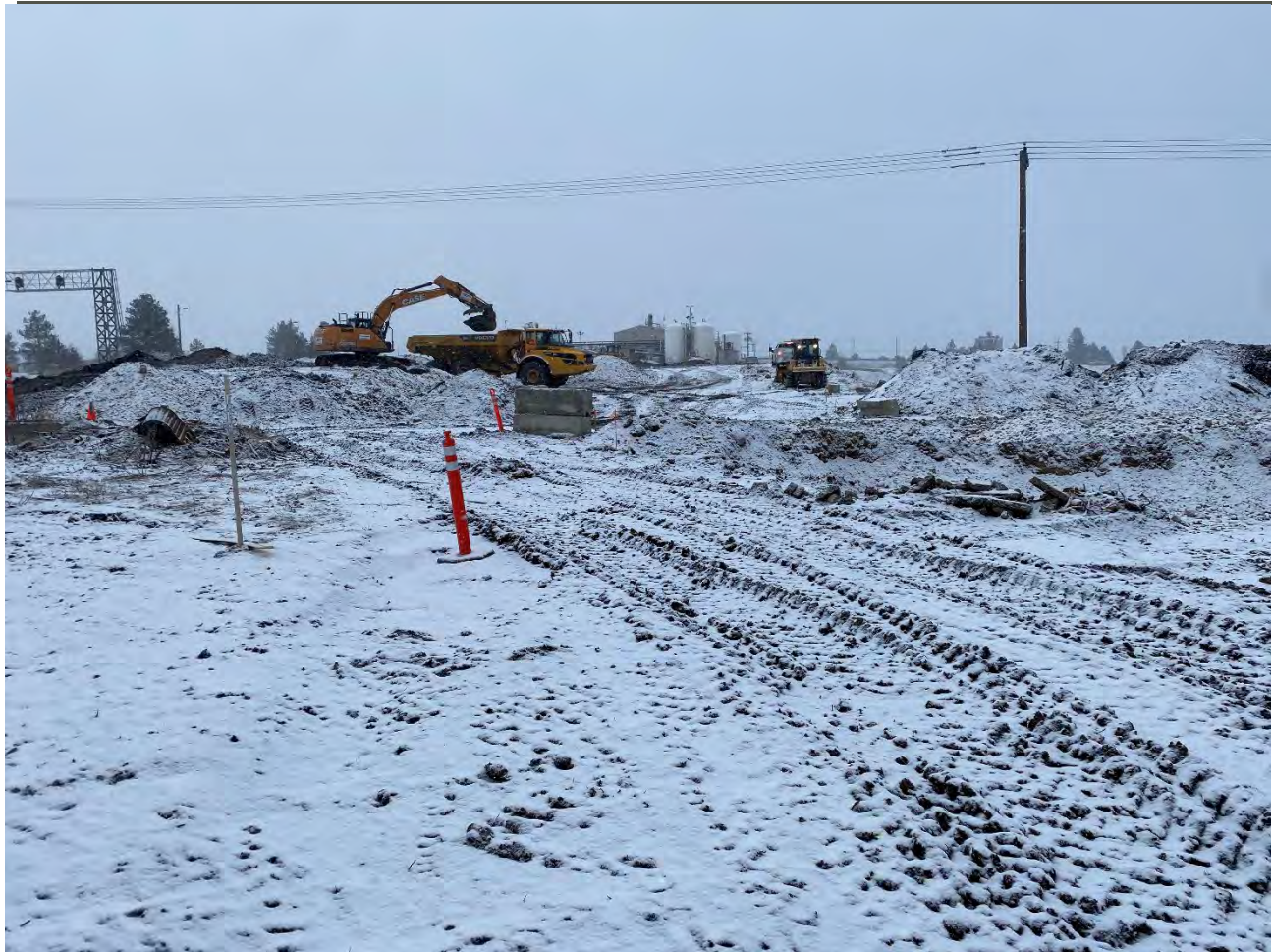
Photograph 2: Building subgrade in upper UPRR cap area.
