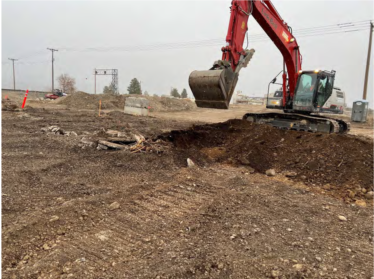
Photograph 1: Interfacing layer of topsoil and subgrade material being excavated out on Pentzer property
