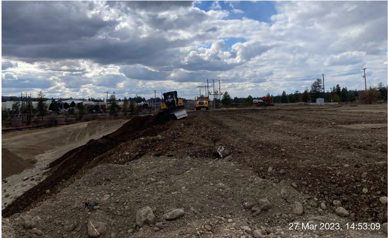
Photograph 3: CAT D6 dozer grading excavated materials dumped on the UPRR slope.
