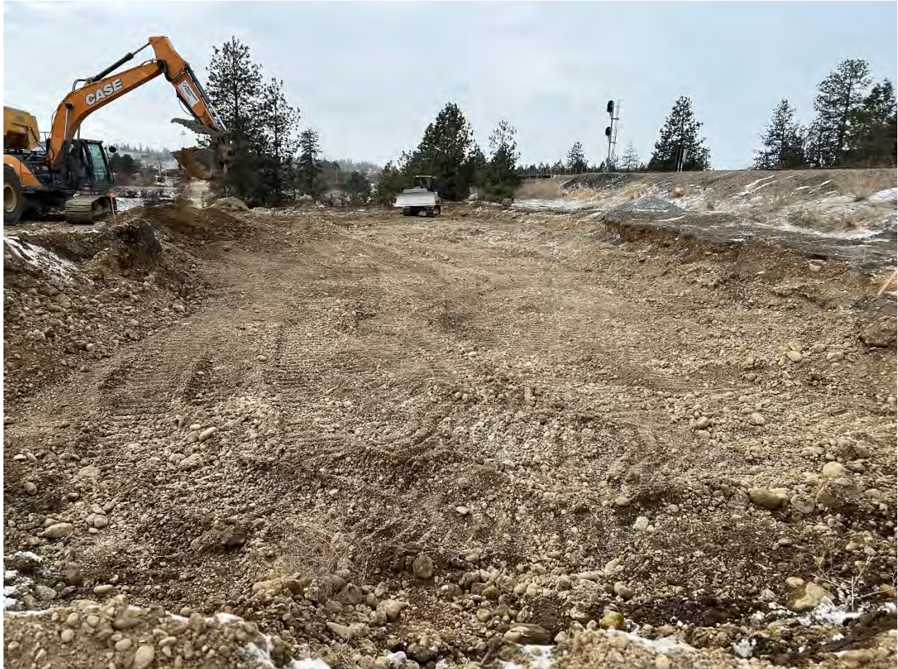
Photograph 1: Excavating and cleaning up of excavation 1.
