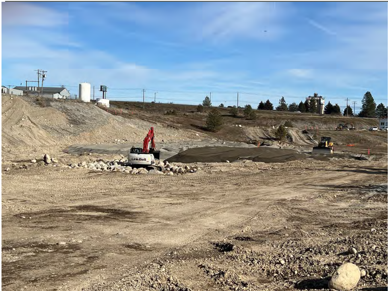
Photograph 3: Placing clean imported backfill in excavation 6. View looking east.
