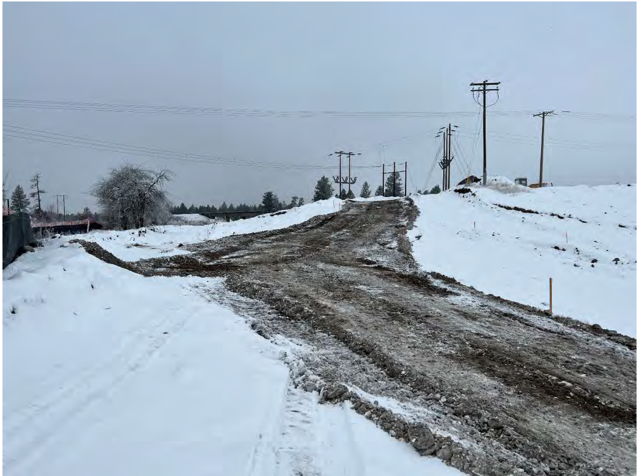
Photograph 1: Cleared access roads from snow and ice for safe travel.
