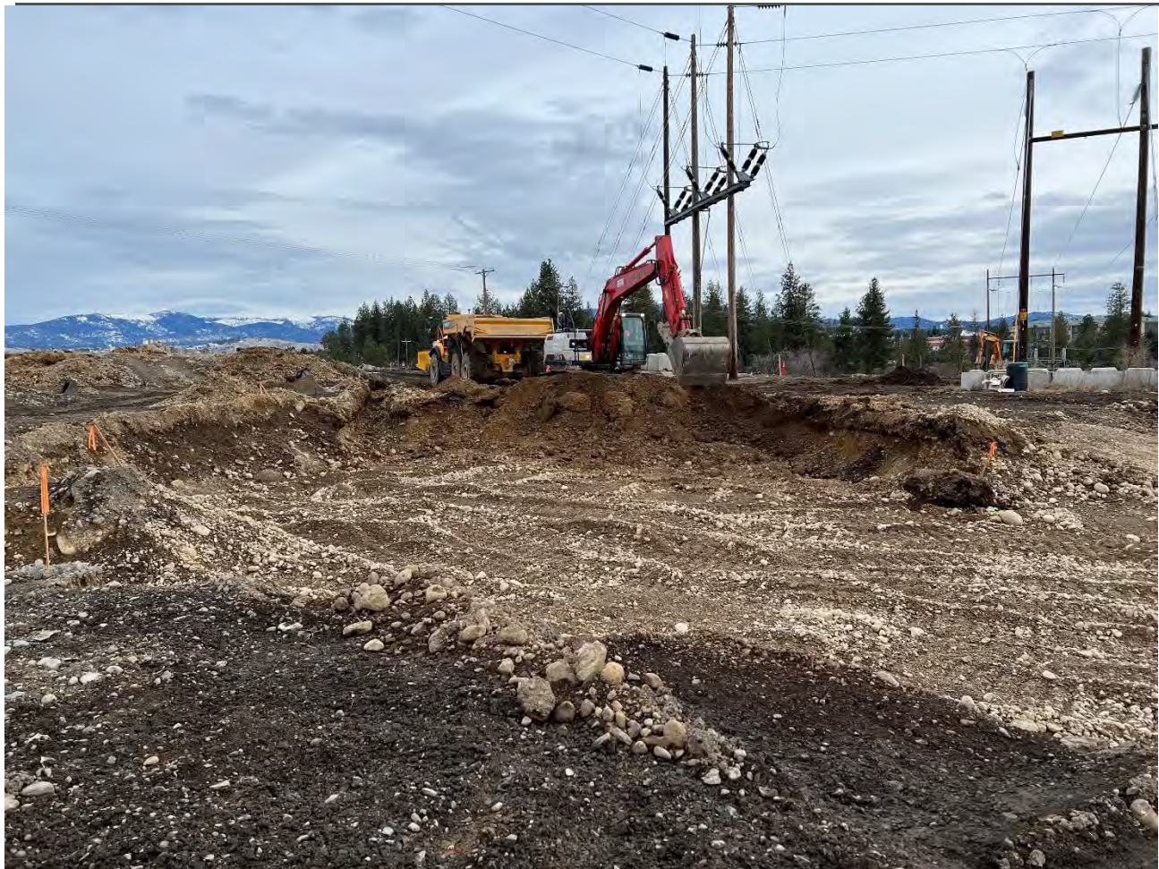
Photograph 2: Excavation 2 on Pentzer property to depth of 4ft.
