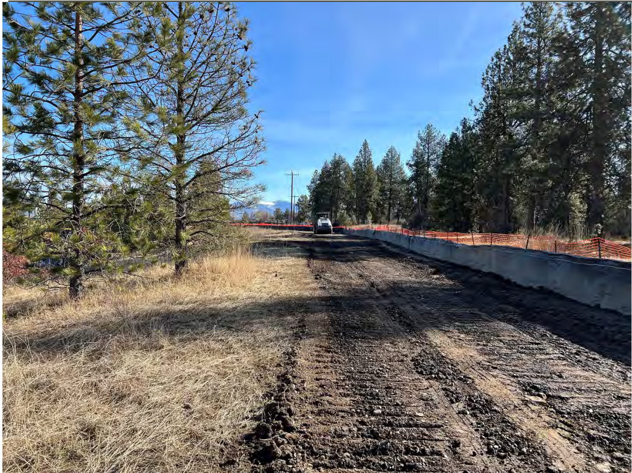
Photograph 2: Cleaning up, placing clean imported backfill, and rolling access road in SE corner of project area. View looking east.
