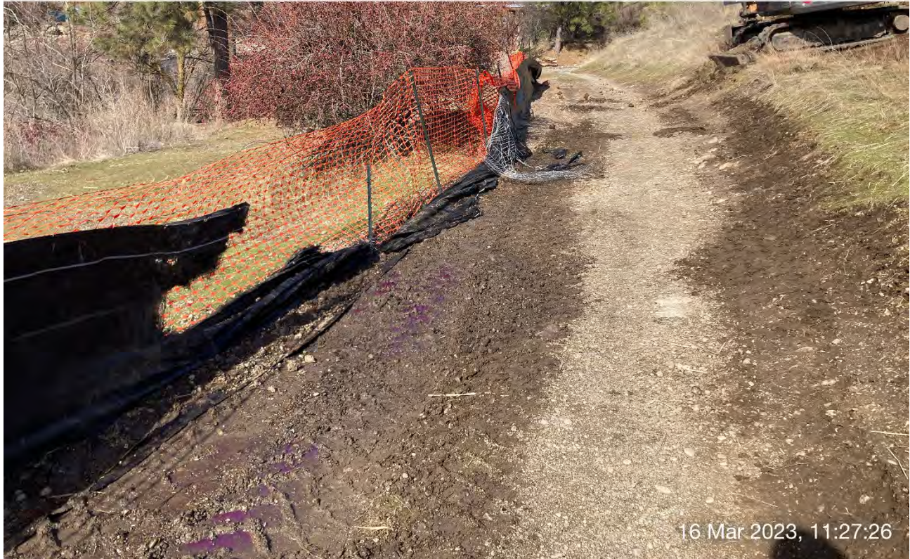
Photograph 5: Diesel fuel spilled by in incorrectly installed fuel cap on the front-end loader on the railroad access road west of the site.
