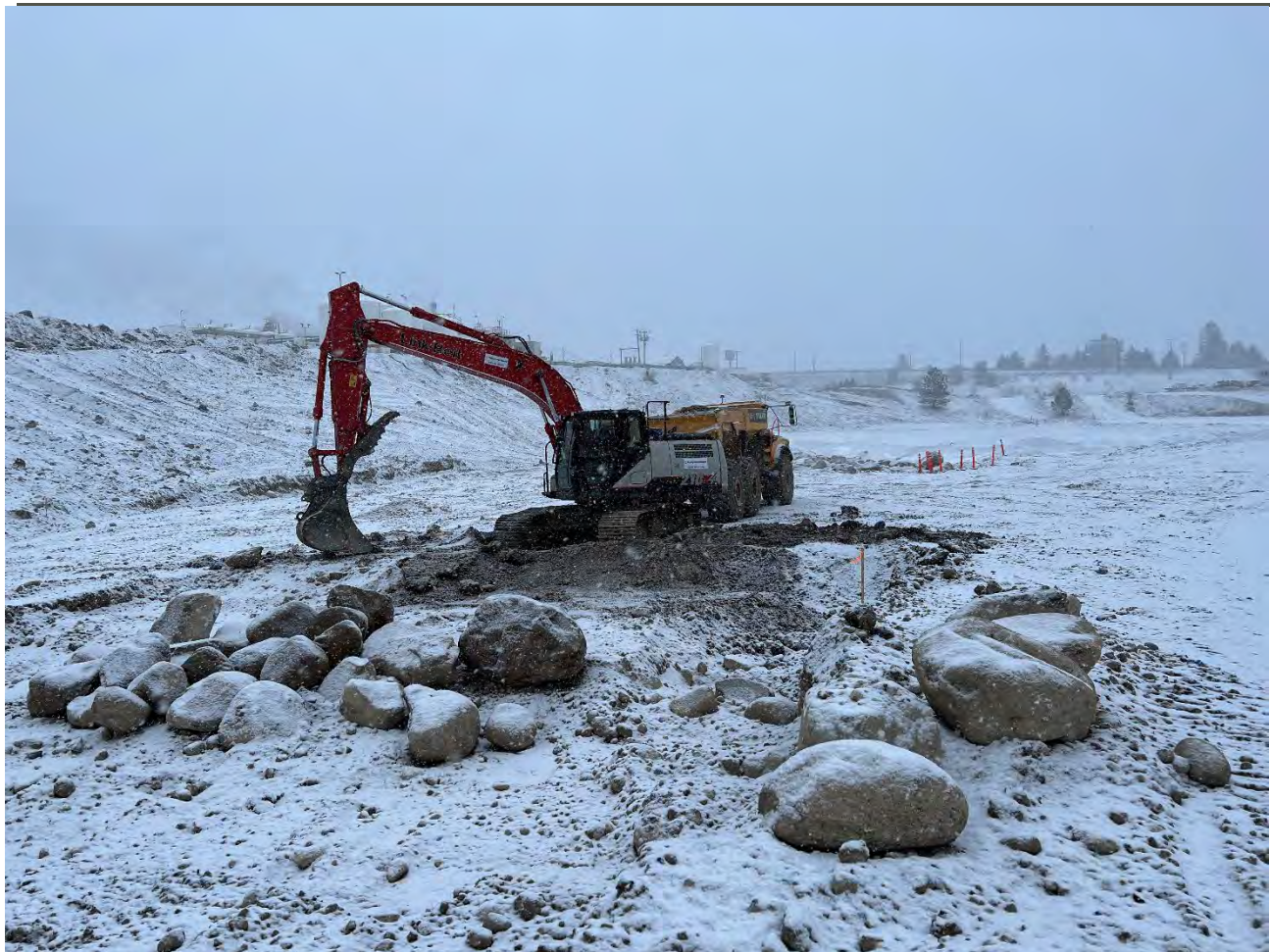
Photograph 2: Removal of additional dross observed on the east wall of excavation 4.
