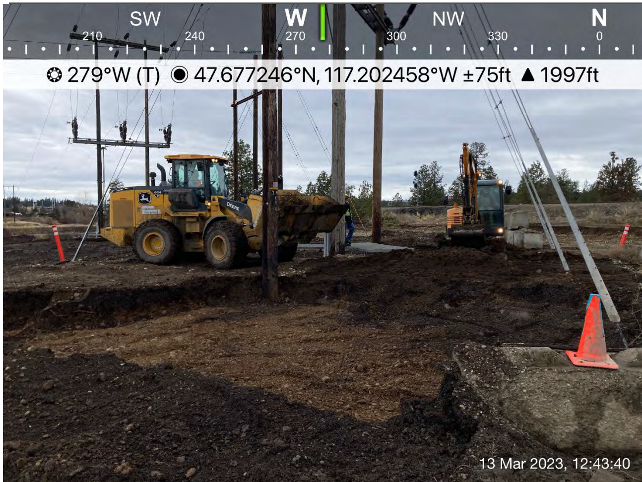
Photograph 3: Excavation around BPA infrastructure on the Pentzer property to a depth of 2-ft.
