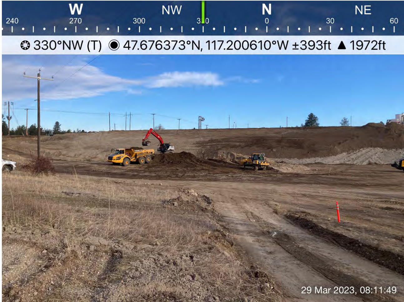
Photograph 1: Front-end loader transferring excavated materials from the stockpile located on the Pentzer property to the UPRR cap area.
