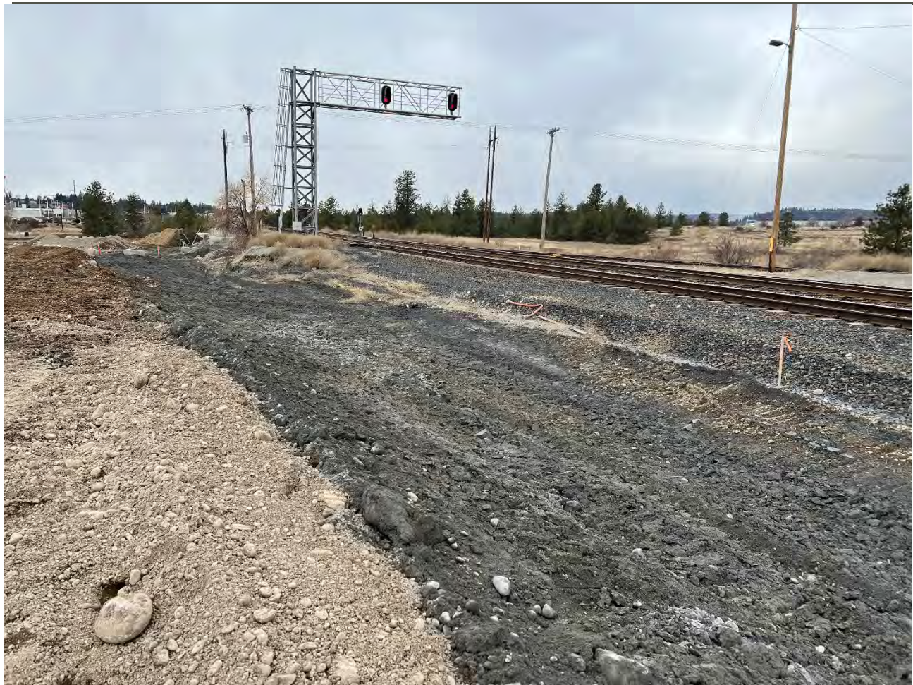
Photograph 5: Railroad ditch subgrade being prepped and graded to drain to west.
