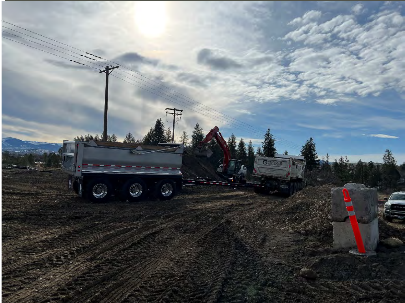
Photograph 2: GrayMar hauling topsoil, vegetation, and excess cross stockpile offsite.
