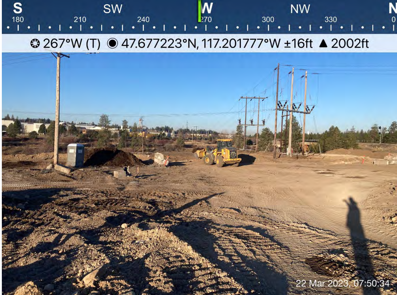
Photograph 1: Front-end loader transferring vegetative materials stockpiled near Excavation 2 to an area in the northeast portion of the Pentzer property.
