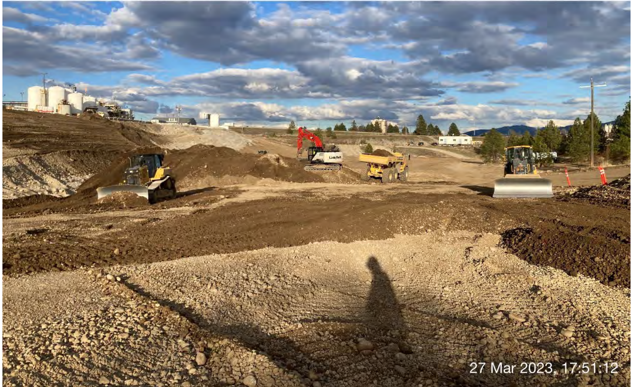
Photograph 4: LinkBelt trackhoe and off-road haul truck transferring stockpiled backfill materials to Excavation 3 and Excavation 4. CAT D6 dozer and John Deere 700L dozer spreading backfill materials in Excavation 4.
