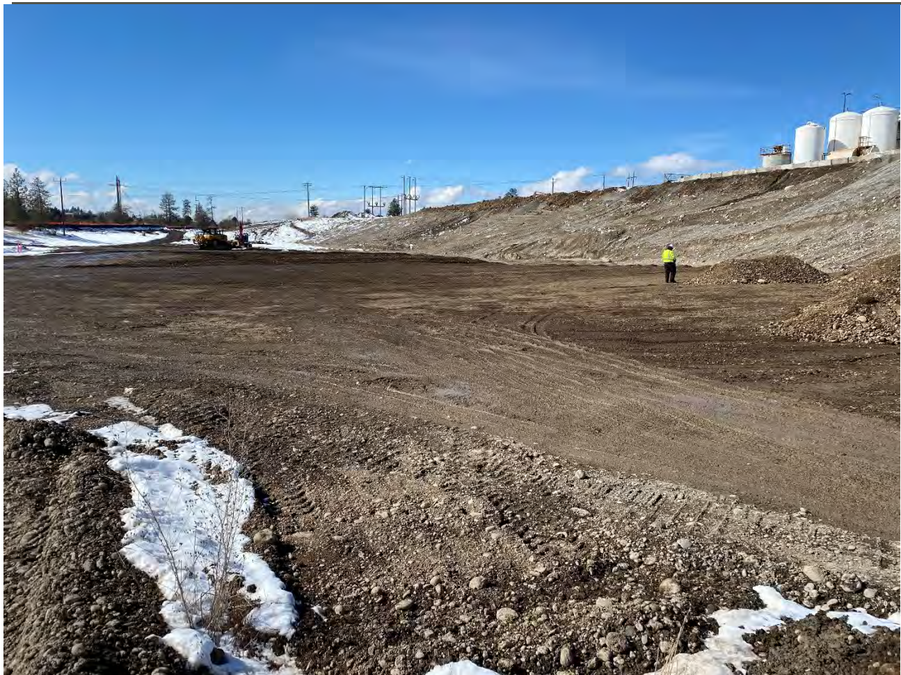
Photograph 3: Compacted backfill on WSDOT property in the afternoon.
