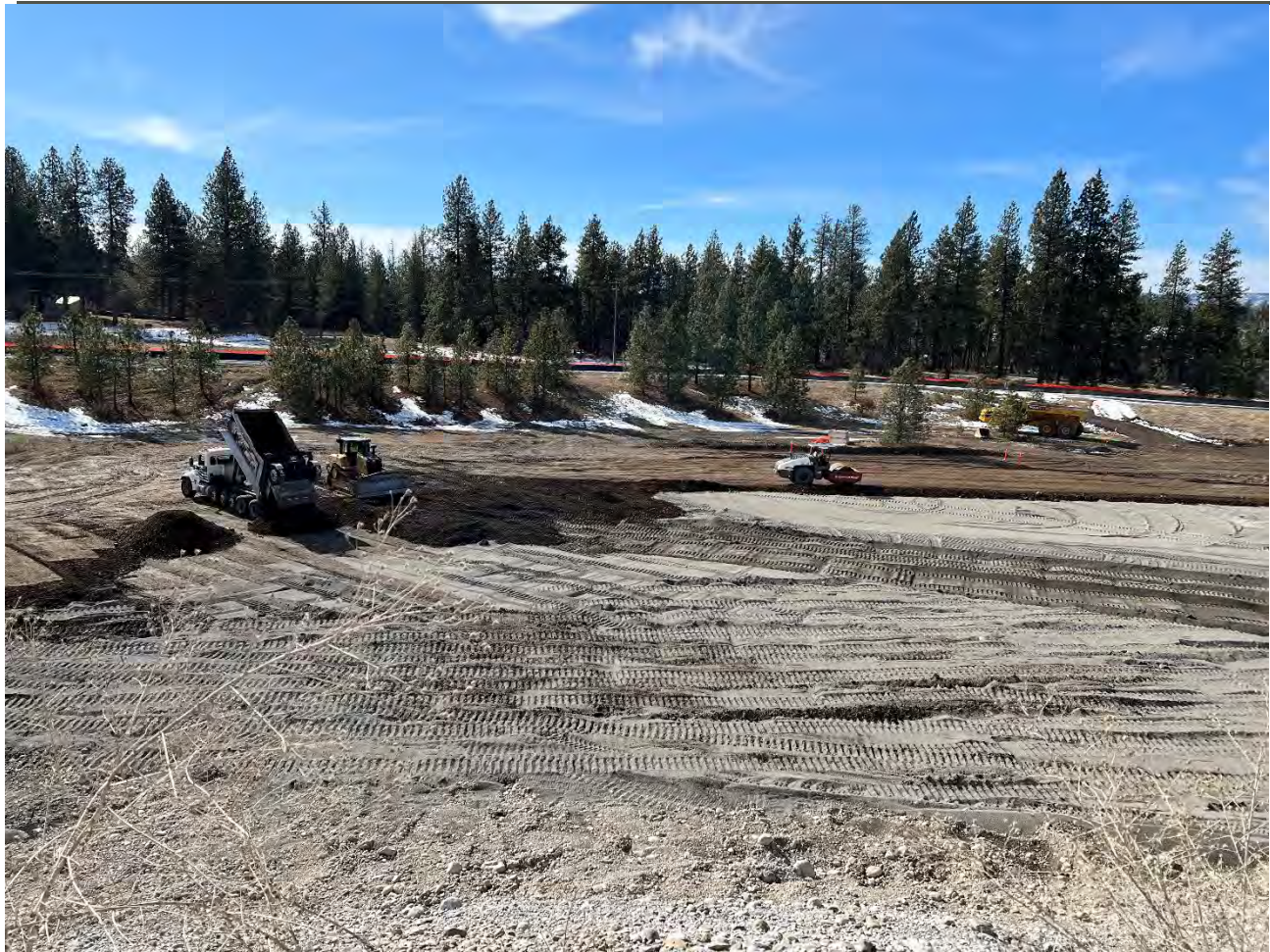
Photograph 3: Placing, spreading, and rolling backfill on WSDOT property.
