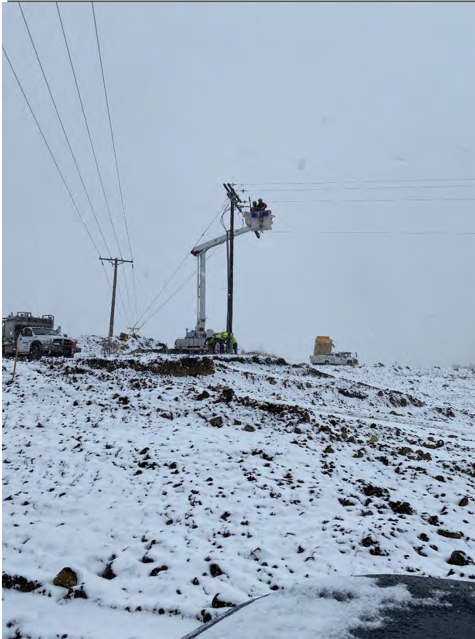
Photograph 3: Avista cutting/removing abandoned lines from utility pole.
