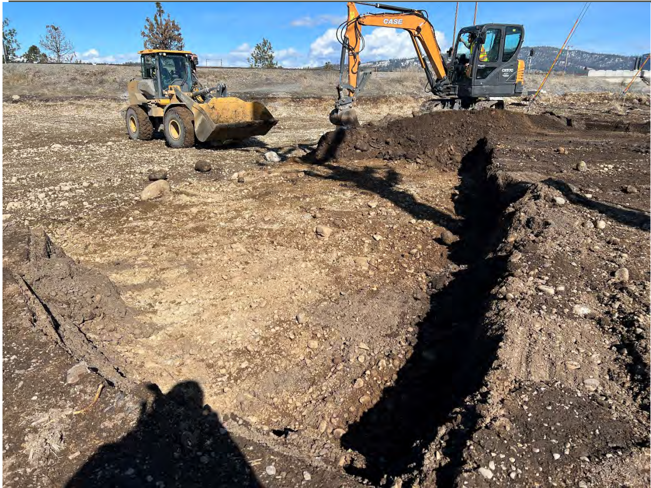
Photograph 3: Excavating around BPA infrastructure to a depth of 2-ft.
