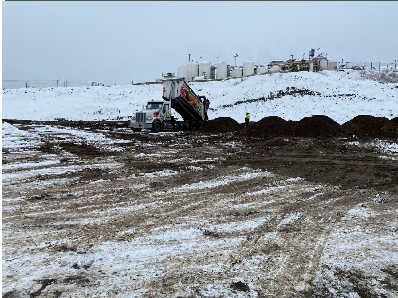
Photograph 2: Importing #5 backfill onto WSDOT Property in the morning
