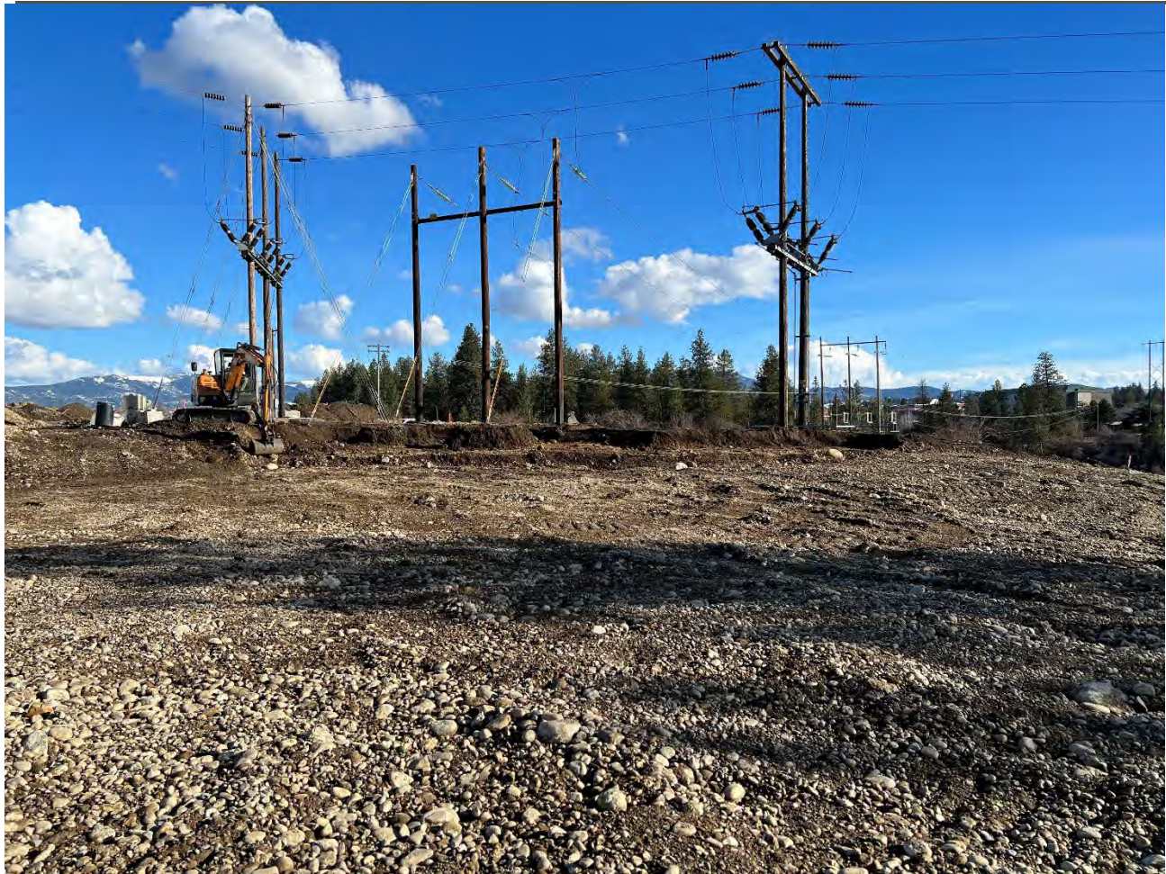
Photograph 4: Excavating around BPA infrastructure to a depth of 2-ft.
