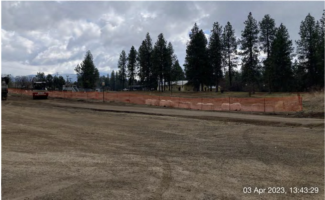
Photograph 3: LinkBelt trackhoe loading rip-rap material from the track-out pad into the off-road haul truck.
