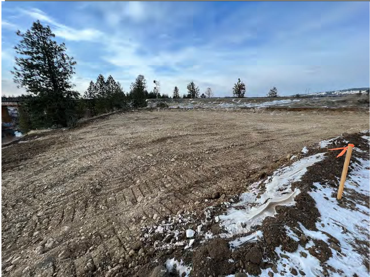
Photograph 2: Excavation 1 ready for sampling after being excavated and cleaned up.
