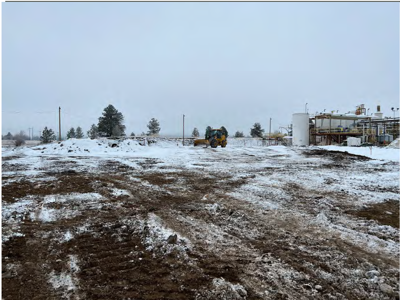
Photograph 2: Clearing ecological cap area of snow and ice.
