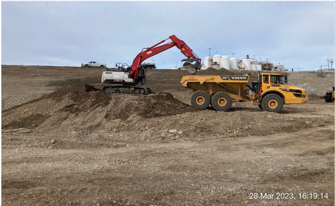
Photograph 5: LinkBelt trackhoe loading backfill materials from the backfill material stockpile located east of Excavation 4 on the WSDOT property into the off-road haul truck for transport.
