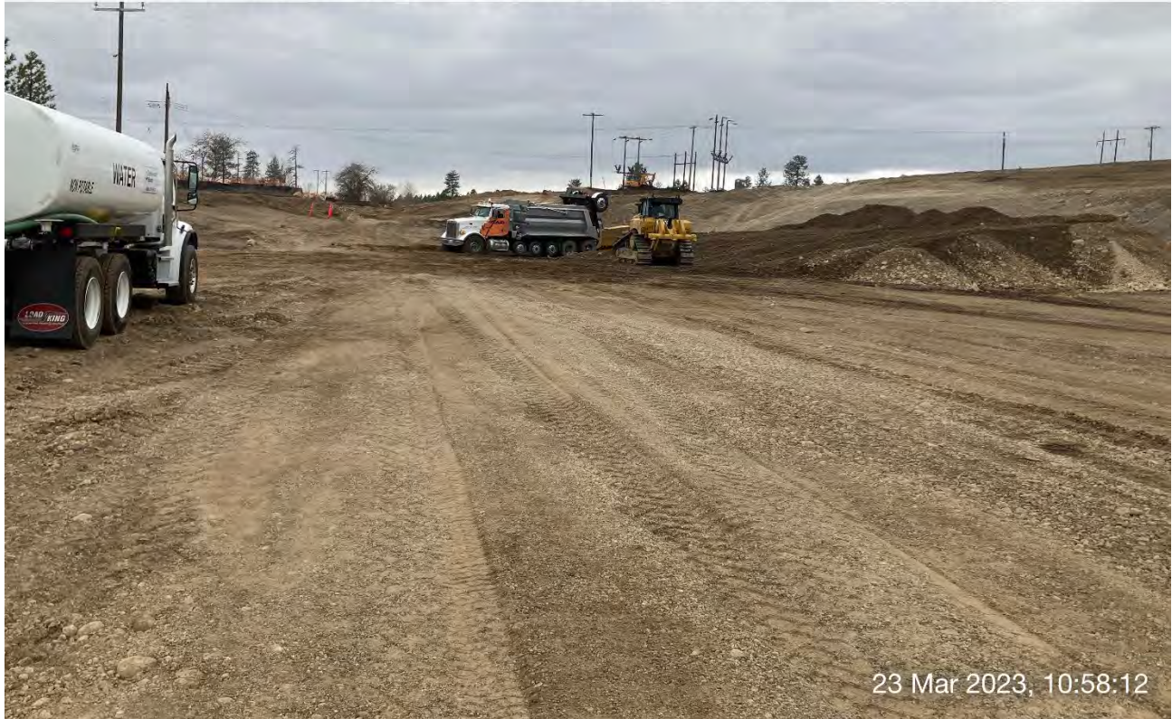
Photograph 2: CAT D6 dozer uses to push backfill material delivered to site.
