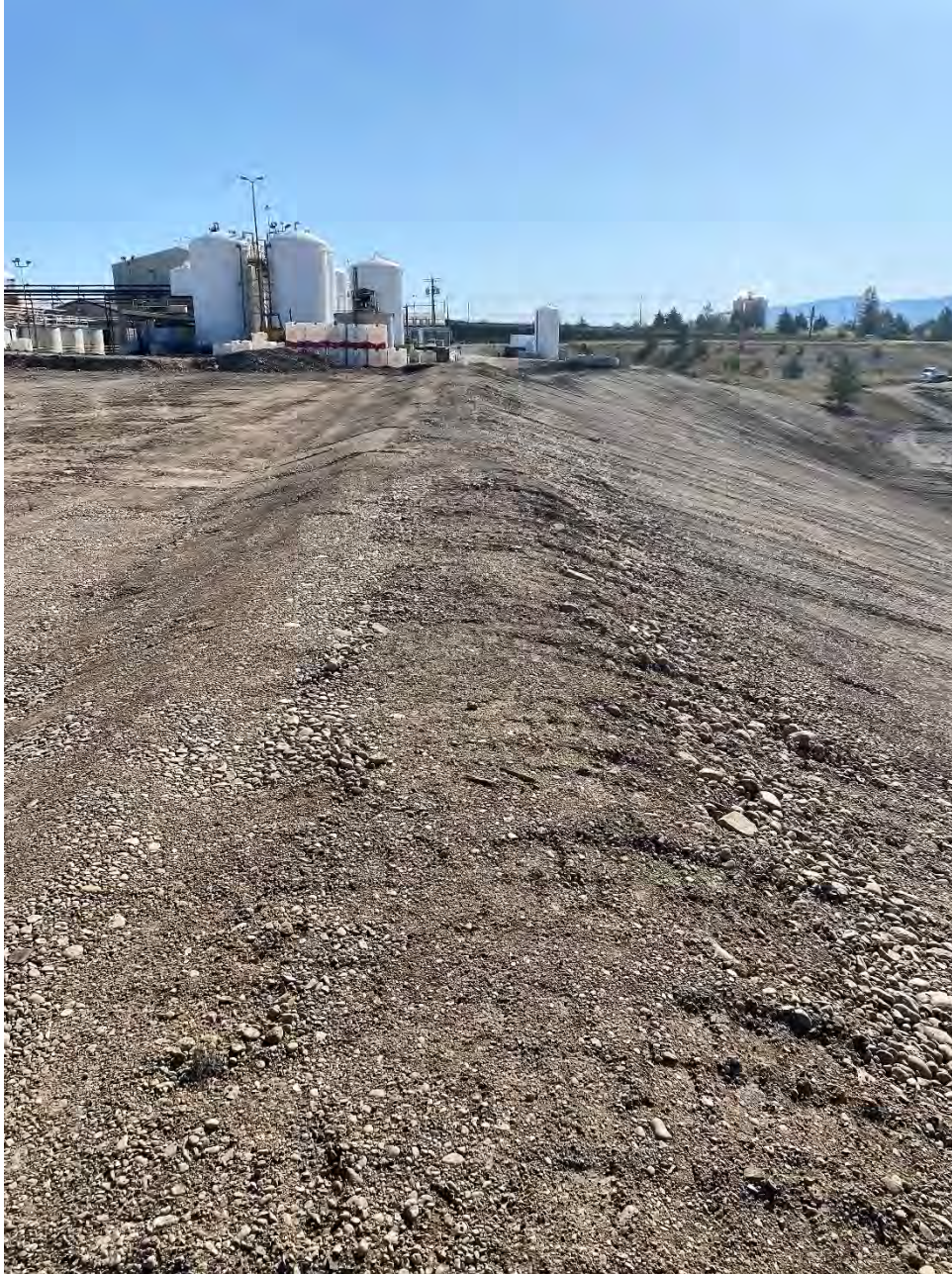
Photograph 1: Completed subgrade for UPRR pad containment south berm looking east .
