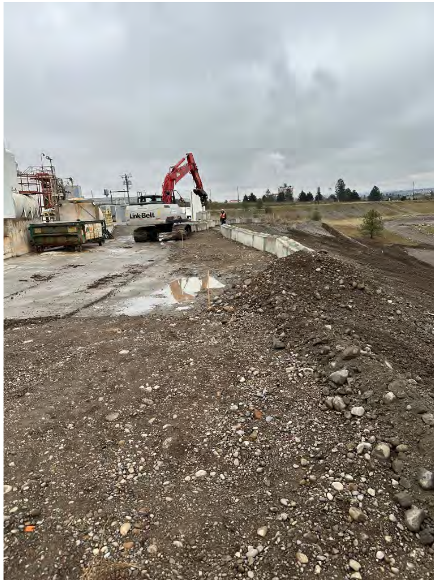
Photograph 1: Moving cement blocks further north on UPRR property
