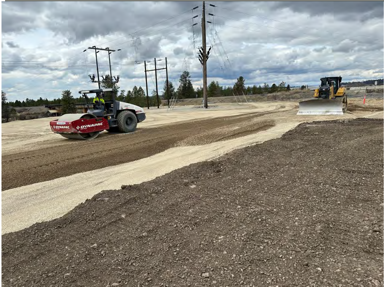
Photograph 3: Completing backfill for Excavation 1, and Excavation 2
