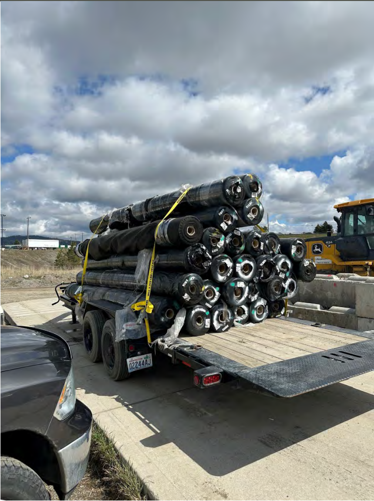
Photograph 5: Geotextile brought on Site for construction of ecological cap
