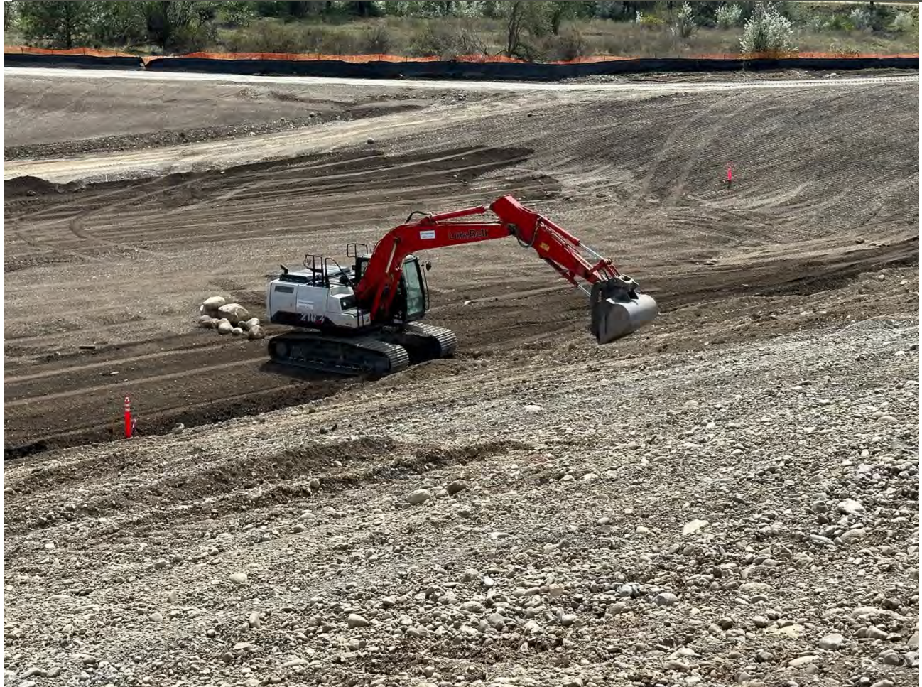
Photograph 4: Removal of large boulders on UPRR sloped section
