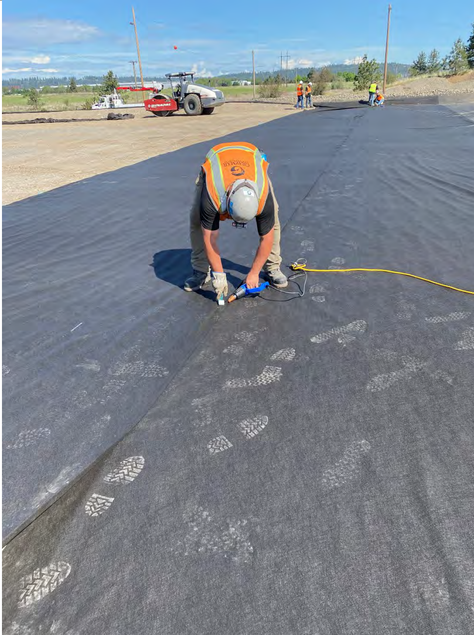
Photograph 4: Welding seam on fabric UPRR pad.
