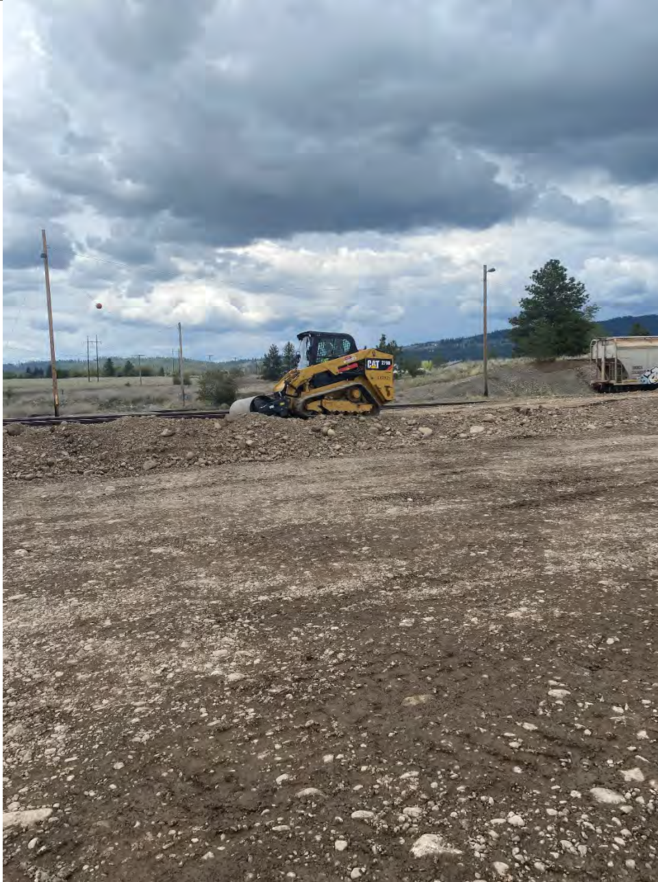
Photograph 3: Compacting containment berm on north side of UPRR pad.
