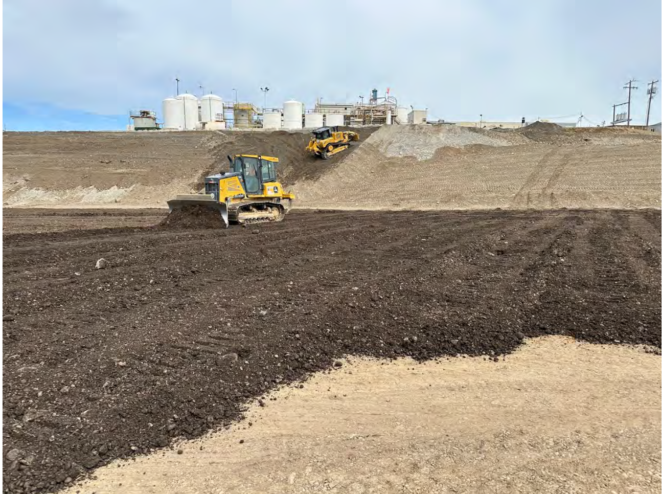
Photograph 2: Spreading 6-inches of topsoil on WSDOT property
