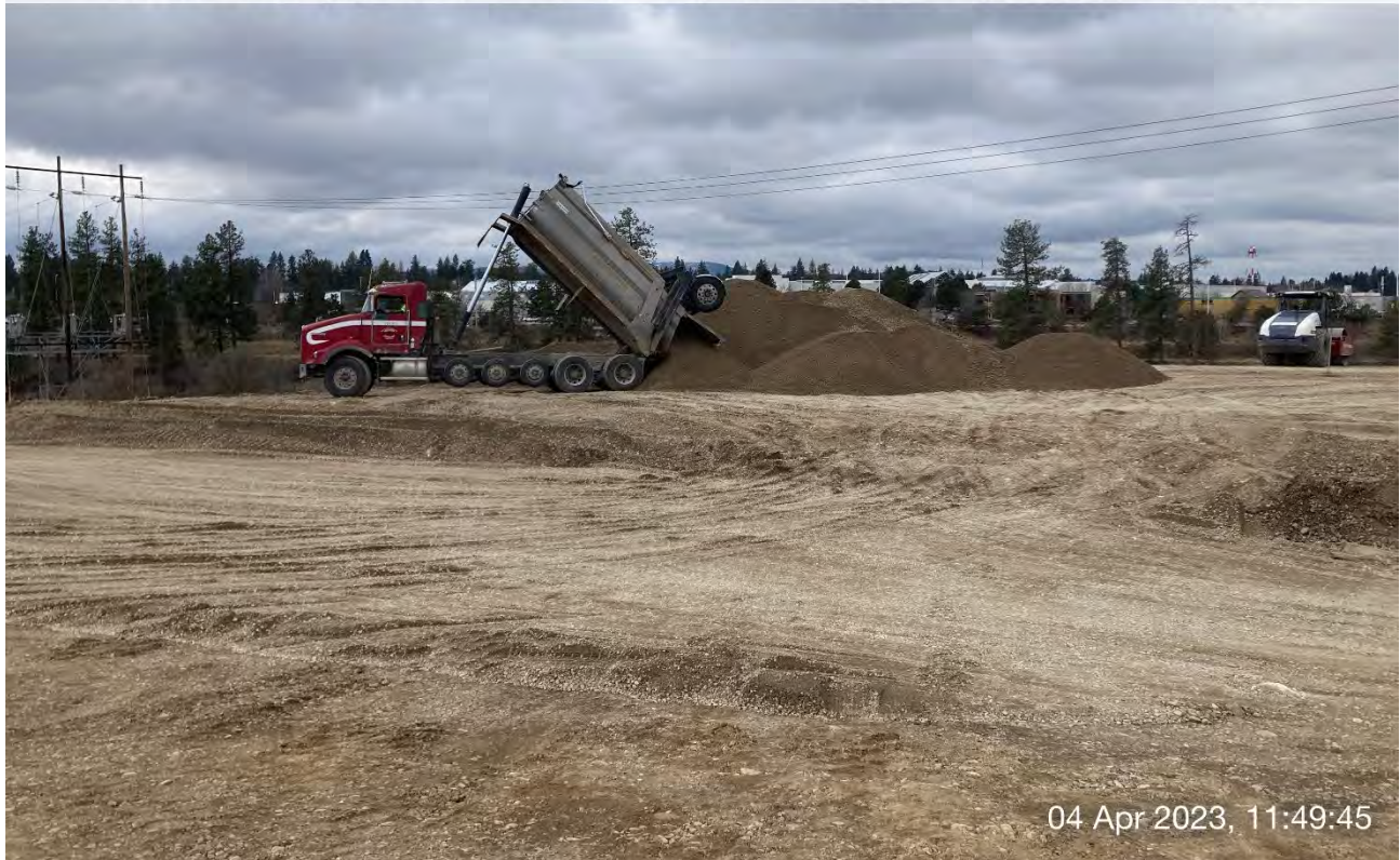
Photograph 3: Interstate Trucking highway dump truck dumping load of backfill material on the Pentzer property, near the southwestern portion of Excavation 2
