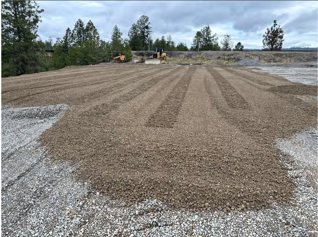
Photograph 2: Backfilling and grading Excavation 1
