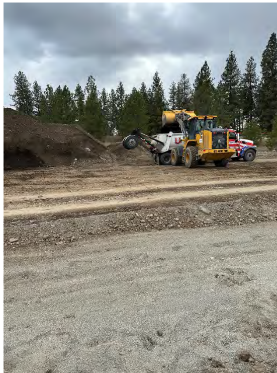
Photograph 3: Moving excess clean fill off site to maintain grading extents
