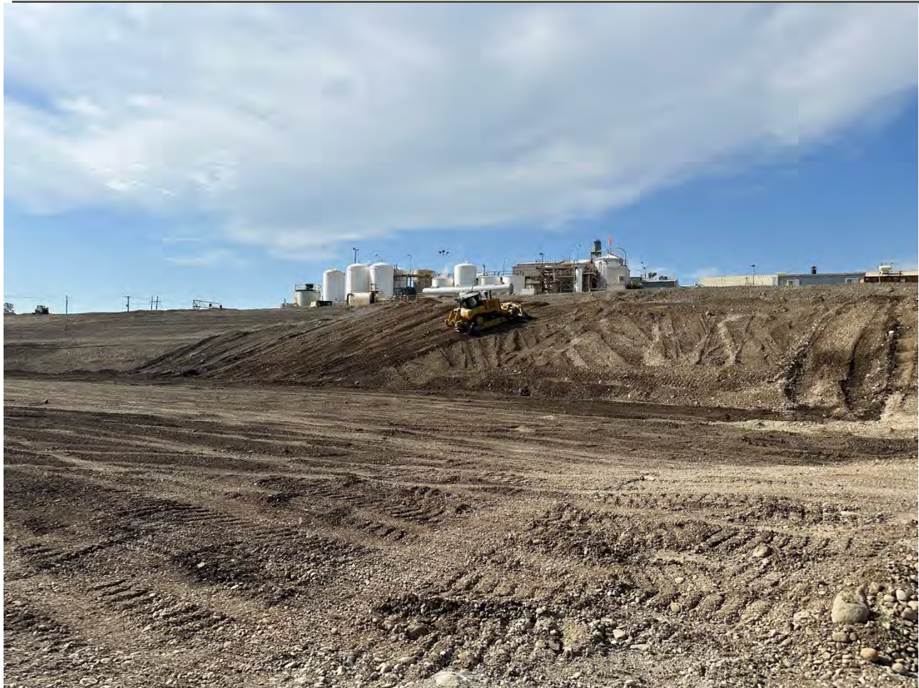
Photograph 2: Grading UPRR sloped section
