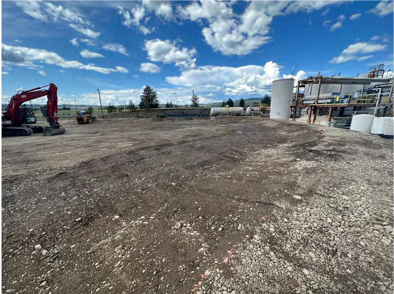
Photograph 1: Compaction/ completion of UPRR containment west berm.
