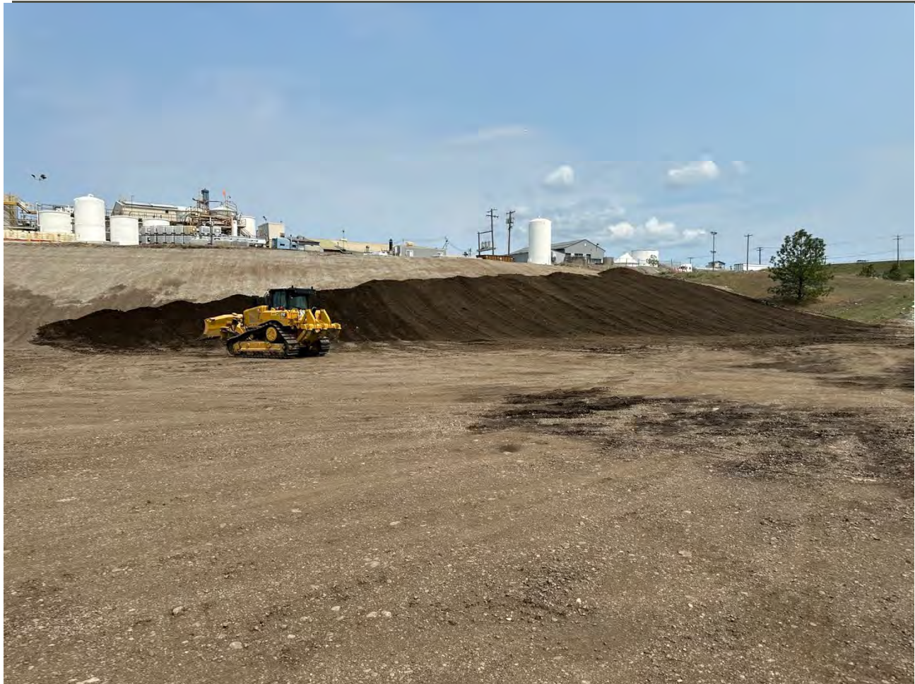
Photograph 3: Placing topsoil on eastern portion of WSDOT side slope.
