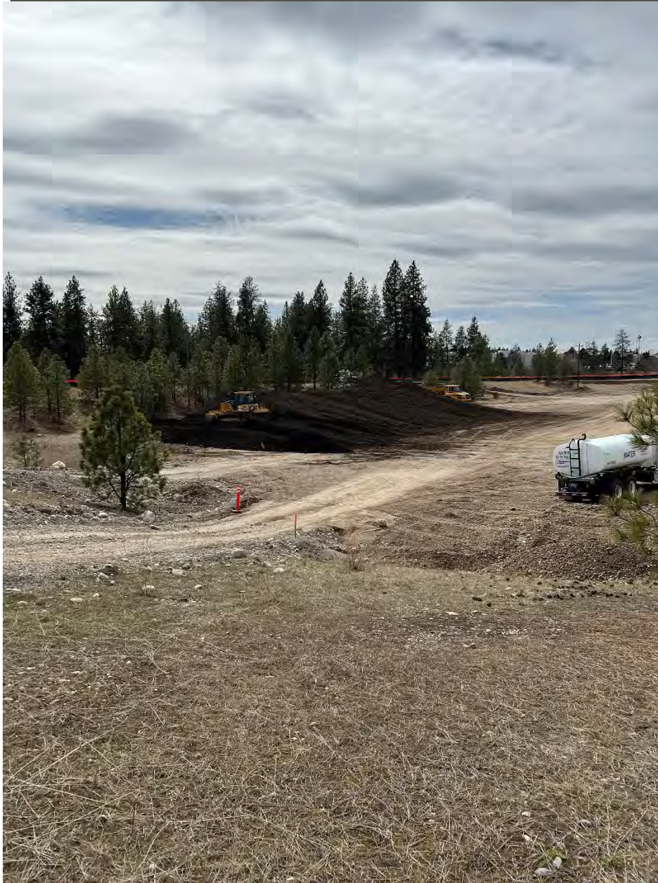
Photograph 3: Topsoil continuing to be received and stockpiled.
