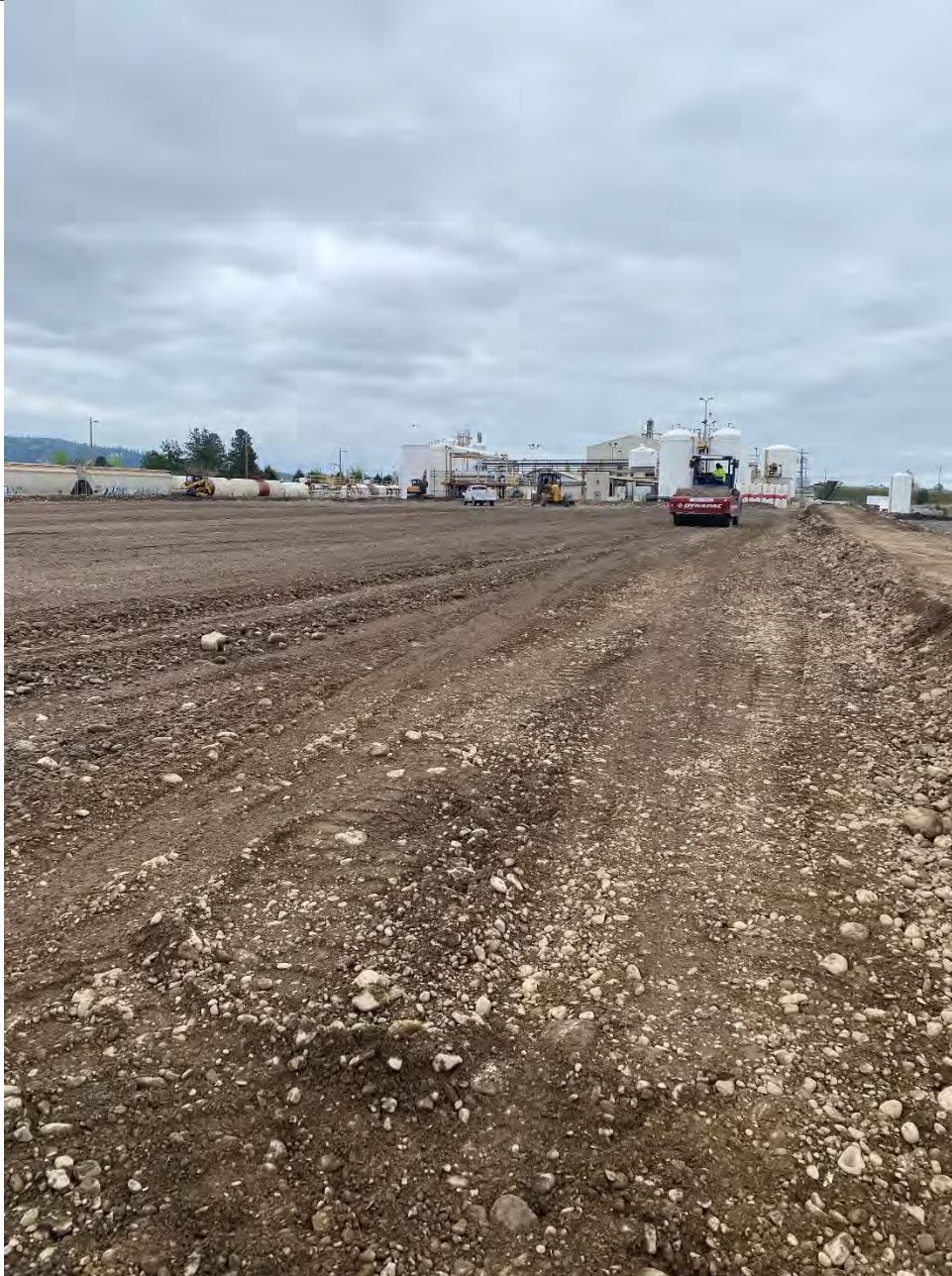
Photograph 2: Compaction of UPRR pad following regrading.
