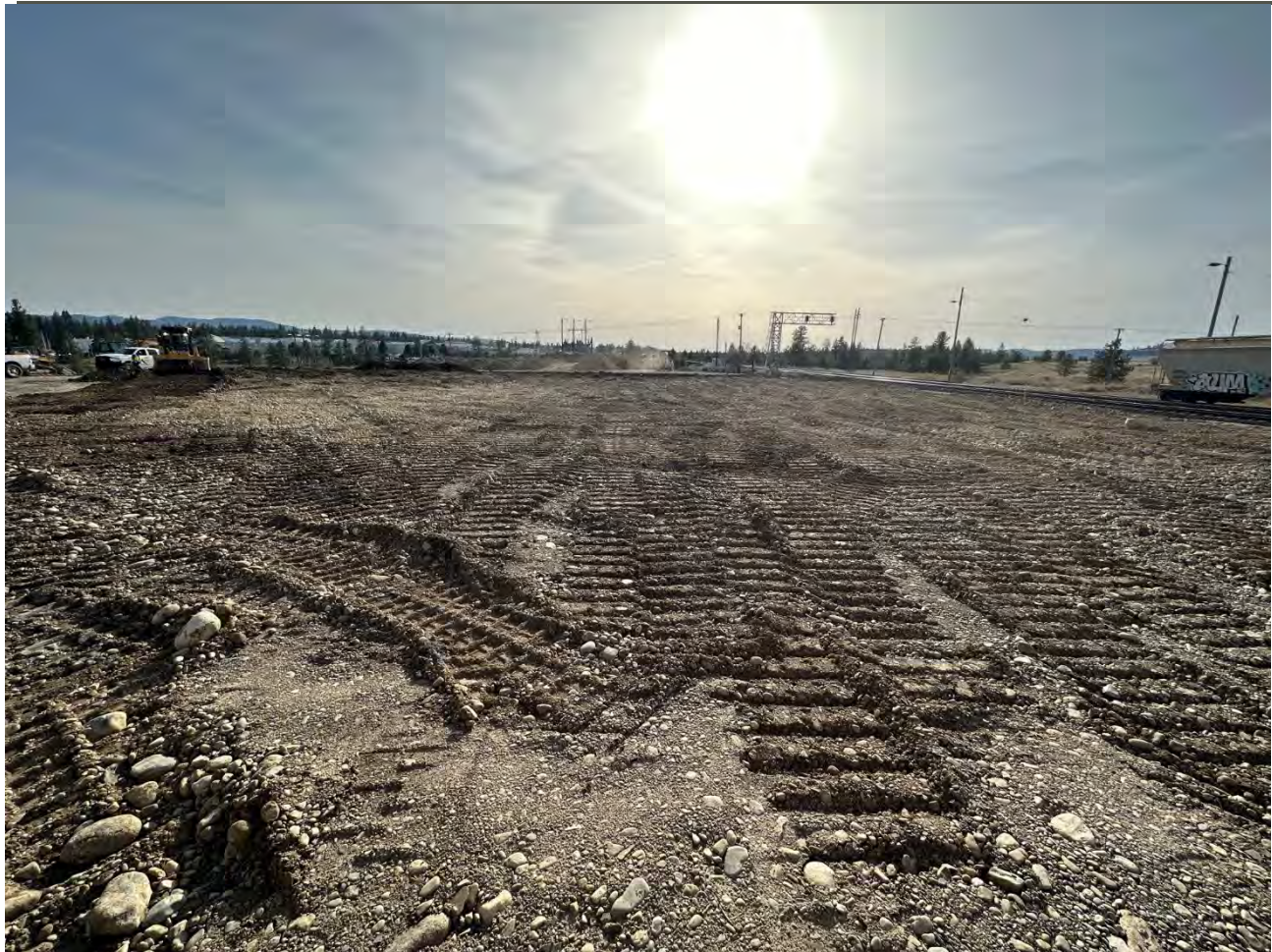
Photograph 5: Placing and grading excavated material from Pentzer property on UPRR pad
