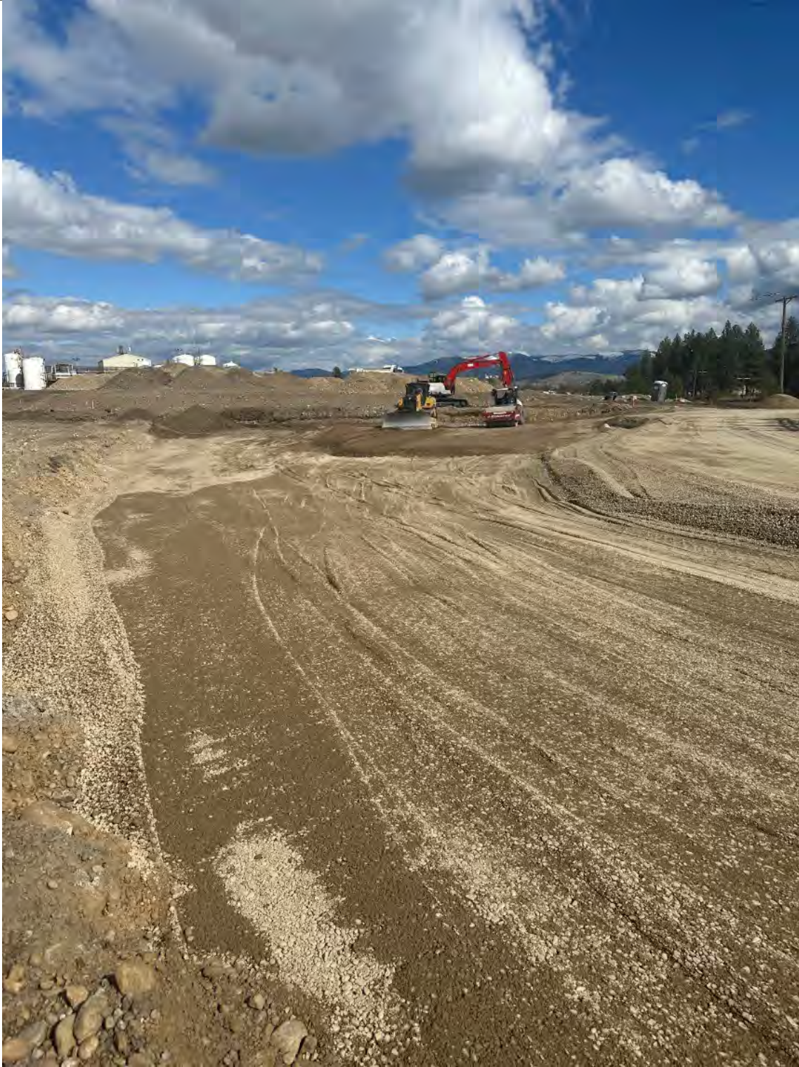
Photograph 2: Backfilling Excavation 1 and Excavation 2 on the Pentzer property
