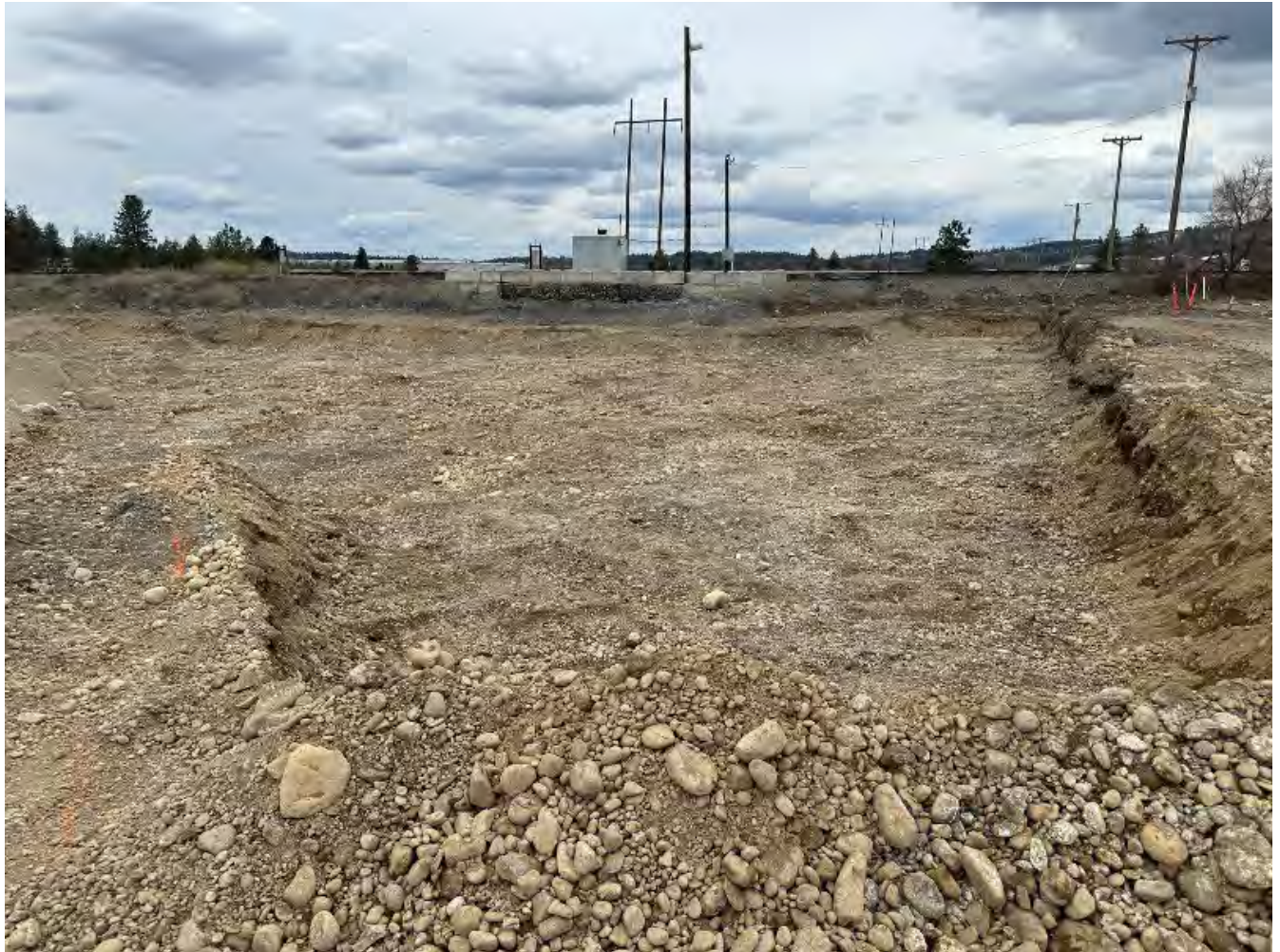
Photograph 2: NE Pentzer property wedge area excavation facing north.
