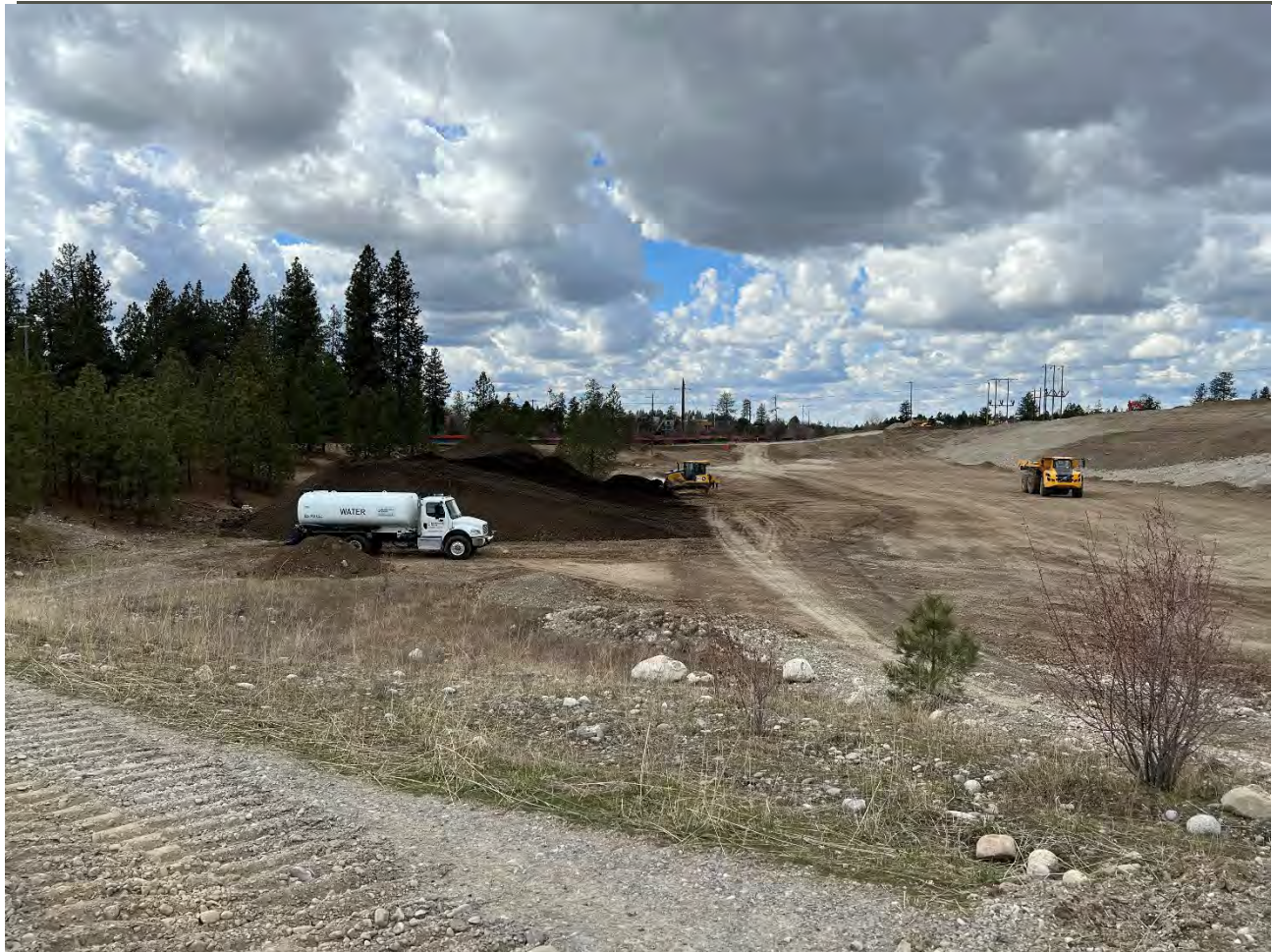
Photograph 2: Receiving and stockpiling of topsoil material on WSDOT.
