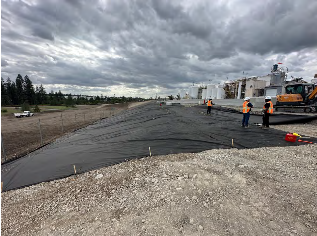
Photograph 1: Filter fabric on eastern portion of UPRR side slope
