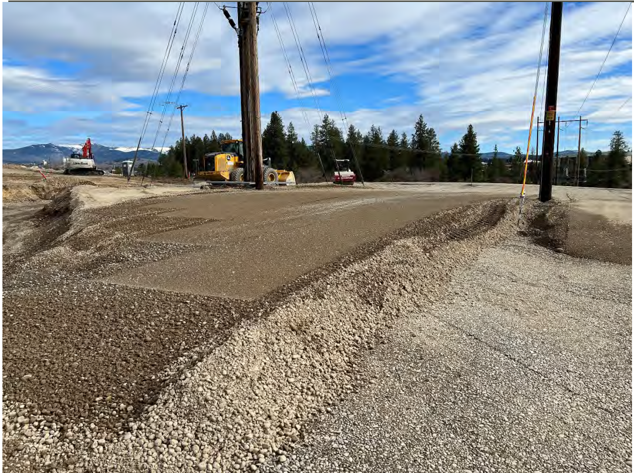
Photograph 2: Pentzer property with backfill being placed and compacted.
