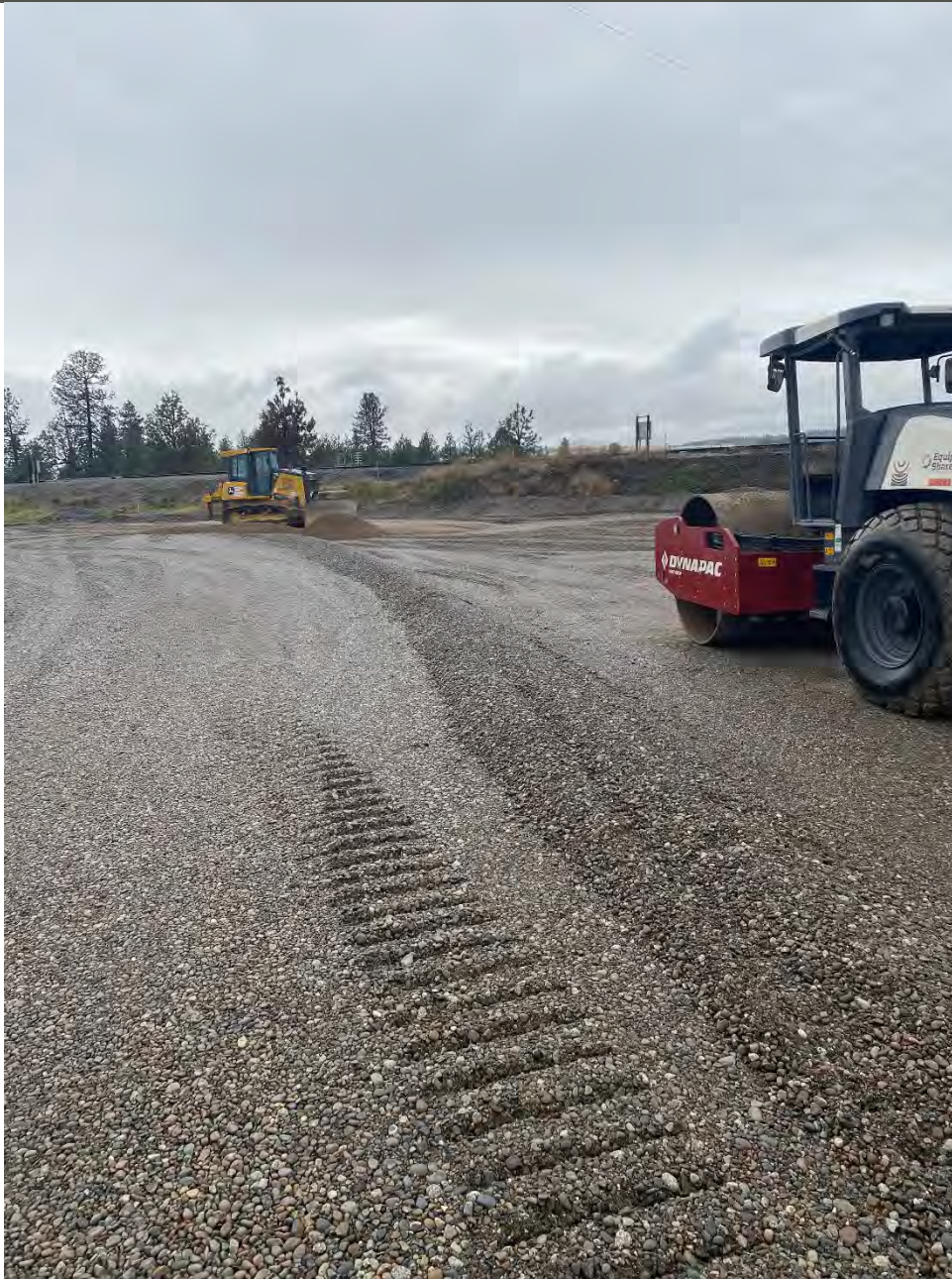
Photograph 3: Backfilling and compacting Pentzer excavation.
