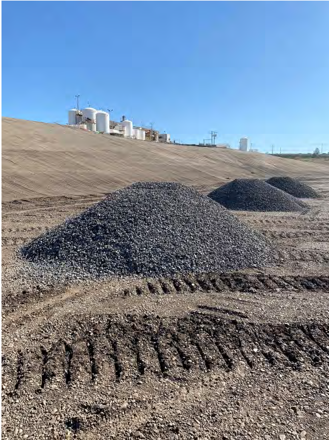
Photograph 2: First three loads of imported ballast for the ecological cap.
