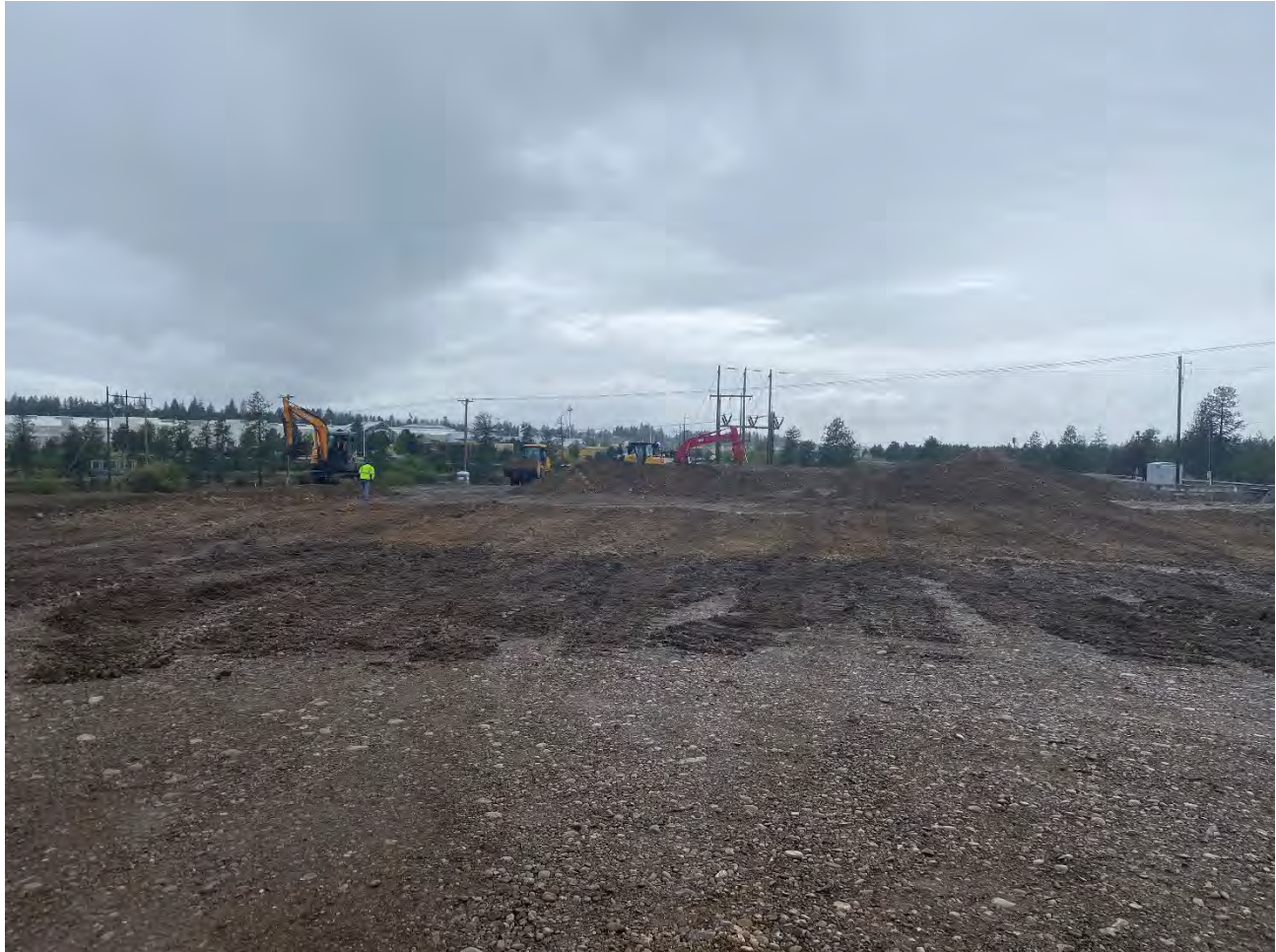
Photograph 1: Placing off property soil from Penzter on UPRR pad and re-grading.
