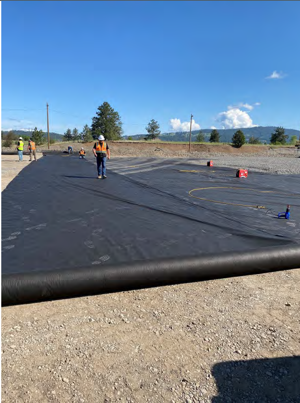
Photograph 5: Placing fabric on eastern third of UPRR pad.
