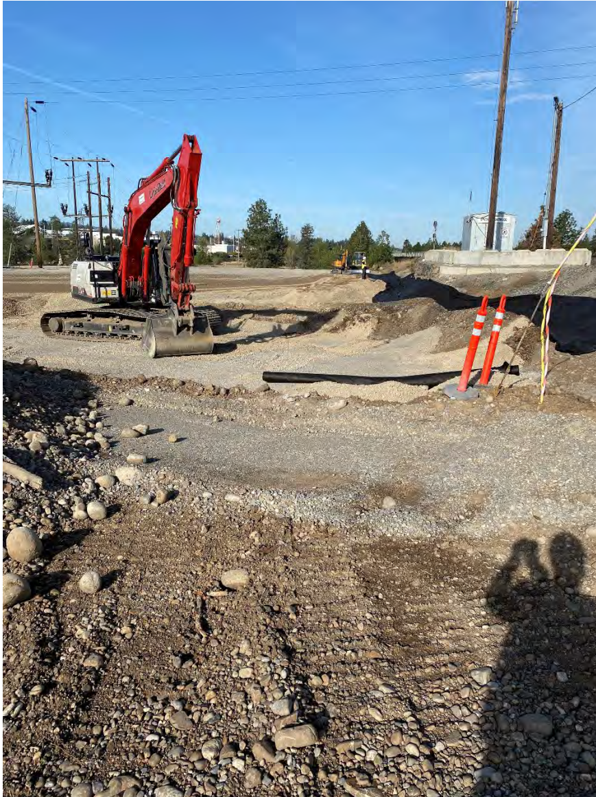
Photograph 1: Placing fabric and clean imported backfill along Pentzer/UPRR boundary.
