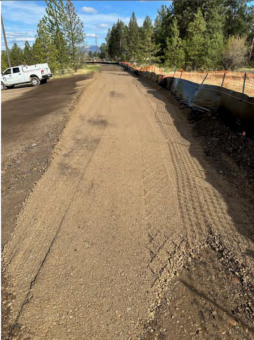
Photograph 6: Backfilling section of southern road to final grade
