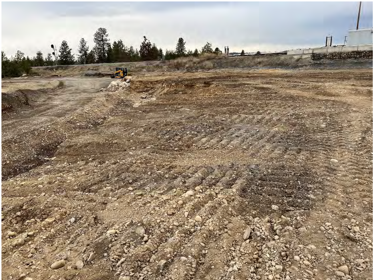
Photograph 1: NE corner of Pentzer property with dross material observed after 6" of material has been scrapped.
