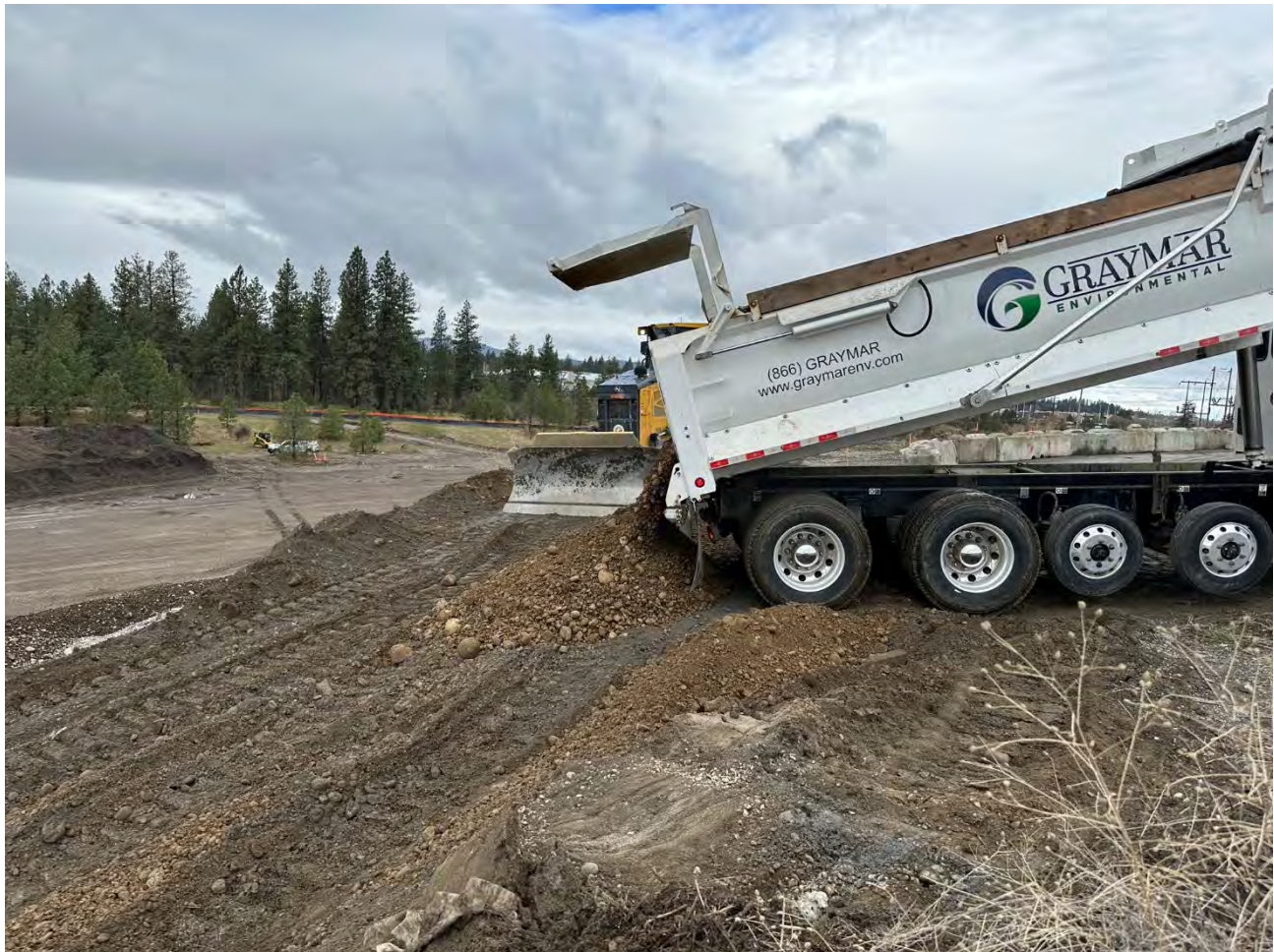
Photograph 1: Adding previously excavated material from Pentzer to UPRR side slope
