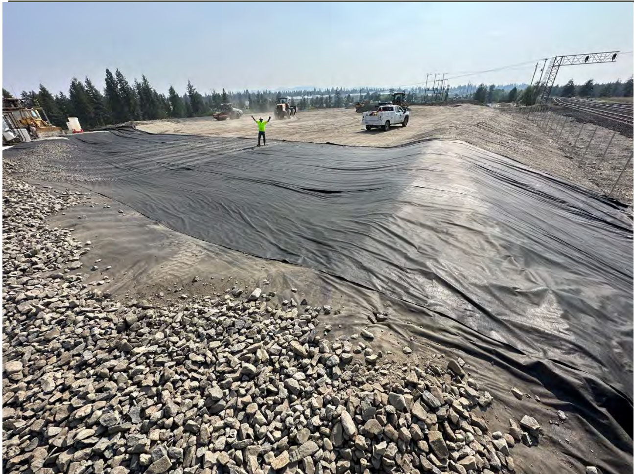
Photograph 2: Filter fabric on north-eastern portion of UPRR pad and berm.
