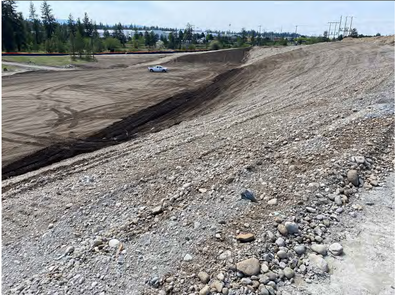
Photograph 3: Constructing 5-foot buffer for WSDOT property at toe of UPRR slope.
