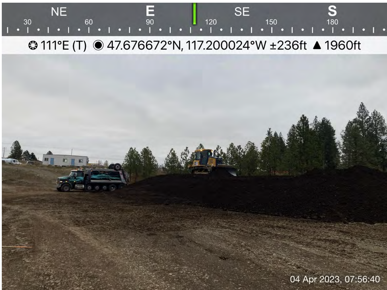
Photograph 1: John Deere 700L dozer manipulating topsoil stockpile.
