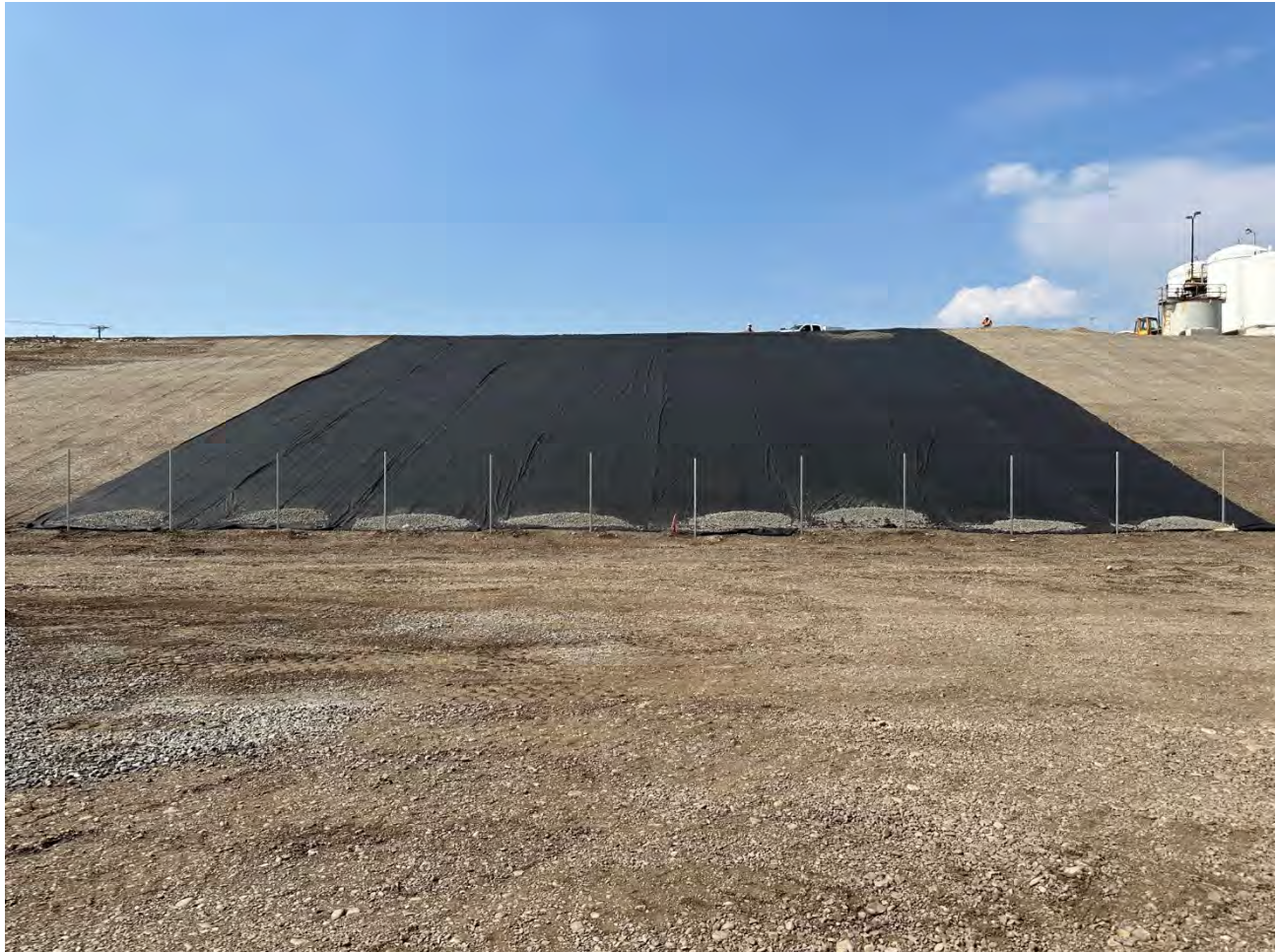
Photograph 1: Filter fabric on center portion of UPRR side slope
