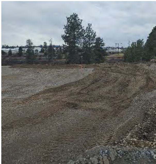
Photograph 2a and 2b: Imported backfill relocated from NW corner of Pentzer property (2a) to the trench (2b) along the UPRR-Pentzer property line via the John Deere 624 loader and LinkBelt 210x4 trackhoe.
