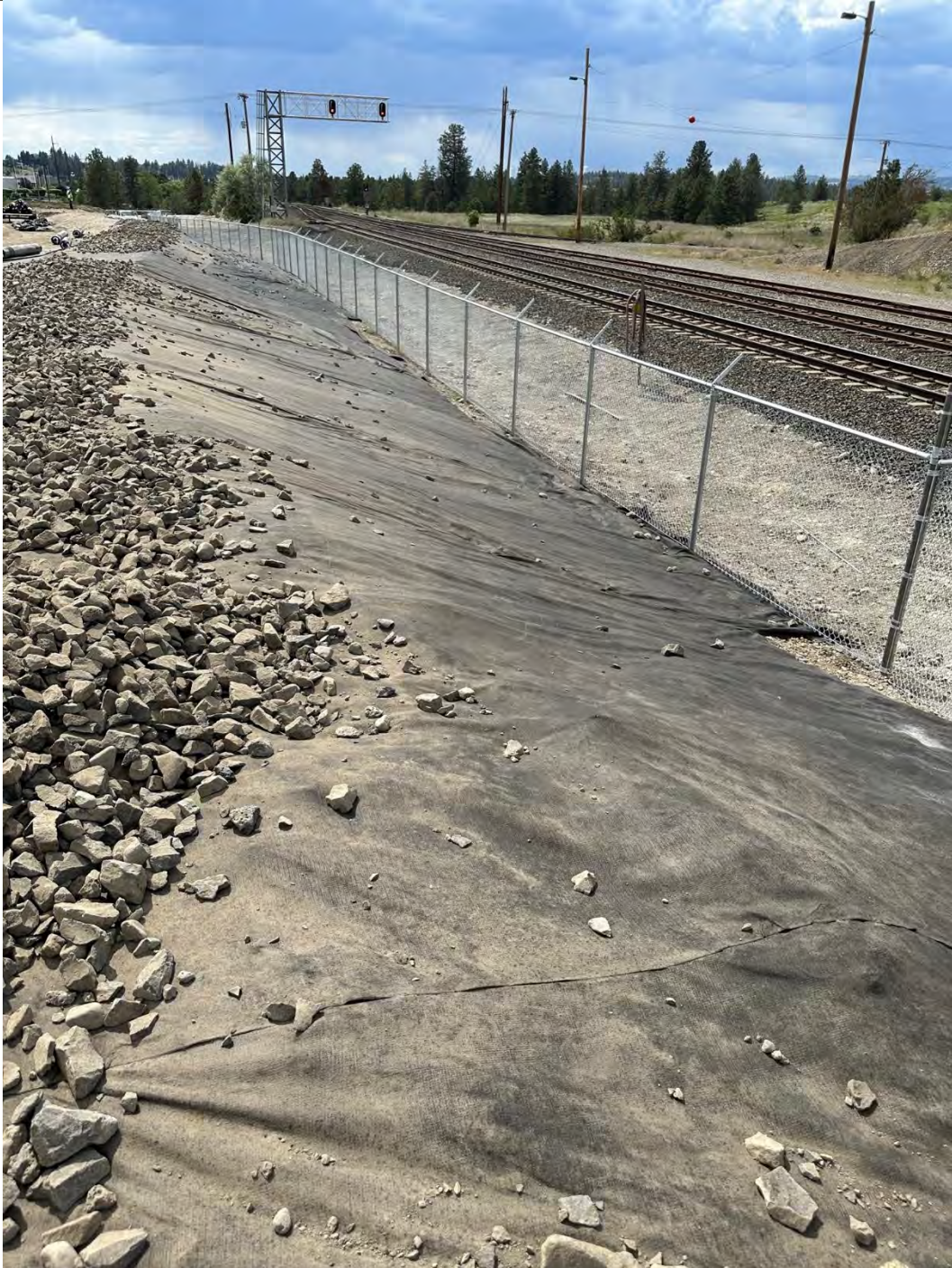
Photograph 6: Adding fencing material to northern portion of UPRR property.
