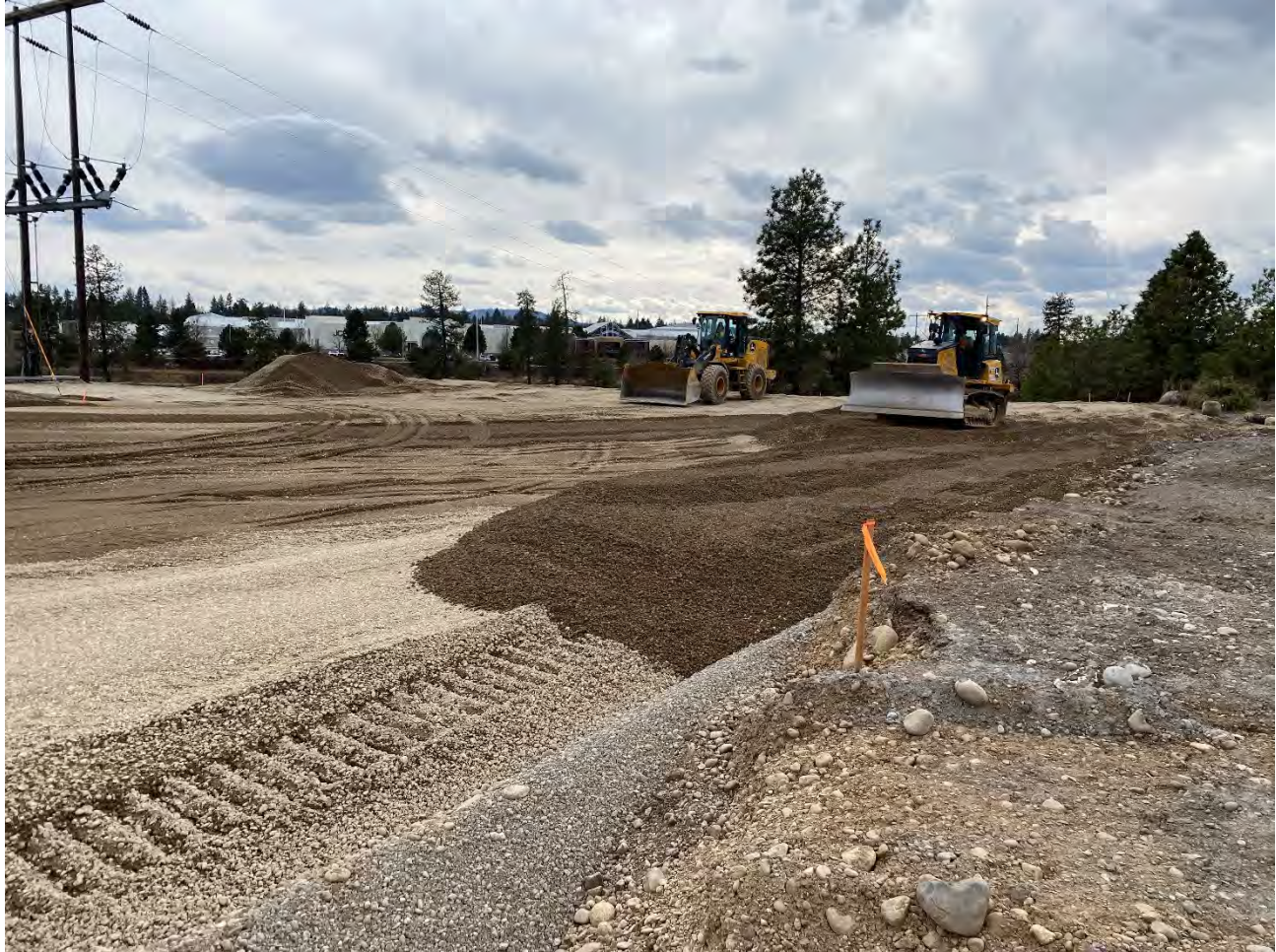
Photographs 1: Placing imported backfill for Excavation 1 and Excavation 2 on Pentzer property.
