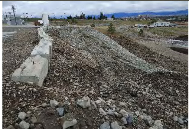
Photograph 2a and 2b: UPRR side slope south of Kemira Facility shows no signs of stormwater erosion.
