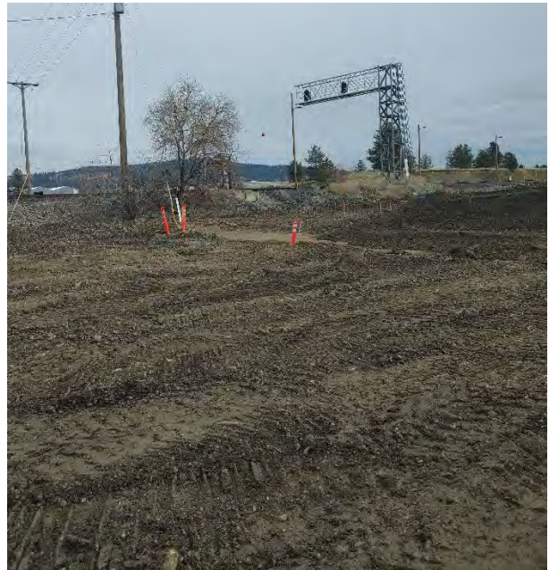
Photograph 2a and 2b: Imported backfill relocated from NW corner of Pentzer property (2a) to the trench (2b) along the UPRR-Pentzer property line via the John Deere 624 loader and LinkBelt 210x4 trackhoe.
