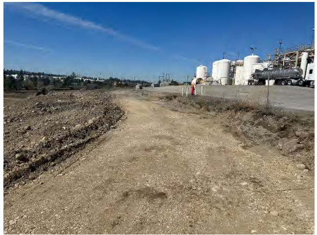
Photographs 1 & 2: Diversion berm grading at top of UPRR slope adjacent to Kemira facility looking east (left) and west (right)
