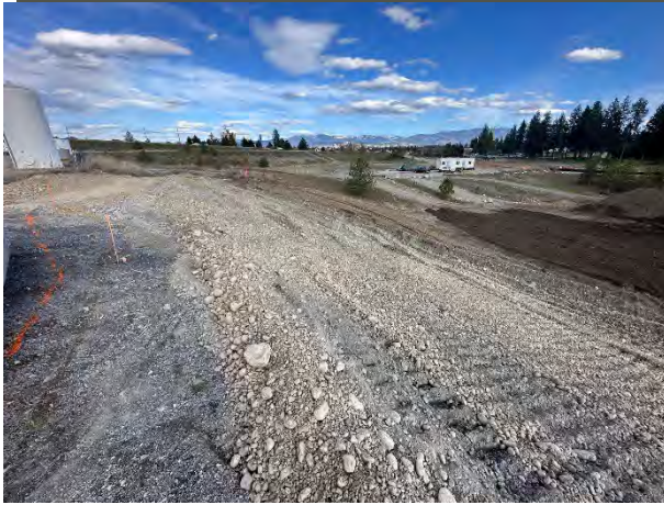
Photographs 3 & 4: Grading UPRR sloped area and ~70% removal of lobe on western side of sloped section.
