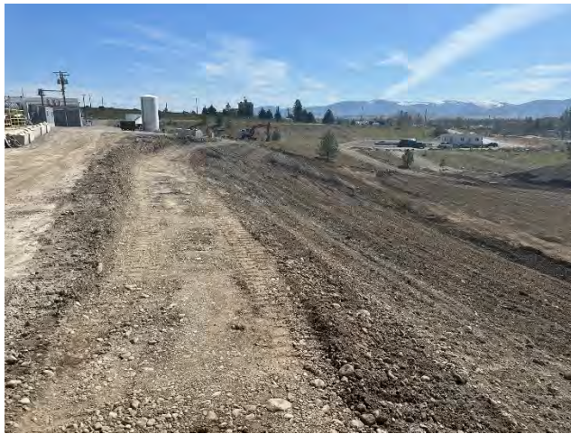
Photographs 1 & 2: Diversion berm grading at top of UPRR slope adjacent to Kemira facility looking east (left) and west (right)
