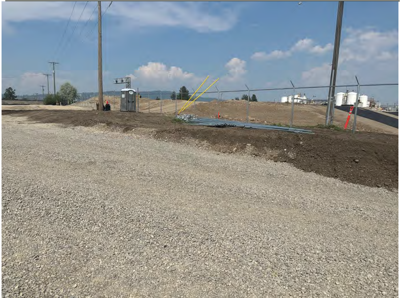
Photograph 4: Fence material on western portion of UPRR property.
