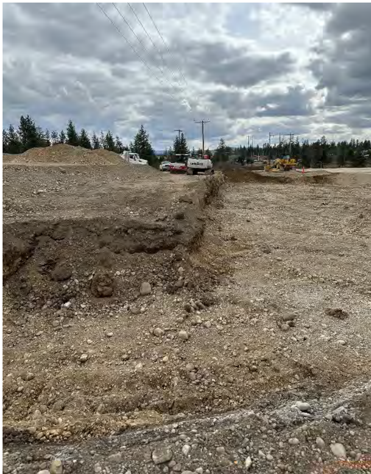
Photograph 1: NE Pentzer property wedge area excavation facing south.
