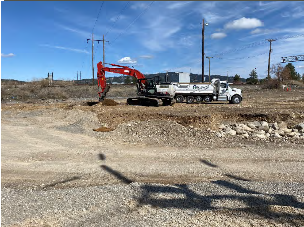
Photograph 3: Excavation of dross impacted soil in the NE Pentzer property wedge.
