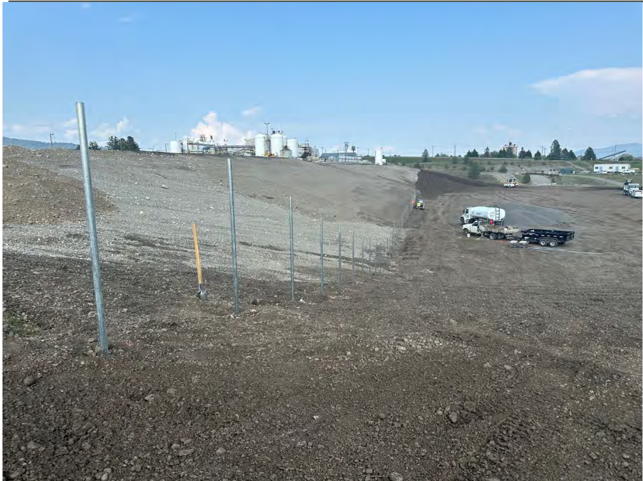
Photograph 2: Installation of fence on southern portion of UPRR property.
