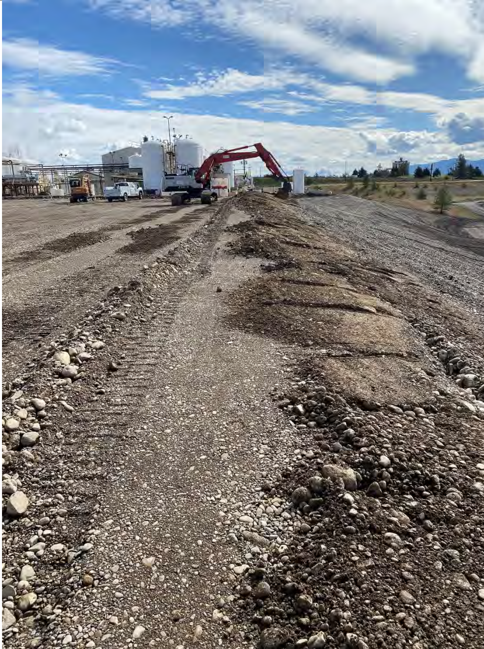
Photograph 3: Building containment berm on south side of UPRR pad.
