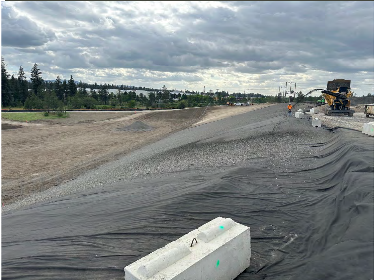
Photograph 3: Spreading 6" of gravel on middle section of UPRR slope.
