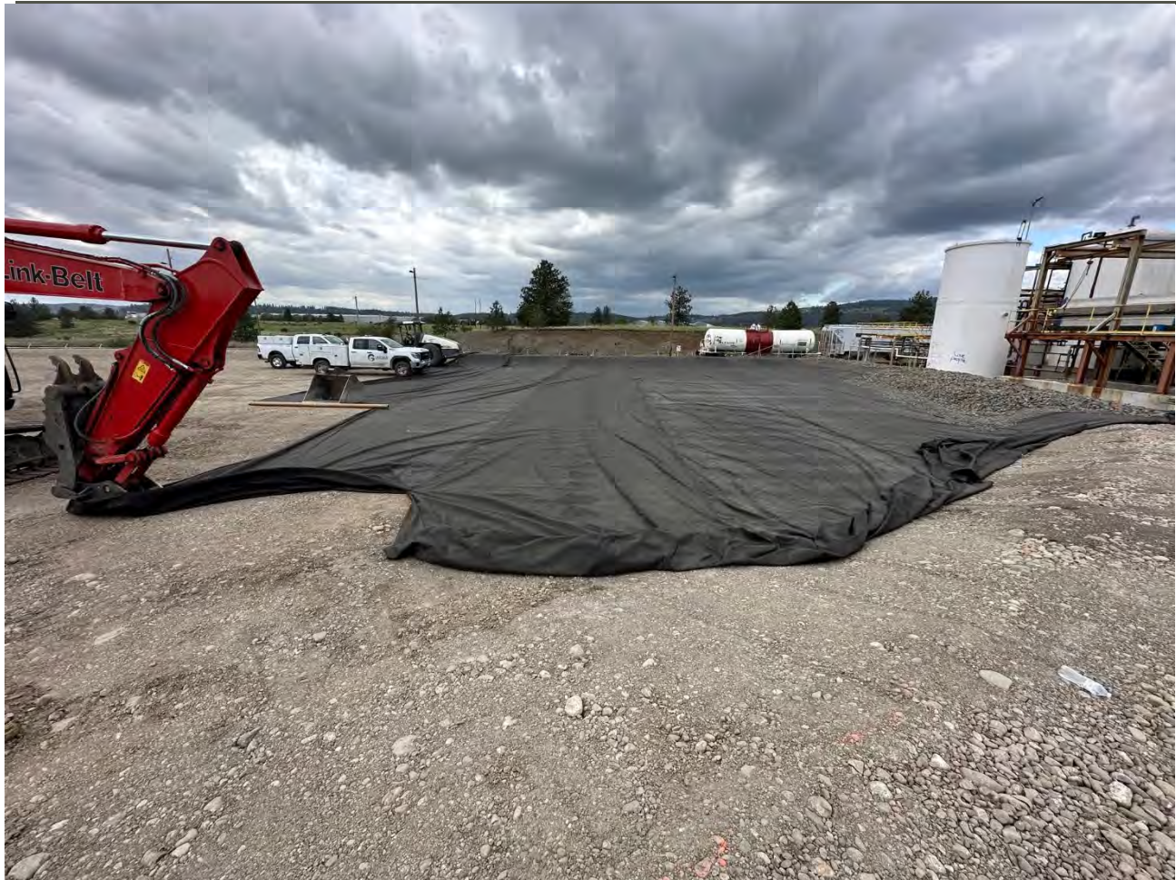
Photograph 2: Filter fabric on eastern portion of UPRR pad
