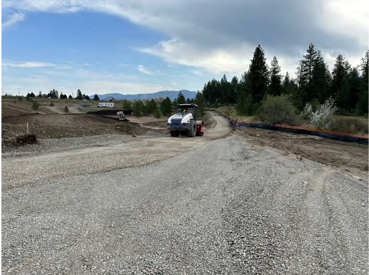
Photograph 5: Backfilling southern road section to final grade
