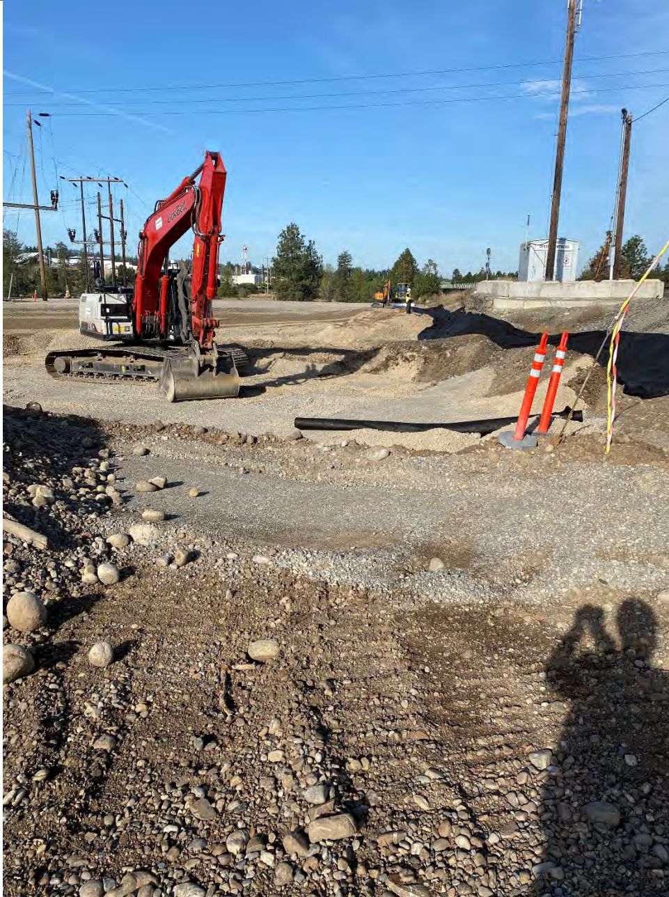
Photograph 3: Placing fabric along Pentzer/UPRR property boundary cut.
