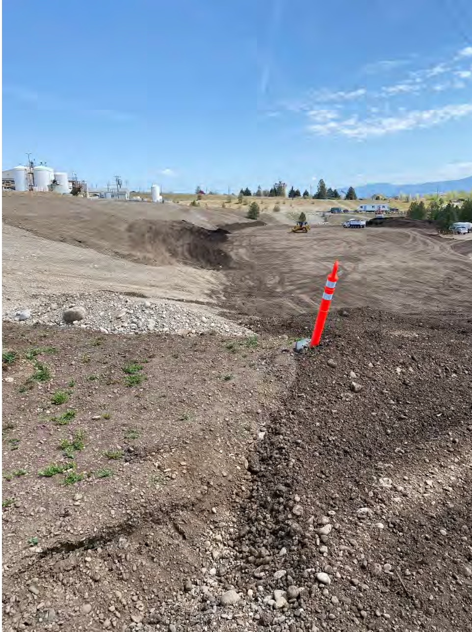
Photograph 1: construction of 5-foot buffer on WSDOT property boundary.
