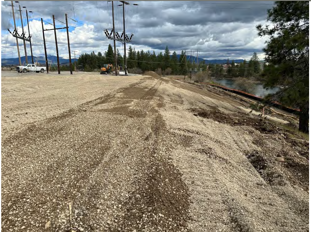
Photograph 3: Grading backfill on Pentzer and Parks and Recreation properties
