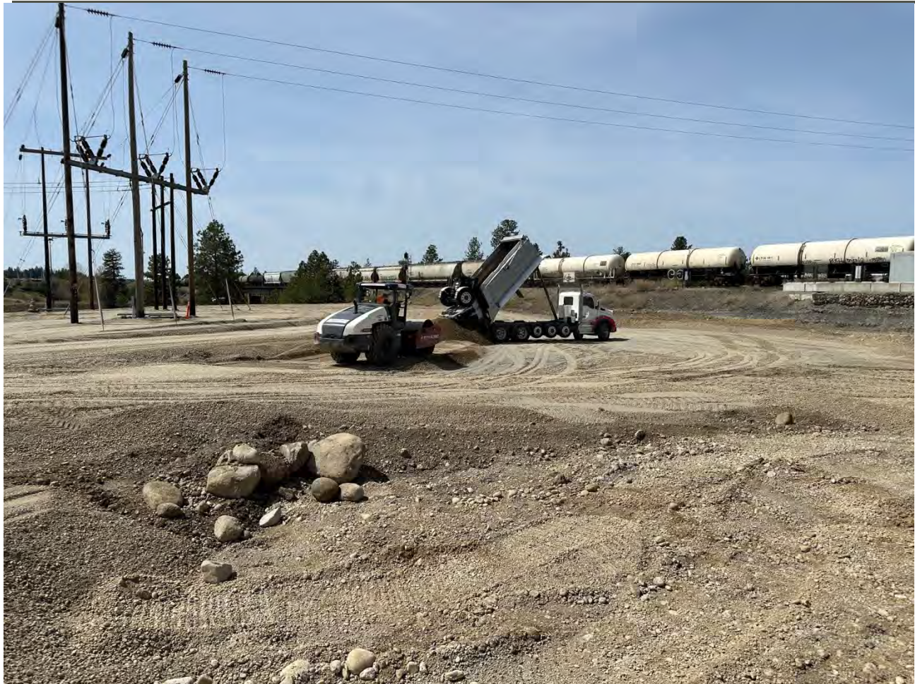
Photograph 4: Backfilling Excavation 2 on Pentzer property.
