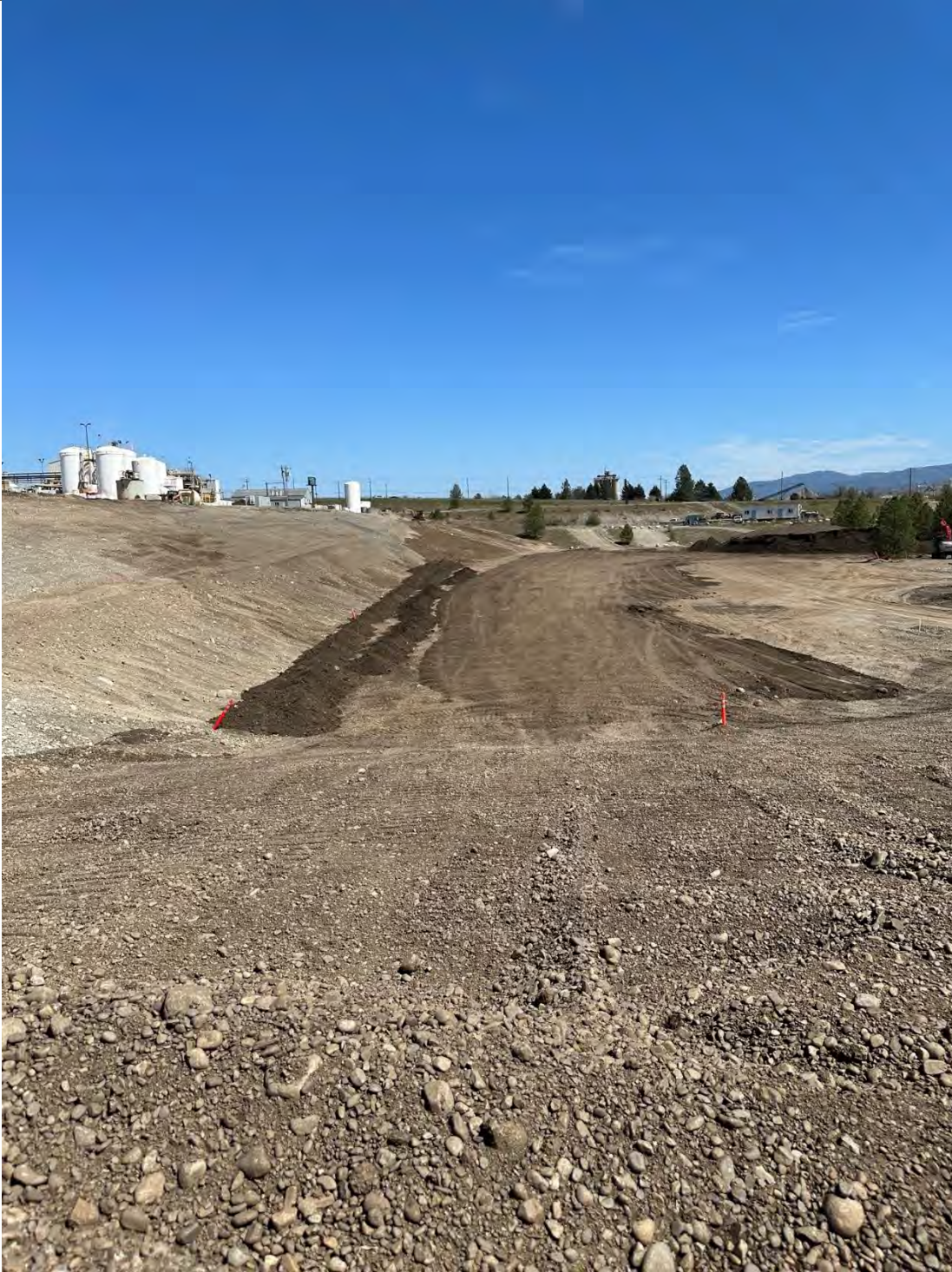
Photograph 4: Placing 6-inch lift of topsoil on WSDOT property
