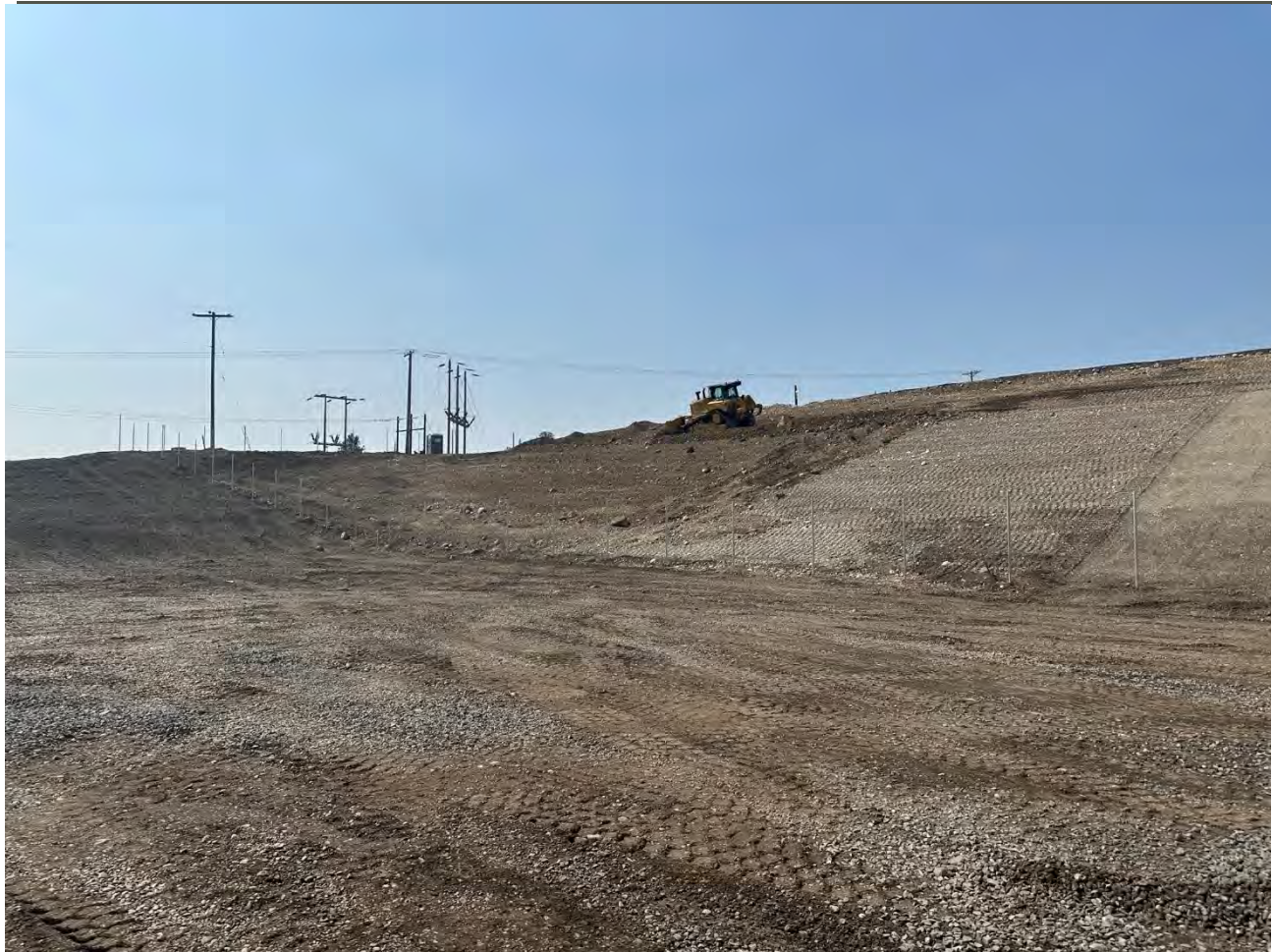
Photograph 4: Grading western portion of UPRR side slope.
