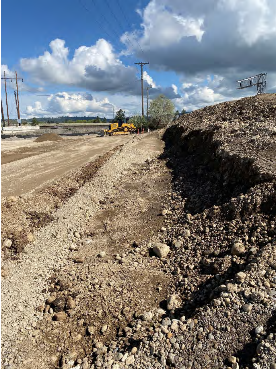
Photograph 1: Cutout of western slope on UPRR pad to construct 5-foot buffer.
