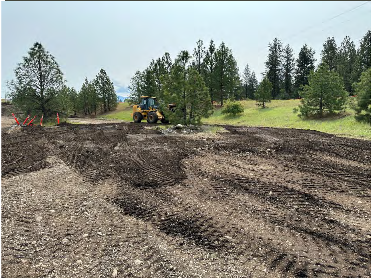
Photograph 4: Placing topsoil on southern portion of WSDOT pad.
