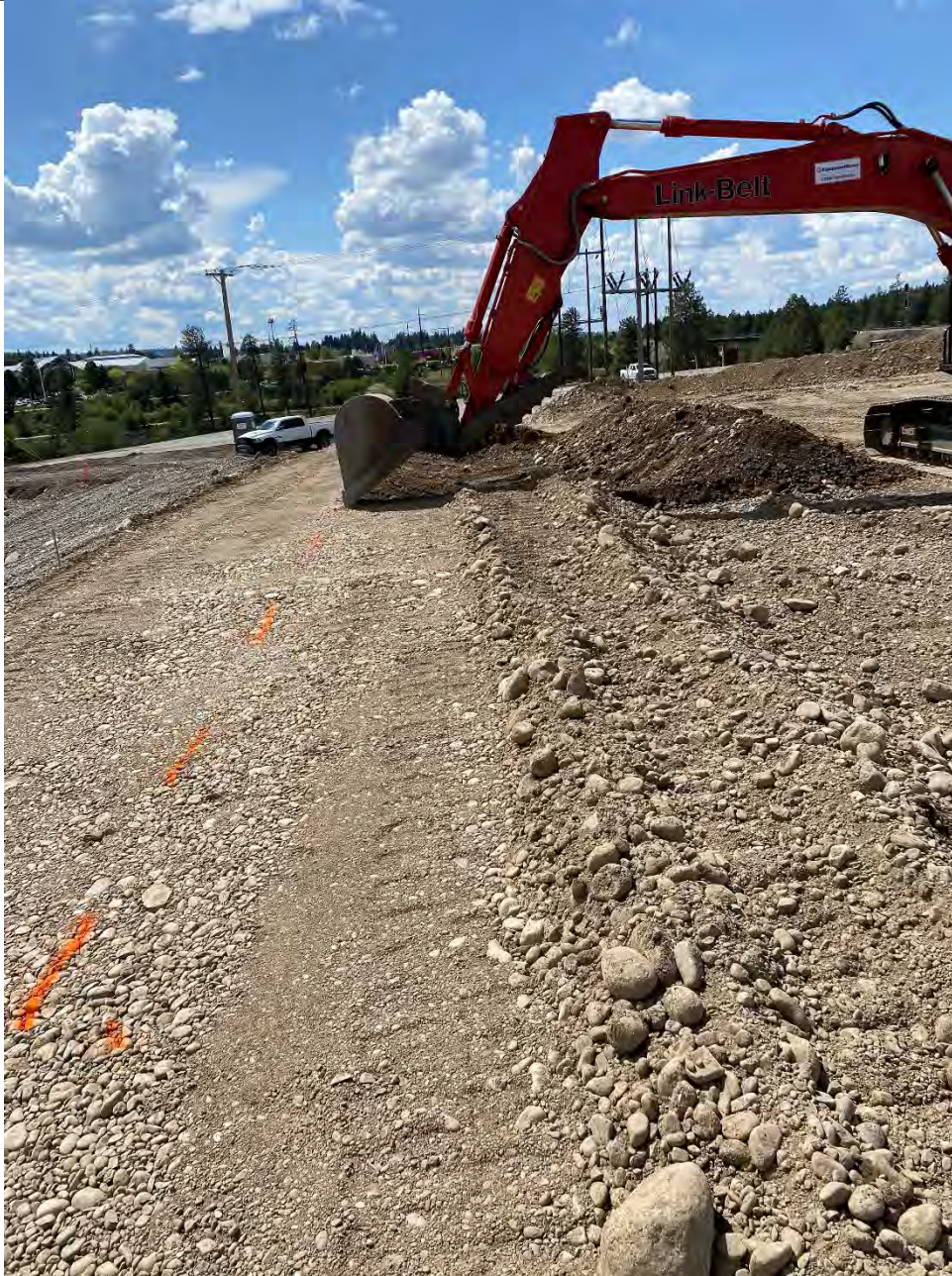
Photograph 5: Cutting backside of south UPRR pad (interior) containment berm 2 to 1.
