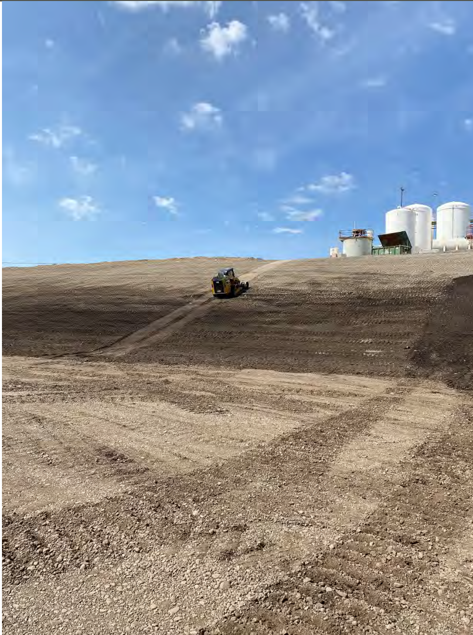
Photograph 2: Testing compaction on UPRR with bobcat roller.
