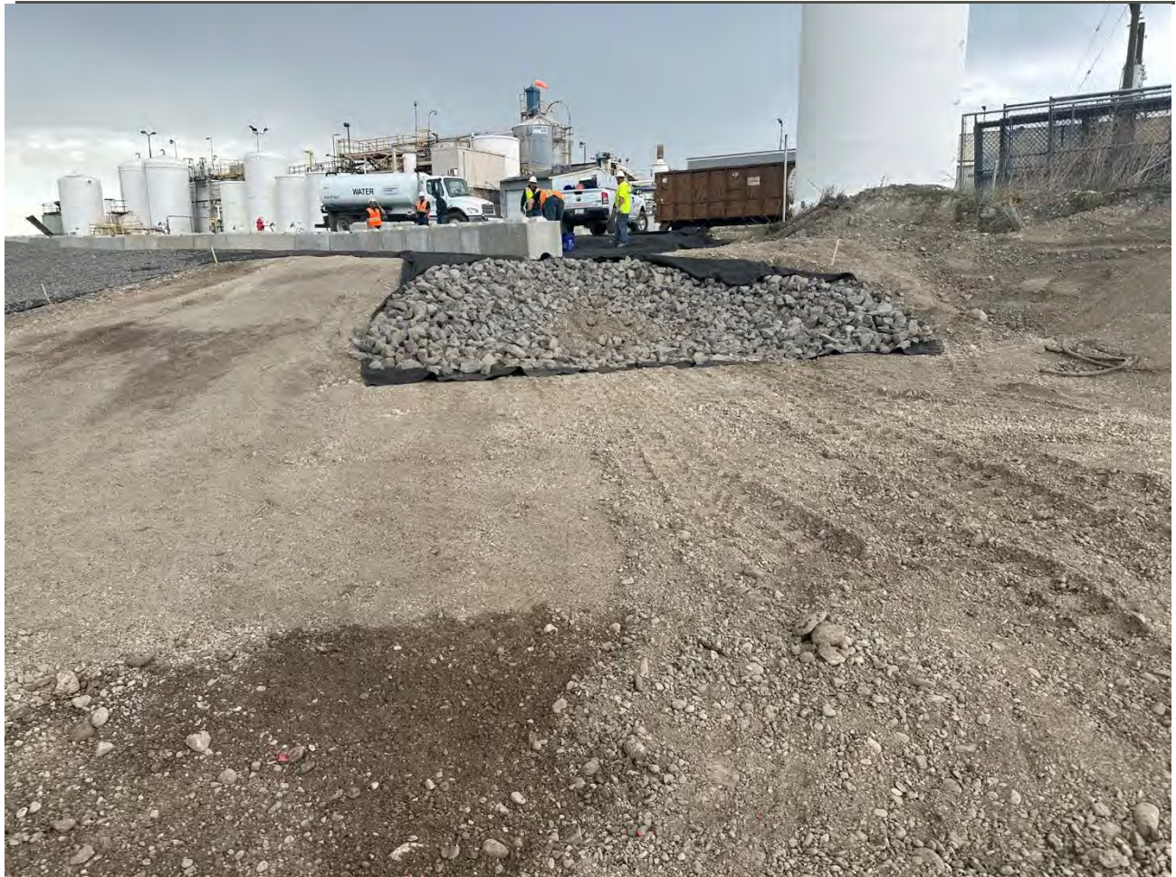
Photograph 5: Splash pad with 2-8" armor rock.
