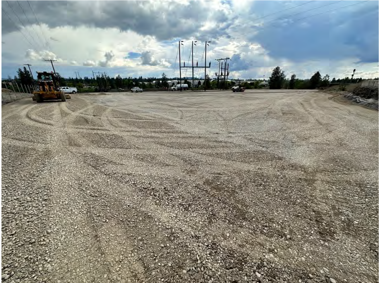
Photograph 1: Backfilling and compacting NE wedge portion on Pentzer.
