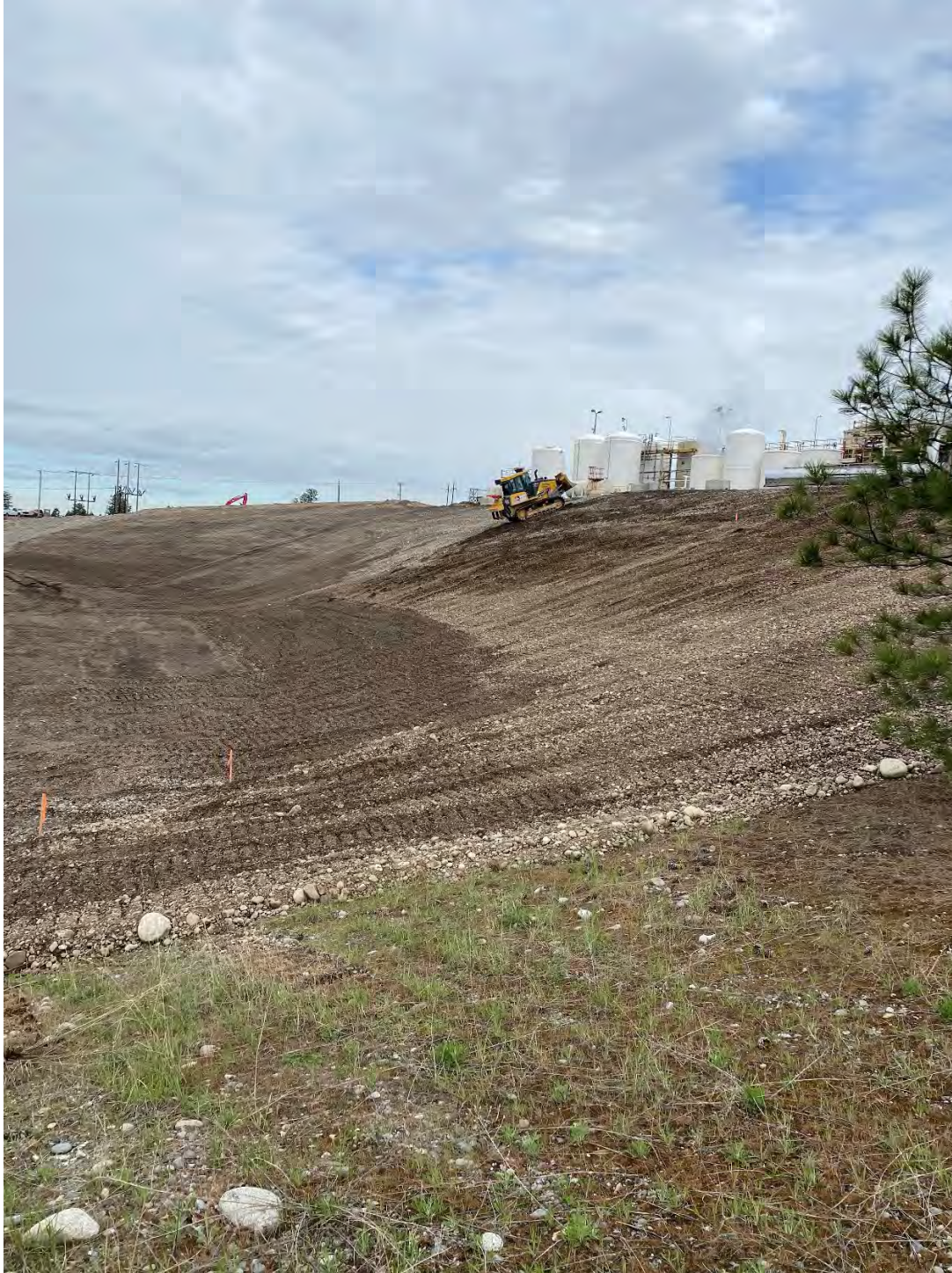
Photograph 1: Tracking southern UPRR slope prep for fabric.
