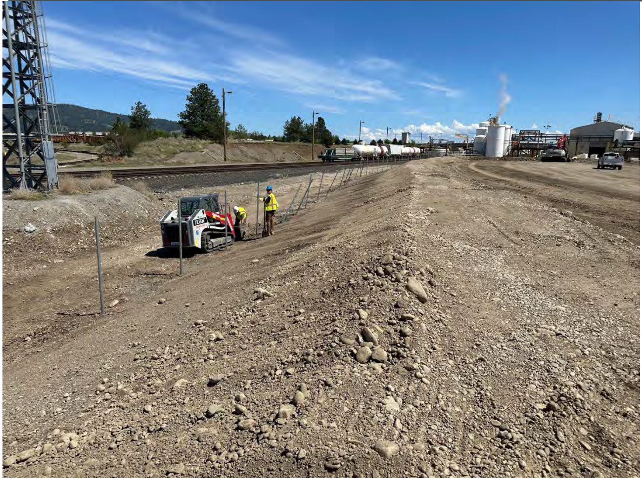
Photograph 3: Installation of fence on northern portion of UPRR property.
