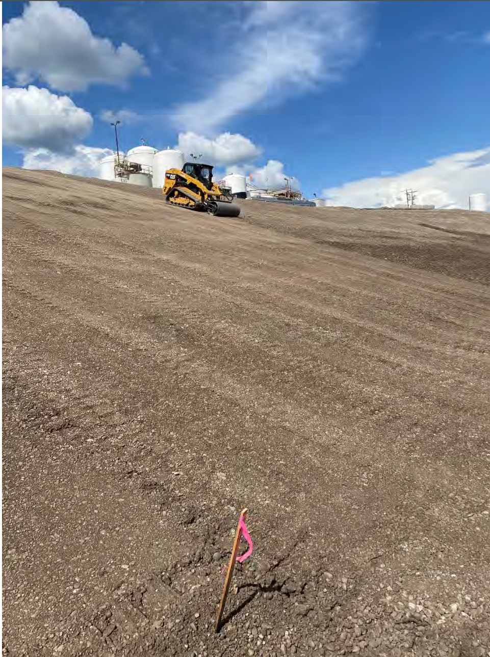
Photograph 2: Rolling/compacting south UPRR slope in preparation for fabric placement.
