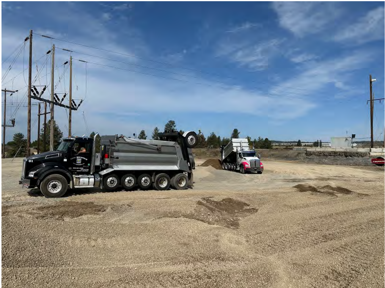
Photograph 1: Backfilling Excavation 2 on Pentzer property
