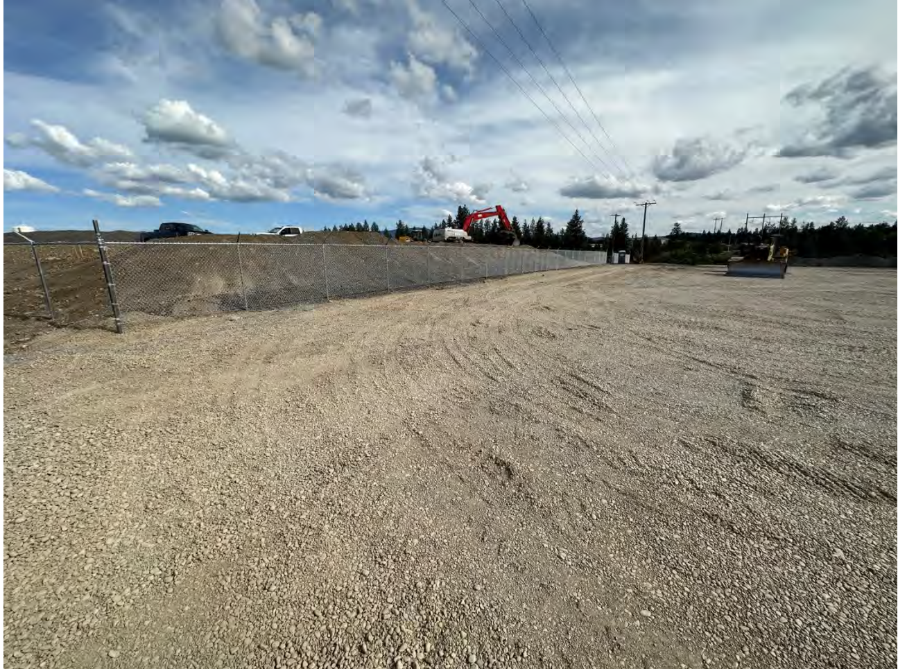
Photograph 5: Fencing material added to western portion of UPRR property.
