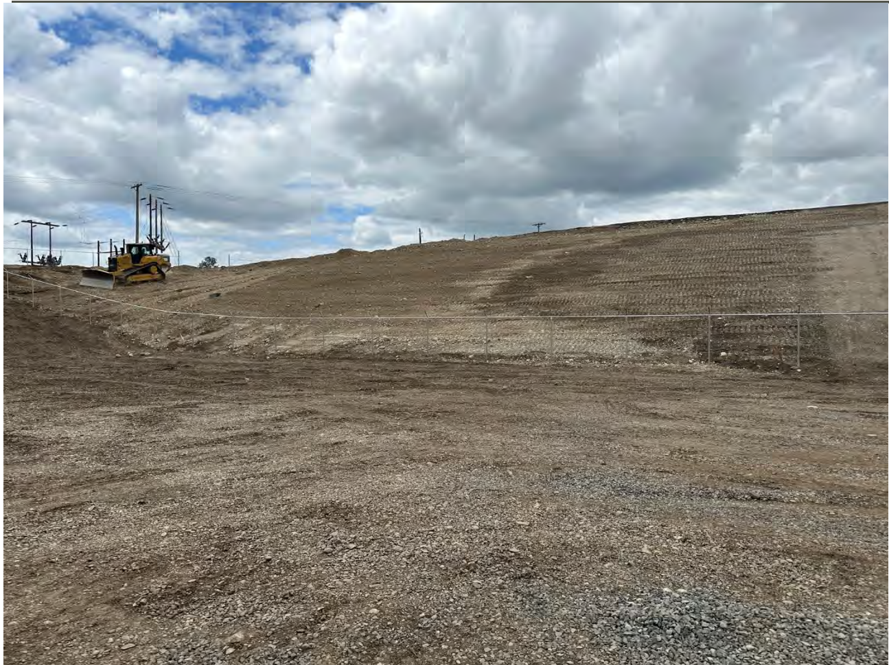
Photograph 4: Grading western portion of UPRR side slope.
