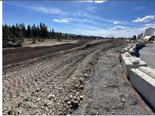
Photographs 3 & 4: Grading UPRR sloped area and ~70% removal of lobe on western side of sloped section.
