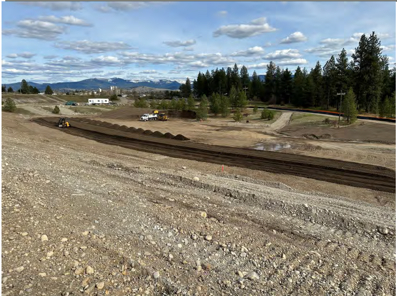
Photograph 4: Placing 6-inch layer of topsoil on WSDOT property
