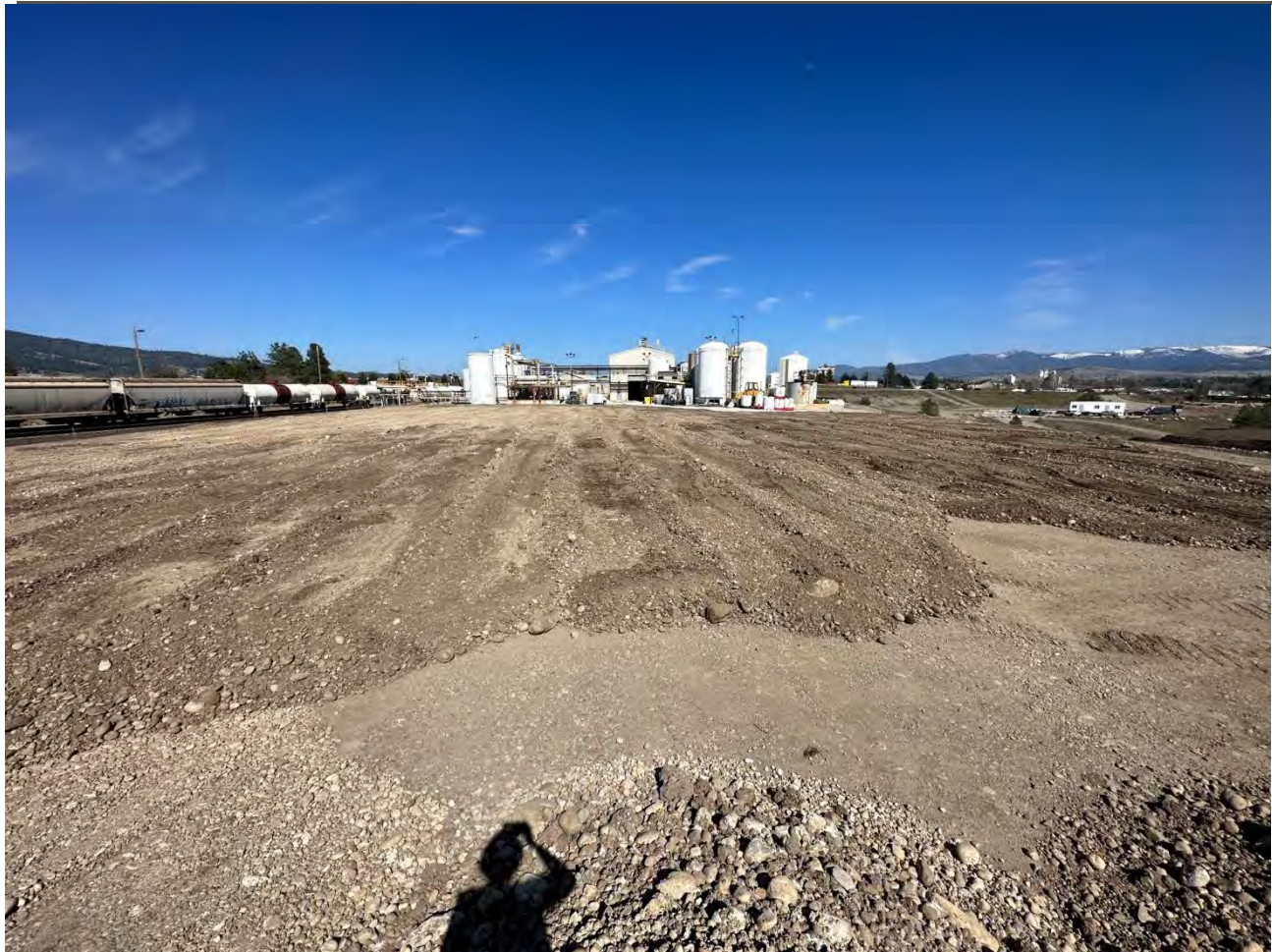
Photograph 5: Spreading excavated material from Pentzer property on UPRR pad
