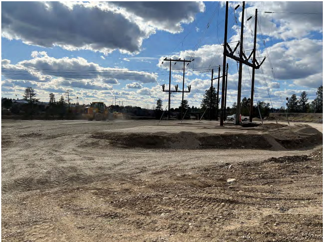
Photograph 1: Placement and grading of backfill material on Pentzer property.
