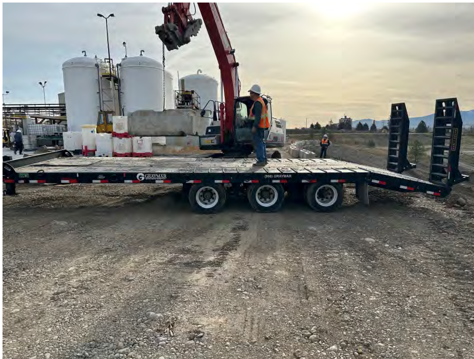
Photograph 1: Removing ecological blocks from top of slope on UPRR property
