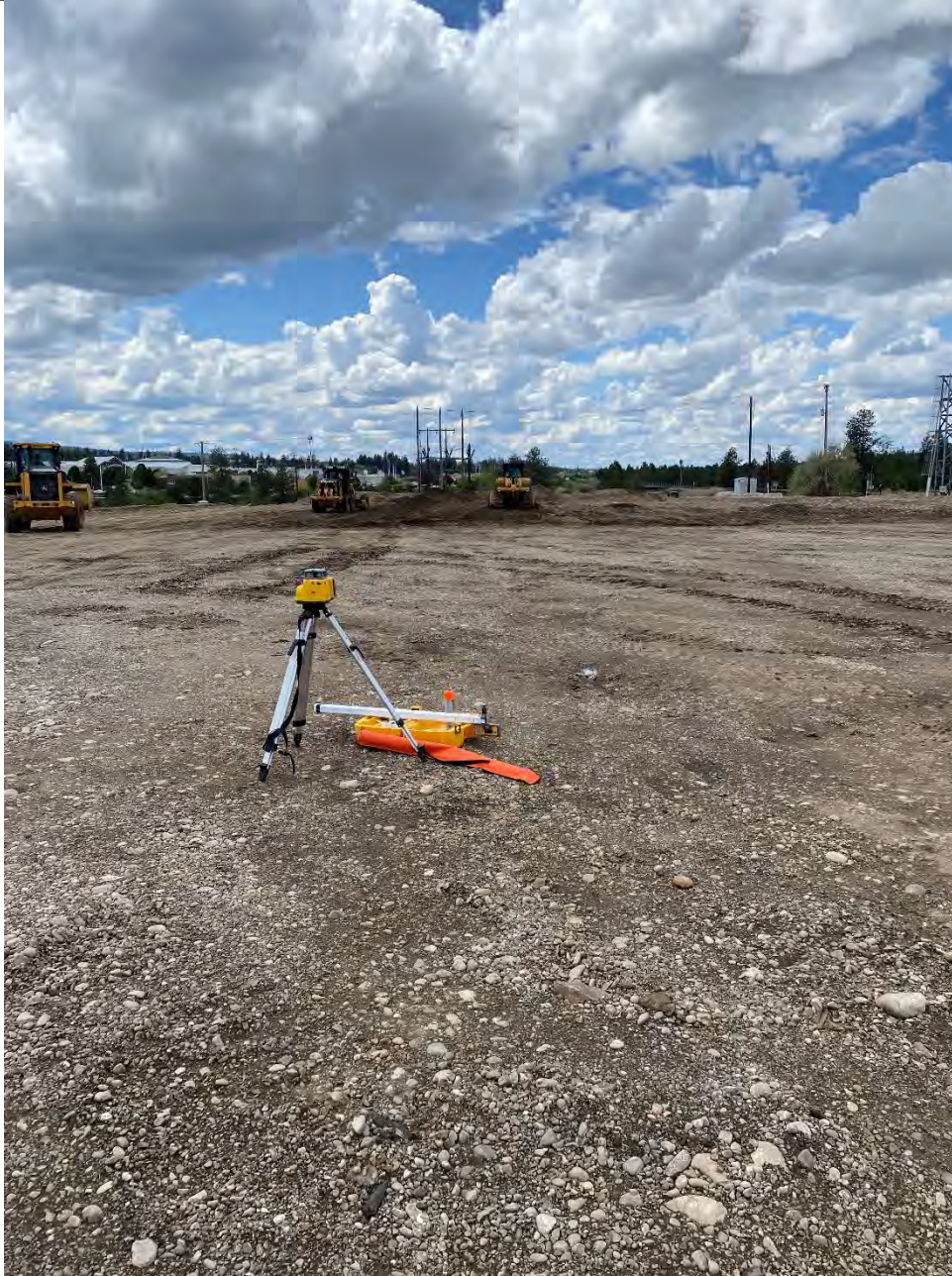
Photograph 2: Grading and compacting UPRR pad.
