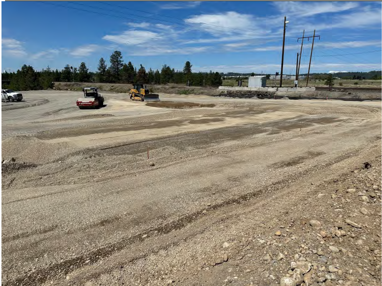
Photograph 5: Backfilling and compacting NE wedge portion on Pentzer.
