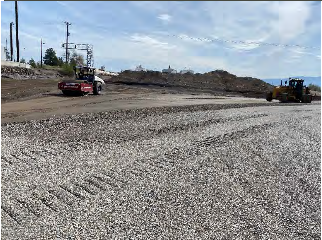
Photograph 2: Backfilling and compacting Pentzer NE wedge area
