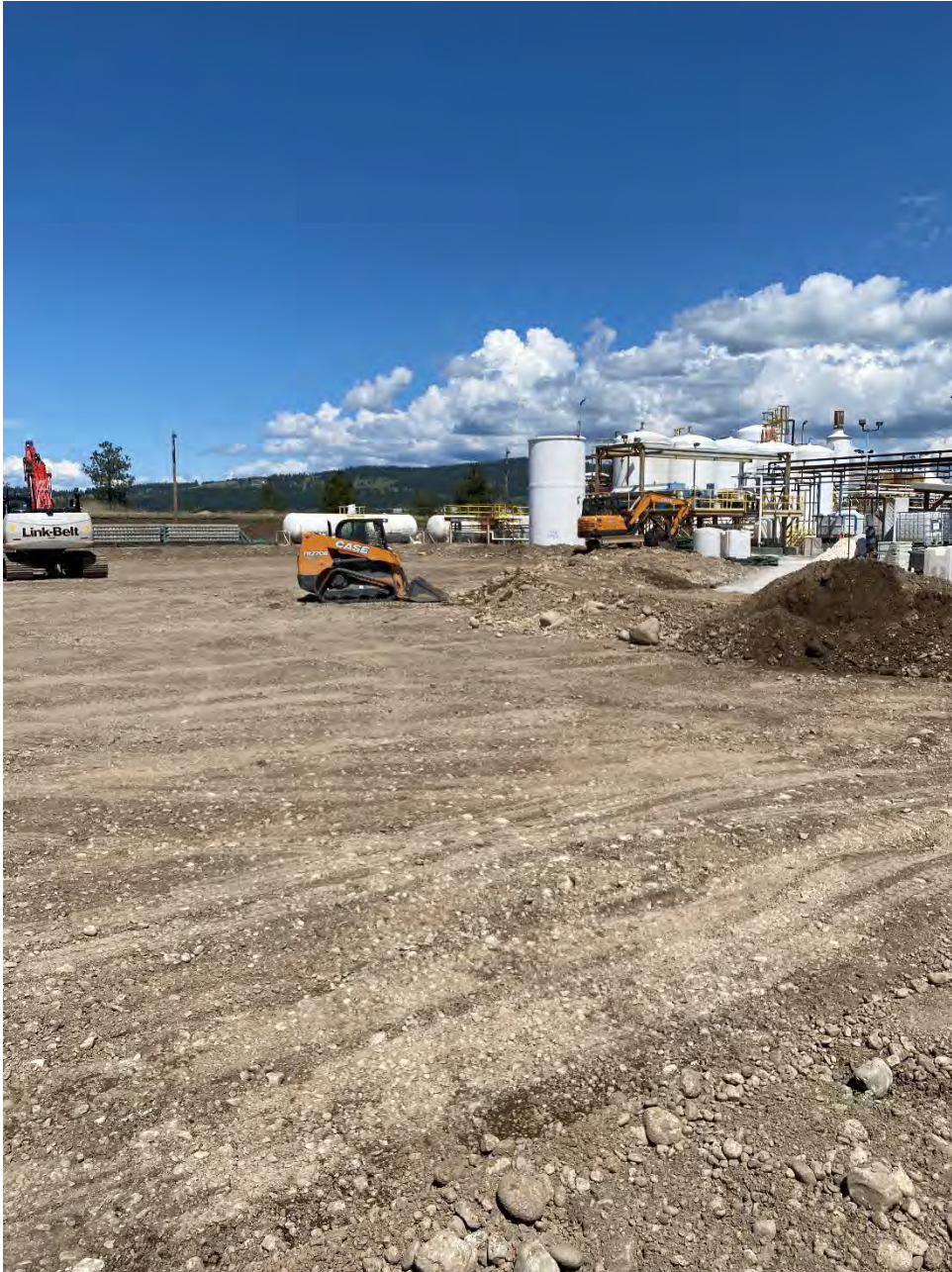
Photograph 1: Constructing East portion of containment berm near Kemira facility.
