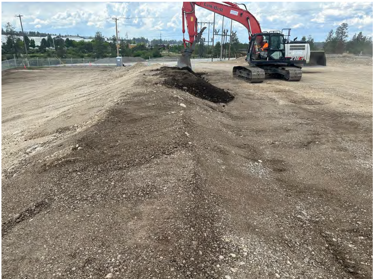
Photograph 4: Constructing diversion berm on western portion of UPRR pad.
