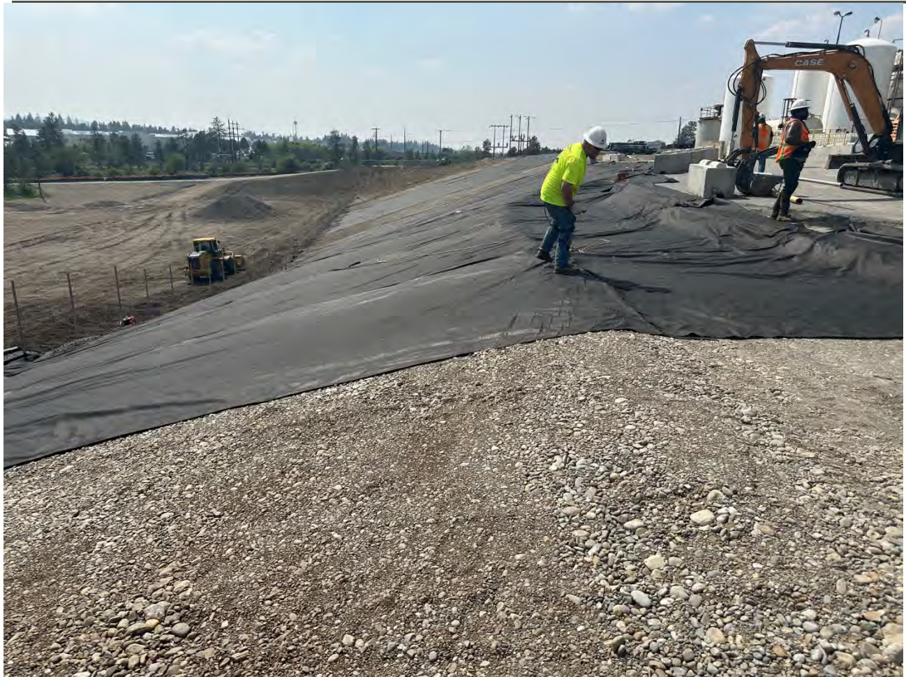
Photograph 3: Filter fabric on Kemira diversion ditch and UPRR side slope.
