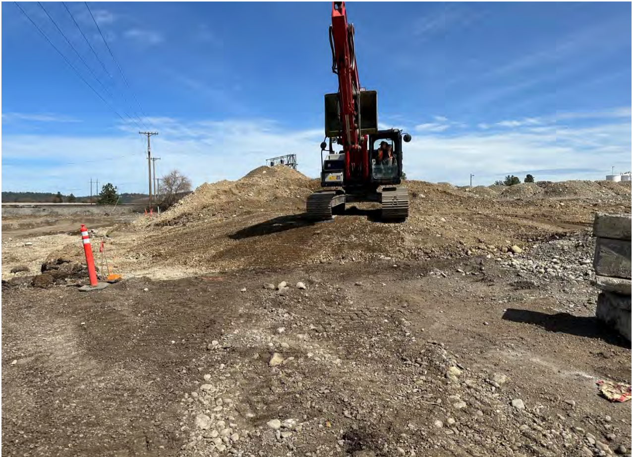
Photograph 5: Backfilling and grading sloped section from UPRR to Pentzer property
