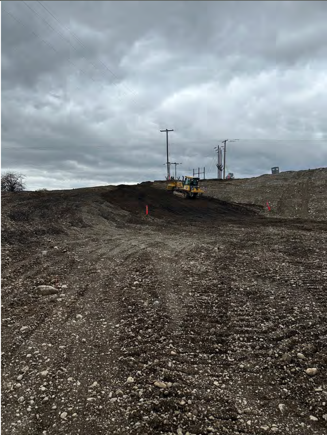
Photograph 4: Grading Southwestern slope on WSDOT Property
