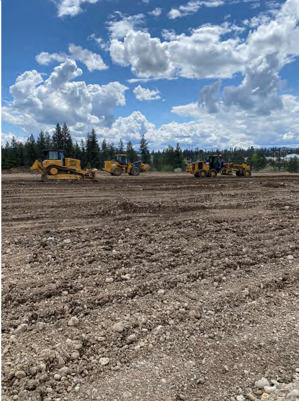
Photograph 4: Placing Pentzer property soil on UPRR pad and grading.
