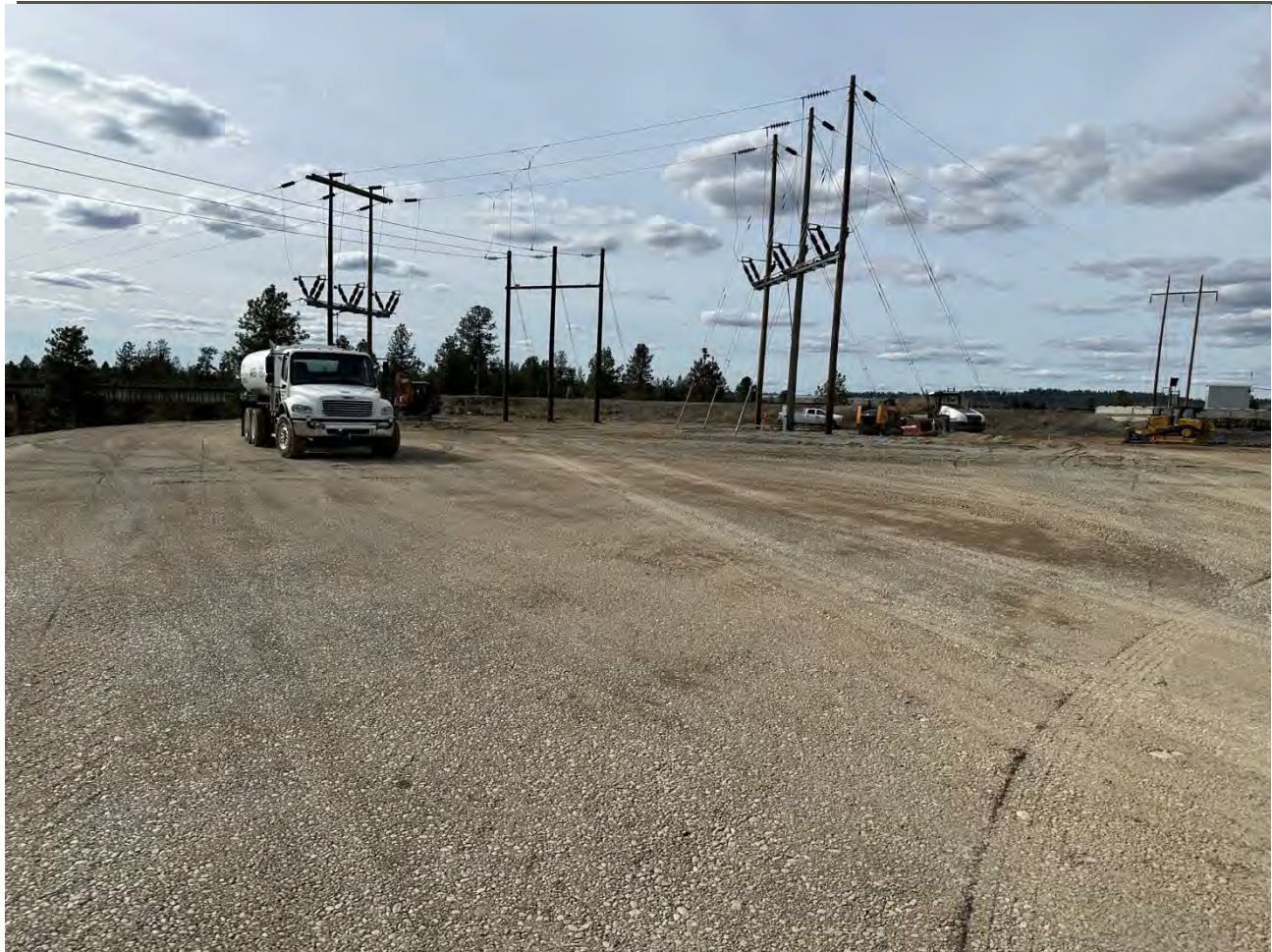
Photograph 3: Backfilling and grading Excavation 1 on Pentzer property
