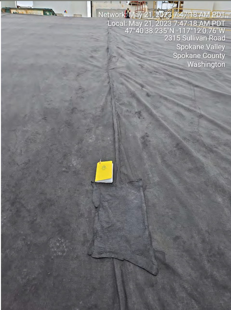
Photograph 3: Completed patch of 15 th seam weld on south slope.
