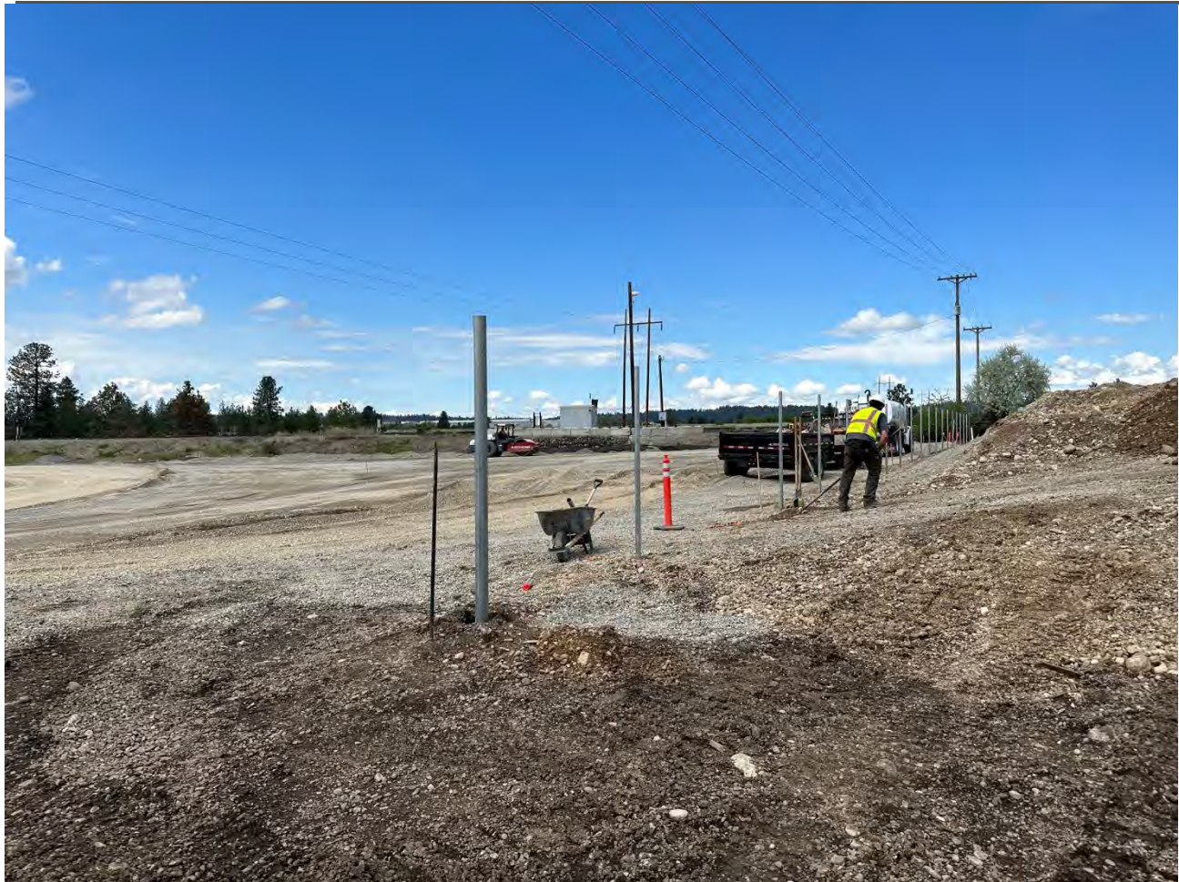
Photograph 2: Installation of fence on western portion of UPRR property.
