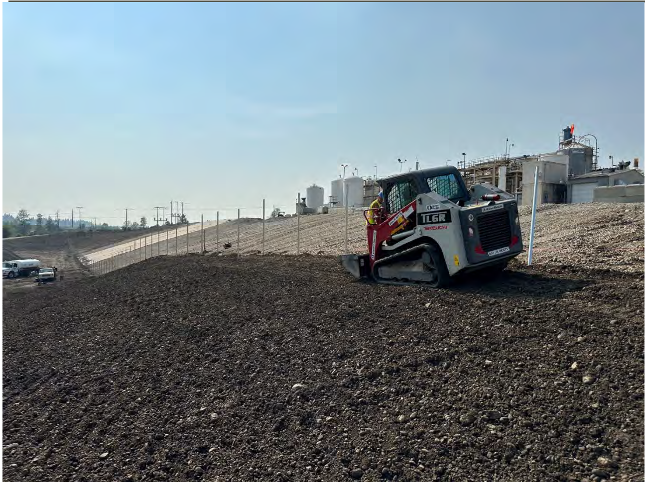
Photograph 3: Installation of fence posts on southern portion of UPRR property.
