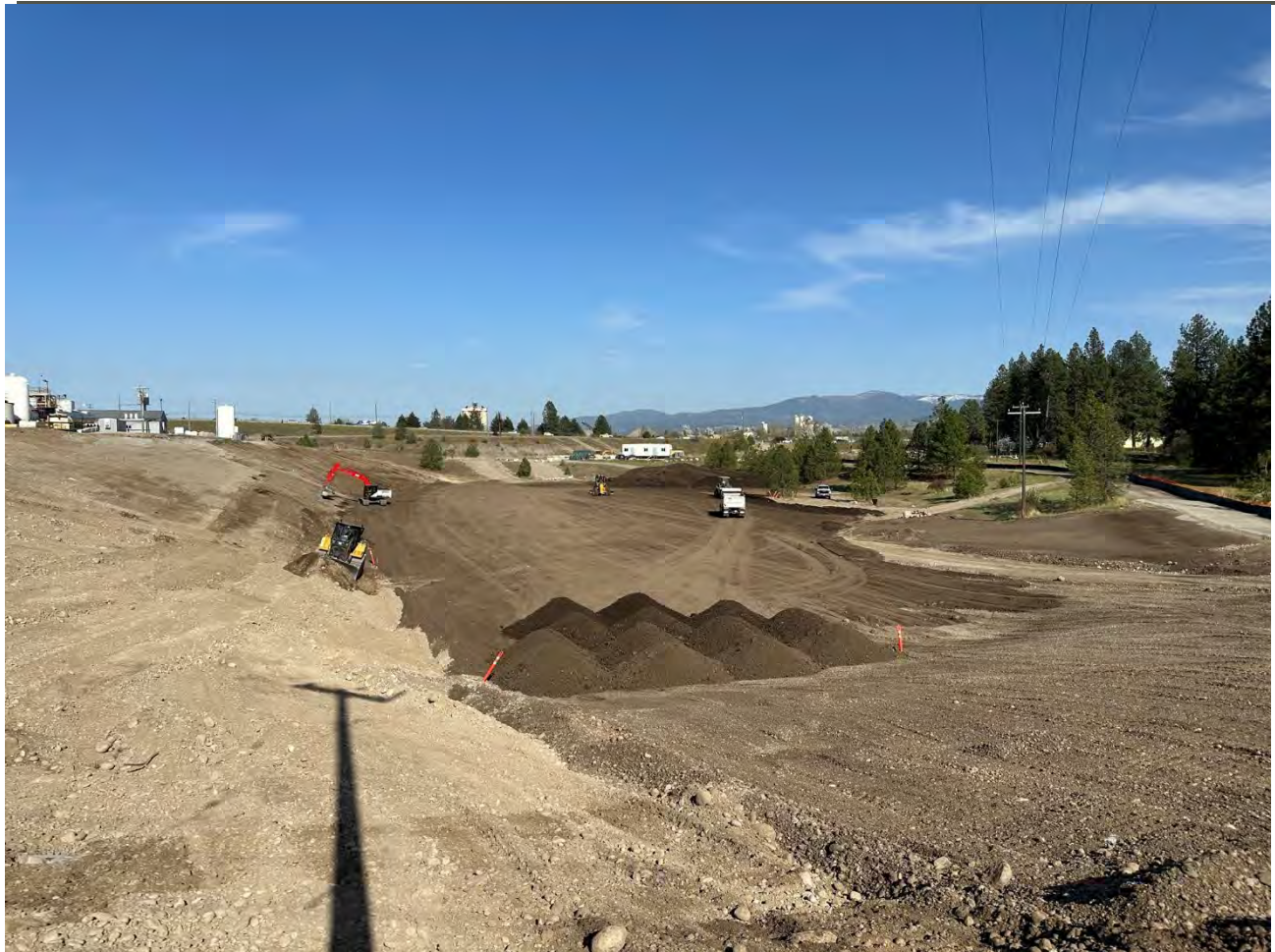
Photograph 3: Placing of topsoil on WSDOT property
