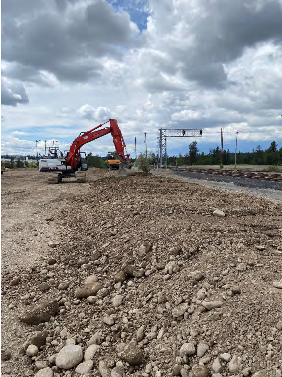
Photograph 2: Building containment berm on north side of UPRR pad.
