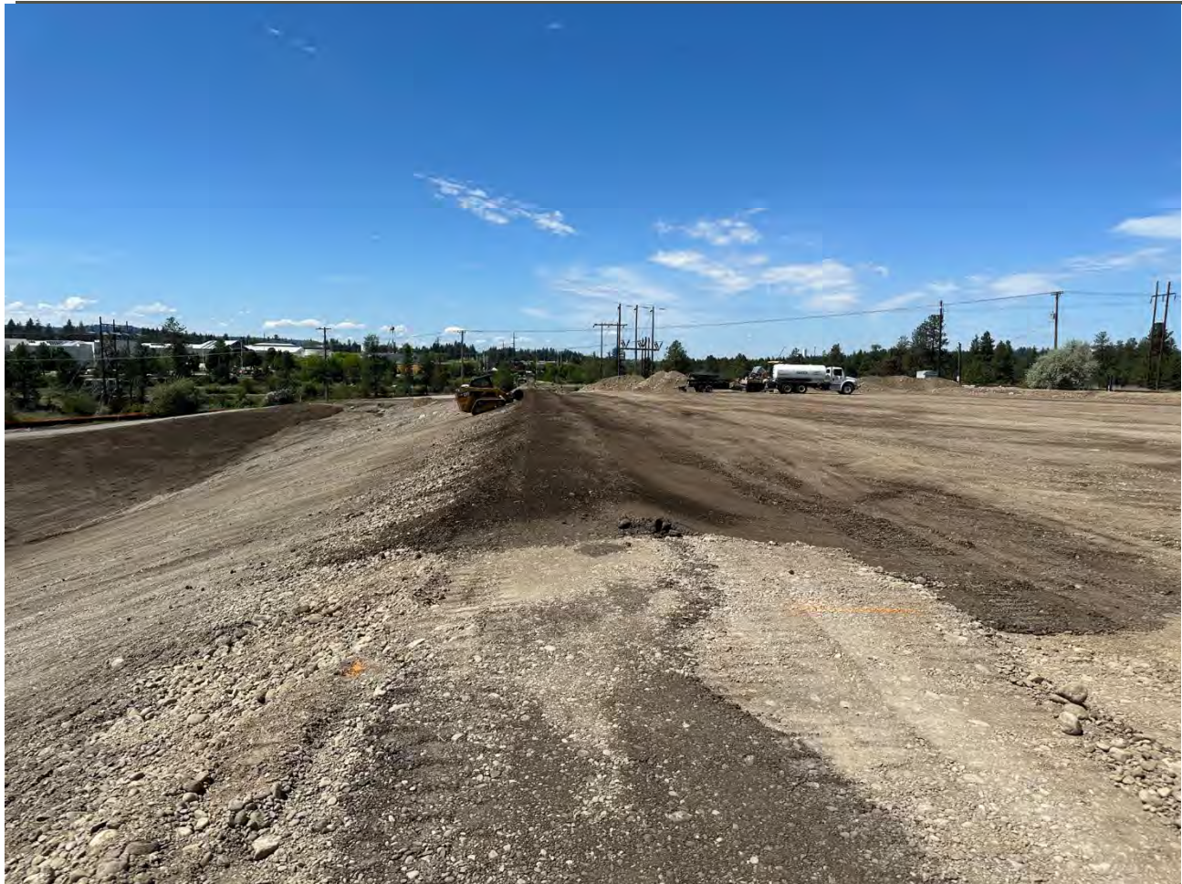
Photograph 2: Completion/ compaction of UPRR containment south berm.
