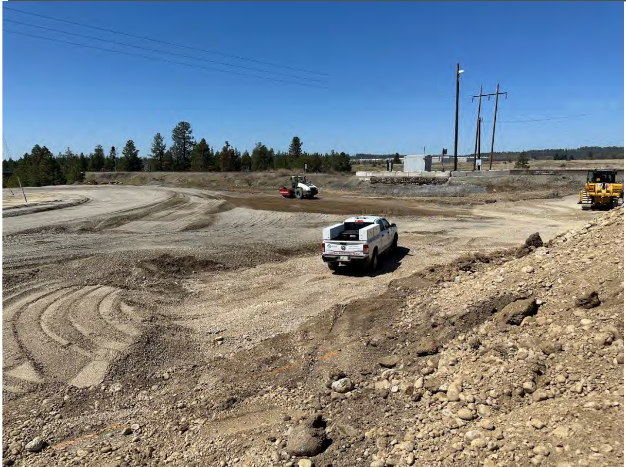
Photograph 3: Backfilling Excavation 2 on Pentzer property
