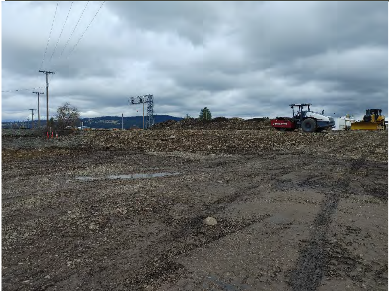
Photograph 4: Capping on the west end of the UPRR property.
