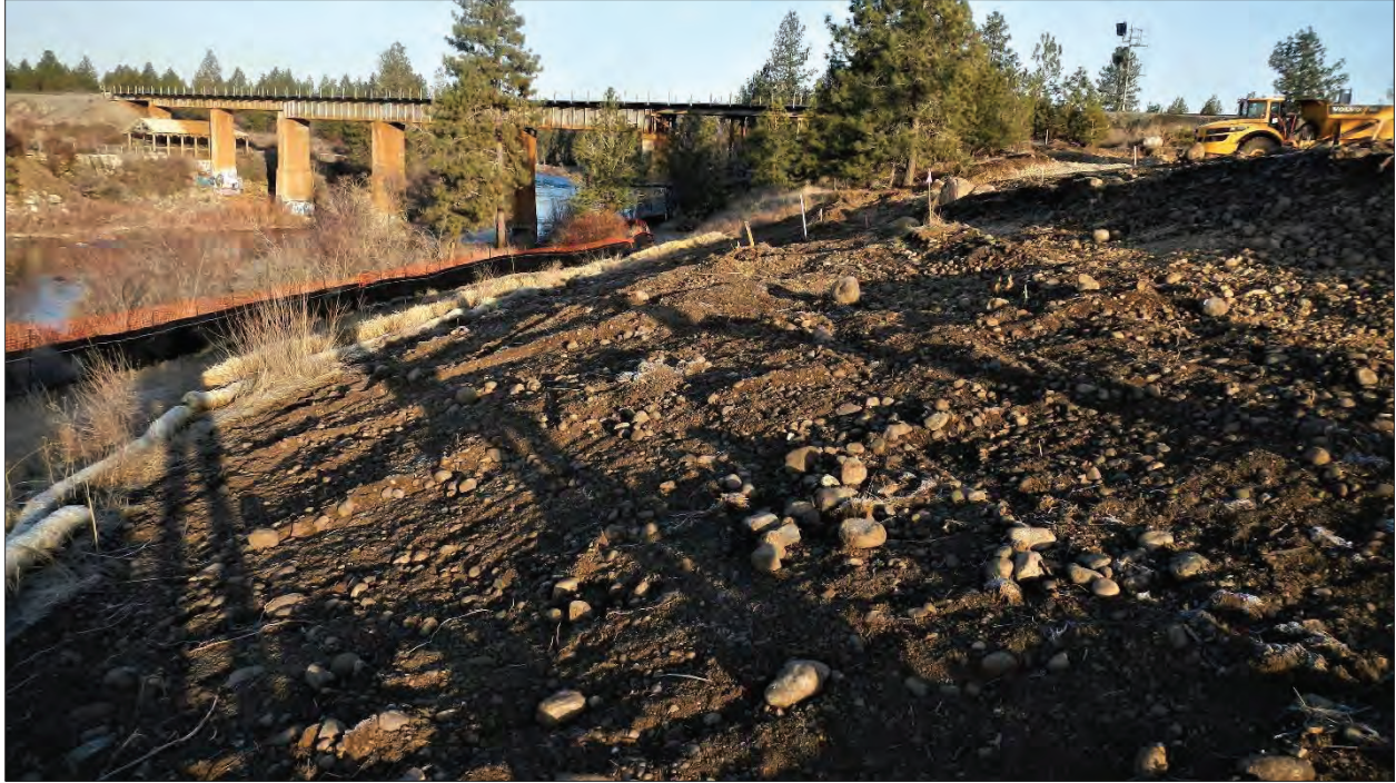
Figure 6. Overview of the Project Area. View to the northwest.
