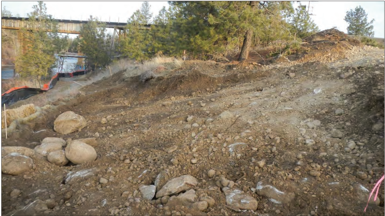
Figure 11. Overview of the Project Area on March 17, 2023. View to the northwest.
