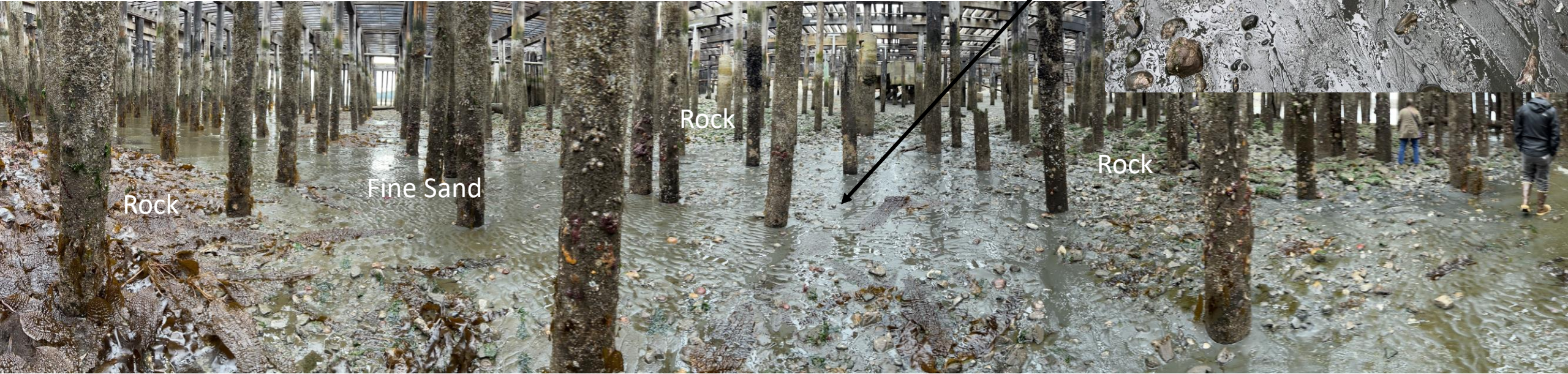
3 Fine Sand interior to coarse rock bands on the outer edges of the pier
