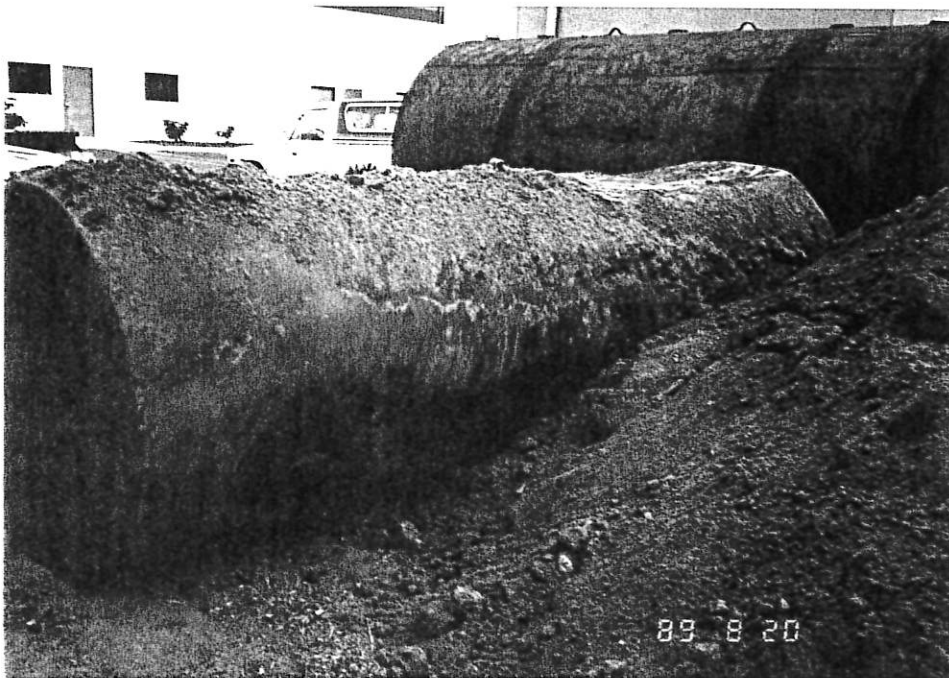
PHOTO NO. 6. Opposite side view of UST no. 10 after removal. The UST had no apparent leakage point, and the fuel dispensing line is suspected of leaking.
