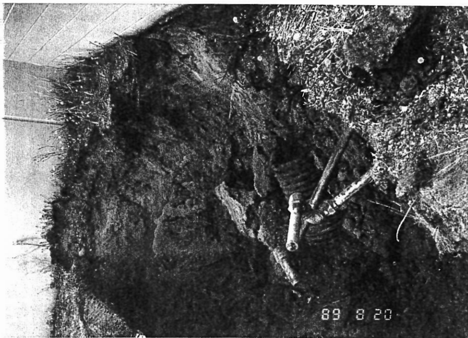
PHOTO NO. 2. Vertical view of the tank pit for UST no. 10. In the foreground, the venting and fuel dispensing pipes are visible. The product line is suspected of leaking.
