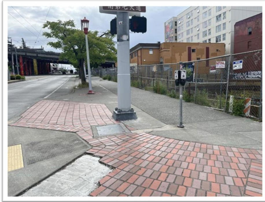
Photograph 1. Sidewalk Area North of 701/709 South Jackson Street Property (South Jackson Street Right-of-Way Area).
