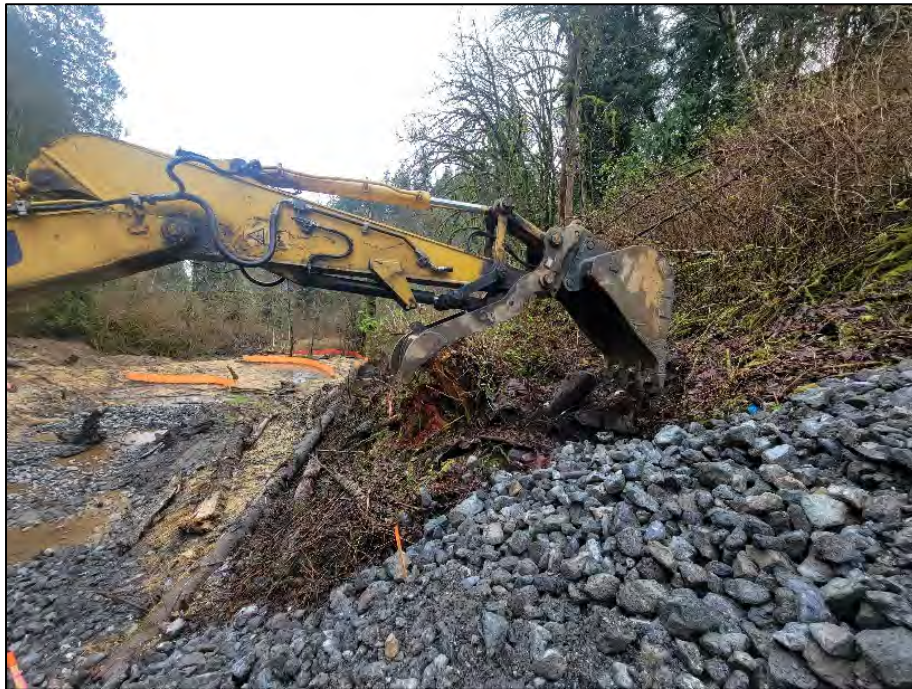
Photograph 12. Excavation of metal debris
