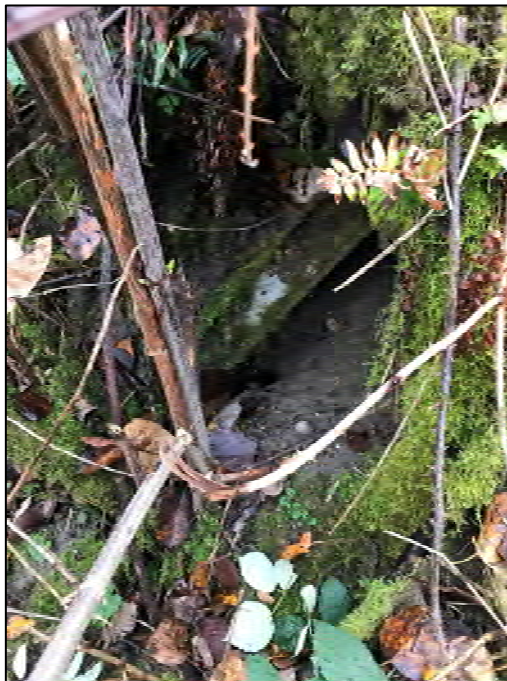
Photograph 6. Close-up of I-beam.
