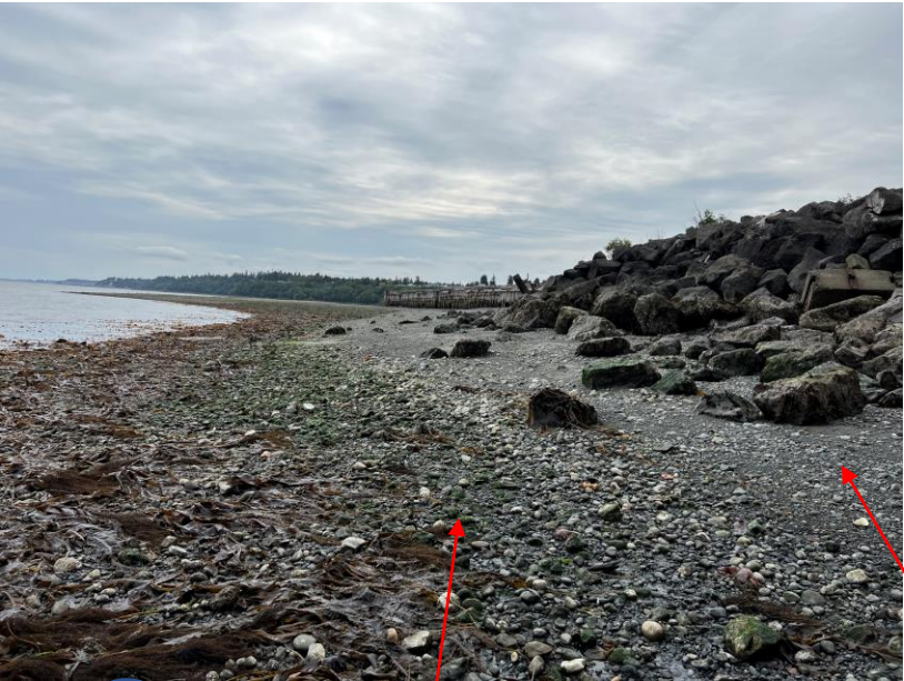
1 East Sandy Gravel Beach at toe of revetment
