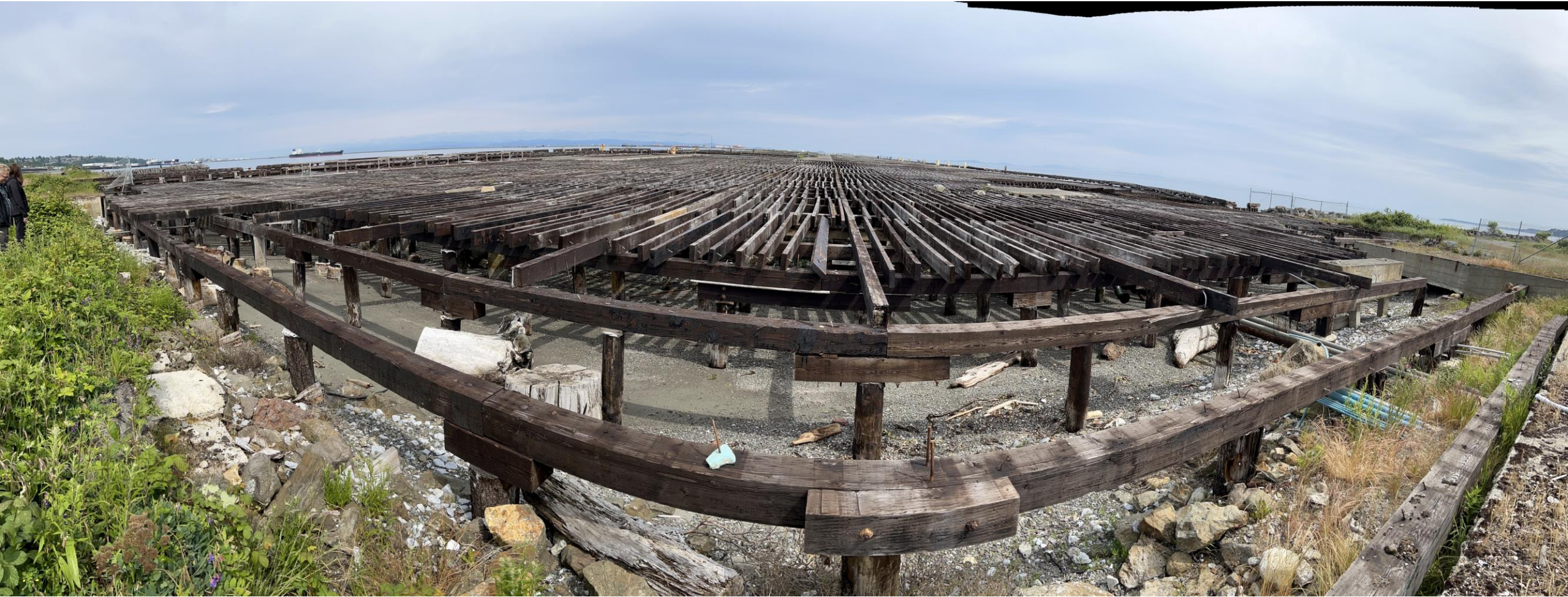
4 Upper Intertidal Beach Berm under pier (nearshore zone only) – gravelly sand
