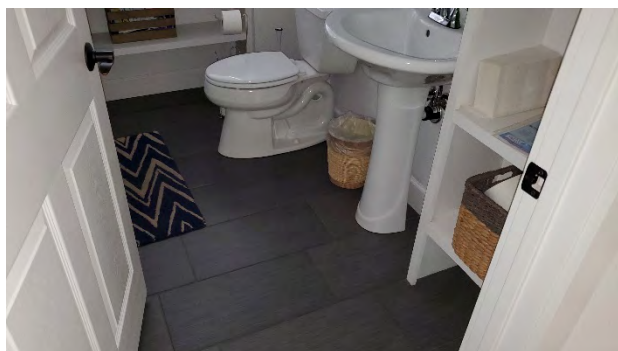
Ceramic floor tiles / mastic (restrooms)
