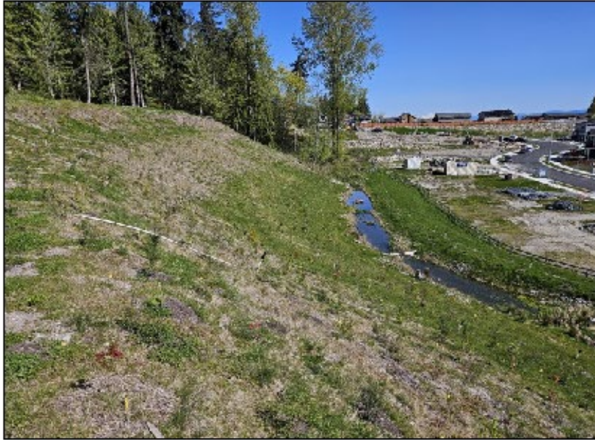
Photograph 4. West slope at about midslope. Facing north.
