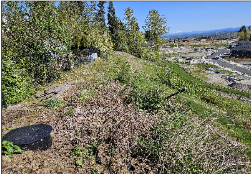
Photograph 6. Top of west slope (note yard waste in foreground). Facing north.
