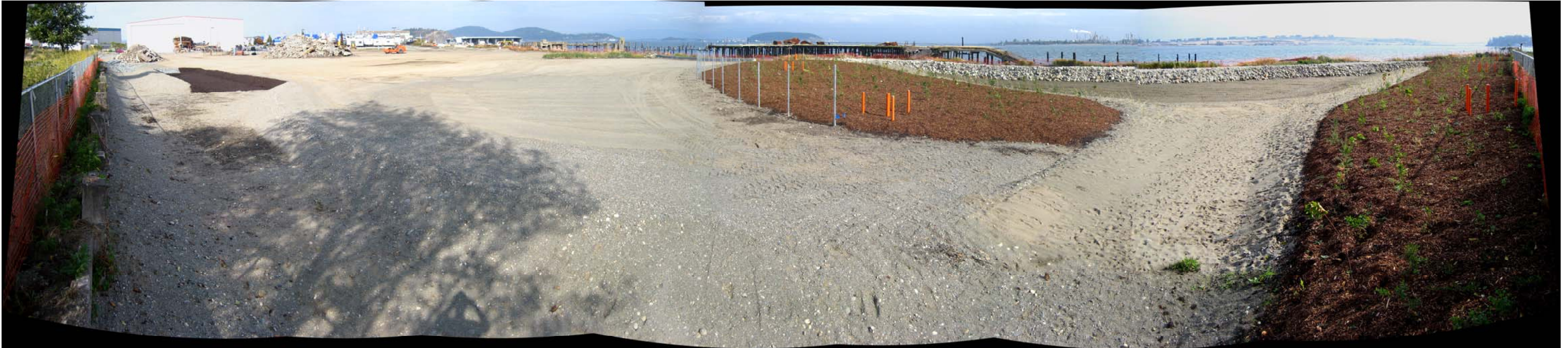
Photograph 43 – Stormwater swale, wetland mitigation, and buffer area construction progress on October 19, 2011.
