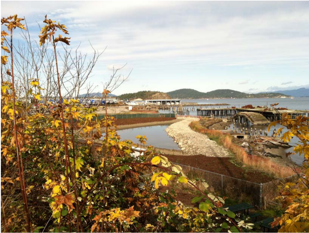
Photograph 31 – Completed wetland mitigation and buffer areas. Note temporary berm in place along OHW line (denoted by high-visibility fence) (November 14, 2011).
