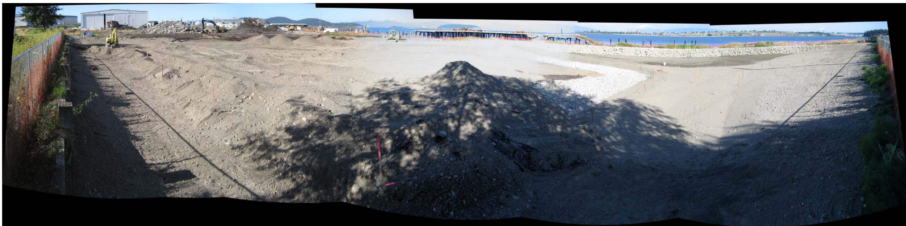
Photograph 35 – Stormwater swale, wetland mitigation, and buffer area construction progress on September 2, 2011.
