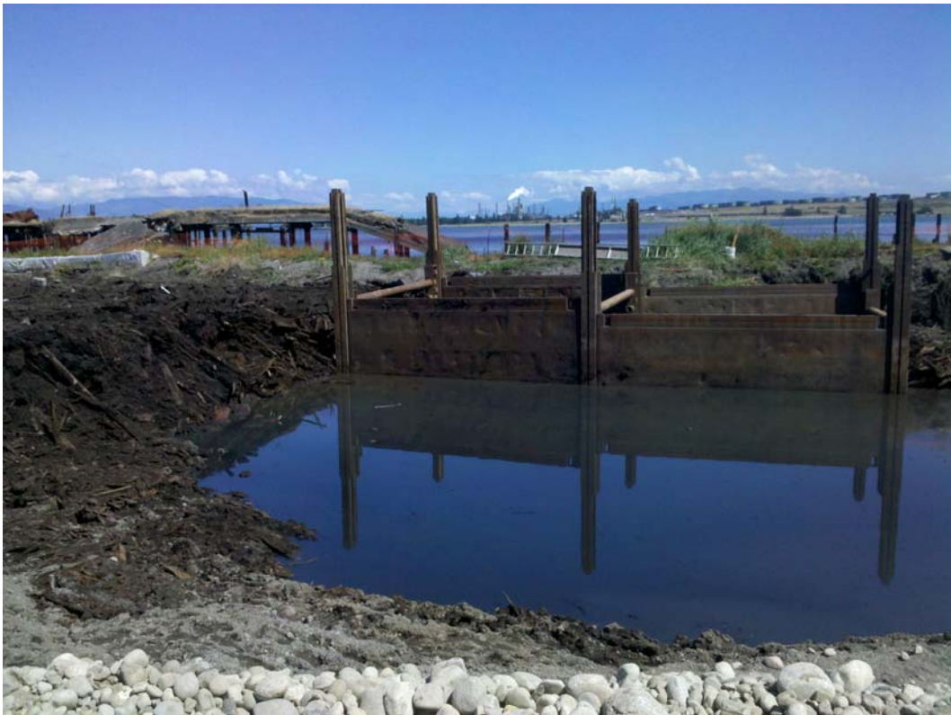
Photograph 10 – Slide rail shoring system (August 3, 2011).
