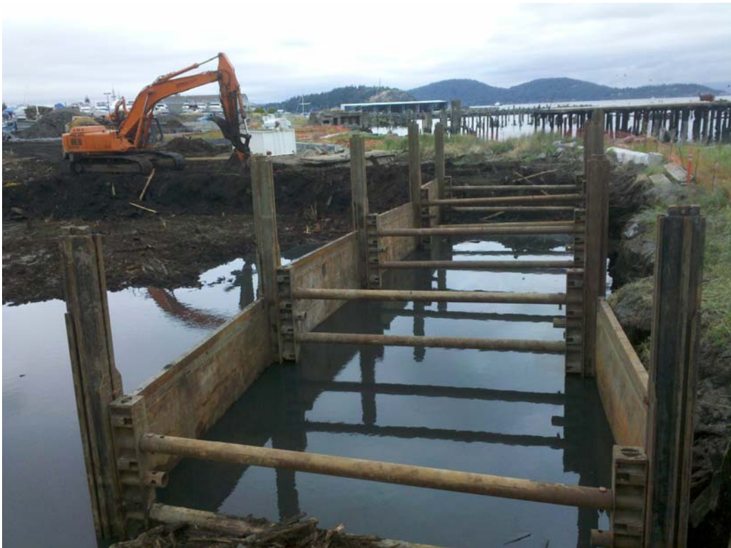
Photograph 12 – Slide rail shoring system. Orange fence marks the OHW line (August 5, 2011).
