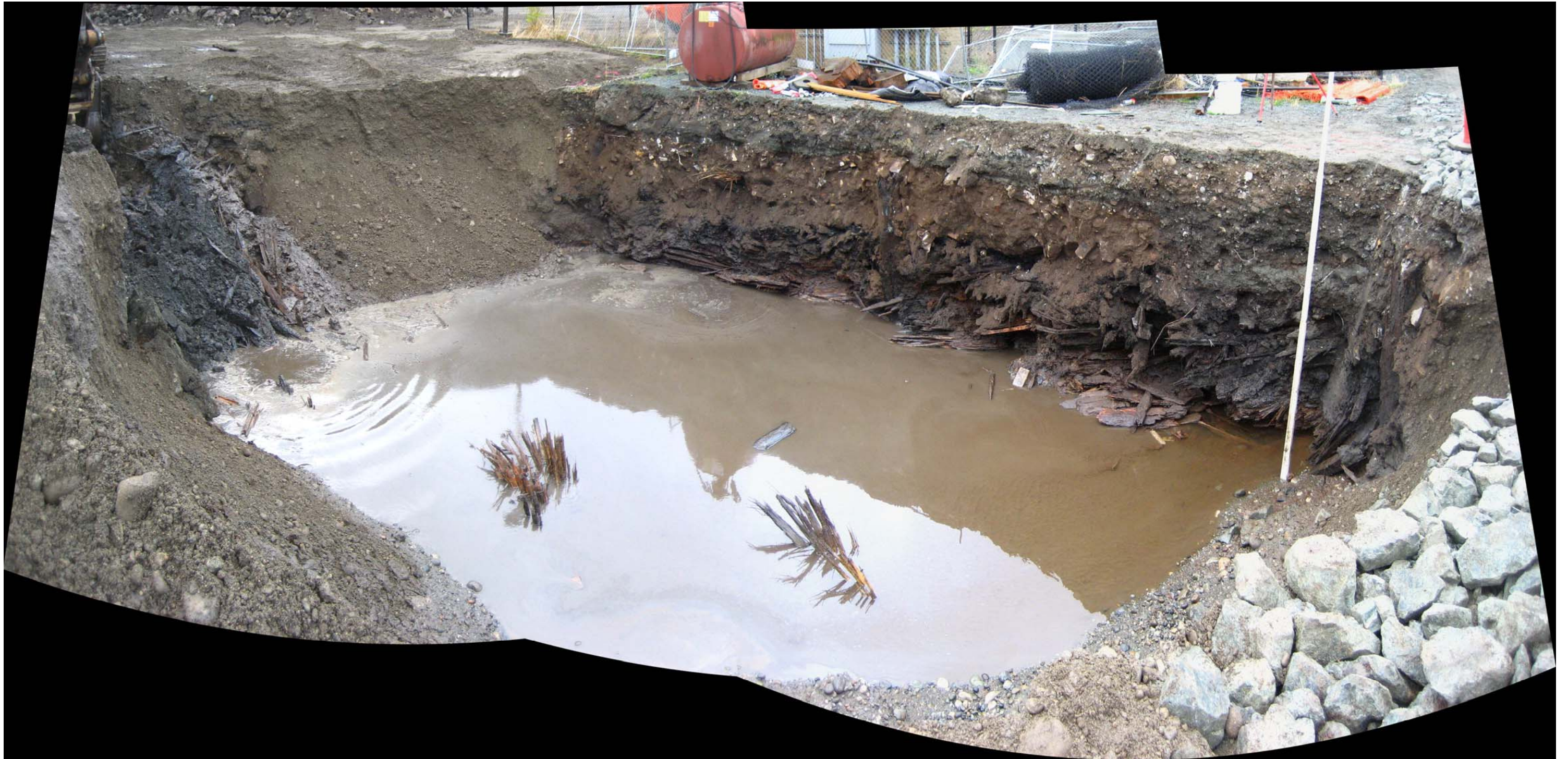
Photograph 48 – Example of stratigraphy observed during excavation. Note ponded groundwater and splintered piling remnants in excavation floor (GMX-S16 cell D and GMX-S43 cell J excavation areas, October 11, 2011).
