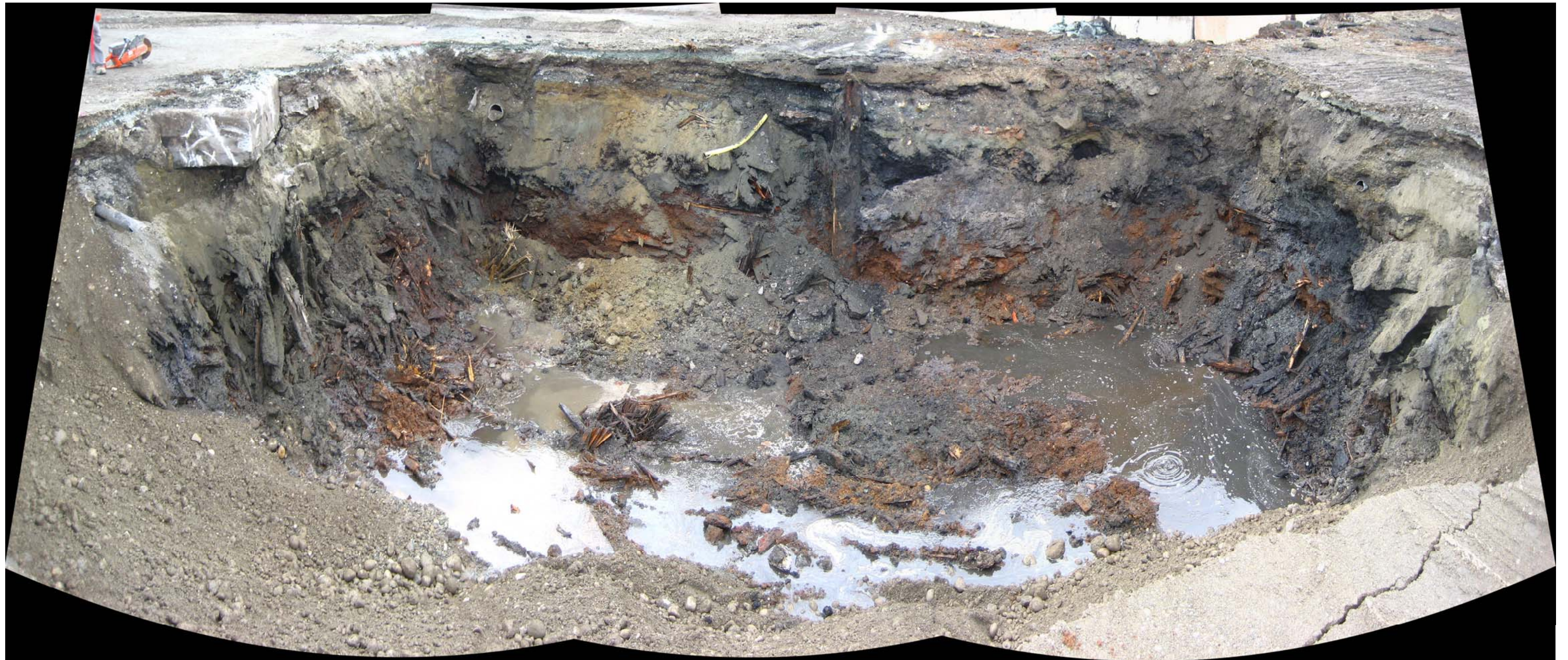
Photograph 49 – Example of stratigraphy and heterogeneity encountered during excavation (GMX-S43 cell K excavation area, October 11, 2011).
