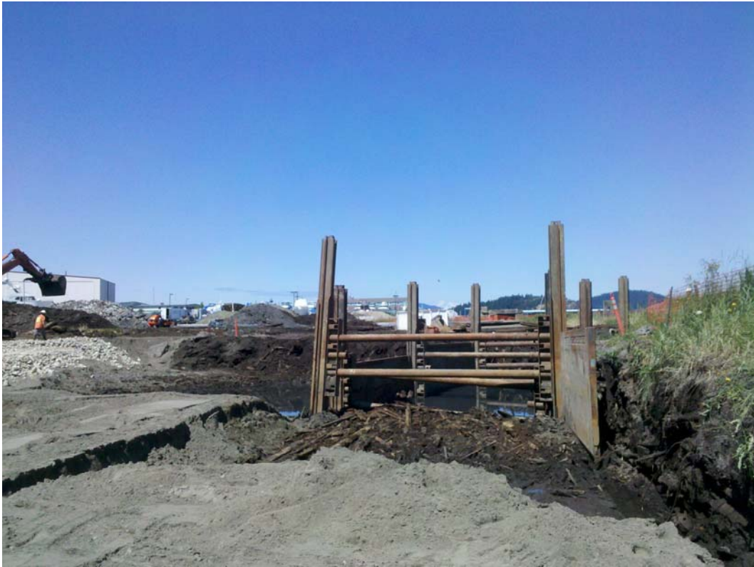
Photograph 9 – Slide rail shoring system. Orange fence marks the OHW line (August 3, 2011).
