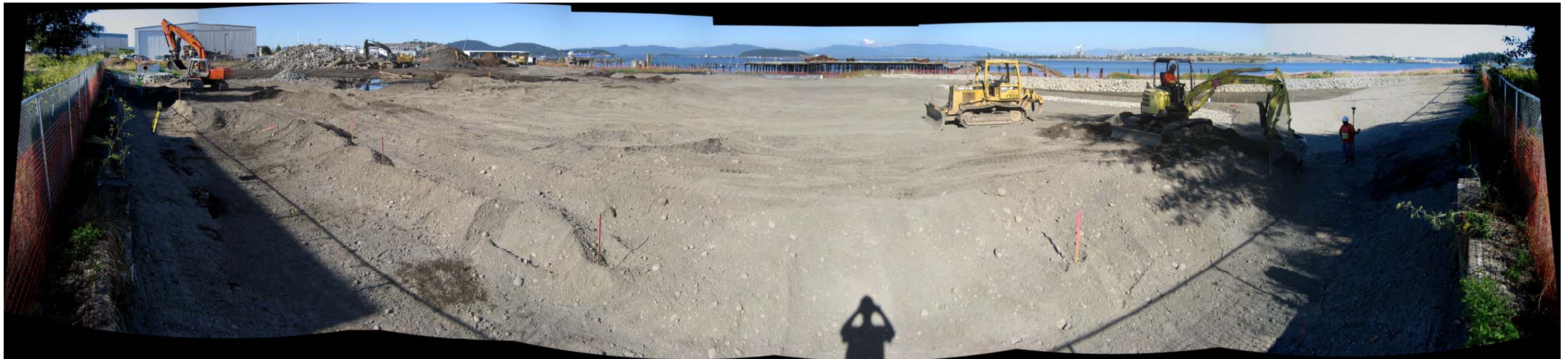
Photograph 36 – Stormwater swale, wetland mitigation, and buffer area construction progress on September 6, 2011.
