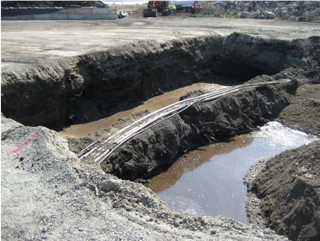
Photograph 7 – Extent of excavation limited by electrical conduit (GMX-MW-03 excavation area, September 8, 2011).
