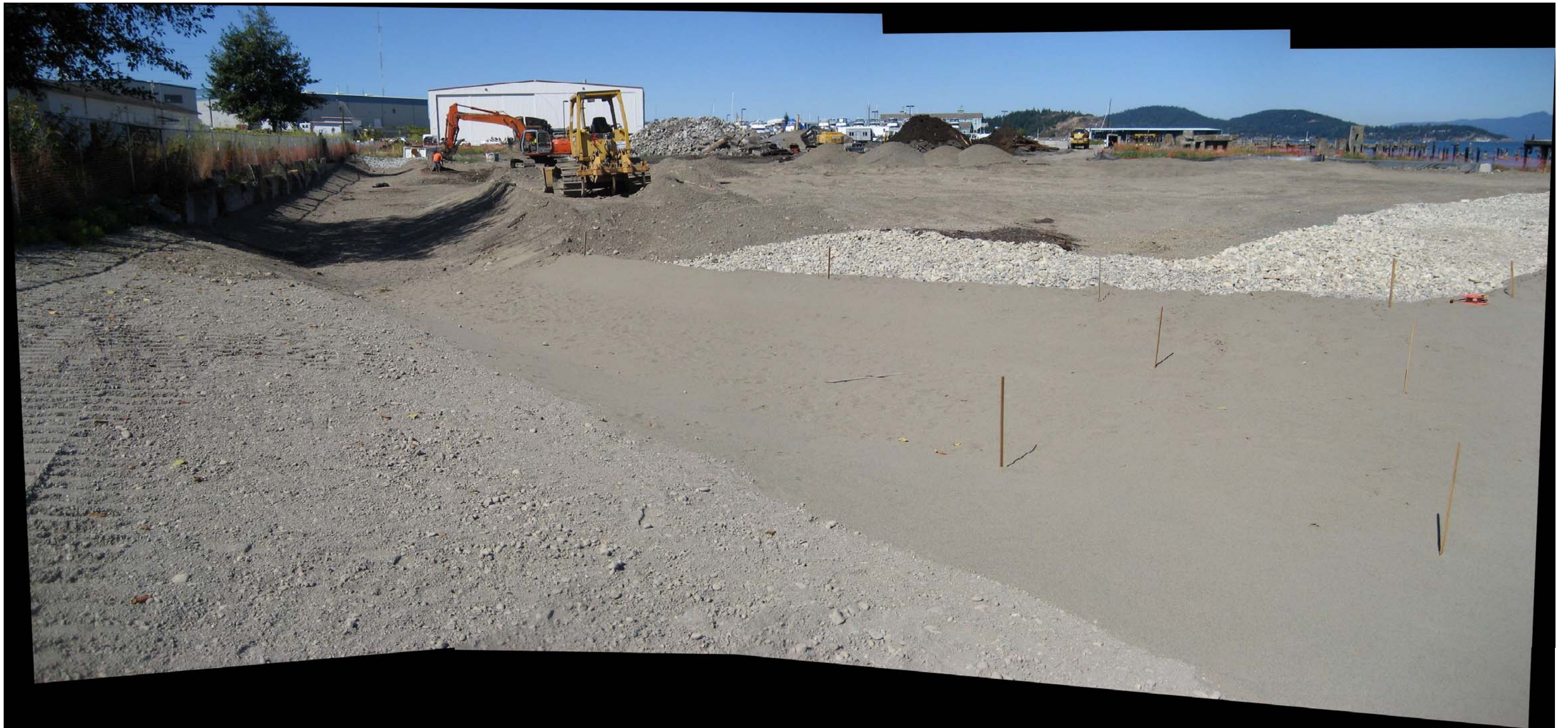
Photograph 46 – Construction of stormwater swale conveyance channel into wetland mitigation area (September 7, 2011).
