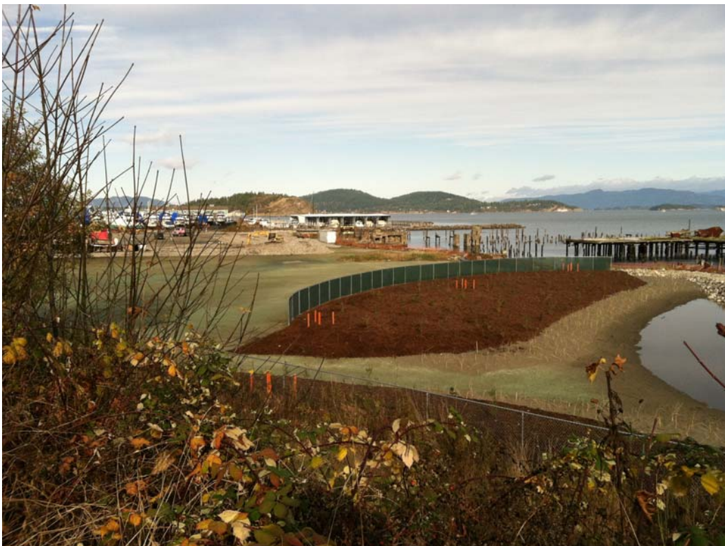
Photograph 30 – Completed wetland mitigation and buffer areas (November 14, 2011).
