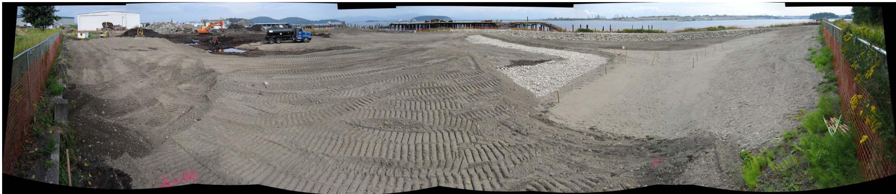
Photograph 34 – Stormwater swale, wetland mitigation, and buffer area construction progress on September 1, 2011.
