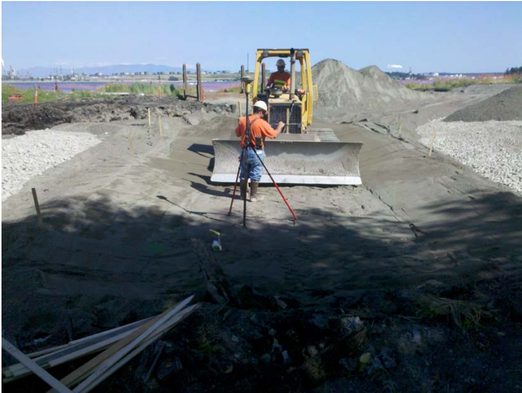
Photograph 21 – Grading beach sand in wetland mitigation area (July 28, 2011).
