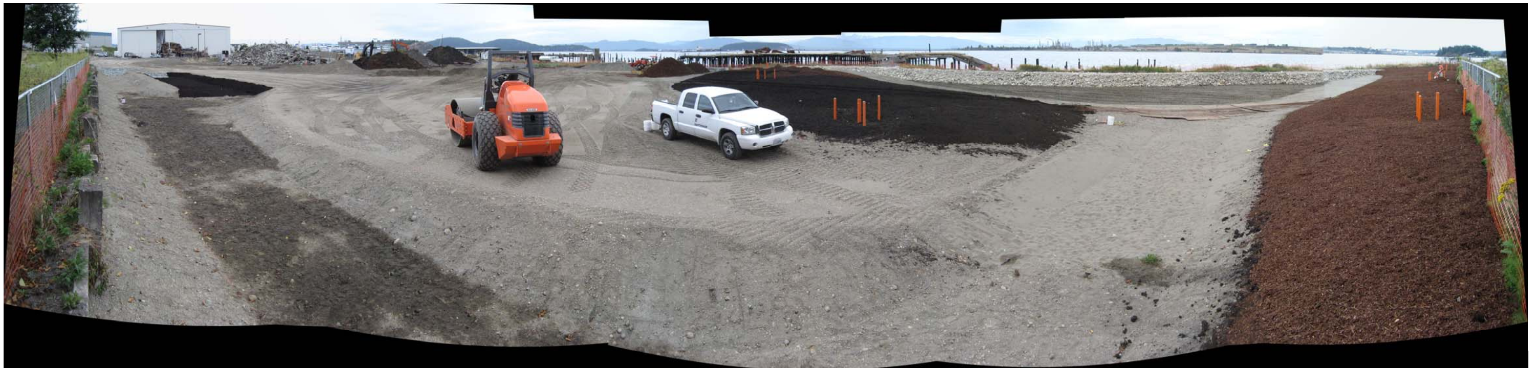
Photograph 41 – Stormwater swale, wetland mitigation, and buffer area construction progress on September 21, 2011.
