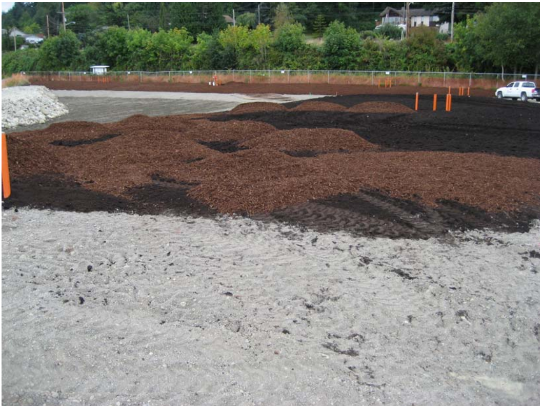
Photograph 26 – Mulch piles to be spread over compost-amended buffer planting area (September 21, 2011).
