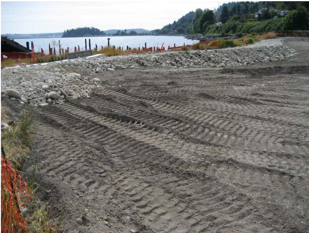
Photograph 22 – Temporary protective berm installed in wetland mitigation area (September 1, 2011).
