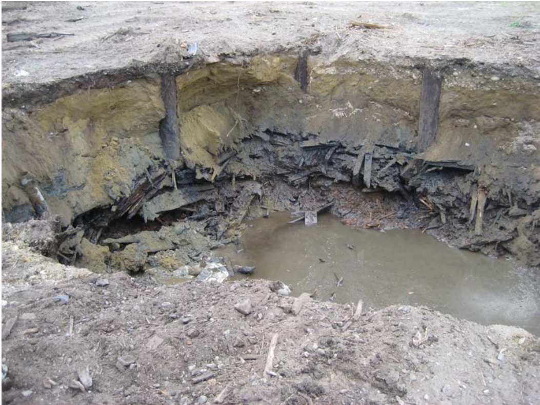
Photograph 4 – Example of soil and wood waste stratigraphy. Note upright pilings in excavation walls (GMX-S41 excavation area, September 15, 2011).
