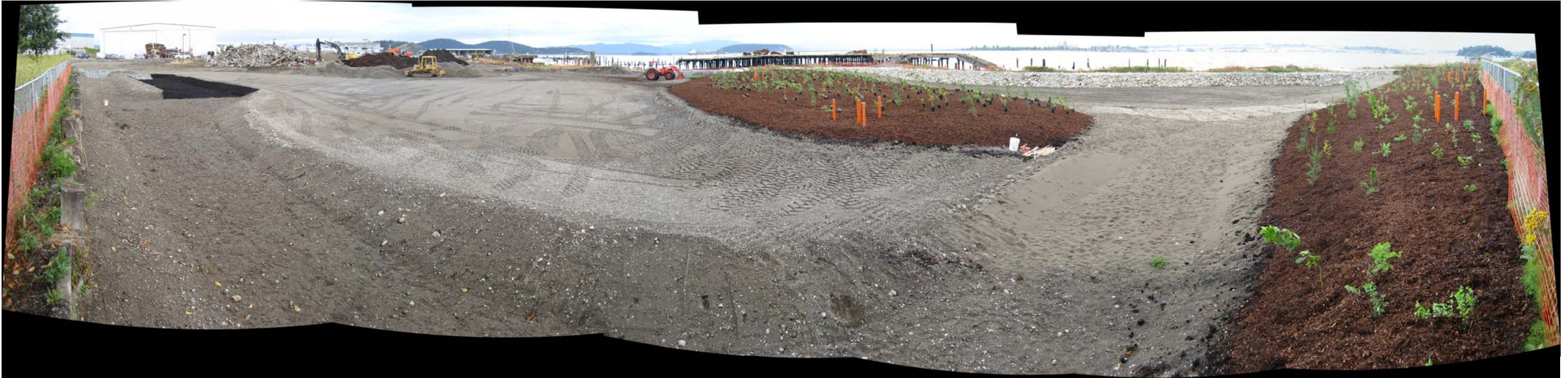
Photograph 42 – Stormwater swale, wetland mitigation, and buffer area construction progress on September 22, 2011.
