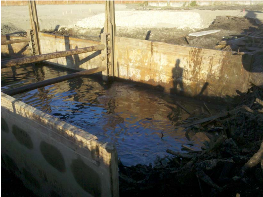
Photograph 11 – Slide rail shoring system (August 4, 2011).
