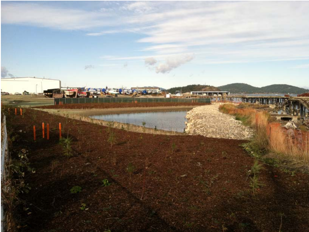
Photograph 33 – Completed wetland mitigation and buffer areas (November 14, 2011).
