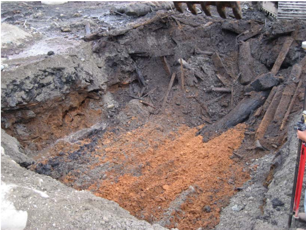
Photograph 2 – Lower fill unit consisting of fine-grained sawdust exposed in floor of excavation (GMX-S49 excavation area, September 14, 2011).
