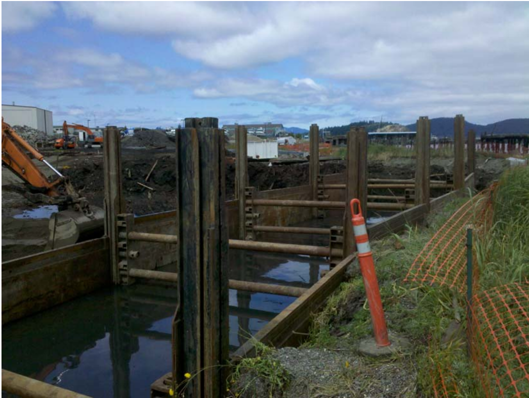
Photograph 13 – Slide rail shoring system. Orange fence marks the OHW line (August 5, 2011).
