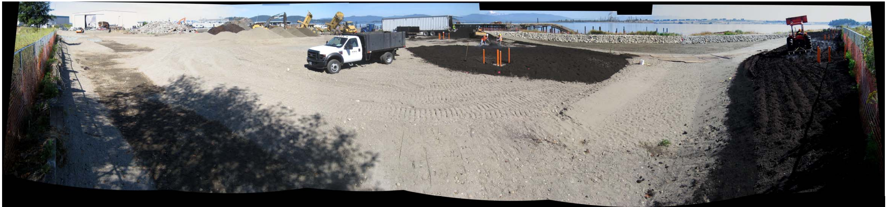
Photograph 40 – Stormwater swale, wetland mitigation, and buffer area construction progress on September 20, 2011.
