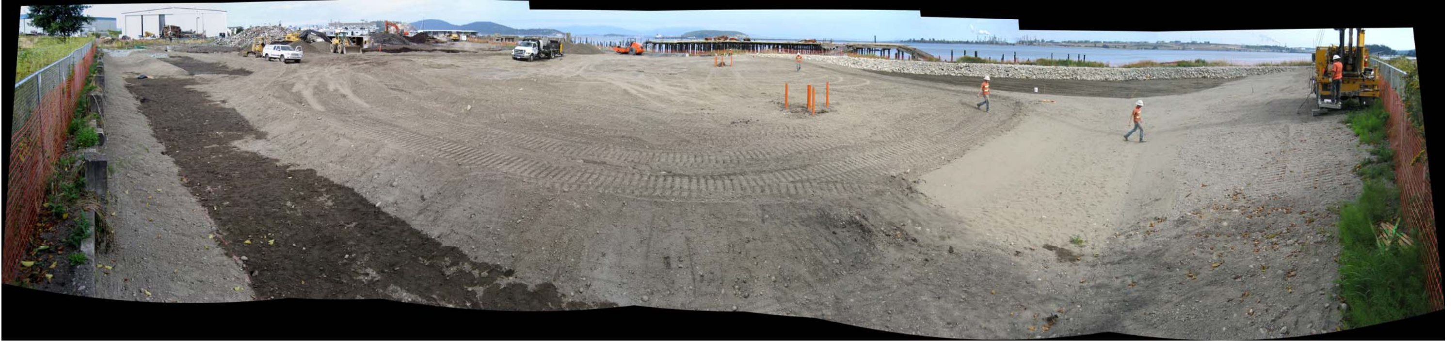
Photograph 39 – Stormwater swale, wetland mitigation, and buffer area construction progress on September 12, 2011.
