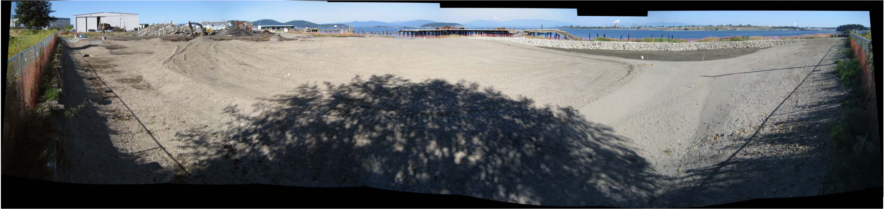
Photograph 38 – Stormwater swale, wetland mitigation, and buffer area construction progress on September 9, 2011.
