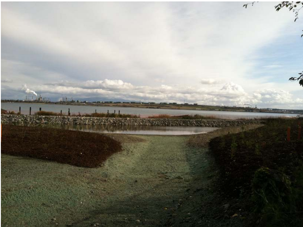
Photograph 32 – Completed stormwater swale conveyance into wetland mitigation area (November 14, 2011).
