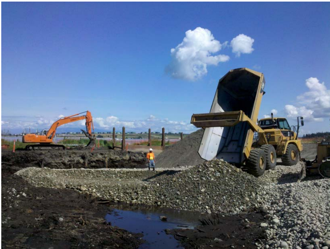
Photograph 18 – Placement of shoreline protection layer material (July 27, 2011).
