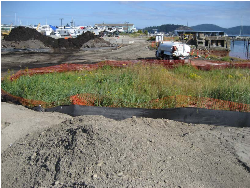
Photograph 16 – Silt fence and high-visibility barrier installed along Wetland E boundary (September 2, 2011).
