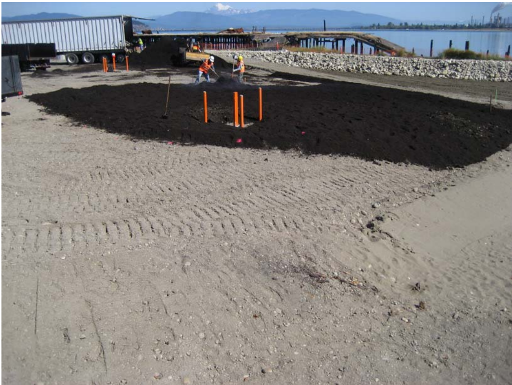
Photograph 24 – Delivery and placement of compost in wetland buffer planting area (September 20, 2011).
