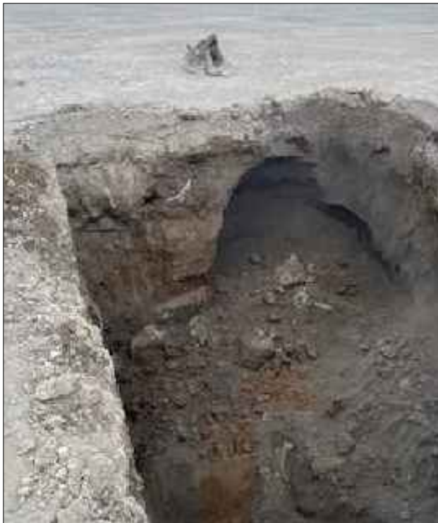
PHOTO 2 Excavation near MW07 - contact of original soil vs. dredge sand fill from 2014 remedial excavation.
