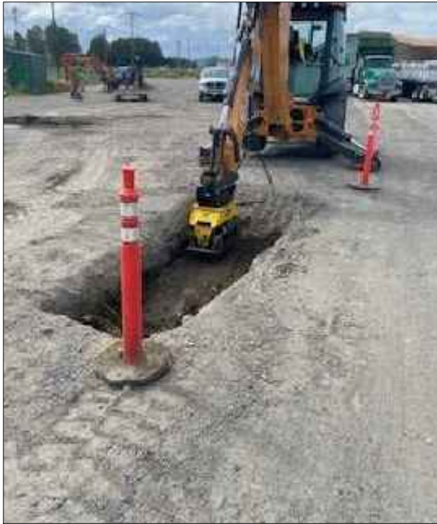
PHOTO 5 Backfill and Compaction.
