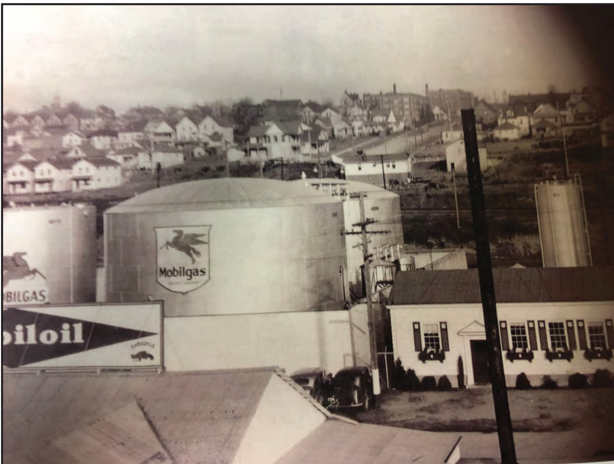
Figure 8. Undated photograph showing gasoline infrastructure after General Petroleum Corporation was rebranded to Mobilgas. The office building on the site is at the right. (Washington Department of Ecology 2014:65)
