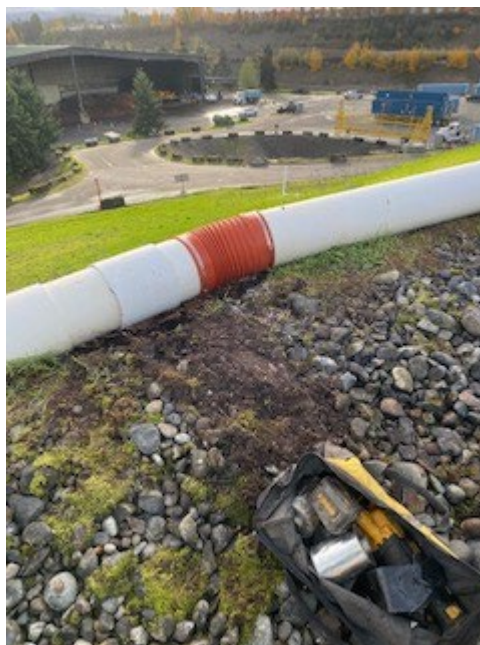
10-inch Header After Repair
