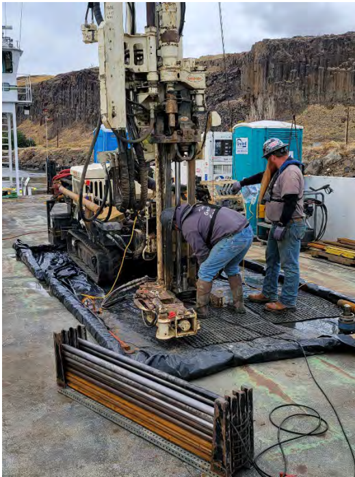
Photograph 3: Drill Rig Set Up with Wipers Date taken: 11/01/2022
