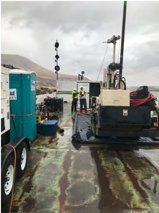
Photograph 7: Alternate Angle of Drill Rig Set Up Date taken: 11/01/2022
