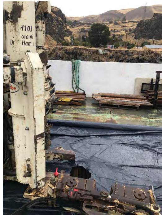
Photograph 8: Drill Rig and Tooling Date taken: 11/01/2022
