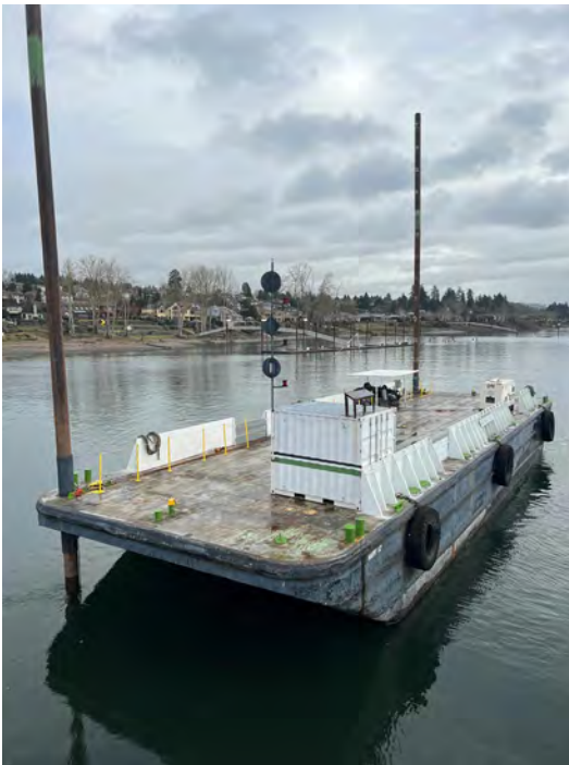
Photograph 1: Barge Setup Before Loading Equipment
