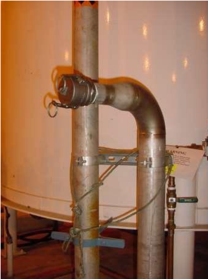
Figure 25. Tank 104 overflow end cap AOD-2.
