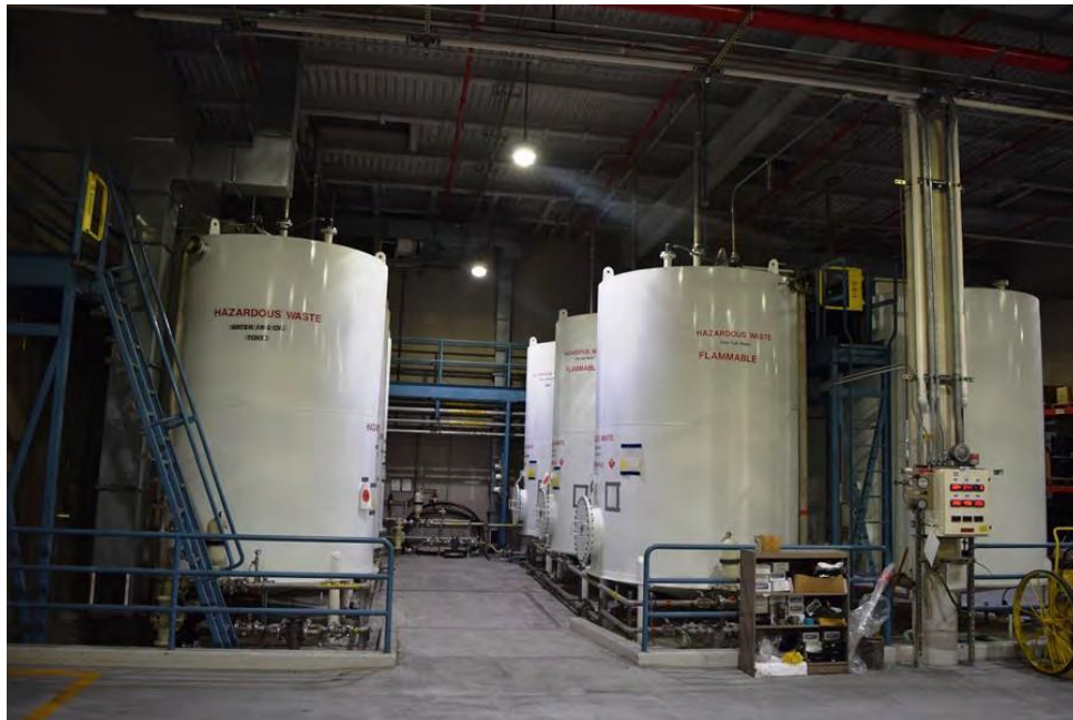
Photo 14: Tank Storage Area (Rm 124), December 2017
