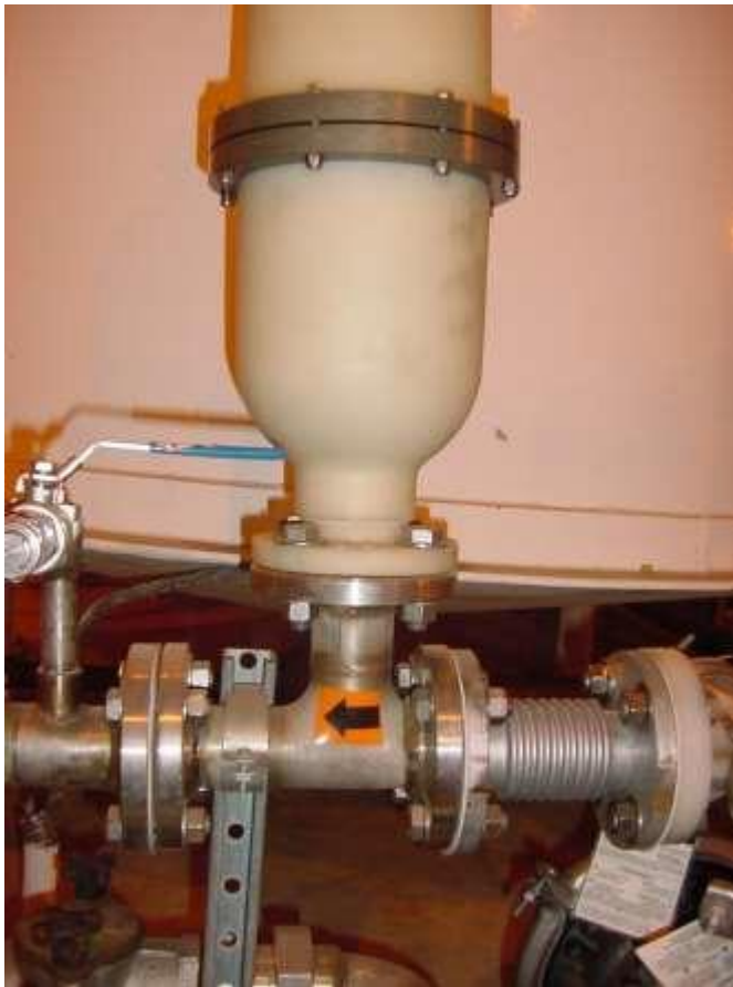
Figure 57. Recirculation fill pipe sampling port valve ARV-5, sample port ARD-3, pressure gage valve ARV-6, and pressure gauge ARF-7.
