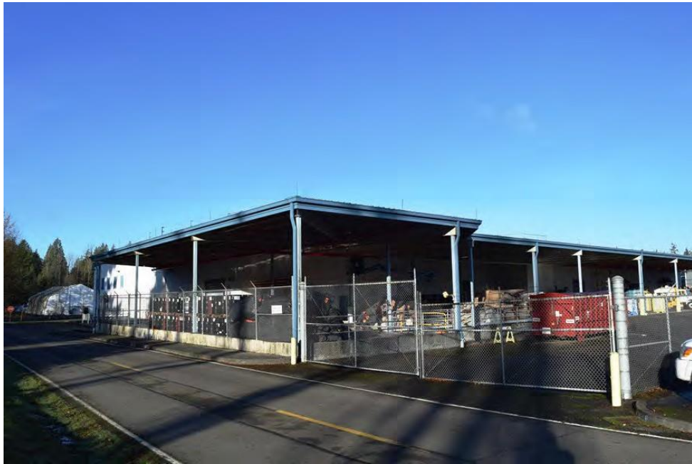
Photo 5: SE Corner, December 2017
