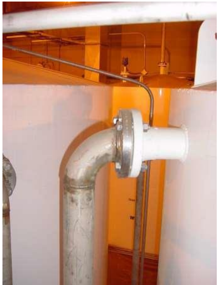
Figure 10. Tank 105 overflow pipe flange AOF-5.
