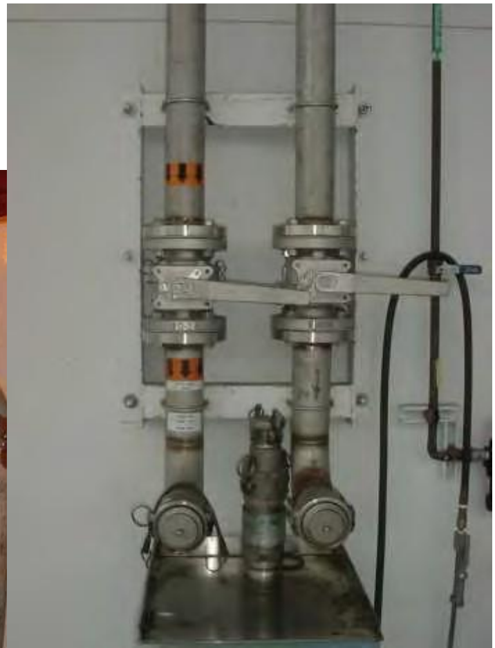
Figure 2. Outside waste tank drain pipe rack valve AOV-10 and end cap AOD-8.
