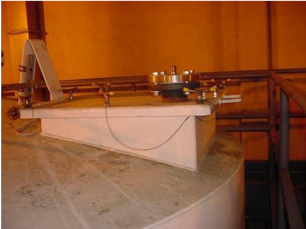
Figure 19. Tank 106 upper access hatch cover CIF-6. Test underside of entire hatch perimeter.
