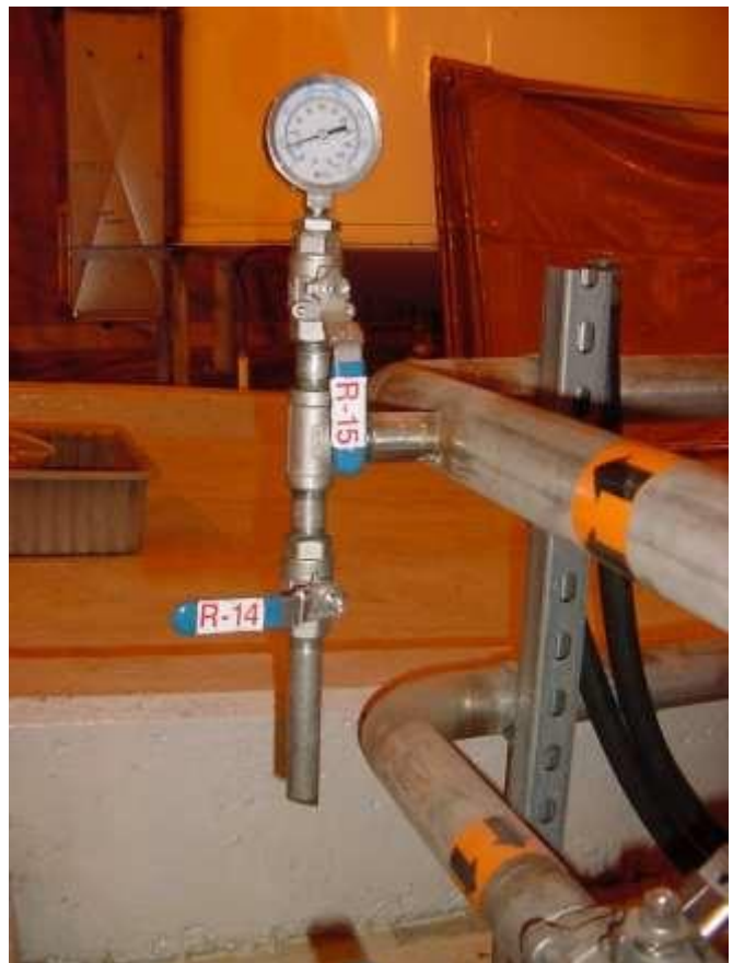
Figure 57. Recirculation fill pipe sampling port valve ARV-5, sample port ARD-3, pressure gage valve ARV-6, and pressure gauge ARF-7.
