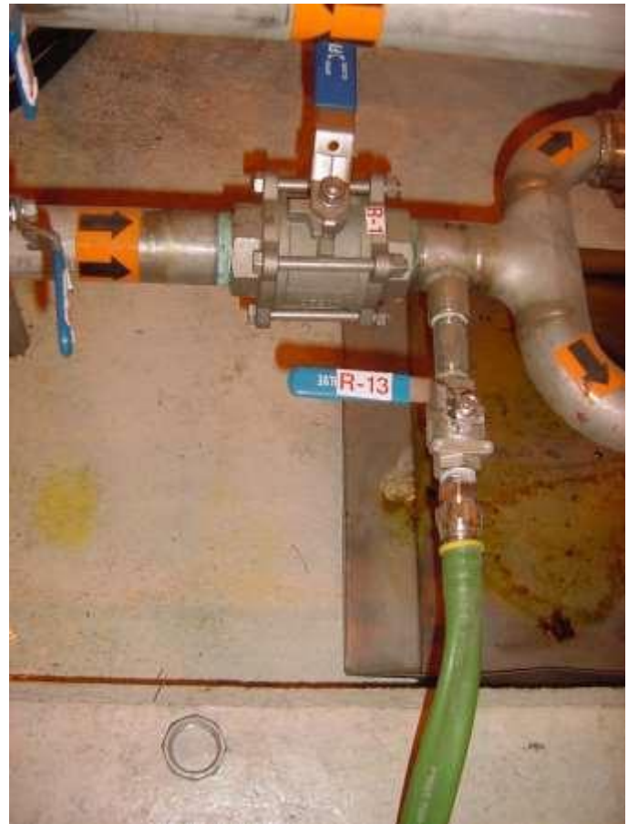
Figure 48. Recirculation drain valves ARV-1, sample port valve ARV-2 and drain sample port ARD-1.
