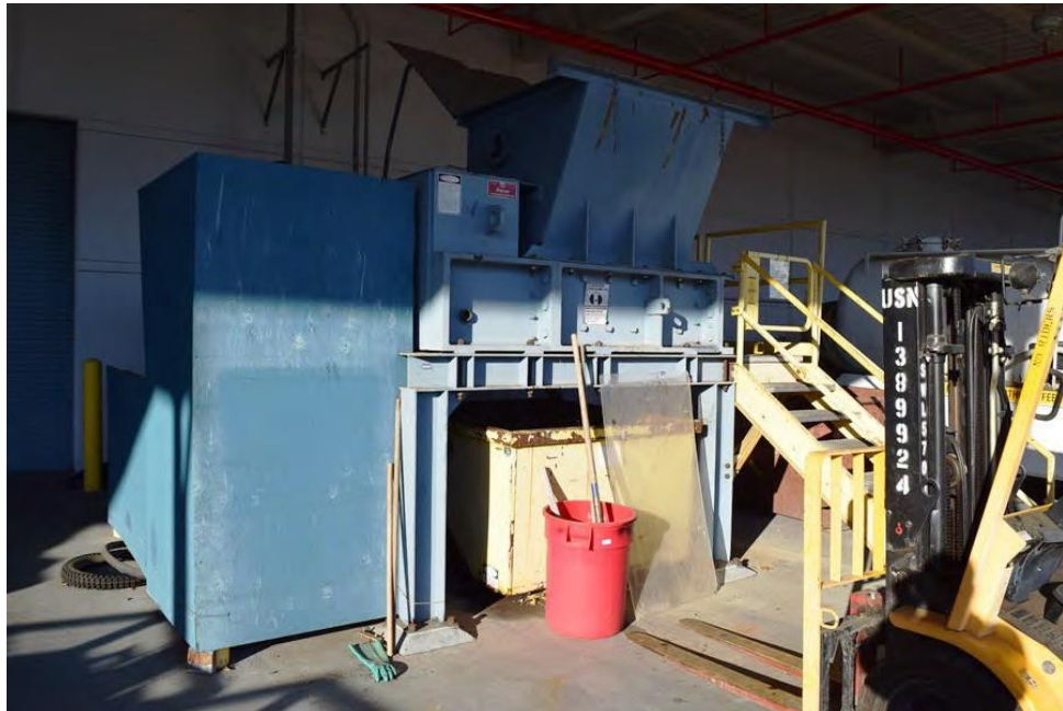
Photo 8: Drum Shredder, December 2017
