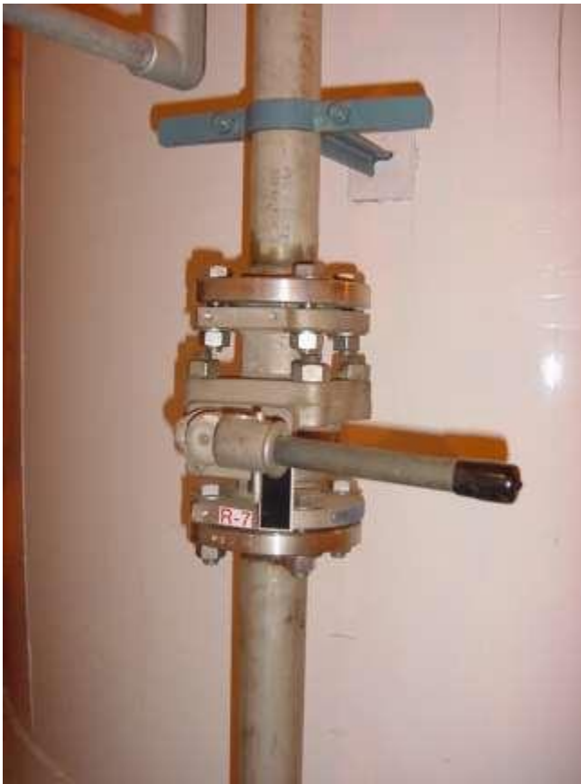
Figure 59. Tank 104 recirculation fill pipe flange ARF-8.
