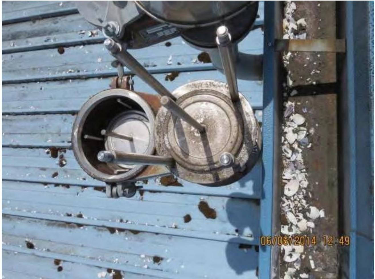
Figure 3. The pressure vent (right side in picture) cover and screen have been removed by detaching 4 wing nuts from the top. The suction vent (left side in picture) cover has been removed by releasing the hold-down wing nuts on both sides.
