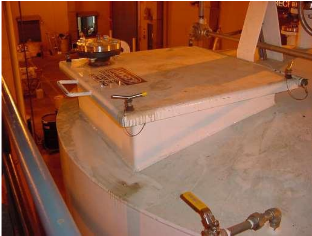
Figure 7. Tank 104 upper access hatch cover AIF-1. Test underside of entire hatch perimeter.
