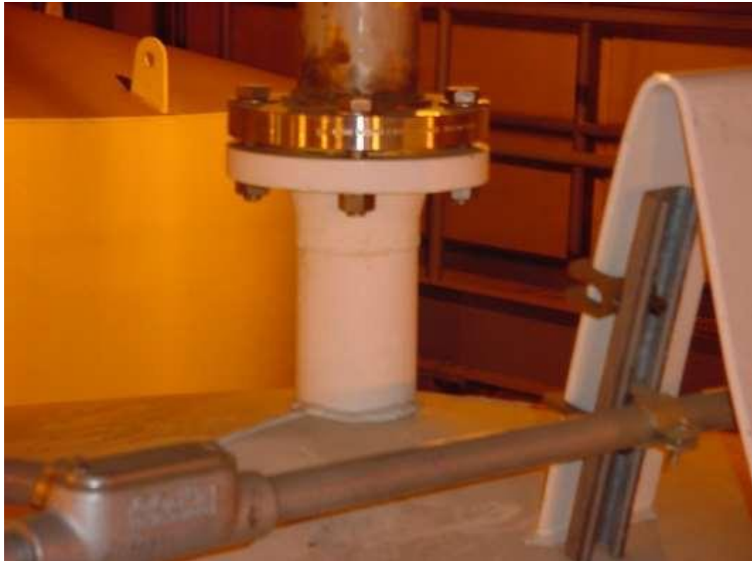
Figure 11. Tank 105 vent flange AOF-4. Test perimeter of vent flange.
