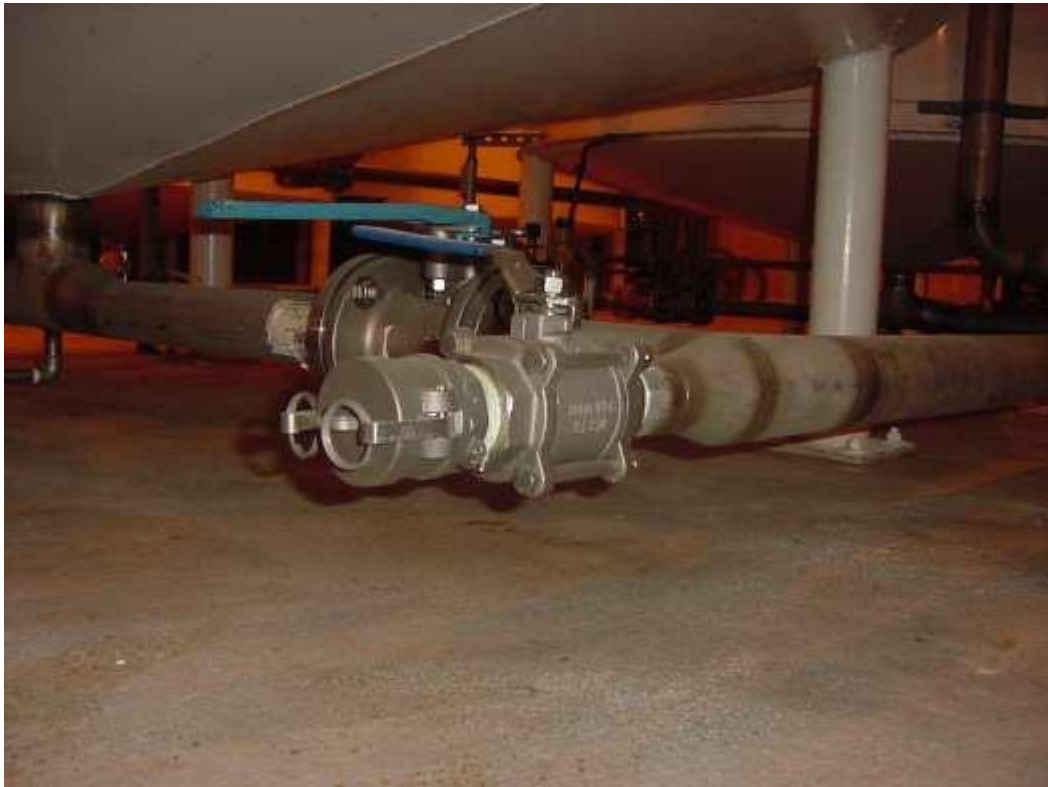
Figure 21. Main drain pipe valve AOV-1 and end cap AOD-1. Test perimeter of cap, perimeter of flanges at either end of valve, valve stem seal, and perimeter of end cap.
