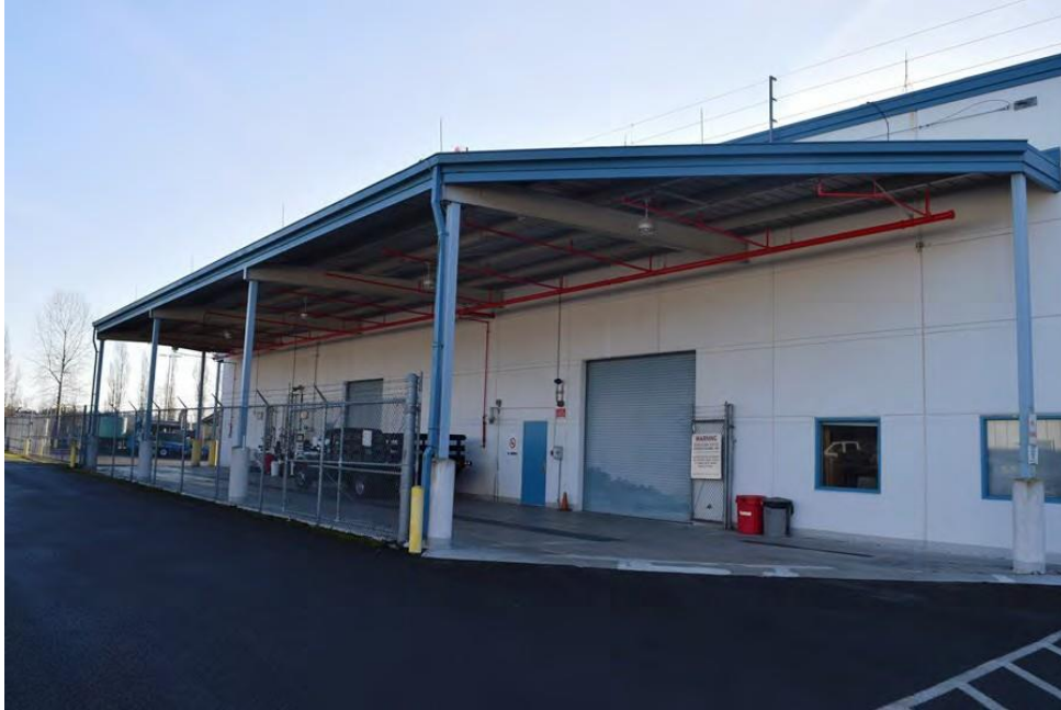
Photo 1: North Loading Area, December 2017
