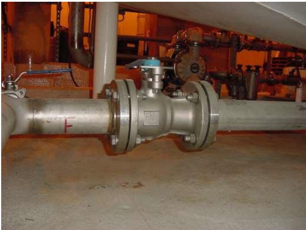
Figure 22. Tank 104 drain valve AOD-2. Test perimeter of flanges at either end of valve and valve stem seal.
