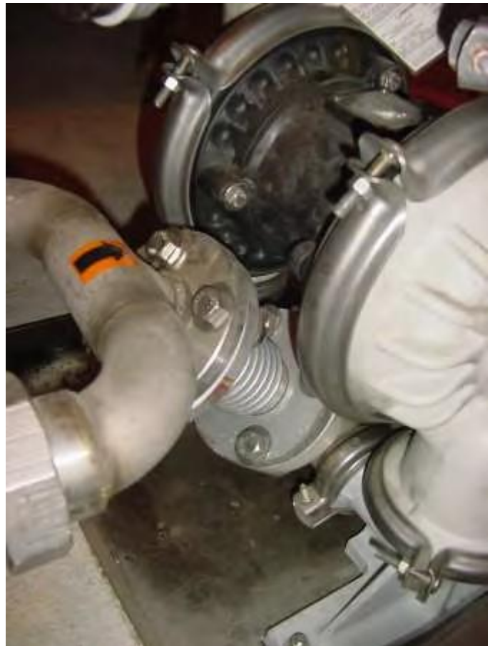
Figure 52. Recirculation drainpipe flex fitting ARF-3.
