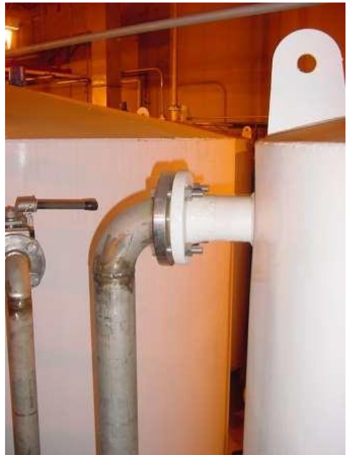
Figure 16. Tank 106 overflow pipe flange COF-5.
