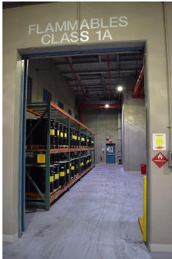
Photo 23: Flammables Class 1A (Rm 136), December 2017
