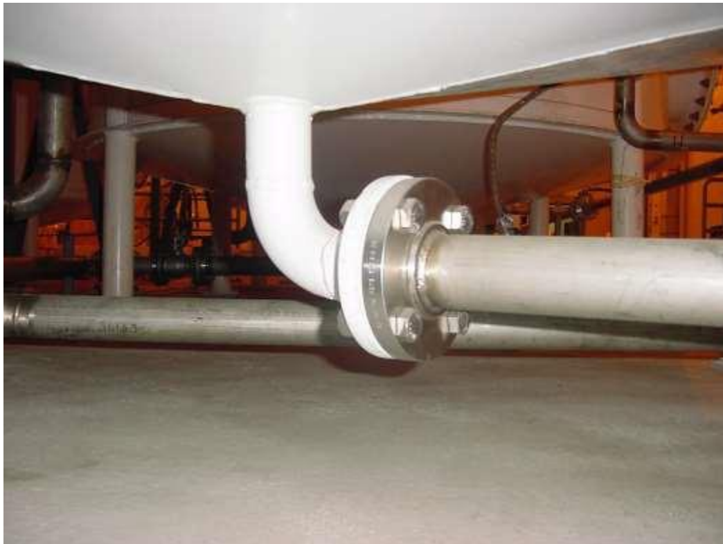
Figure 38. Tank 106 drain pipe flange (to be deleted in upgrade). Test perimeter of flange.
