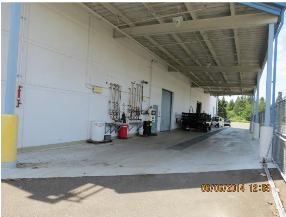
Picture 2: the north spill containment area viewed from the northeast.
