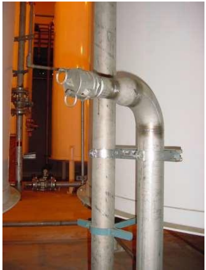
Figure 26. Tank 105 overflow end cap AOD-5.
