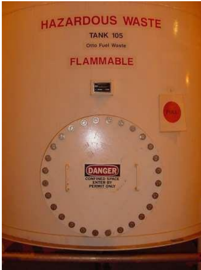
Figure 35. Tank 105 bottom access cover AOF-6.
