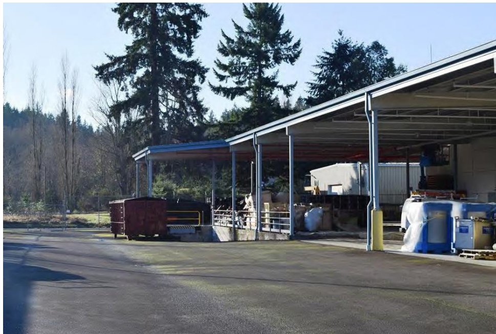
Photo 6: SE Storage Area, December 2017
