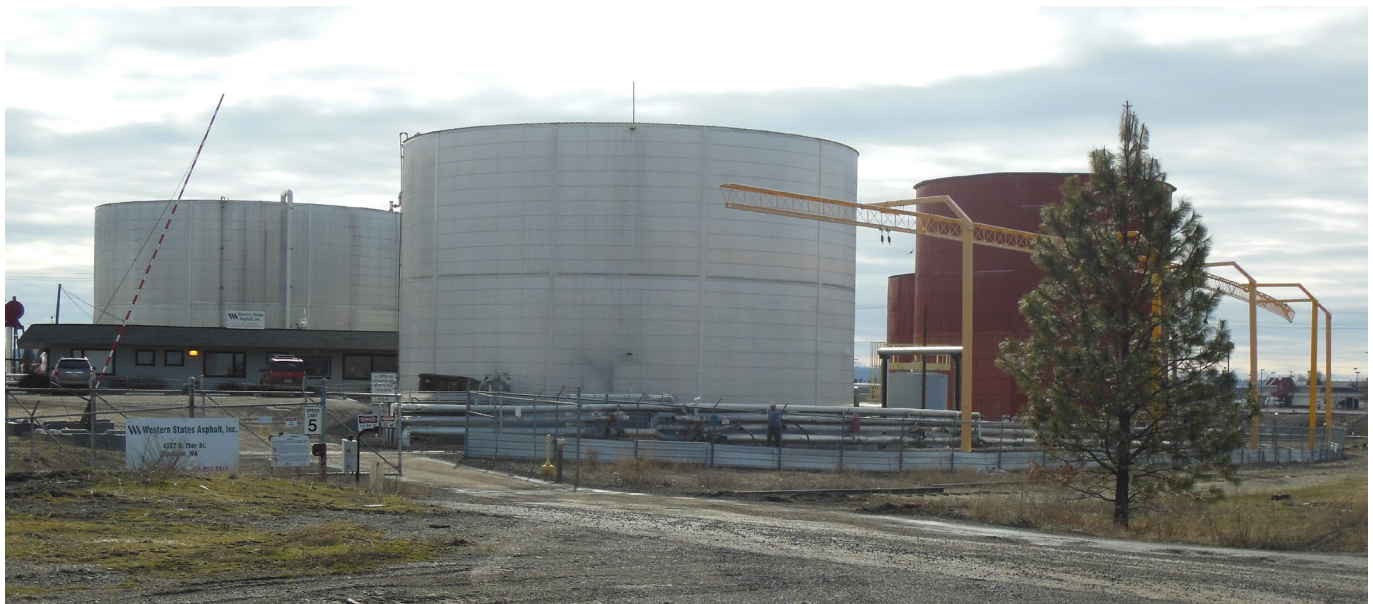
Figure 2. The western edge of the site in 2013.
