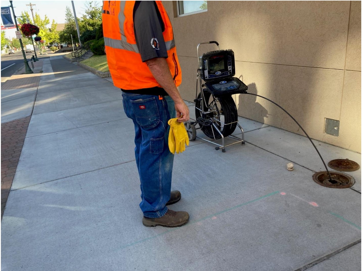
Picture 2: Video inspection of cleanout located in sidewalk on 2 nd Avenue
