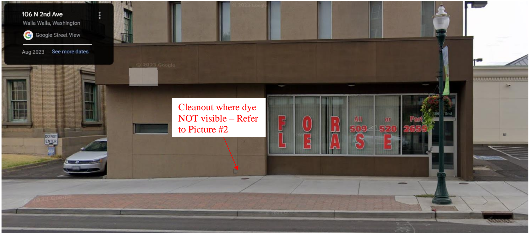
Figure 2: Street view of 106 N. 2 nd Avenue building showing the cleanout where the video inspection was performed (Source: Google Maps)
