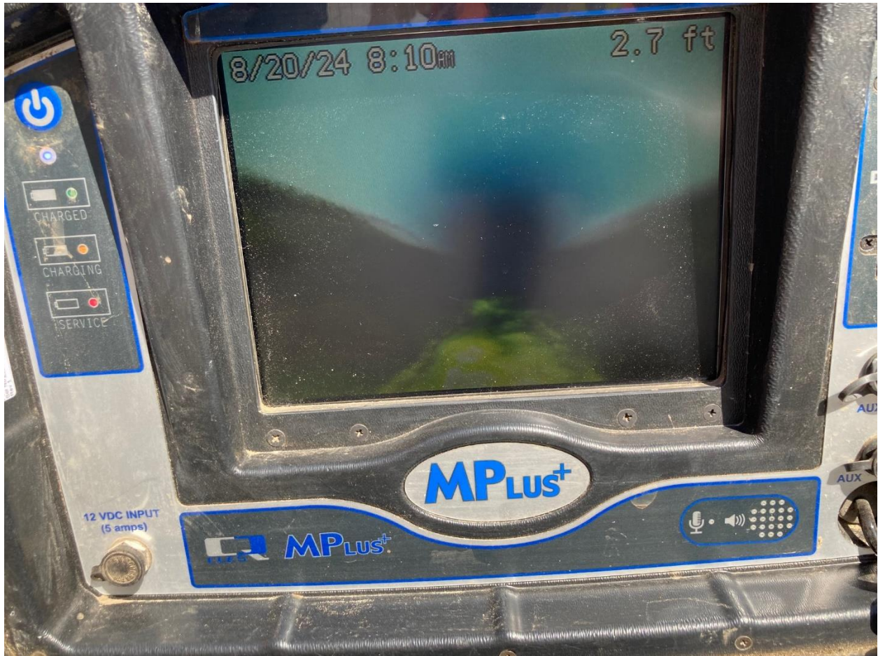
Picture 7: Screen of video inspection of cleanout in sidewalk on Rose Street. Dyed water (green) visible
