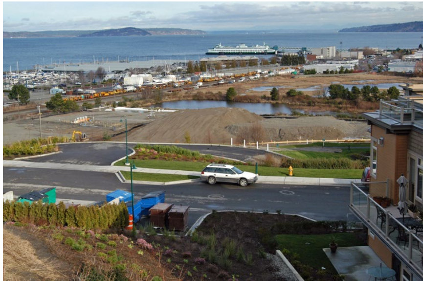
Figure 4: View of cleanup Site from upper area
