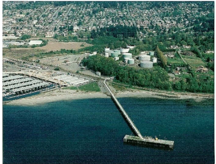
Historic view of fuel terminal
