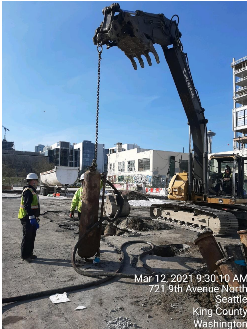
Photograph 22: ECI vacuums oil from Hoist-6 cylinder.
