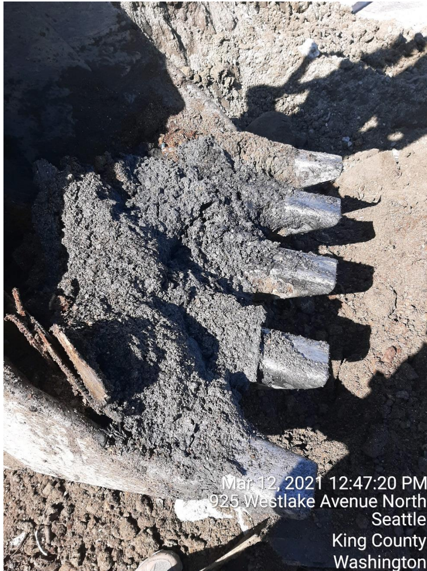
Photograph 9: Below left. Soil from UST-A below tank location, at a depth of 15 feet bgs.
