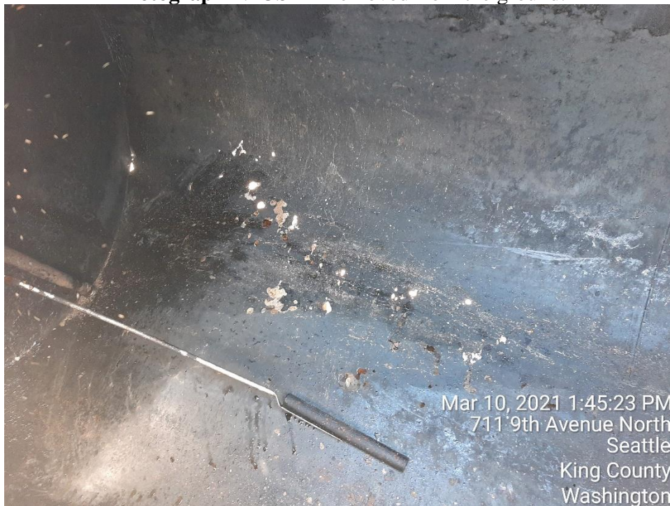
Photograph 8: Holes in the bottom of UST-A.
