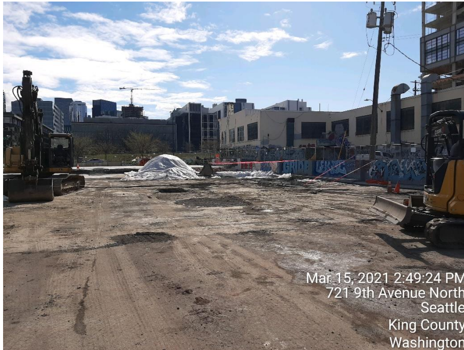
Photograph 24: Western hoists lined, backfilled, and compacted.
