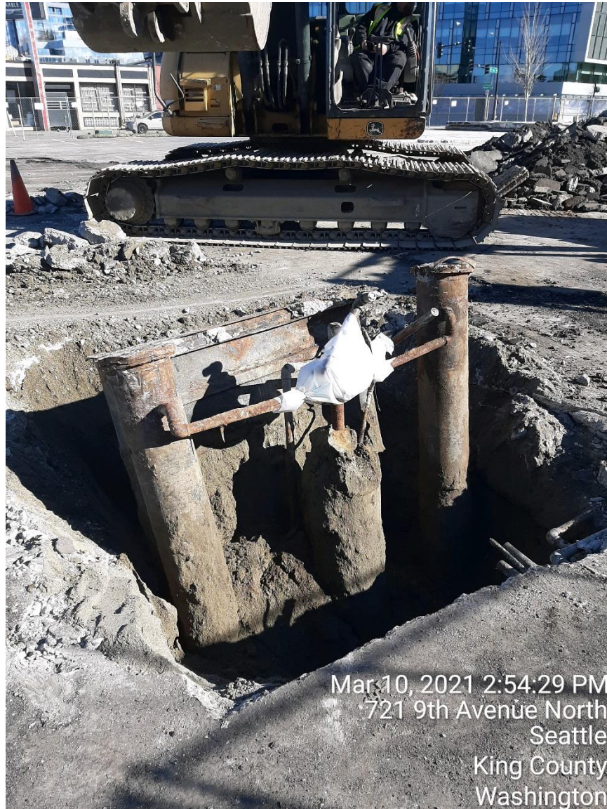
Photograph 18: Above right. Hoist-5 being pulled from the ground.
