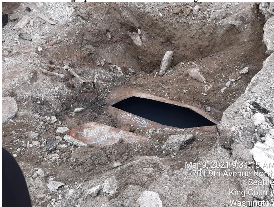
Photograph 6: UST-A cut open for tank cleaning.
