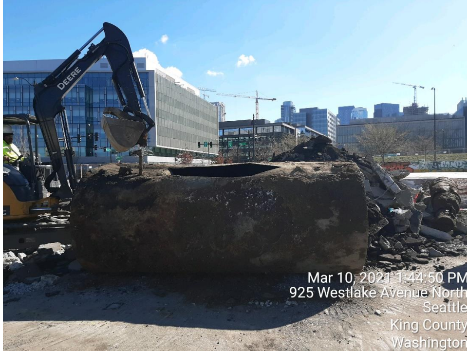
Photograph 7: UST-A removed from the ground.
