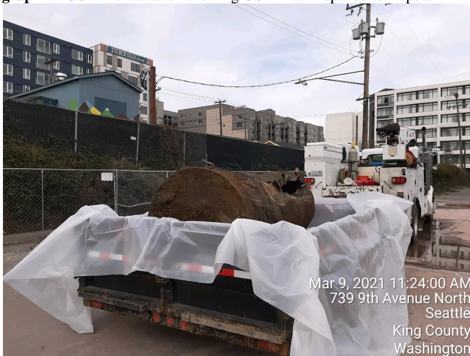
Photograph 2: UST-L removed from the excavation.
