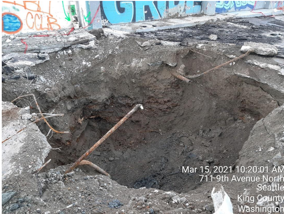
Photograph 11: Capped lines at the UST-A excavation.
