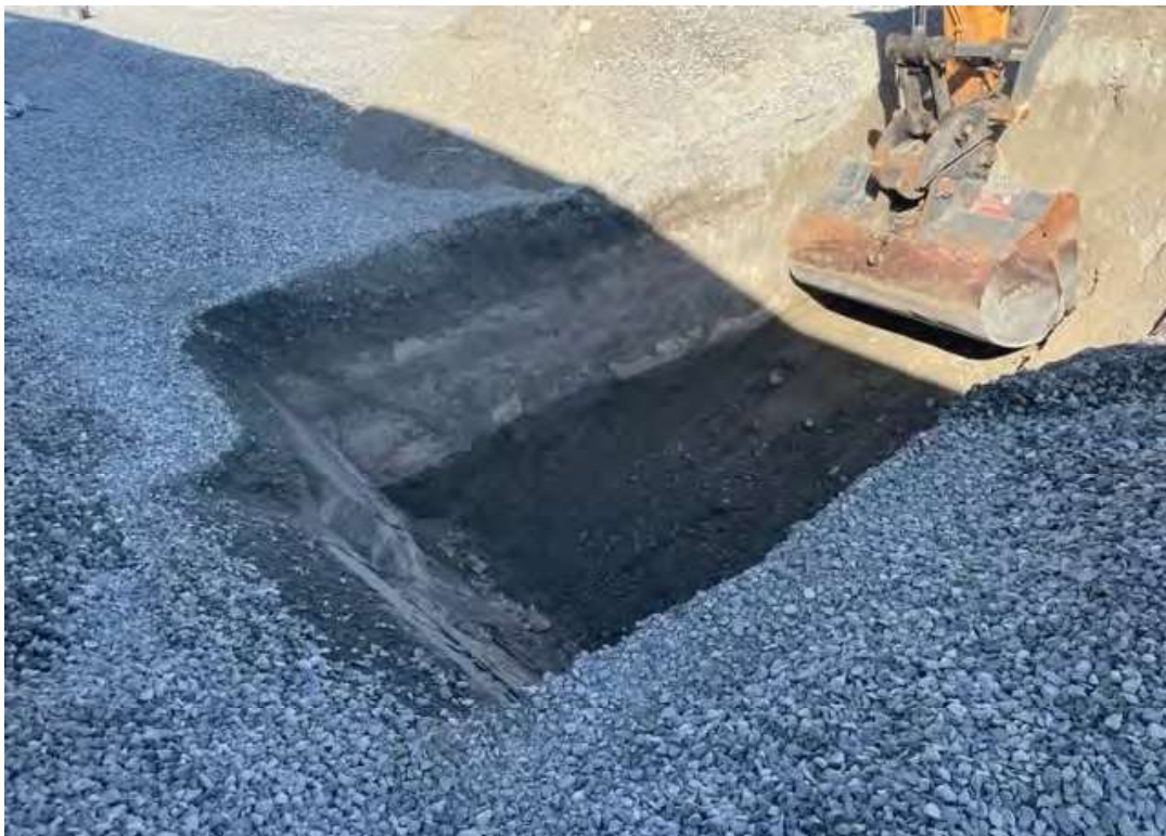
Impacted soil was removed (6)
