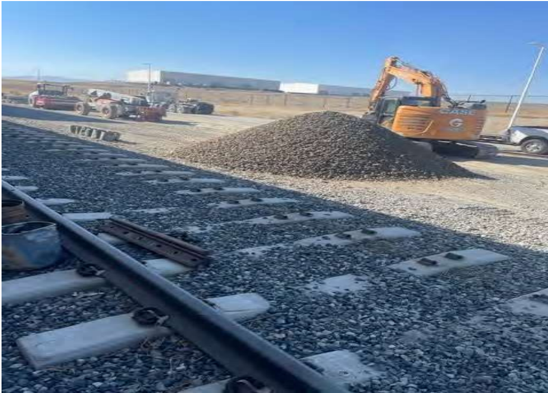
Railroad balast being spread over the site (13)
