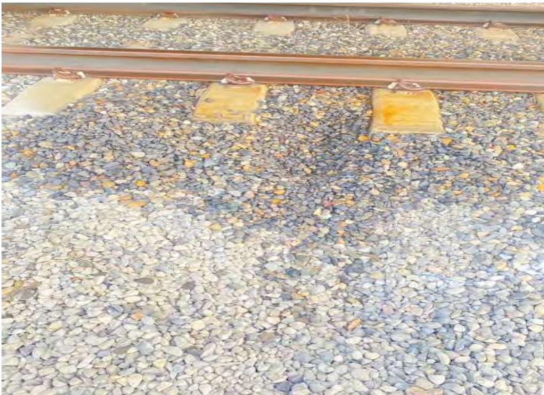
Diesel released in the ground under the tracks (2)
