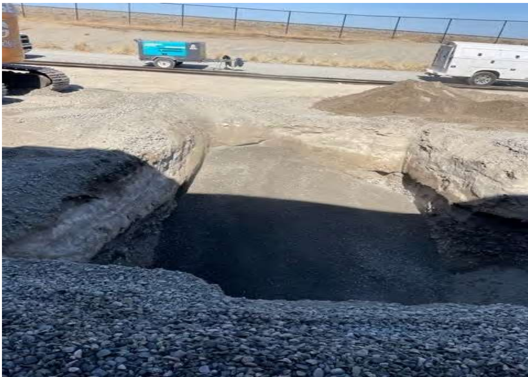
Excavated area being refilled (10)
