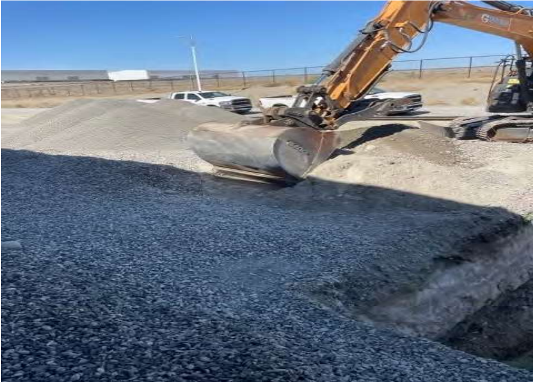
Backfill being placed in the cleared site (9)
