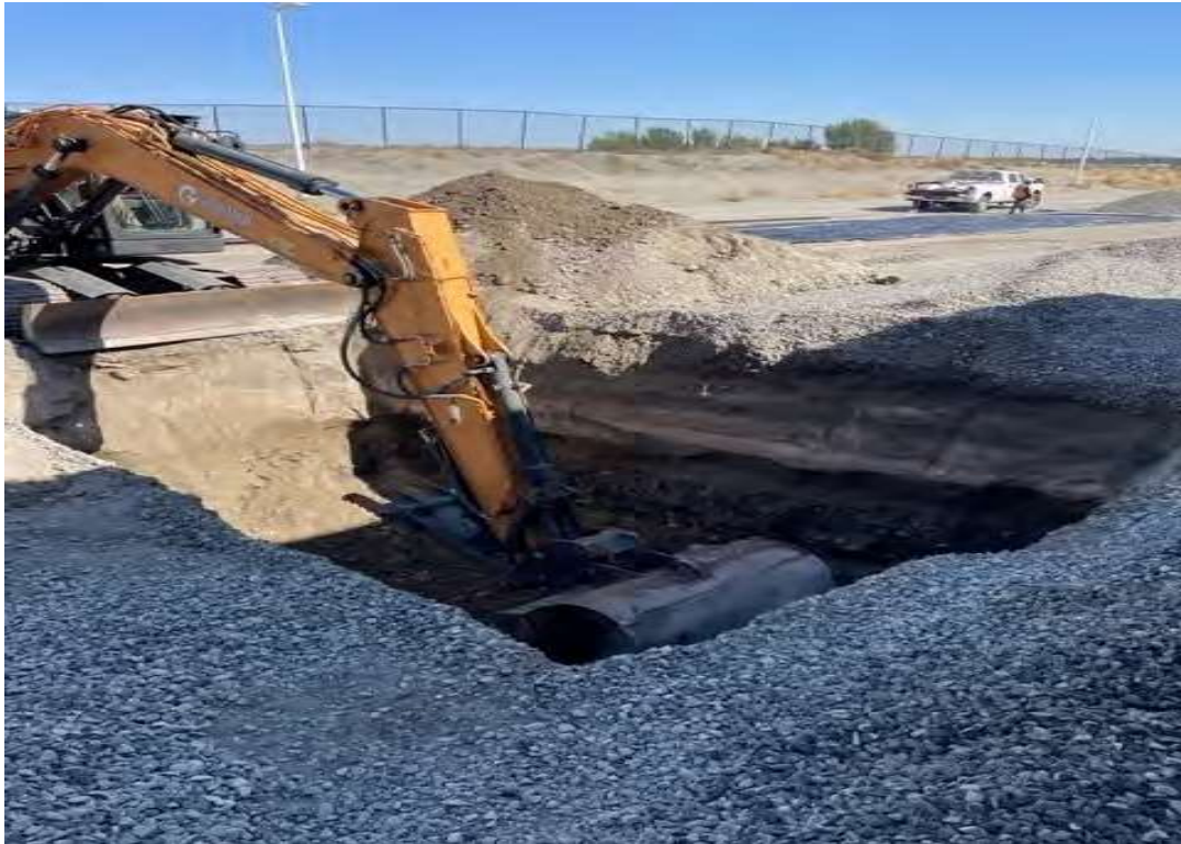
The excavation continued to clear the diesel release (7)
