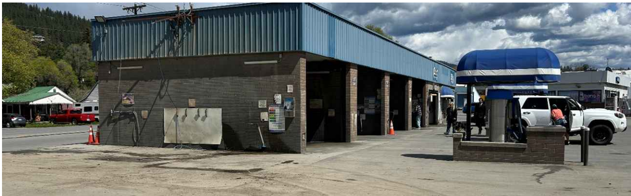
Photo 4: Looking east at the truck wash on the far west end of the carwash building. The wash bays, including the truck bay on the left, have interconnected drains that appear to lead off site.
