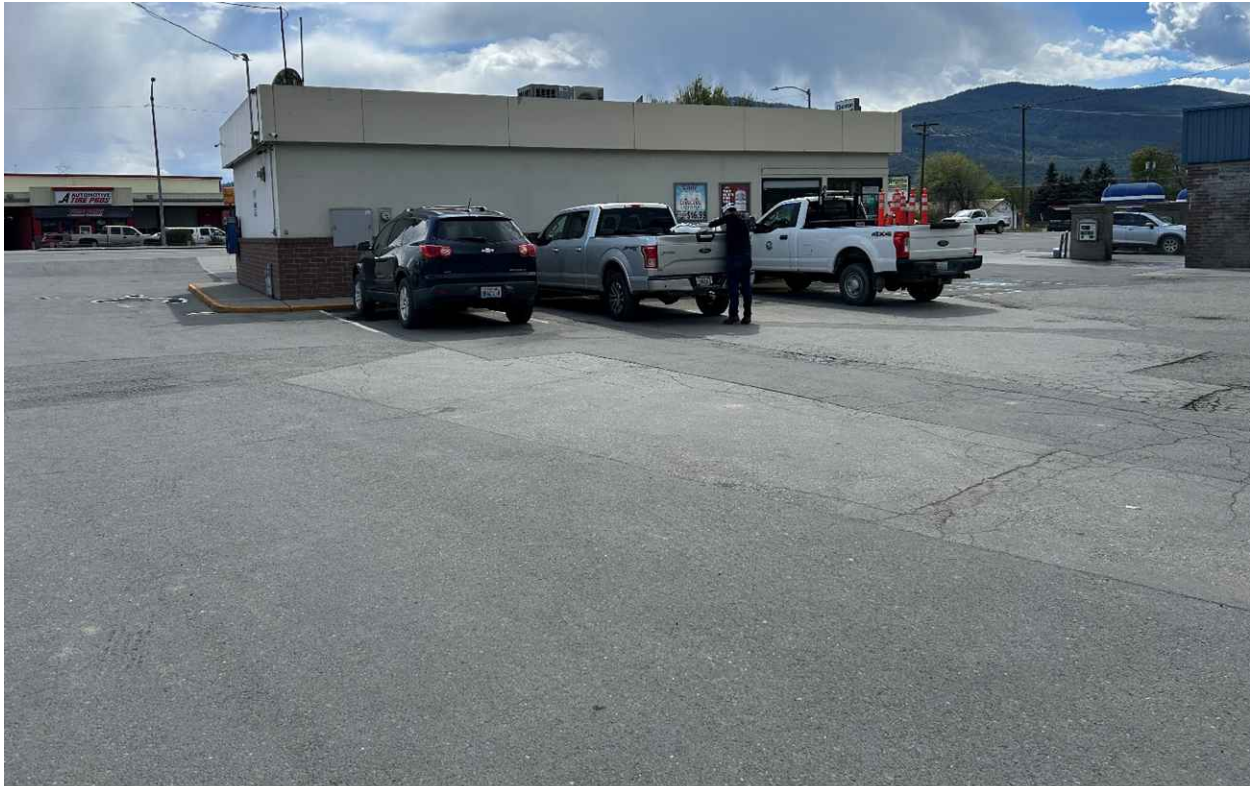
Photo 13: Looking south at the northern wall of the convenience store building. The store may be built over a closed-in-place UST, proximal to its northern wall. The pavement patches in the foreground may have been where larger USTs were located (and removed in 1989) that supported the “bulk plant” uses of the subject property in the 1950s and 1960s.
