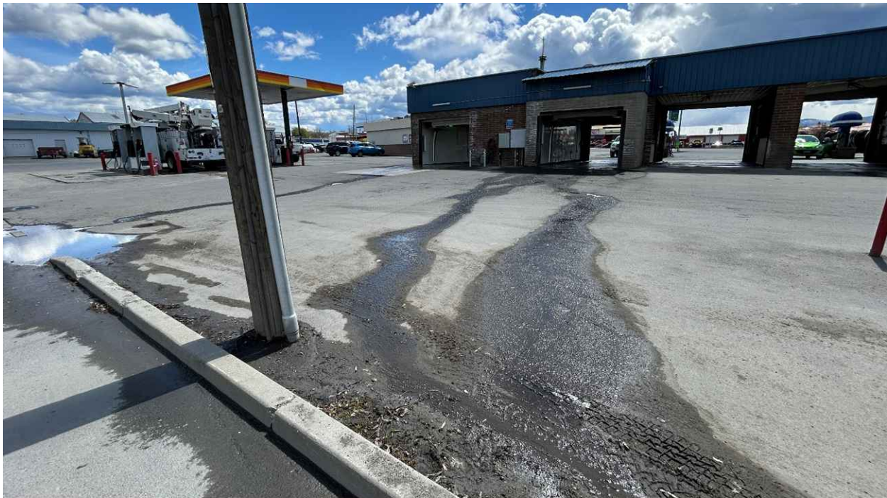
Photo 7: Looking southeast at the wash bays from along W. 6 th Avenue. The bays runoff but the water doesn't seem to leave the subject property. Left are the northern pump islands. Several pole-mounted transformers were observed nearby that did not appear leaking.
