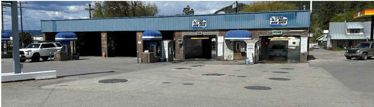
Photo 3: Looking north at the UST nest onsite (1989). There are two diesel tanks here and two gasoline tanks. The carwash facility rests in the background (1987).
