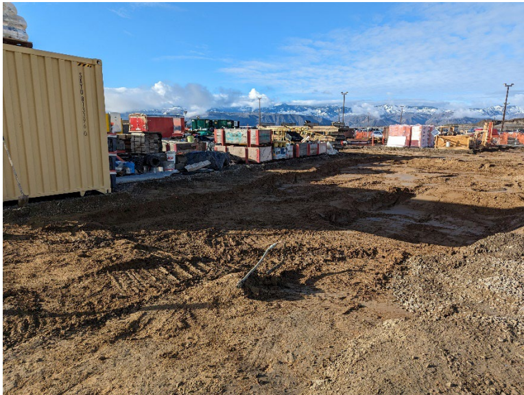
The spill occurred in a graveled area. About 1-foot of impacted gravel and soil was removed throughout the remedial excavation.
