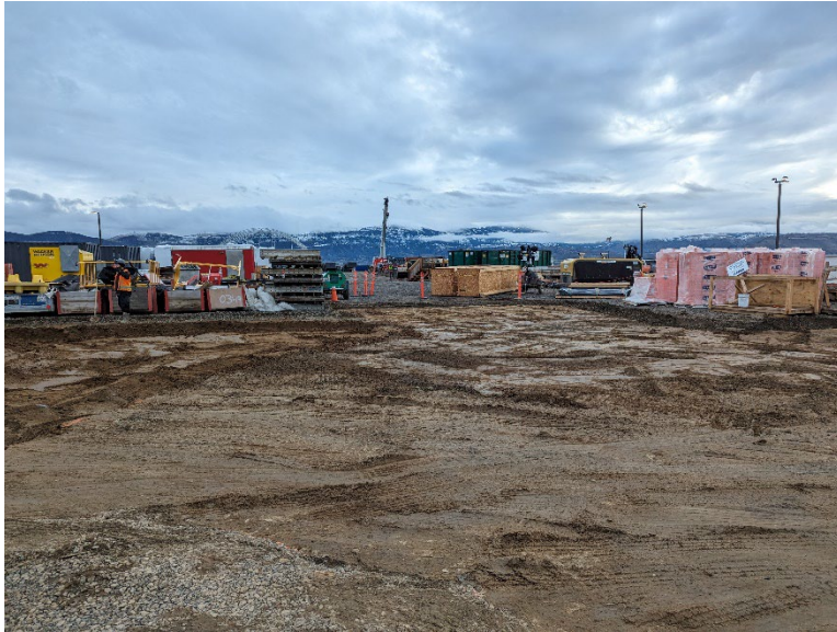
The diesel spill occurred in a construction laydown area. Gravel was removed and underlying soil was field screened for diesel impact.
