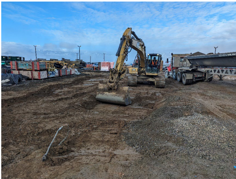
Petroleum impact was observed to extend to a maximum of 3-feet bgs in the east portion, in the vicinity of where the spill occurred.
