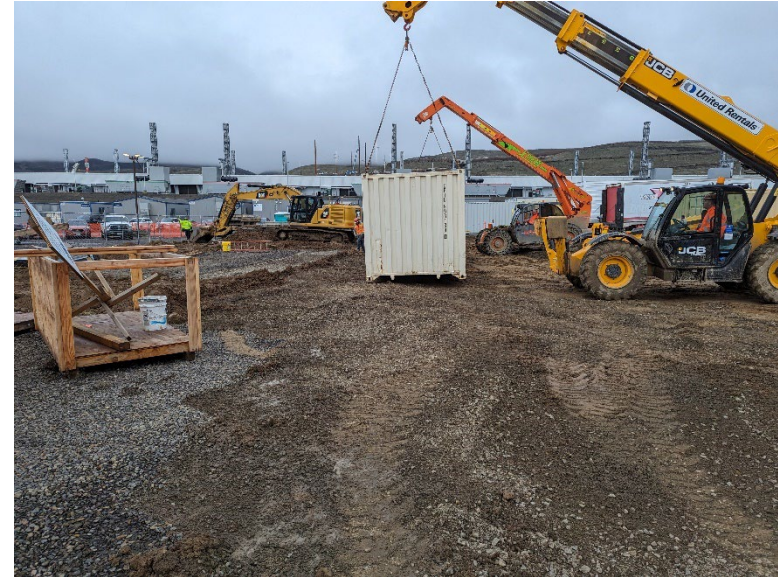
The spill occurred while fueling a portable fuel tank from a tanker truck. Storage containers were relocated to access soils.
