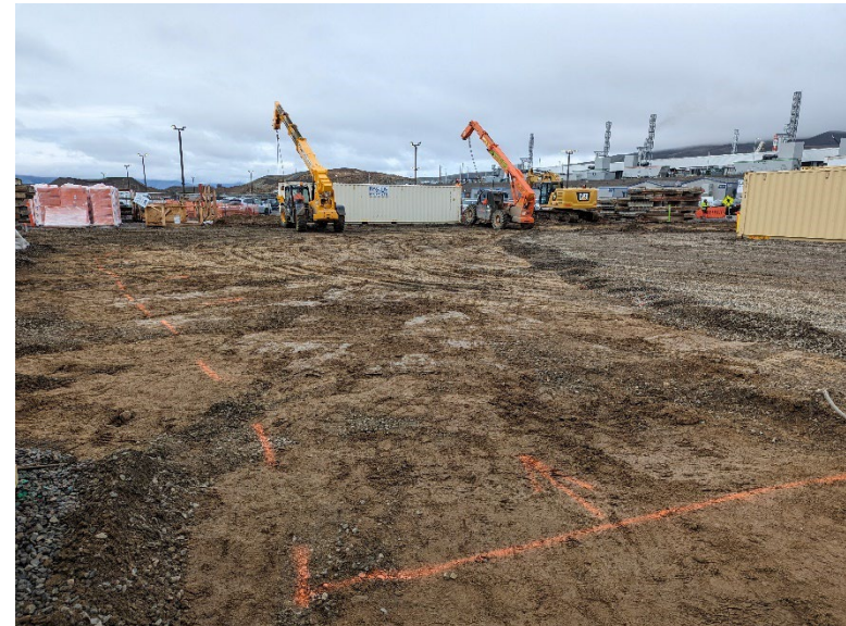
An area of impacted soil was delineated with pink construction paint prior to excavation.
