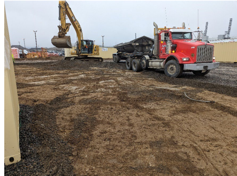
All soil exhibiting field screening indications of petroleum impact was excavated for disposal at Greater Wenatchee Landfill.
