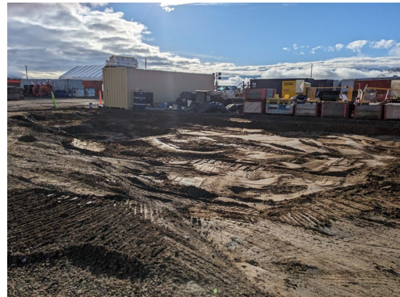
View of the final excavation looking southeast. Laboratory analytical determined all petroleum impacted soil was excavated.
