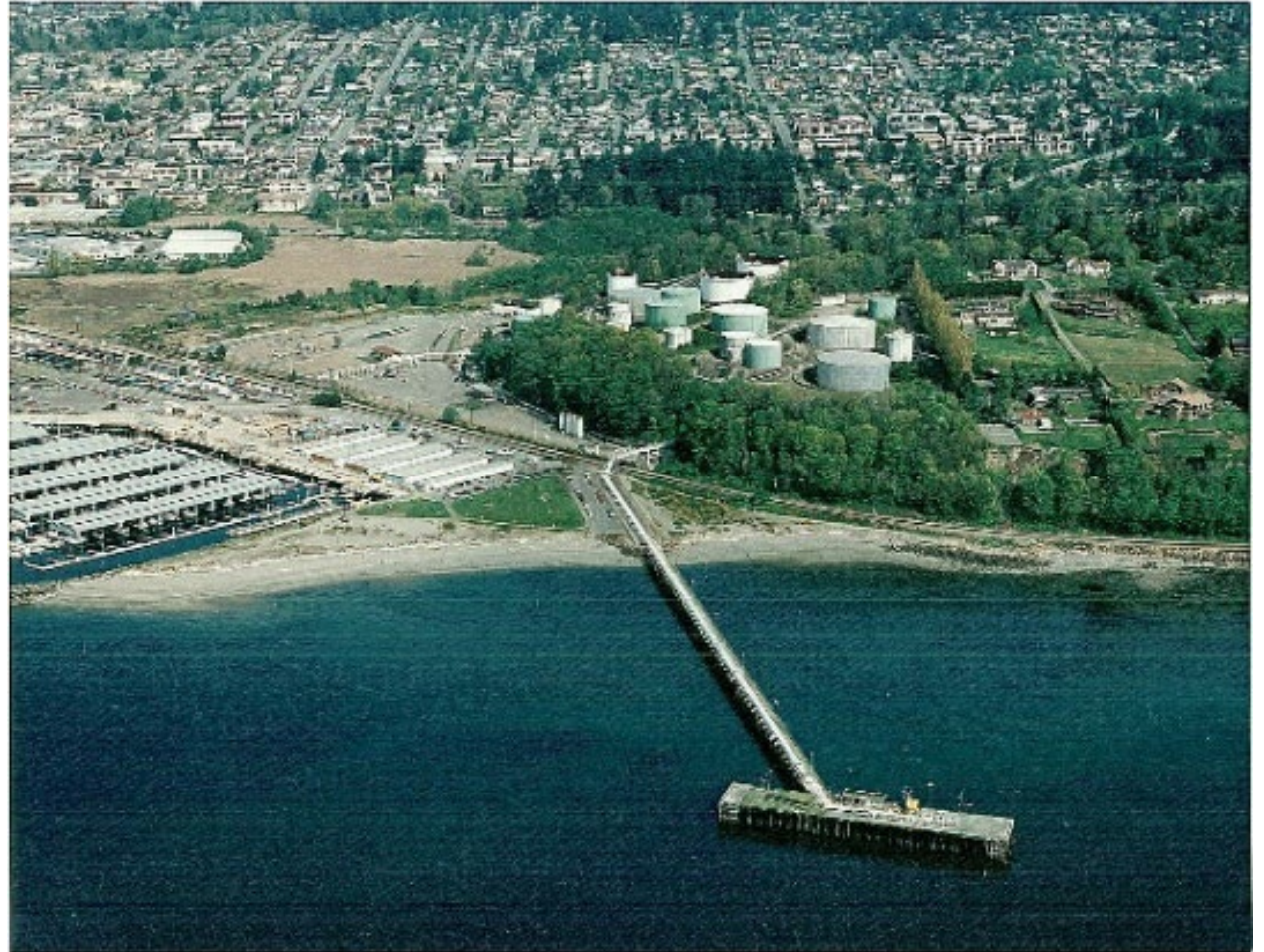
Historic view of fuel terminal
