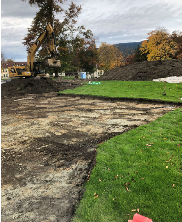
1: Overexcavation in former ward building area looking northeast.
