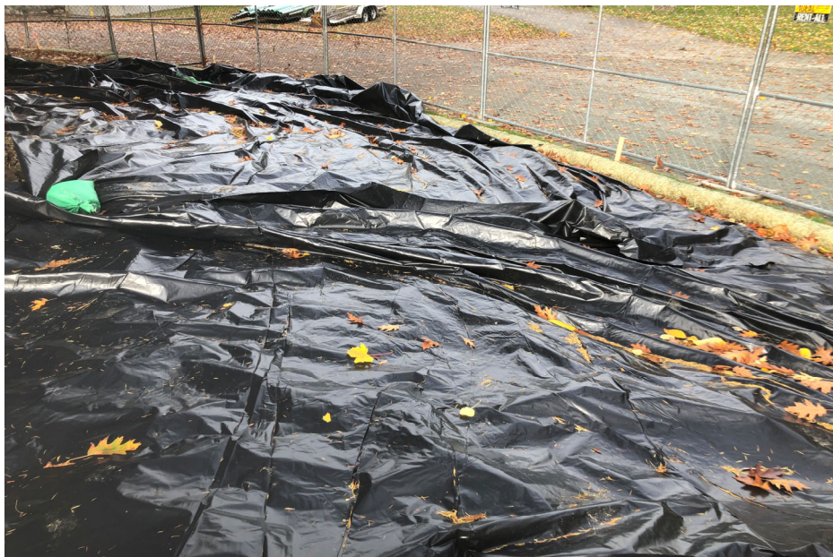
2: Hand tool excavation covered with plastic sheeting looking north.
