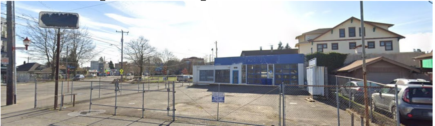
C L Auto Repair Cleanup Site (photo courtesy: Google Maps)
