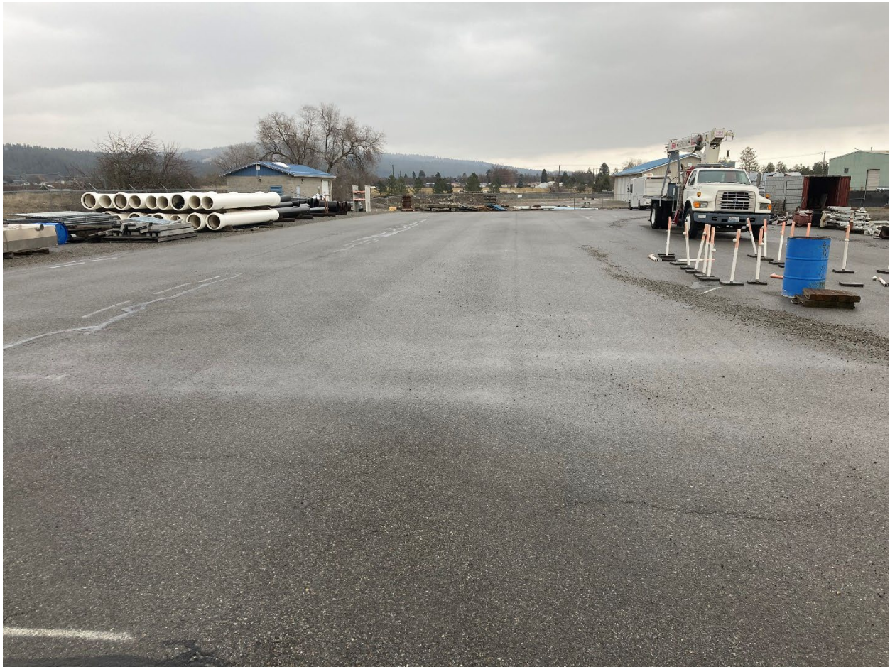
Photo 3: The capped area with vehicle and equipment storage, from the west
