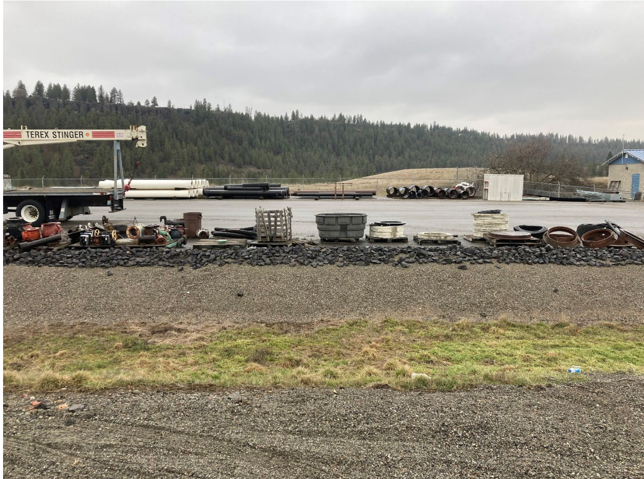
Photo 1: The drainage swale and asphalt cap, from the south
