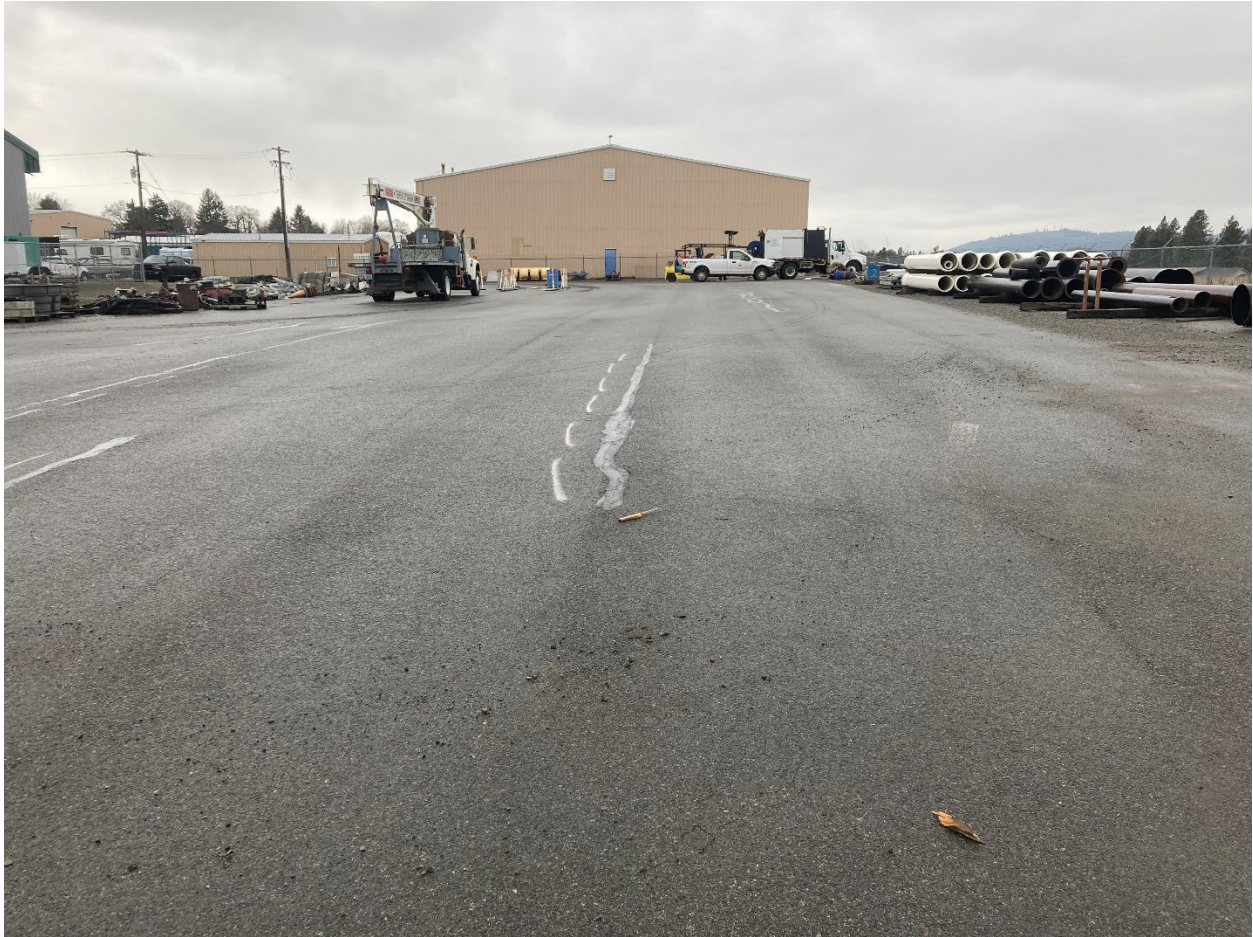
Photo 2: The capped area with vehicle and equipment storage, from the east
