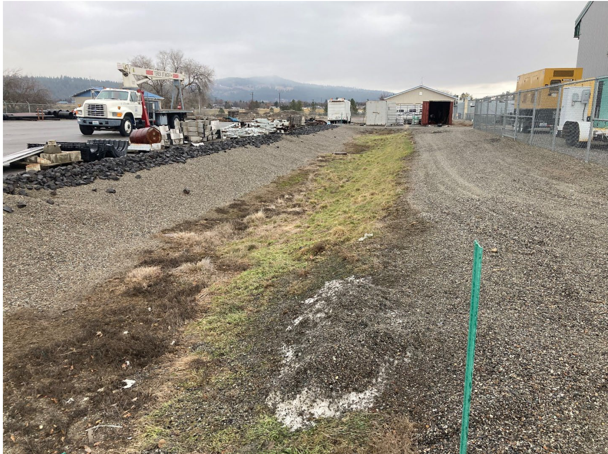
Photo 4: The drainage swale with adjacent gravel and asphalt surfaces, from the west
