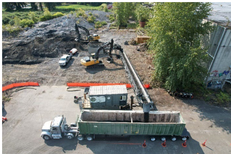
Figure 5: Dross pile removal progress (2023)
