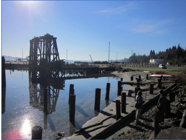
Photo 1: 2012 photo of Mill Site prior to clean up and removal of loading pier. Photo credit: J. Krausmann, USFWS.
