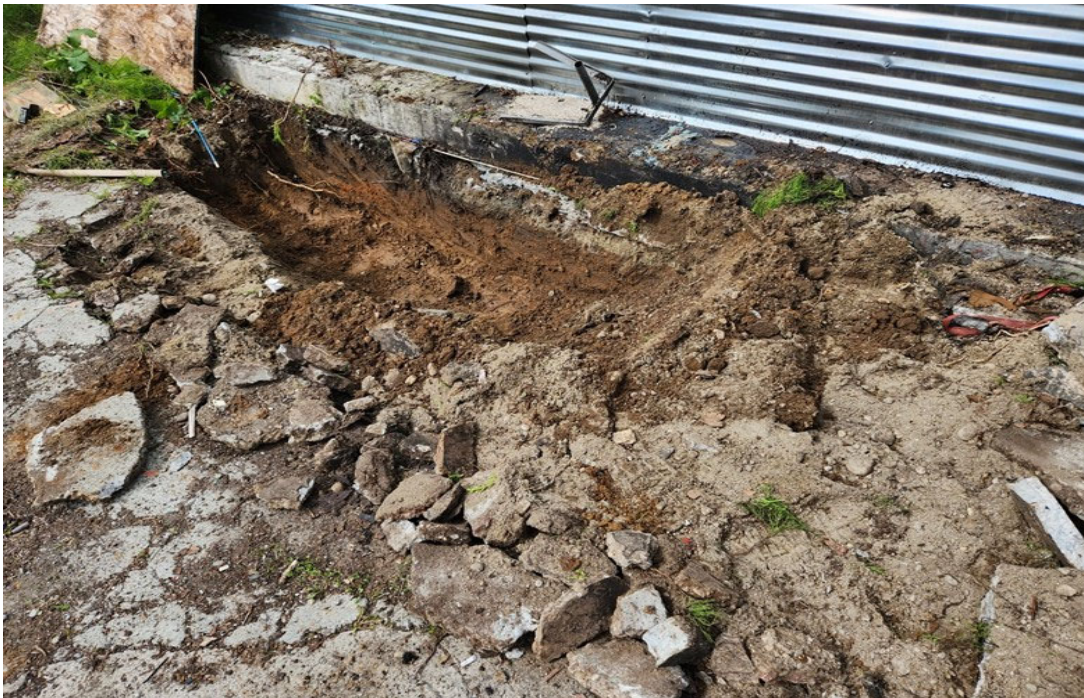
8. AOC B during Excavation
