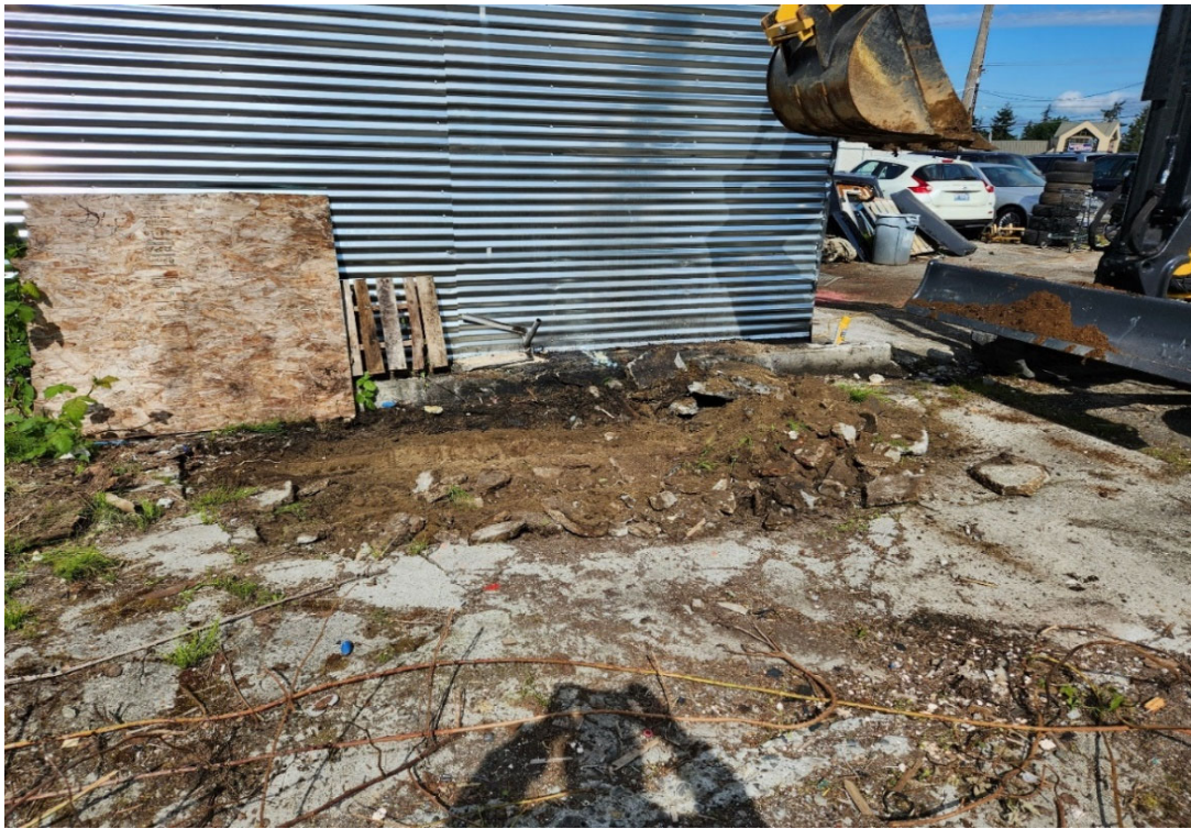
7. AOC B stained area excavation
