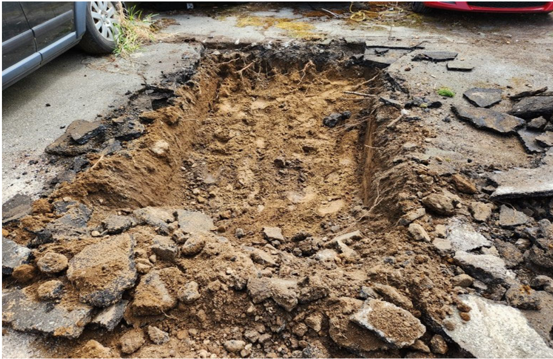
5. AOC A Excavation
