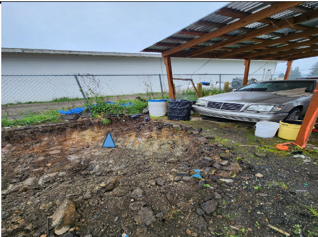
11. AOC C excavation in previously document shallow "hotspot" as indicated by blue triangle.
