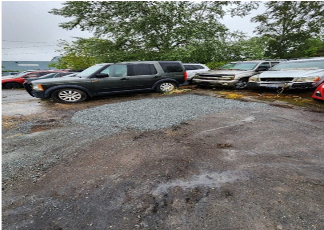
6. AOC after excavation and backfill with gravel
