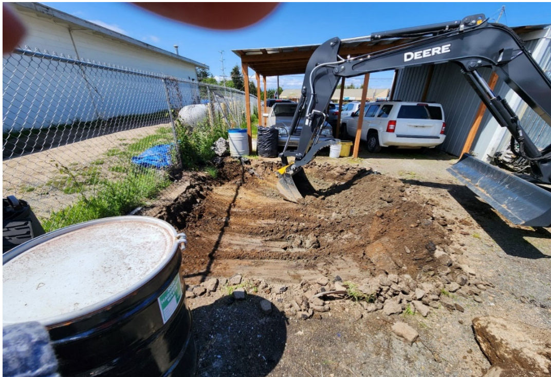
10. AOC C during excavation
