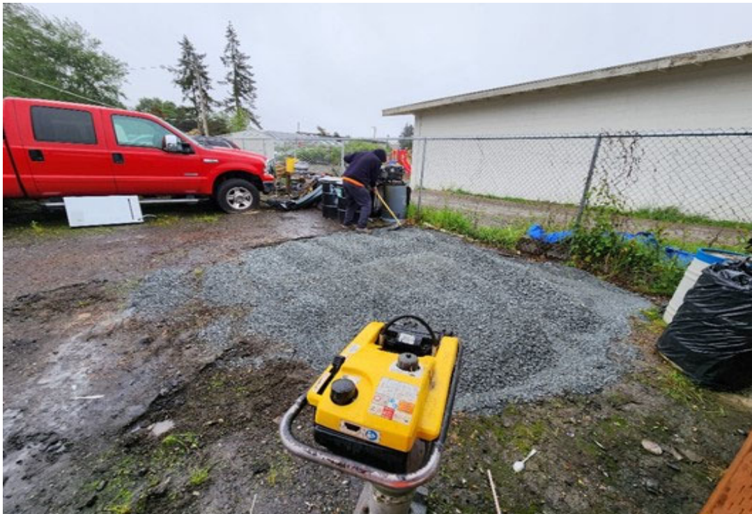
12. AOC after excavation and backfill with gravel
