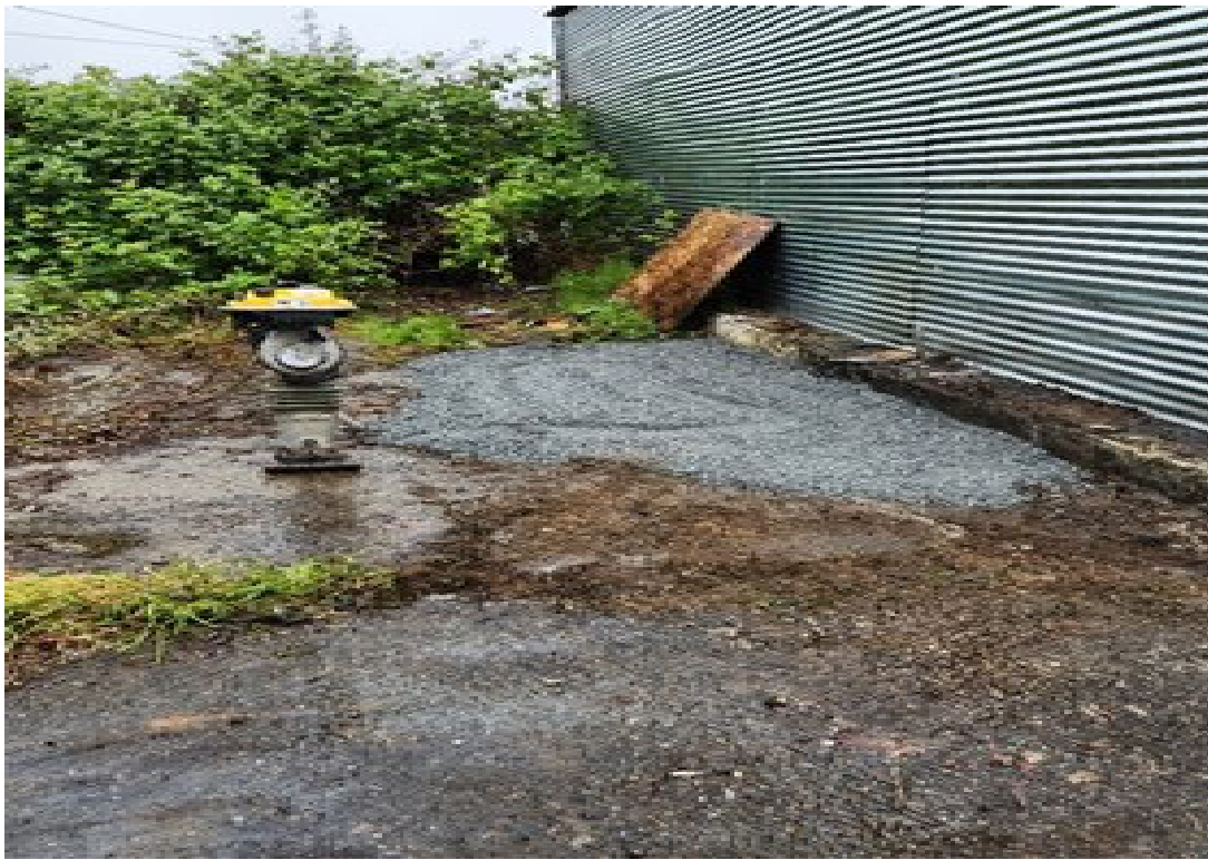
9. AOC B after excavation and backfill with gravel
