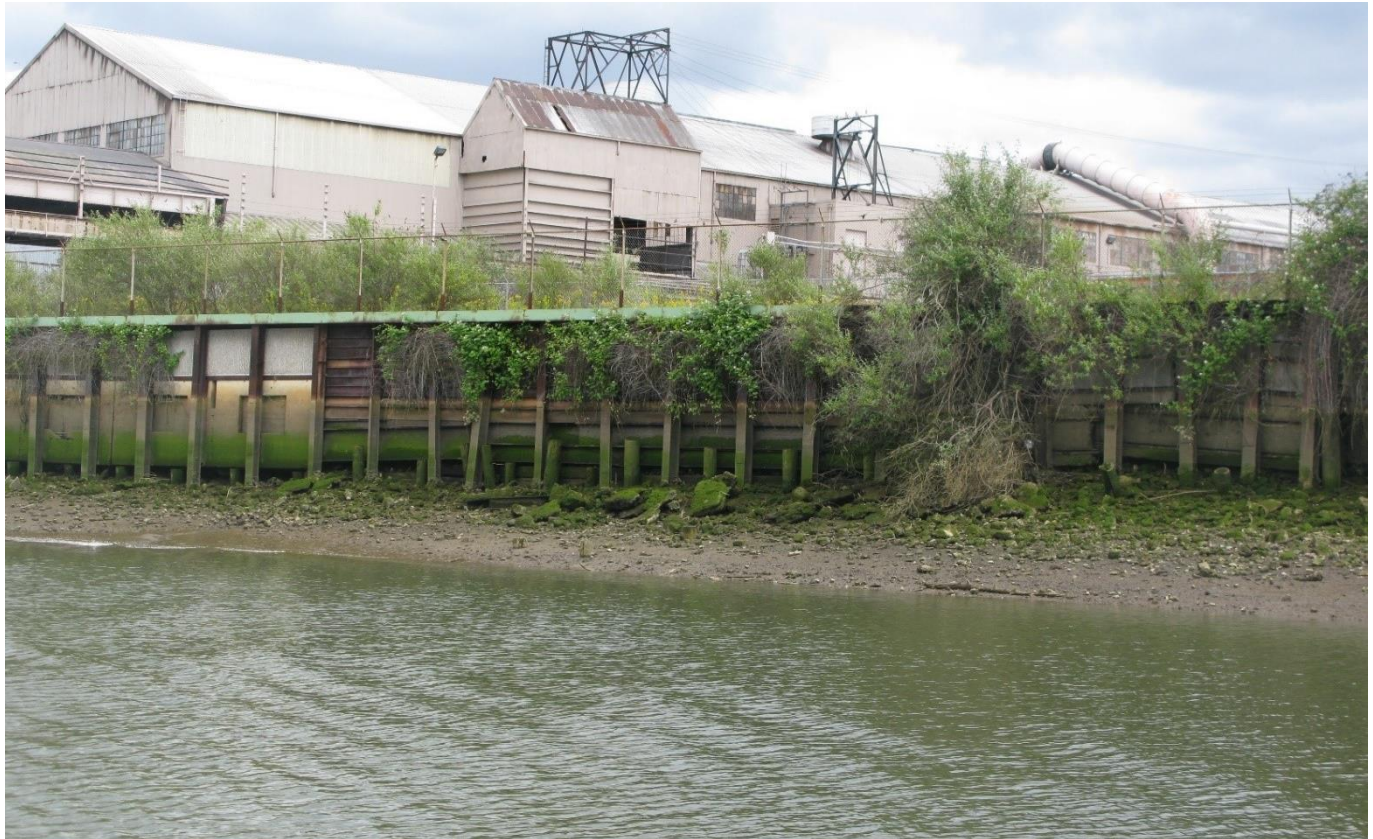
Port of Seattle 物业北侧的木质挡土墙
