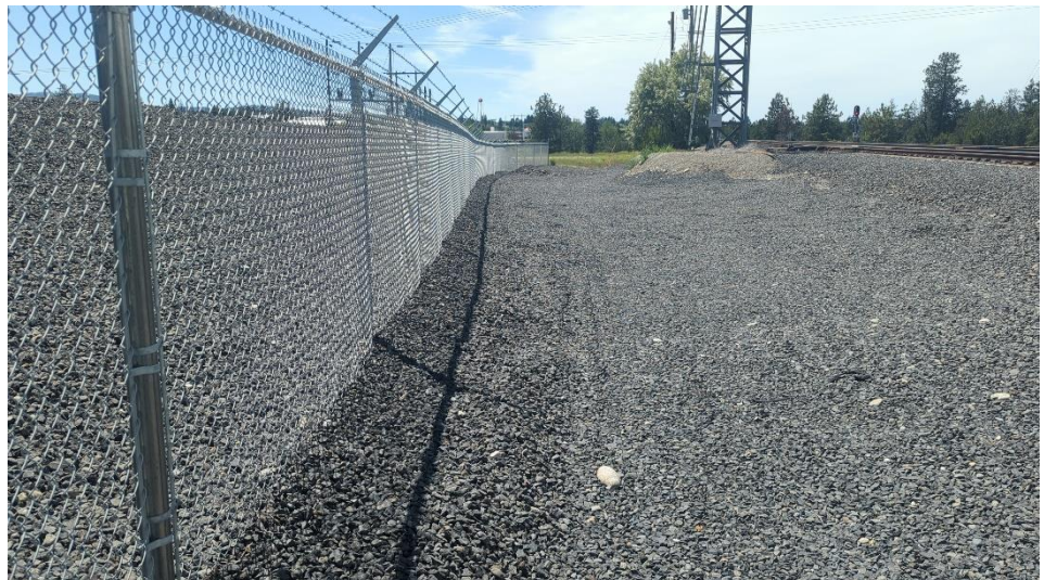
Railroad ditch overview. View looking west.
