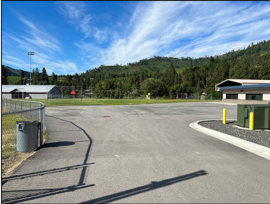
Photo 1: Peshastin Dryden Elementary School (view to the south)
