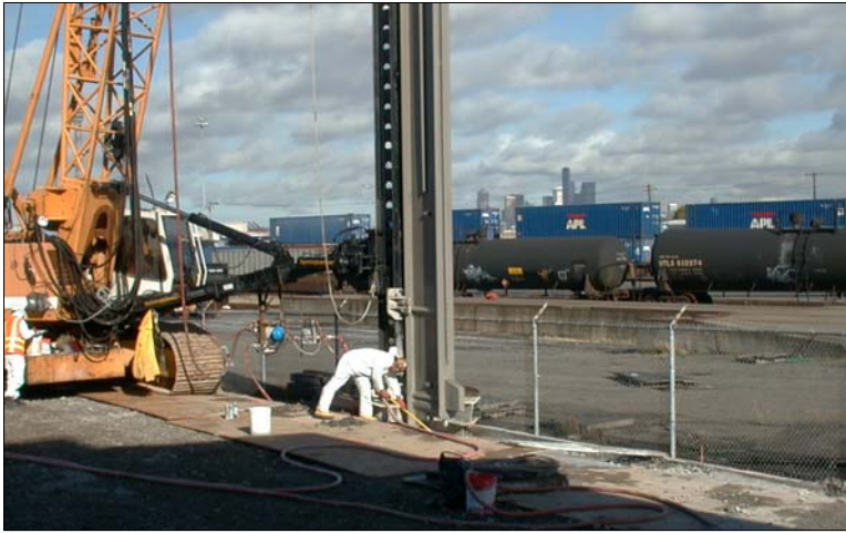
Phase 2 cleanup using bioremediation and extraction pumping to remove petroleum from groundwater and saturated soils in July 2001.
