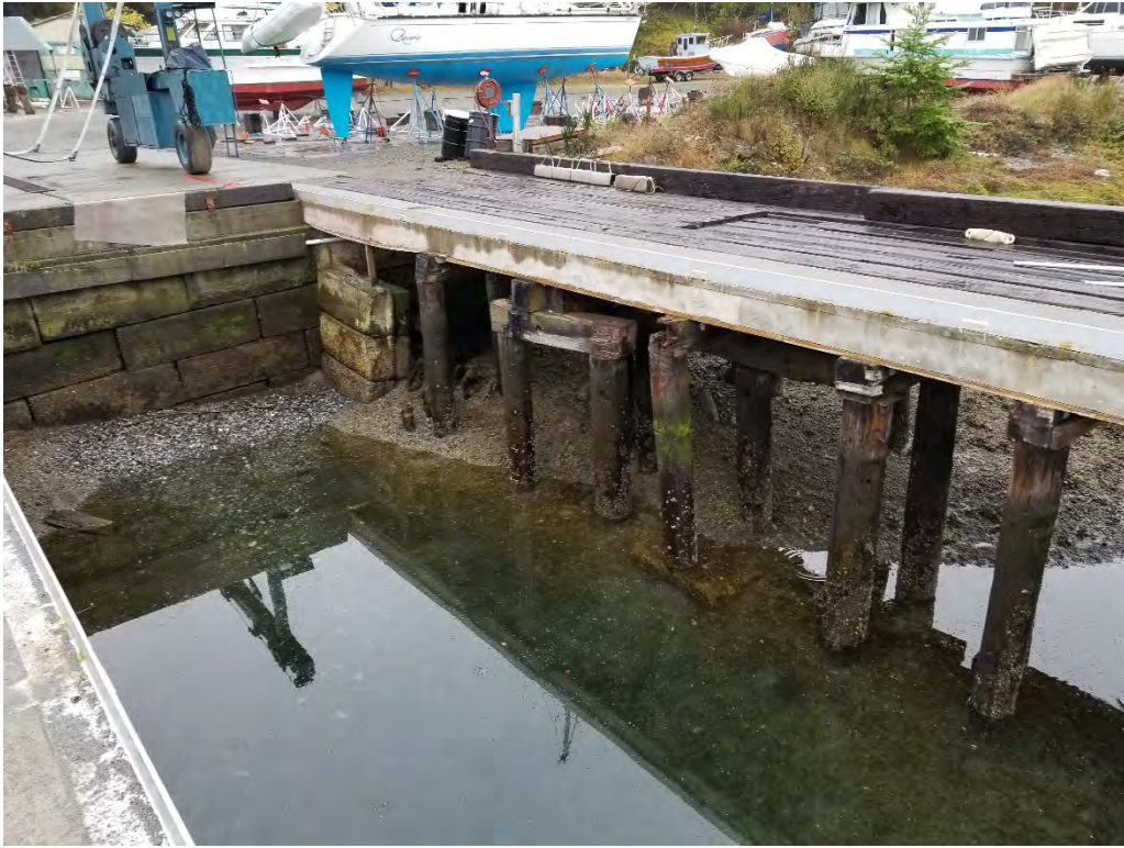
Photograph 13. Concrete ecology block bulkhead inside of the boat haul-out.
