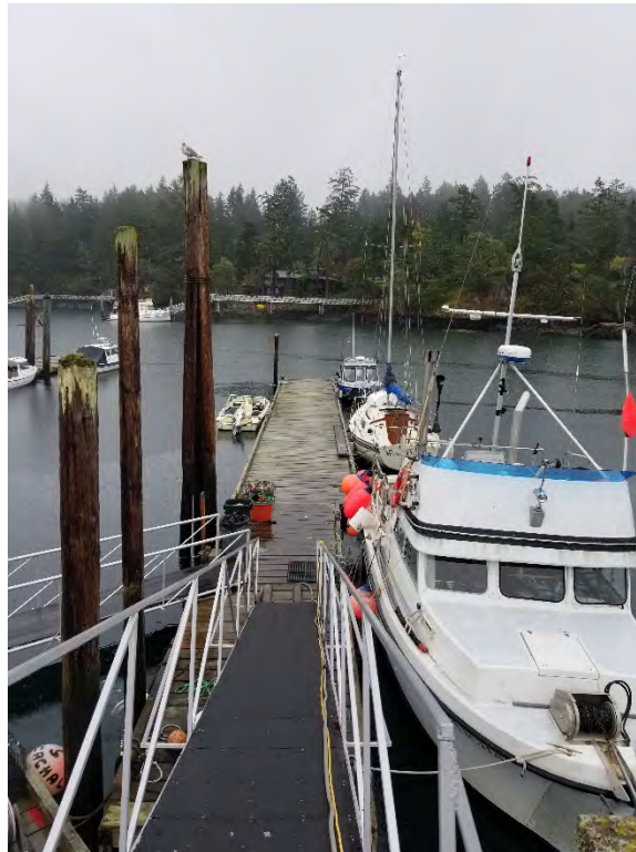
Photograph 8. Close up of solid surfaced gangways.
