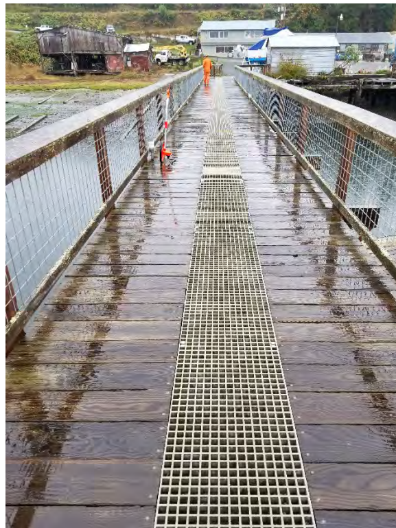
Photograph 2. Close-up of marina pier surfacing.
