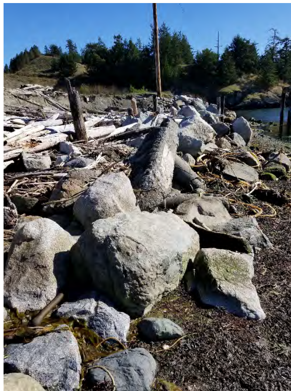
Photograph 4. Close up of concrete debris and creosote-treated piles among driftwood.
