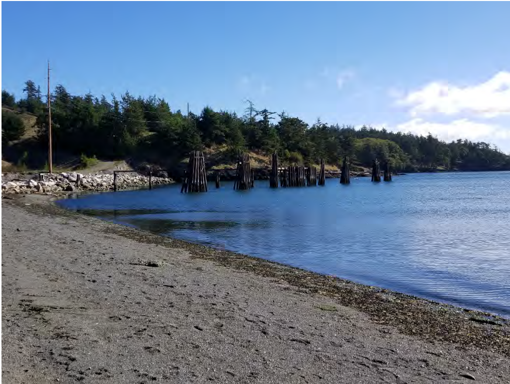
Photograph 3. Defunct barge landing with creosote piles, concrete debris.
