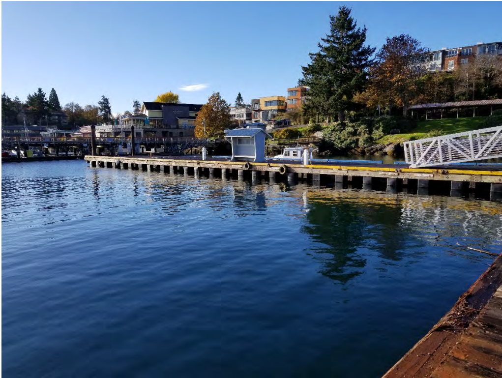
Photograph 3. Load dock with solid timber surfacing, tire bumpers, and creosote-treated pilings at the end of the dock.
