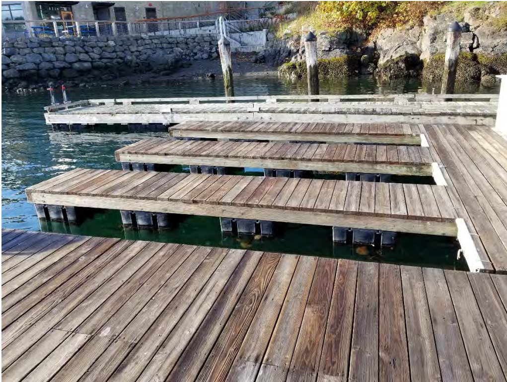
Photograph 7. Solid surfaced treated wood floats off of the Fuel Pier, creosote-treated piles, rock debris from retaining wall spilled on the pocket beach.
