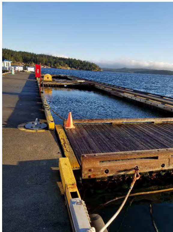
Photograph 2. Seaplane float and Breakwater C with solid surfacing.
