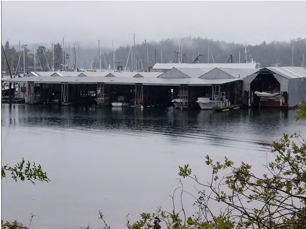
Photograph 5. Covered boat houses with solid roofing.
