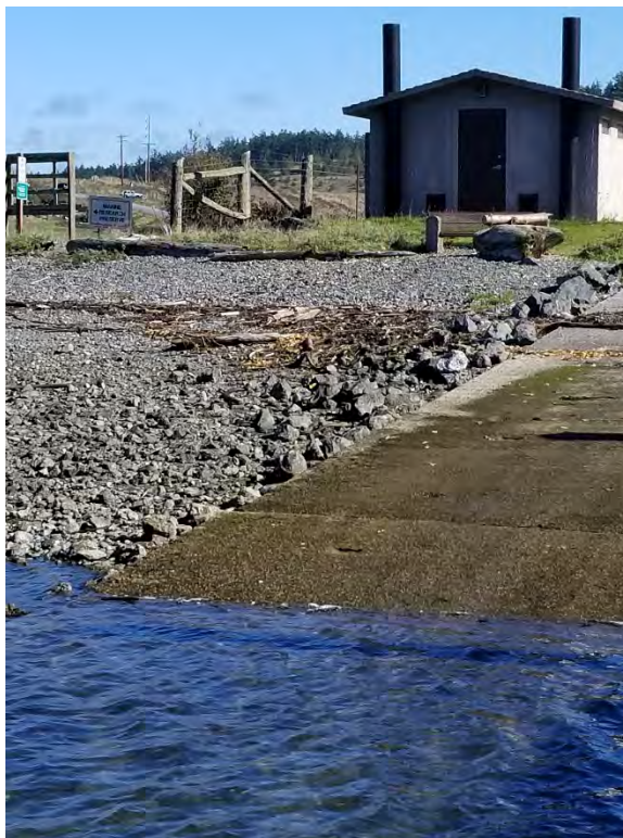
Photograph 6. Concrete boat ramp and adjacent angular rock.
