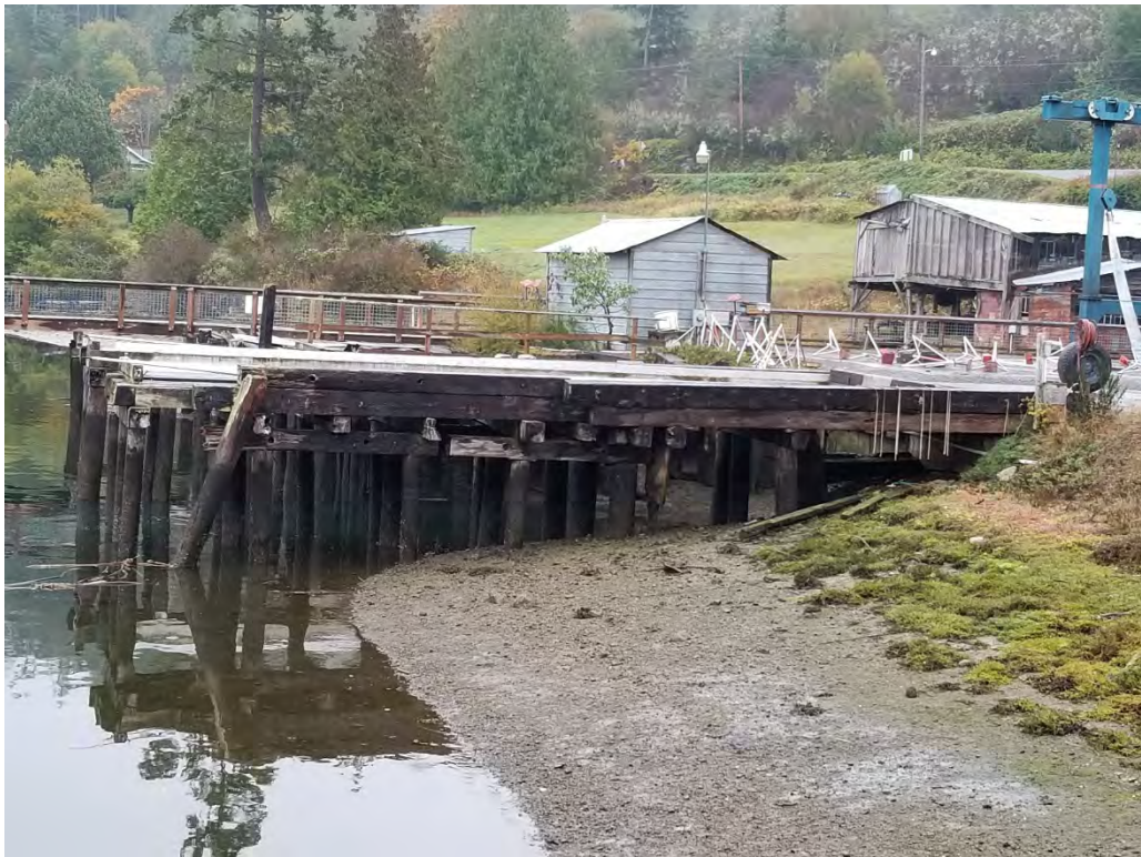
Photograph 12. The solid-surface boat haul-out structure, supported by creosote-treated pilings.
