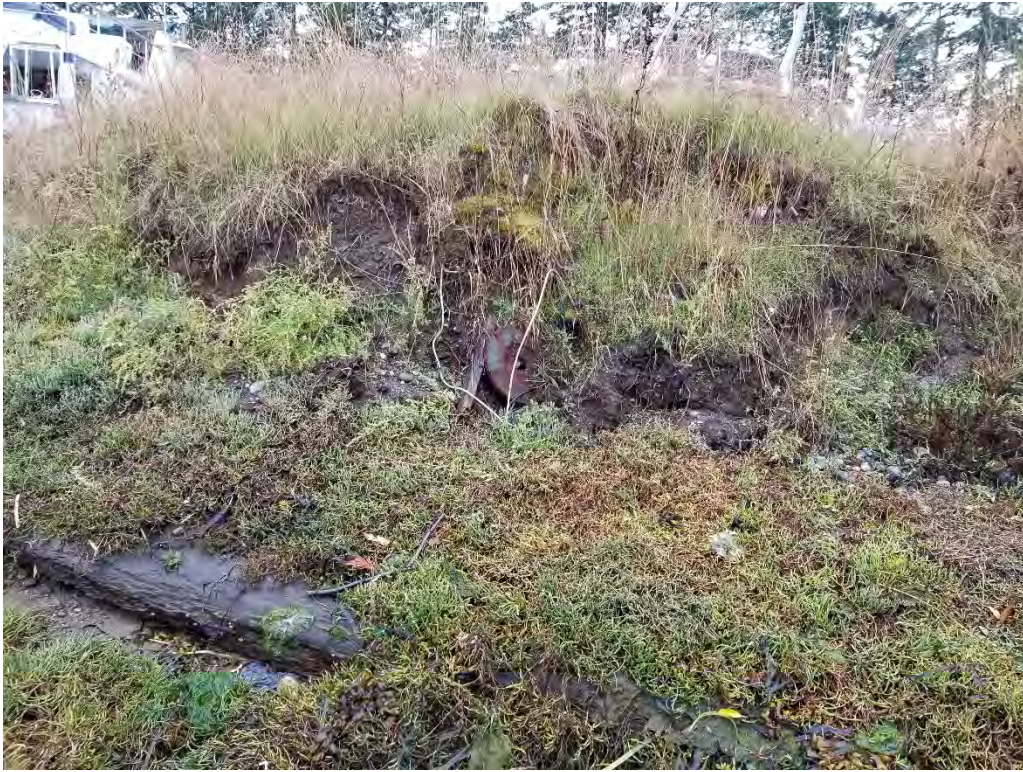
Photograph 11. Close-up of berm between the bulkhead/fill area and the boat haul-out.
