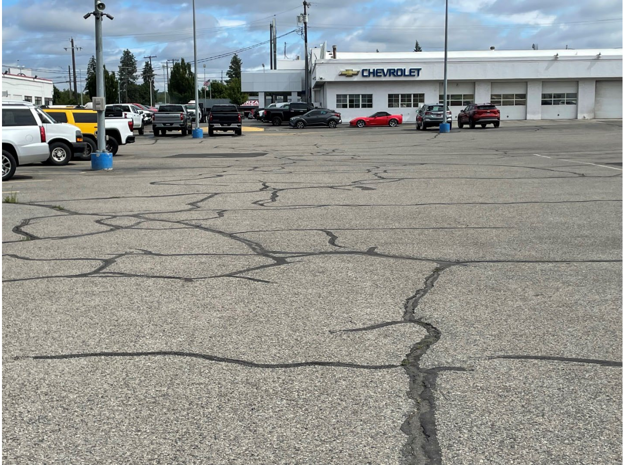
Photo 1: Appleway Chevrolet capped area of contamination – from the south
