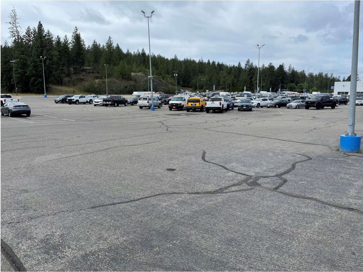
Photo 3: Appleway Chevrolet capped area of contamination – from the northeast
