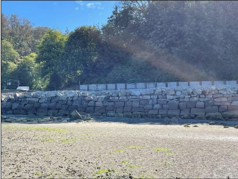
Photograph 36. Southern shoreline conditions near Pigeon Creek in Area B; typical. Vertical rock wall supporting the adjacent railroad tracks, facing South.
