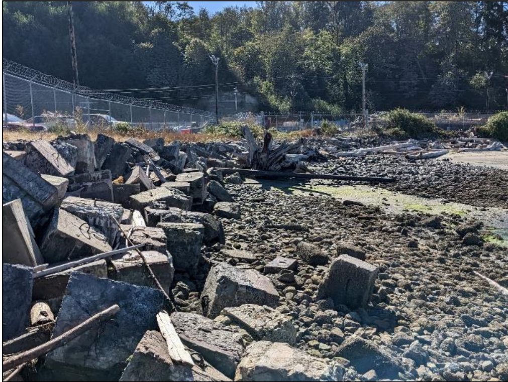
Photograph 32. Armored slopes of the southern shoreline in Area A north of Pigeon Creek. Large concrete blocks facing South.
