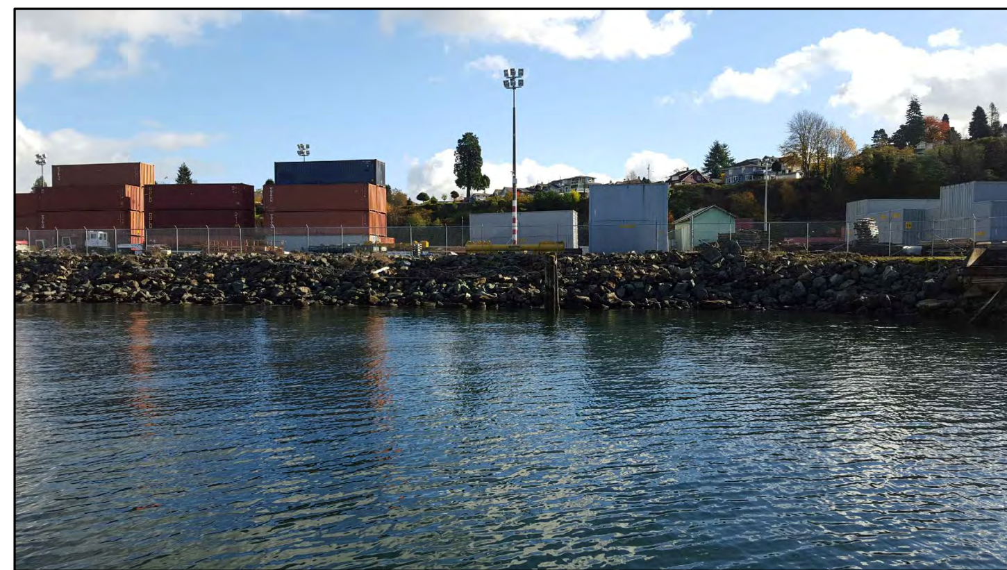
VIEW OF SOUTH TERMINAL SHORELINE LOOKING SOUTHEAST 4 3
