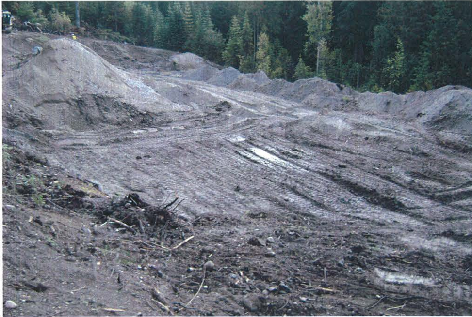
9. Staging of soils to be compacted in repository
