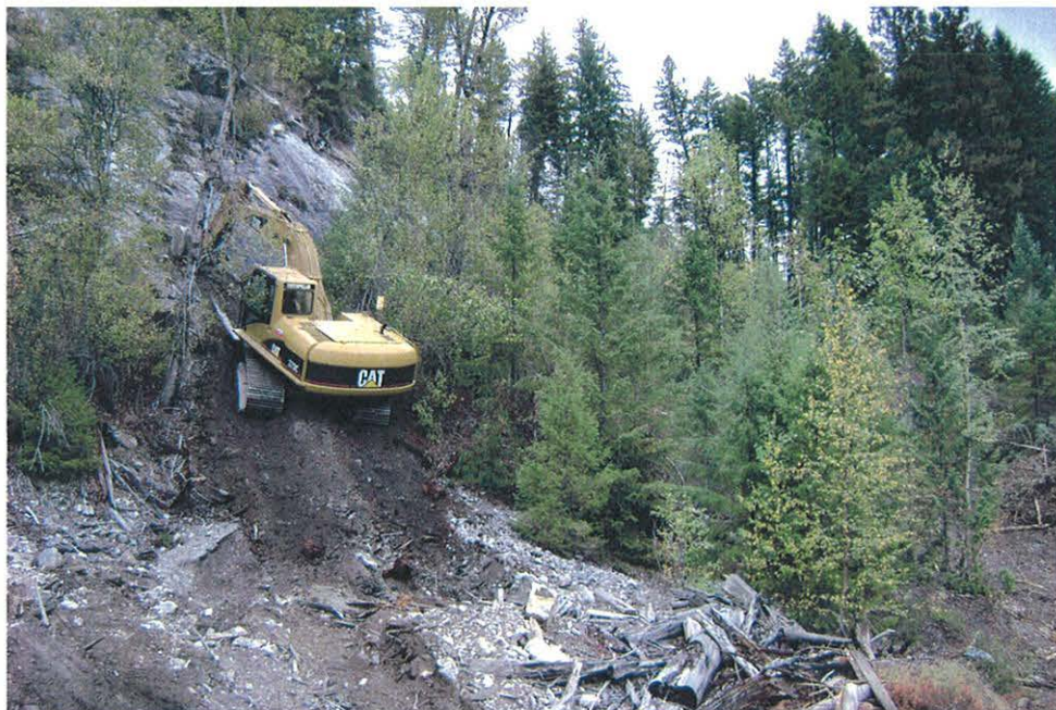
8. Removal of soils near foundations of Mill.
