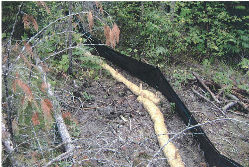
2. Installation of BMP prior to soil movement
