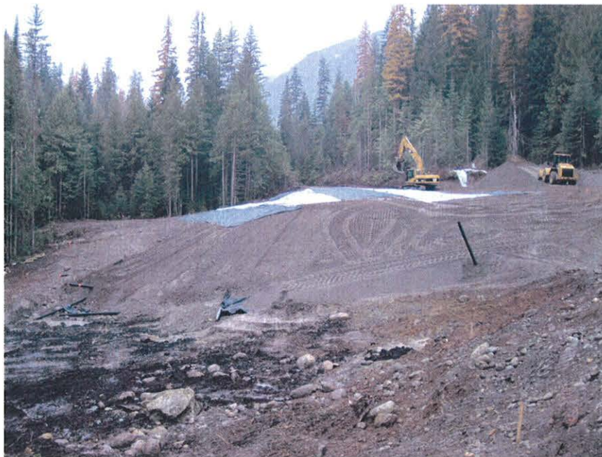
12. Repository prior to membrane installation
