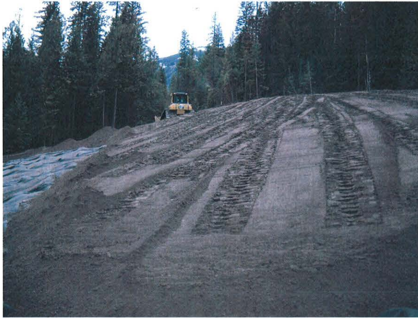
15. Cover soil being applied on repository
