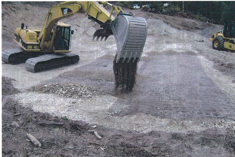
6. Repository area geogrid base
