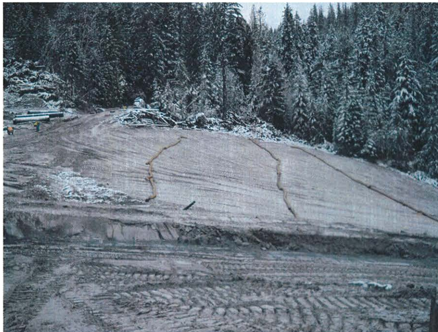
16. Removal area graded and backfilled
