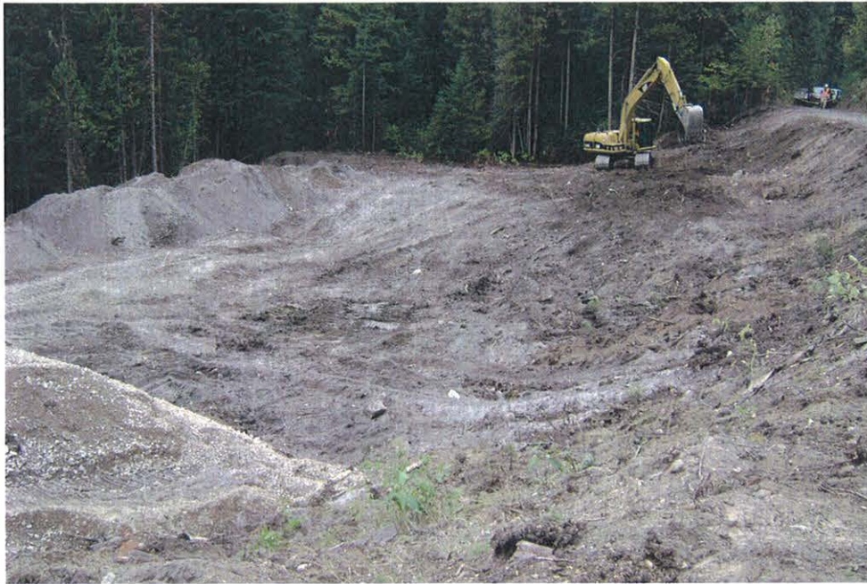
5. Cleared base of the repository area
