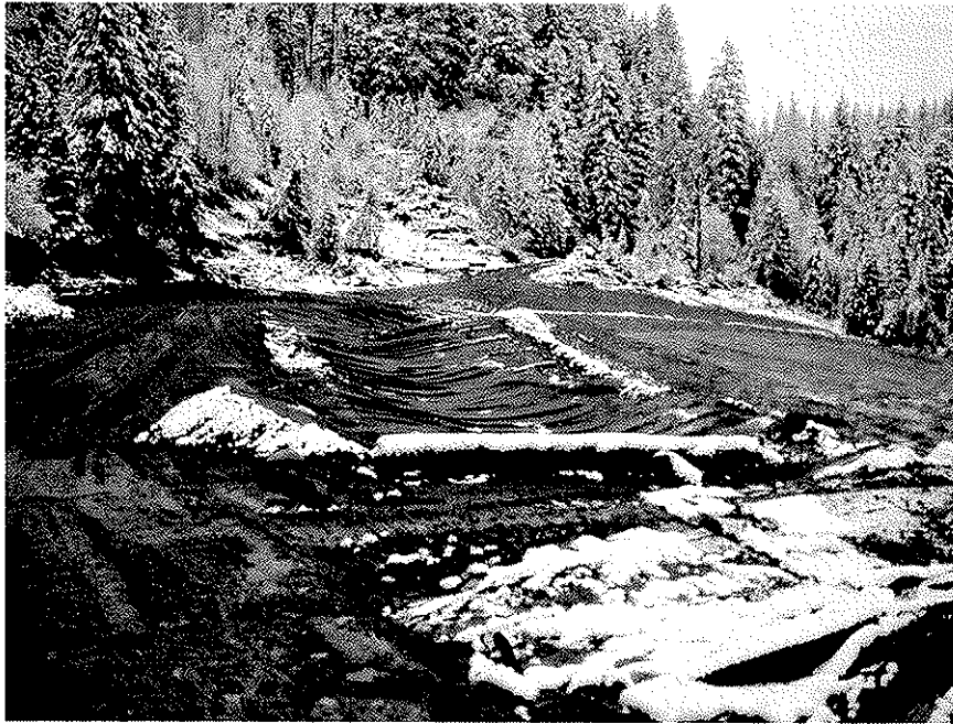
17. Repository cover soils in place
