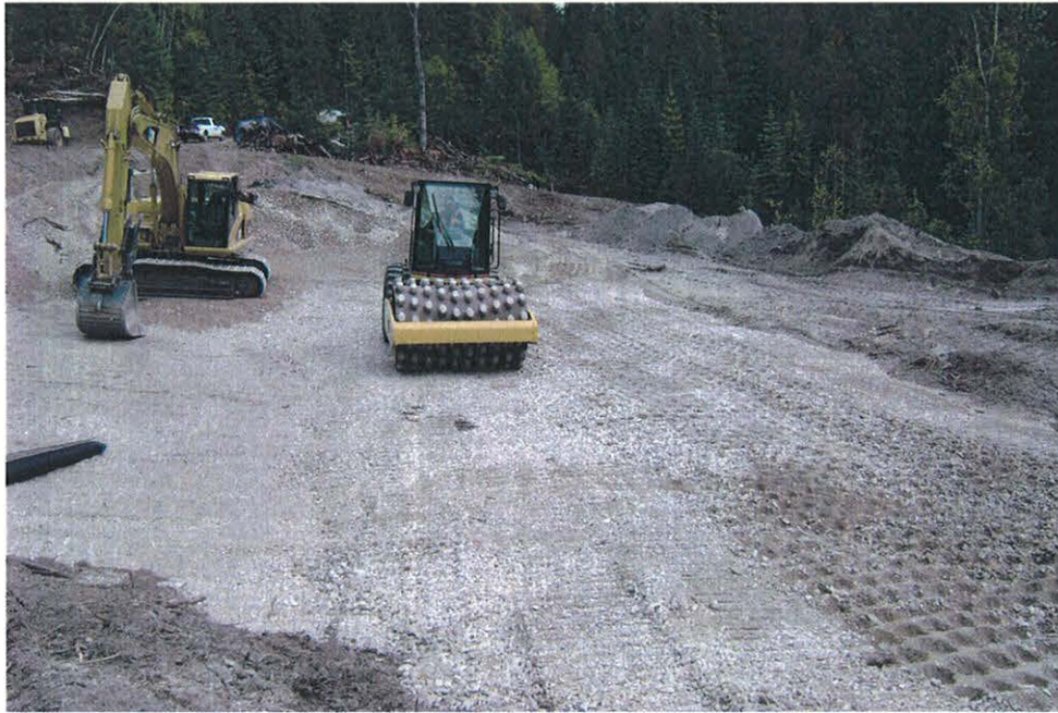
7. Compaction of repository lift
