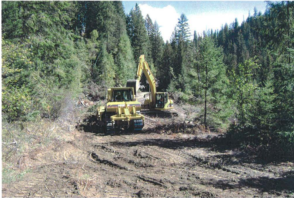
1. Mobilization to site and initial site clearing
