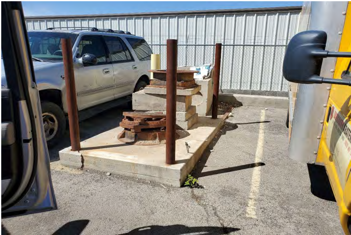
WELL LOCATED BEHIND CONCRETE FOOTING
