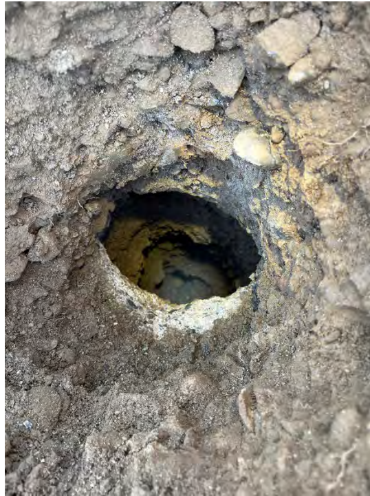
Photograph 9. Concrete present during use of airknife (B-12).
